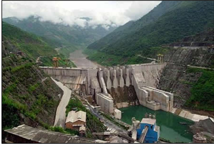
Figure 1: Mekong Dam in China's Yunnan Province
