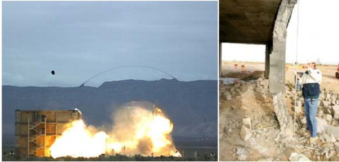
Figure 9. Testing of structural columns in multi-story office buildings to exterior blast effects.
