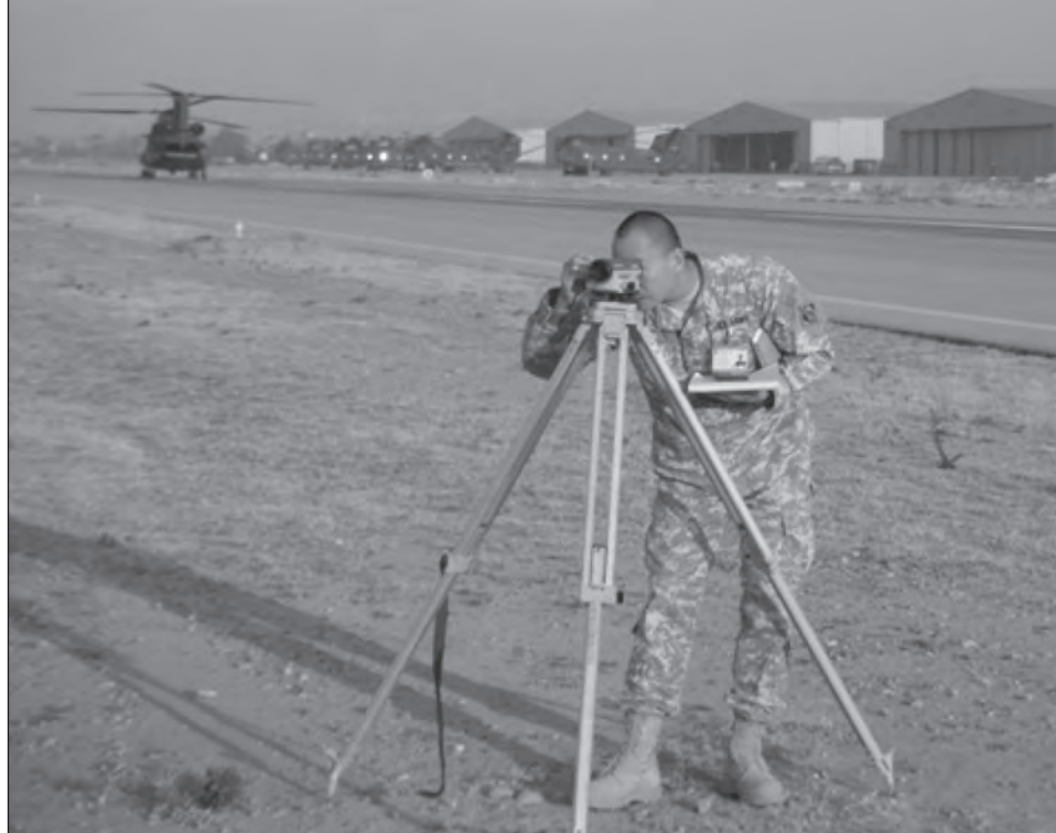
A Soldier verifies grading for helipad improvements at Ghazi Air Base.
