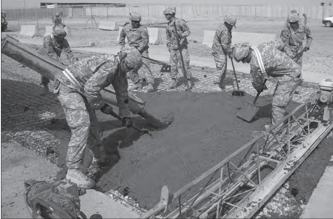
Engineers place a concrete pad for a gate construction project.
