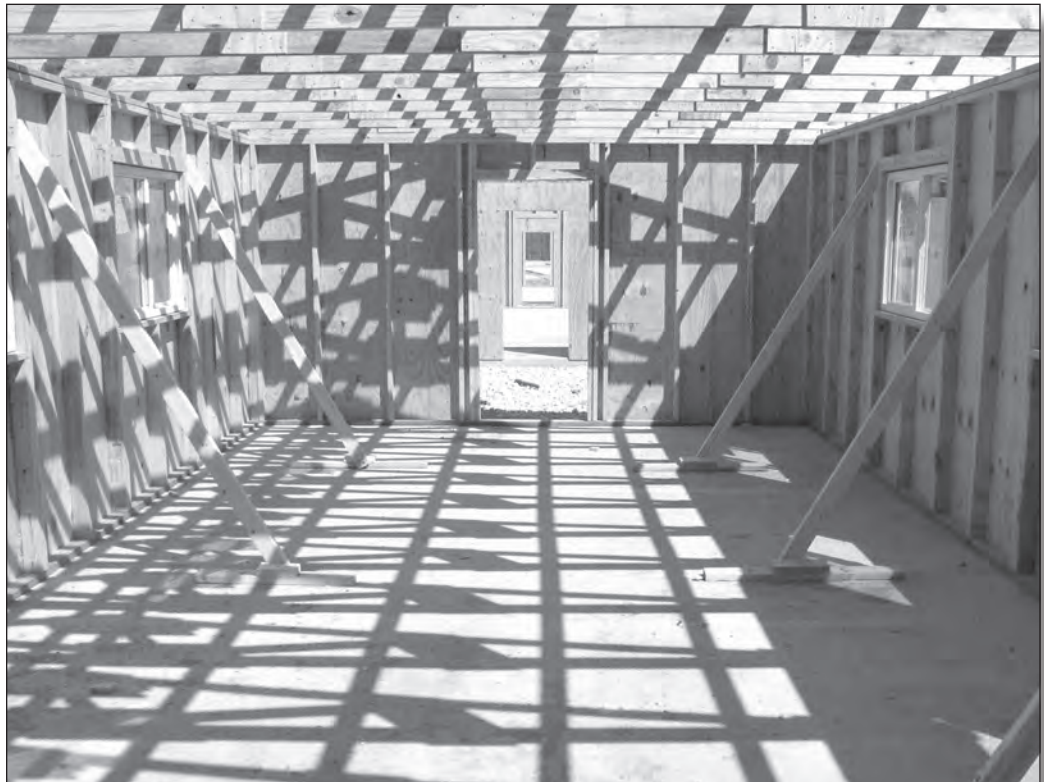
The interior of a SEA hut during construction
