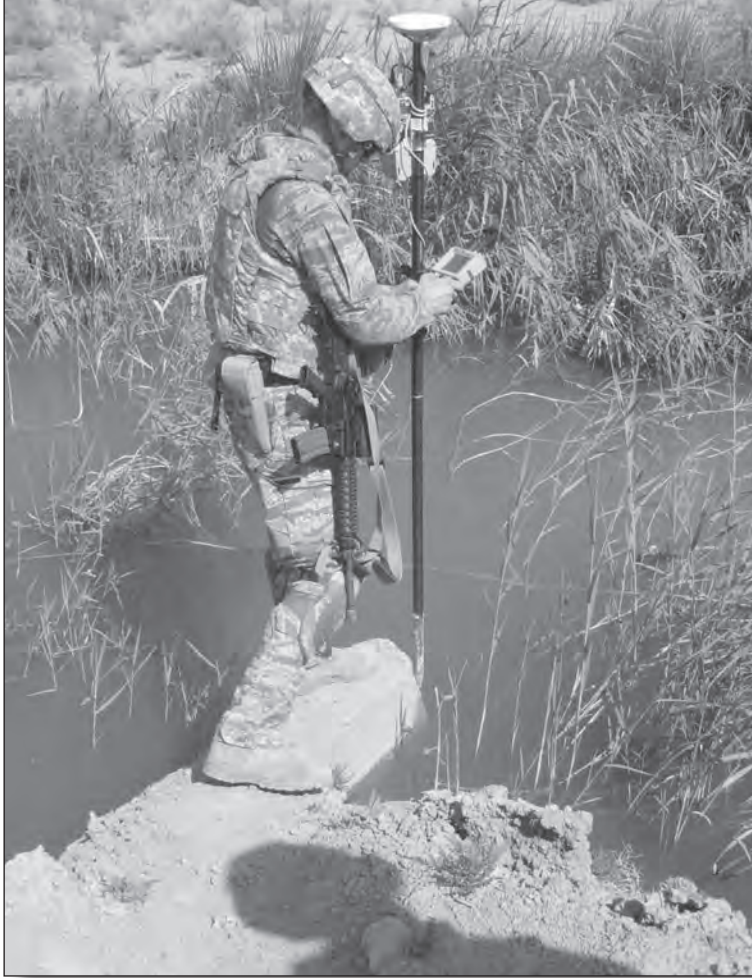
An Airman conducts a survey for a road project.
