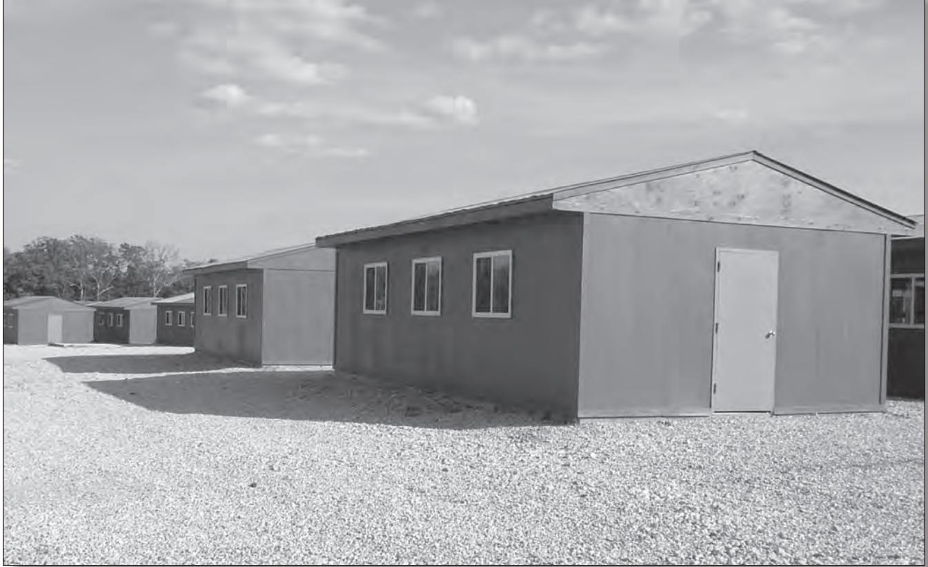
Finished structures at TA 239
