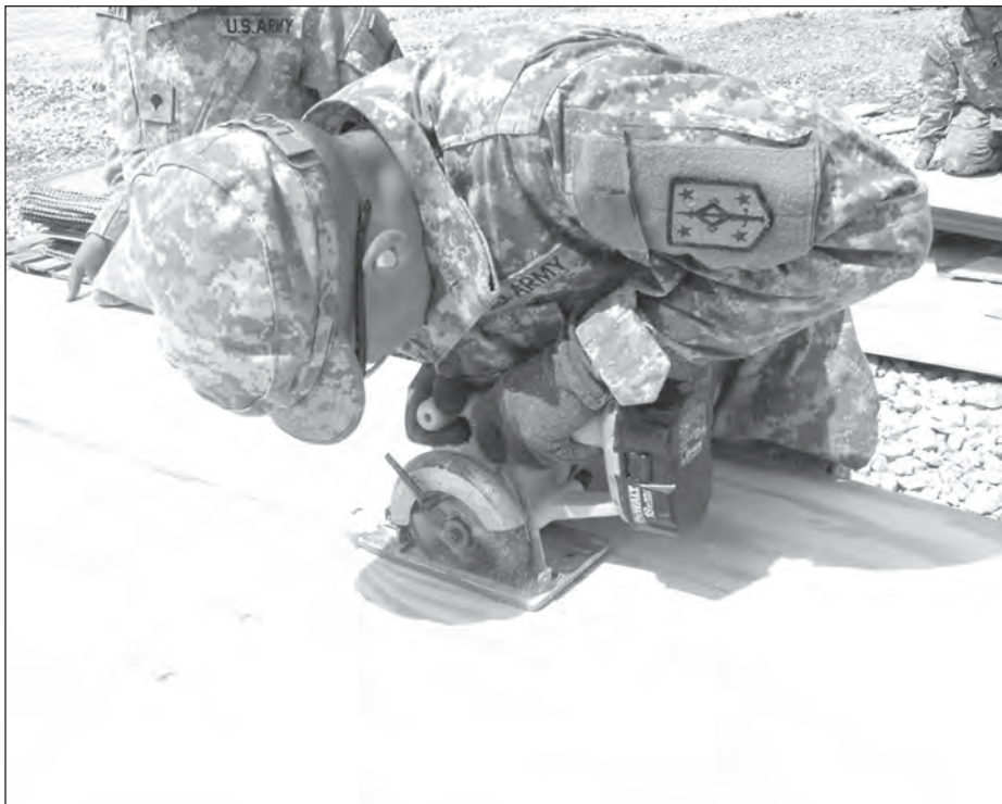
Engineers at work on SEA huts
