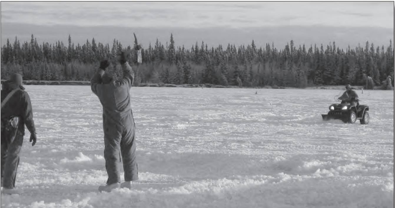
A Soldier drives a four-wheeler with an attached snowplow to construct an initial berm for the ice bridge. Two Soldiers in the foreground break up the rough surface with hand-tools.
