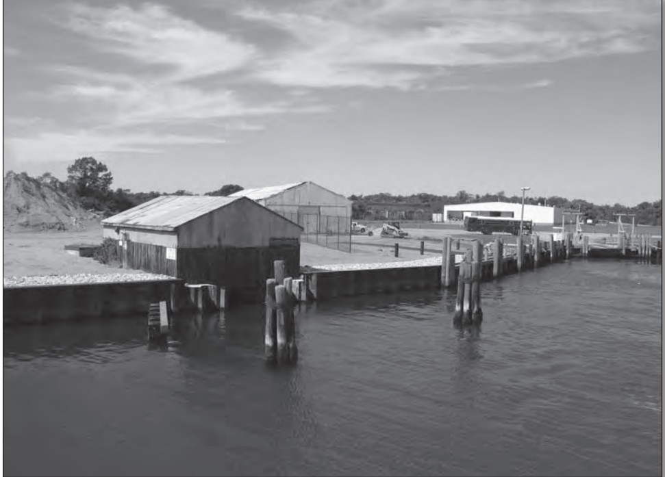
Restored bulkhead on Plum Island
