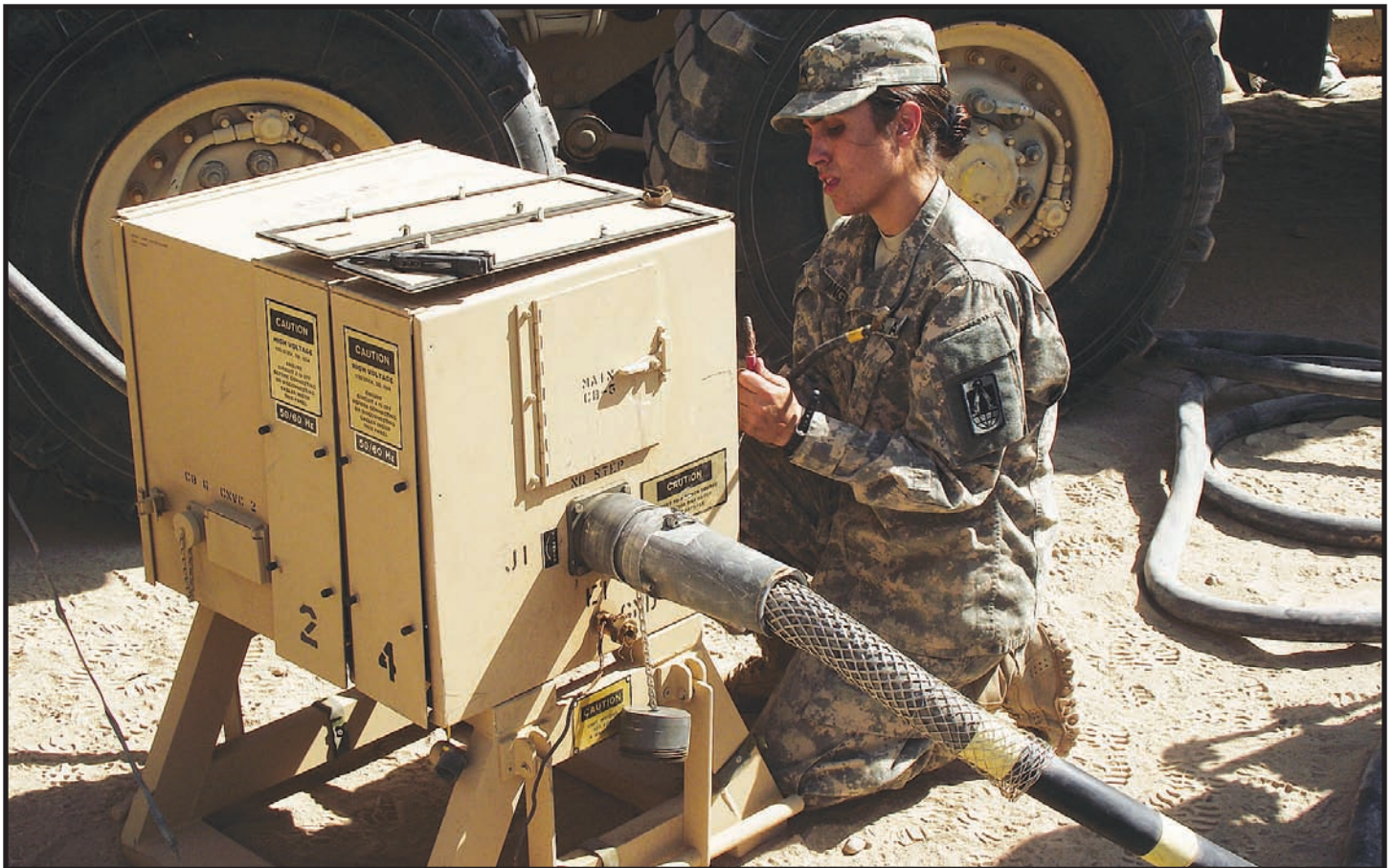
CPL Kari Anglin, 40th Expeditionary Signal Battalion, disconnects a generator at Victory Base Camp in Iraq in September 2011 prior to a STT's redeployment.
