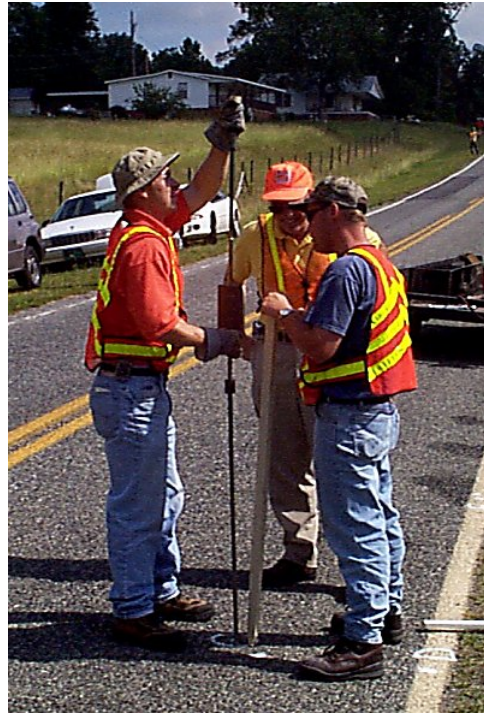
Figure 6. Dynamic Cone Penetrometers being used to determine CBR. The left panel depicts the DCP and magnetic ruler. The right panel illustrates the typical use of the DCP to measure CBR of a road.
