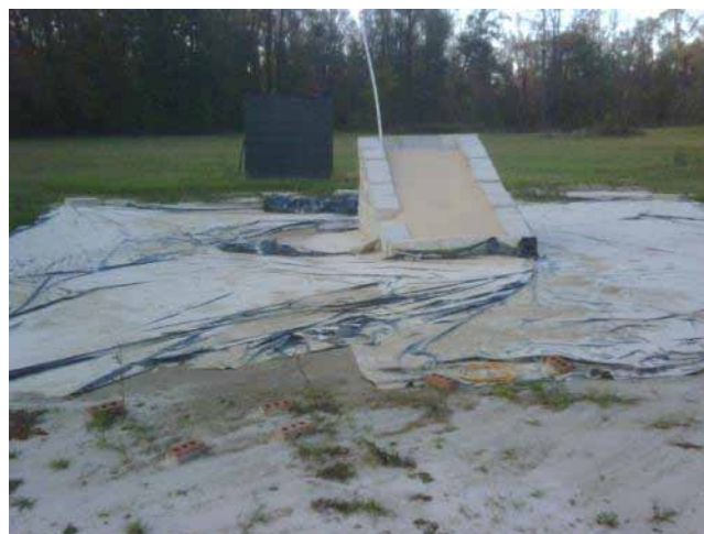
Figure 26. Flood damage, November 2009.
