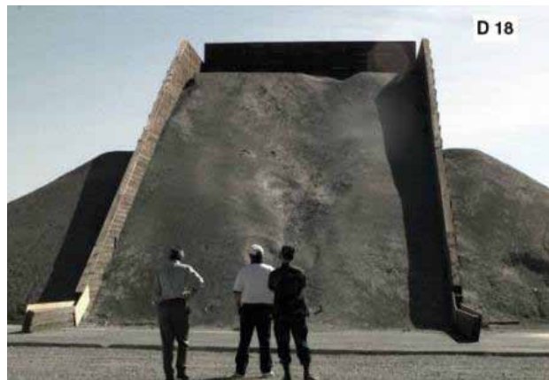
Figure 4. The catch box at Yuma Proving Ground.
