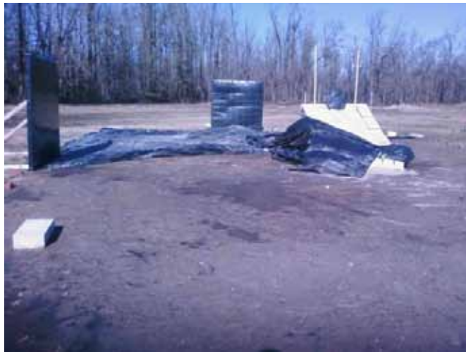
Figure 25. Storm and flood damage at the BBTS, January 2009.
