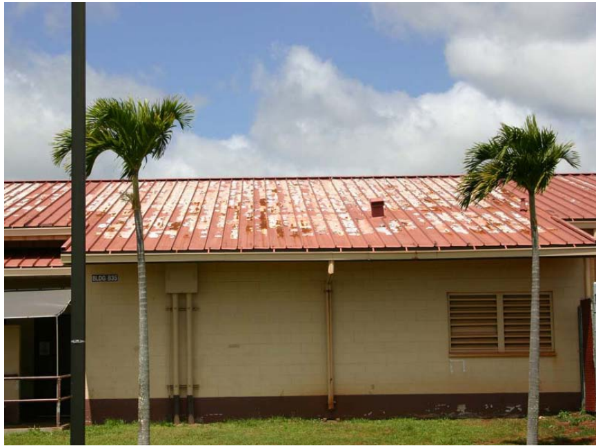
Figure 10. Roof of Building 835 before re-cover. Paint was peeling off in large sheets.
