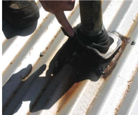
b. Badly corroded steel around exhaust stack
