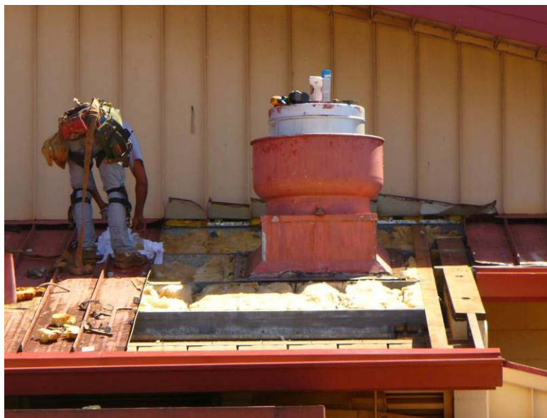
Figure 21. Demolition of lower roof above kitchen area.
