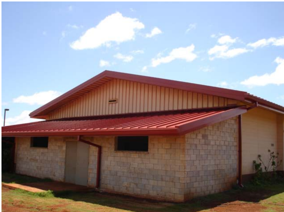
Figure 25. Building addition with finished standing seam roof.
