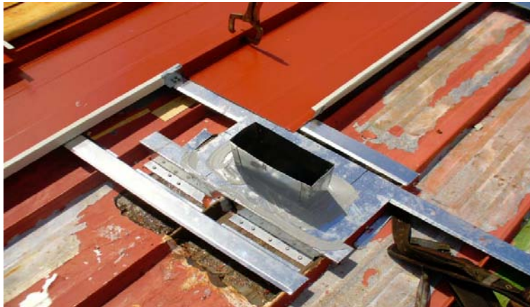
Figure 19. Installation of vent flashing support purlins.
