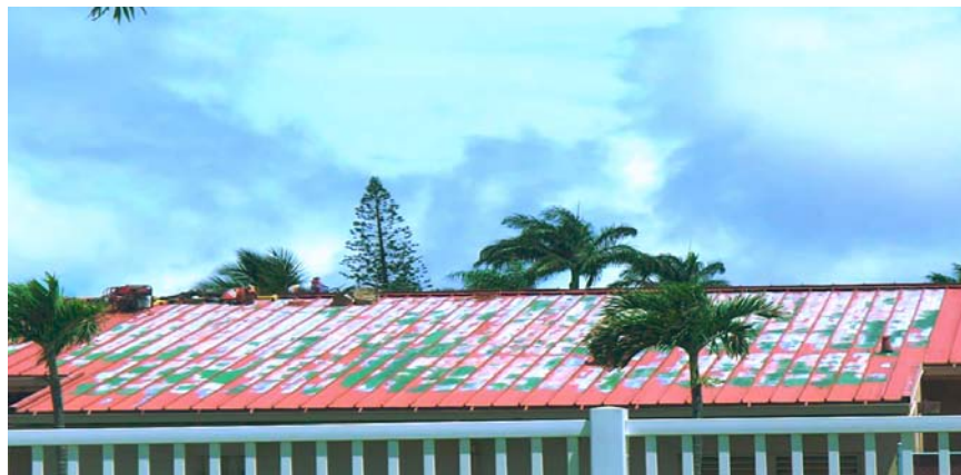
Figure 11. Pressure washed and rust-treated roof areas.
