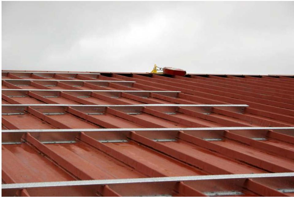
Figure 13. Installed custom manufactured sub-purlin system designed to bridge underlying metal roof panel ribs..
