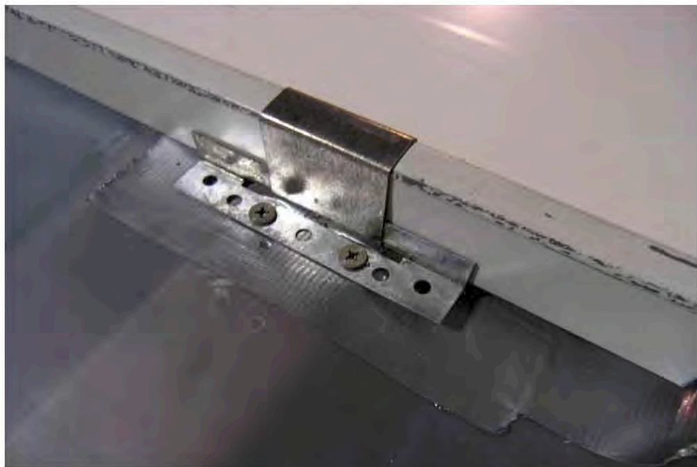
PHOTOGRAPH 8 EXPANSION CLIP INSTALL
