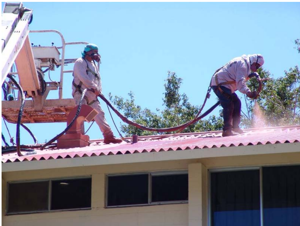
Figure 7. Spraying topcoat.
