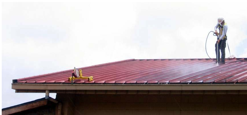
Figure 12. Pressure washing upper roof
