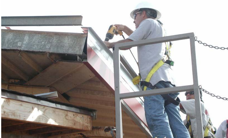
Figure 14. Installation of fascia flashing.
