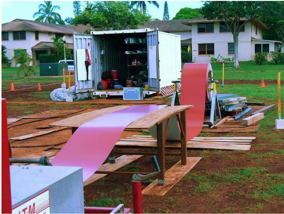
Figure 15. Coil material fed to former.
