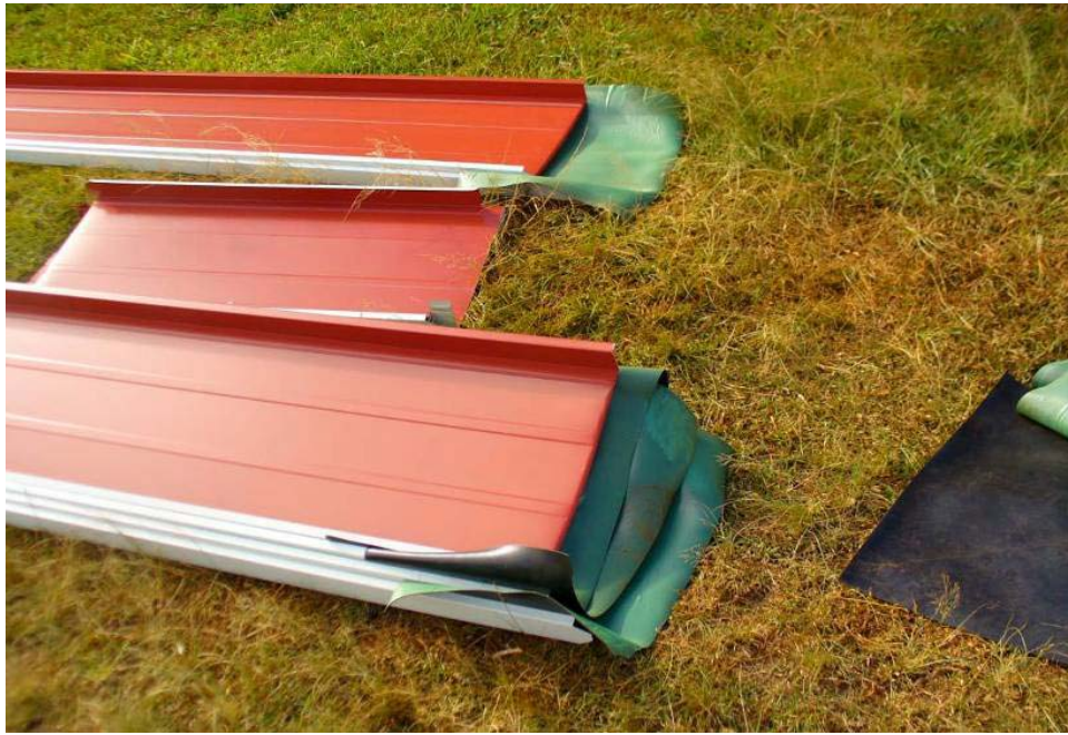
Figure 17. Fabricated panels with pieces of rubber sheets protecting the PVDF finish.
