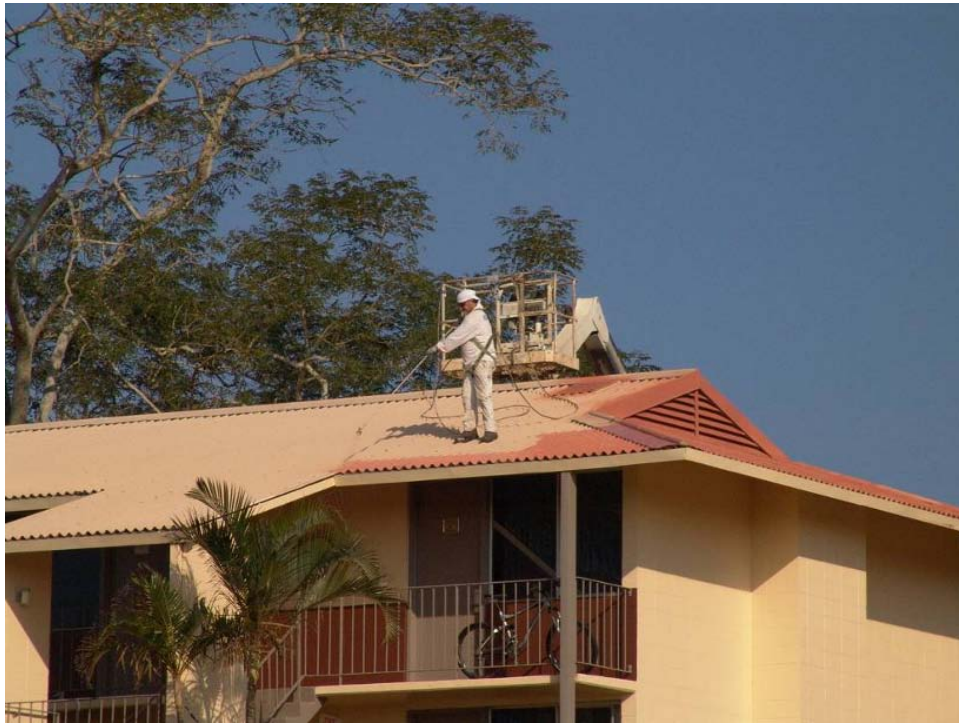
Figure 6. Spraying primer coat.
