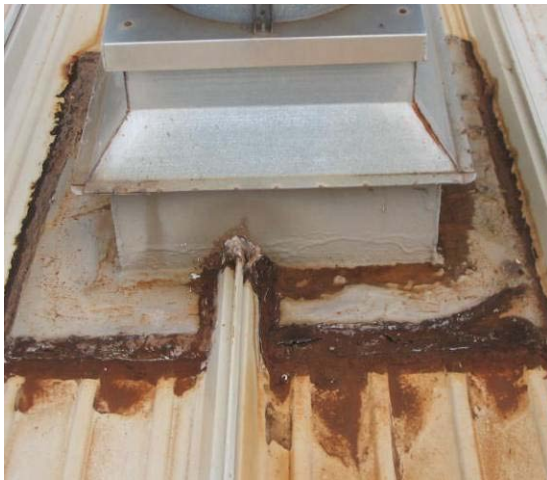
c. Severe corrosion around air vent.
