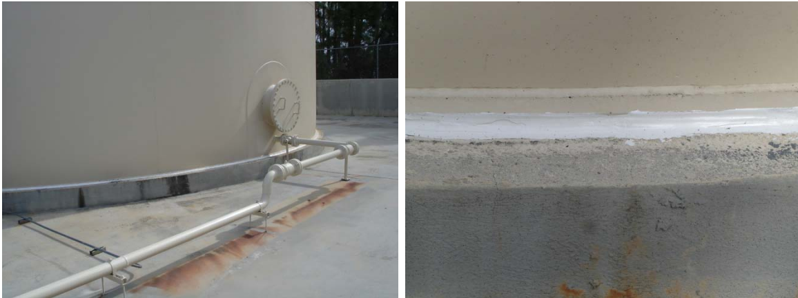
Figure 11. SikaFlex sealant at tank base.
