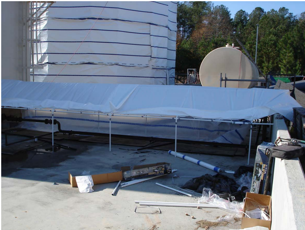
Figure 12. Preparation of piping containment.
