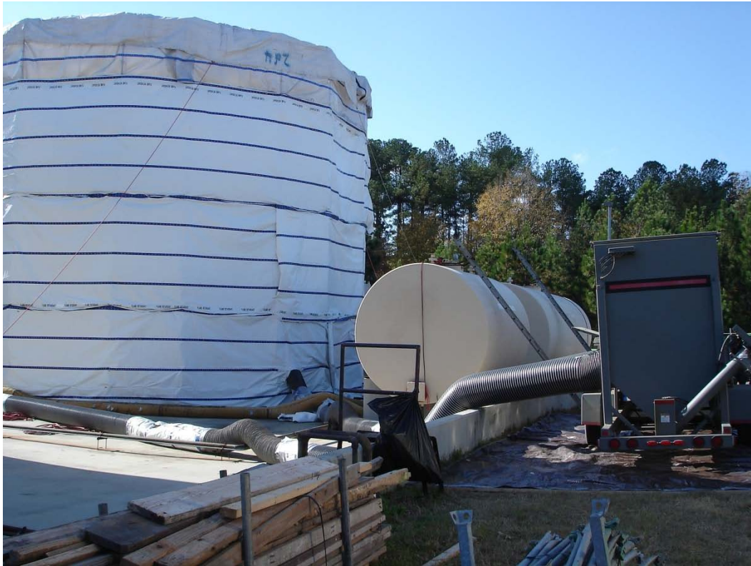
Figure 5. Scaffolding fully contained with environmental controls in place.
