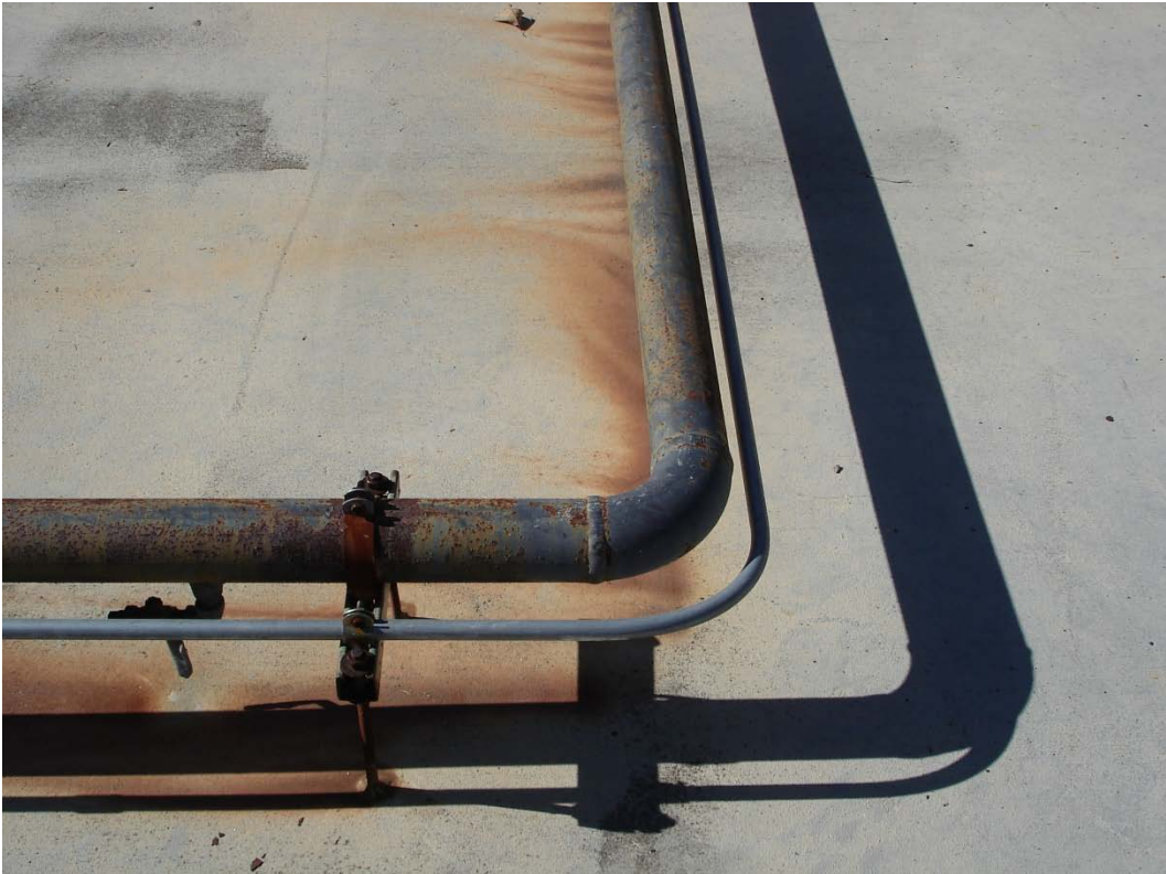
Figure 2. Corroded fuel tank piping with electrical conduit.
