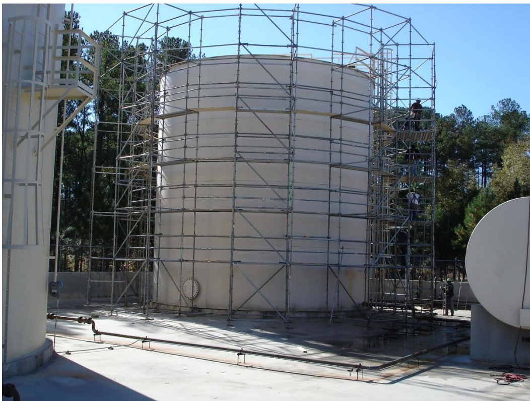
Figure 4. Scaffolding erected around fuel oil tank #2.
