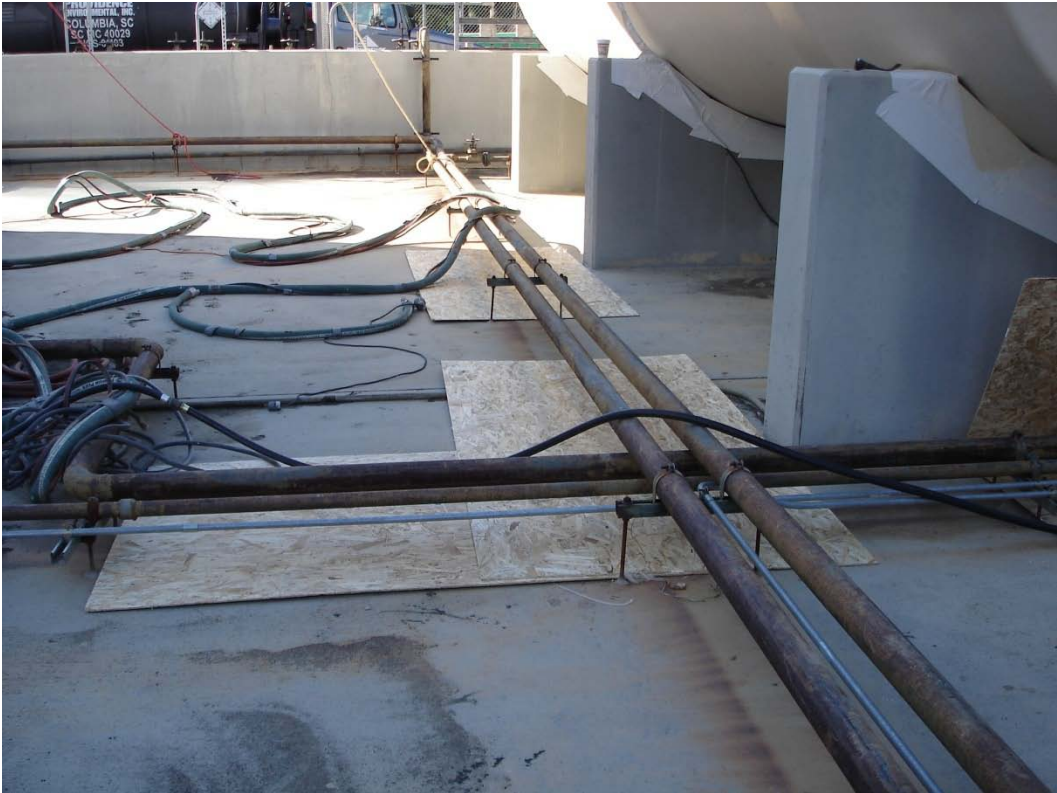
Figure 3. Corroded fuel tank piping.
