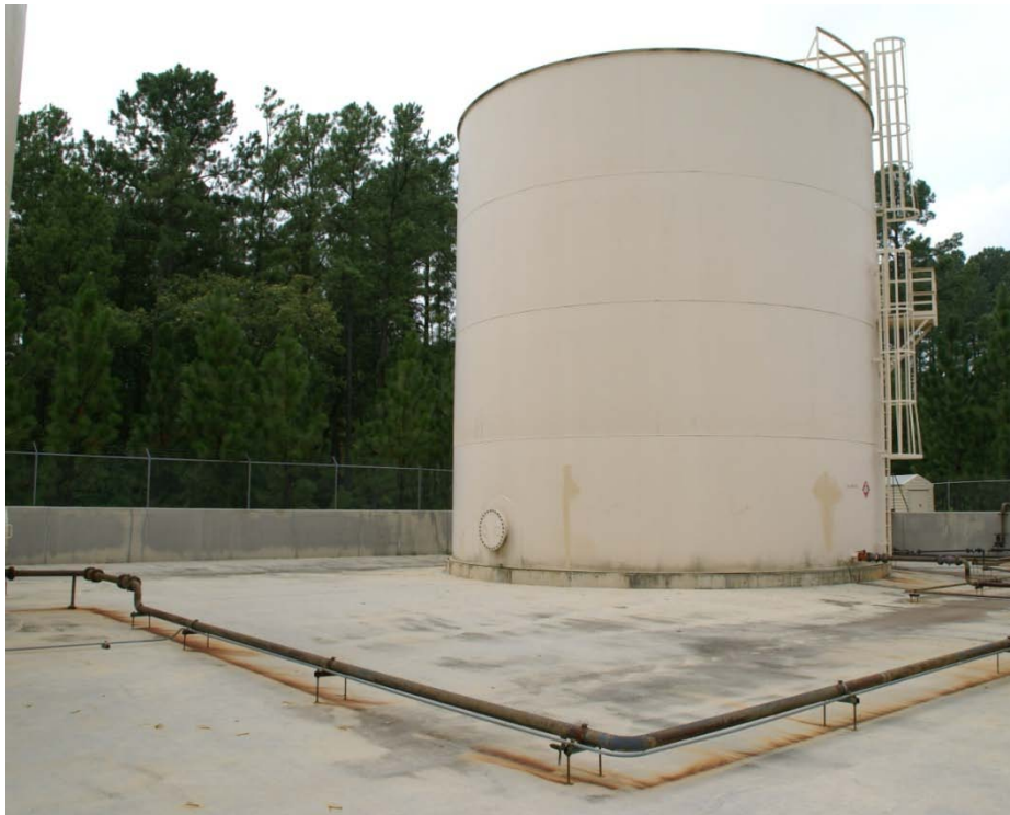
Figure 1. Fort Bragg fuel oil tank #2 with piping (foreground).
