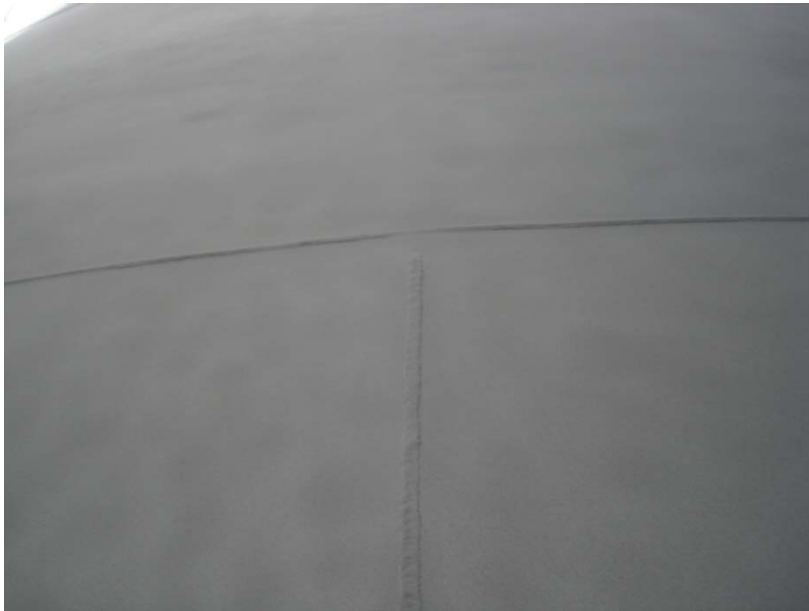
Figure 6. Abrasive blast-cleaned tank surface.
