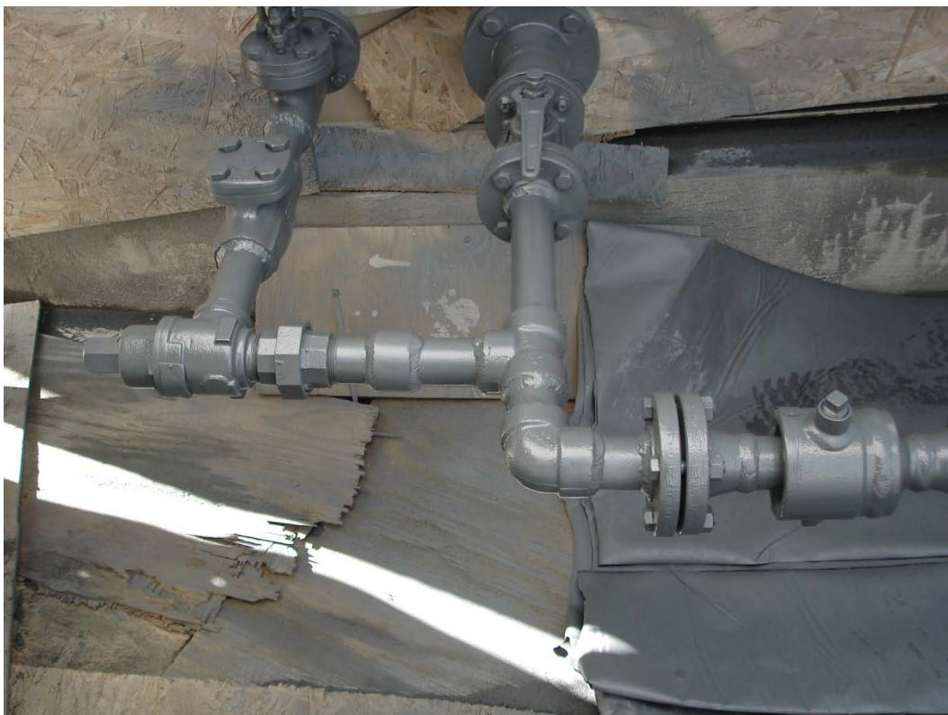
Figure 15. Hybrid CNT/zinc primer on piping.
