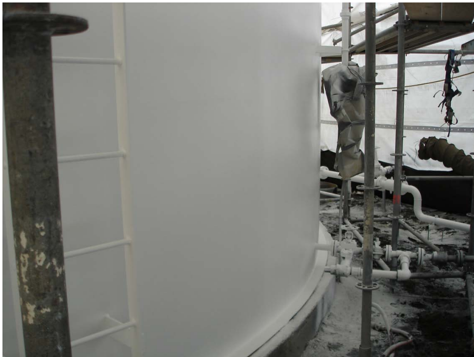
Figure 10. Intermediate epoxy primer.
