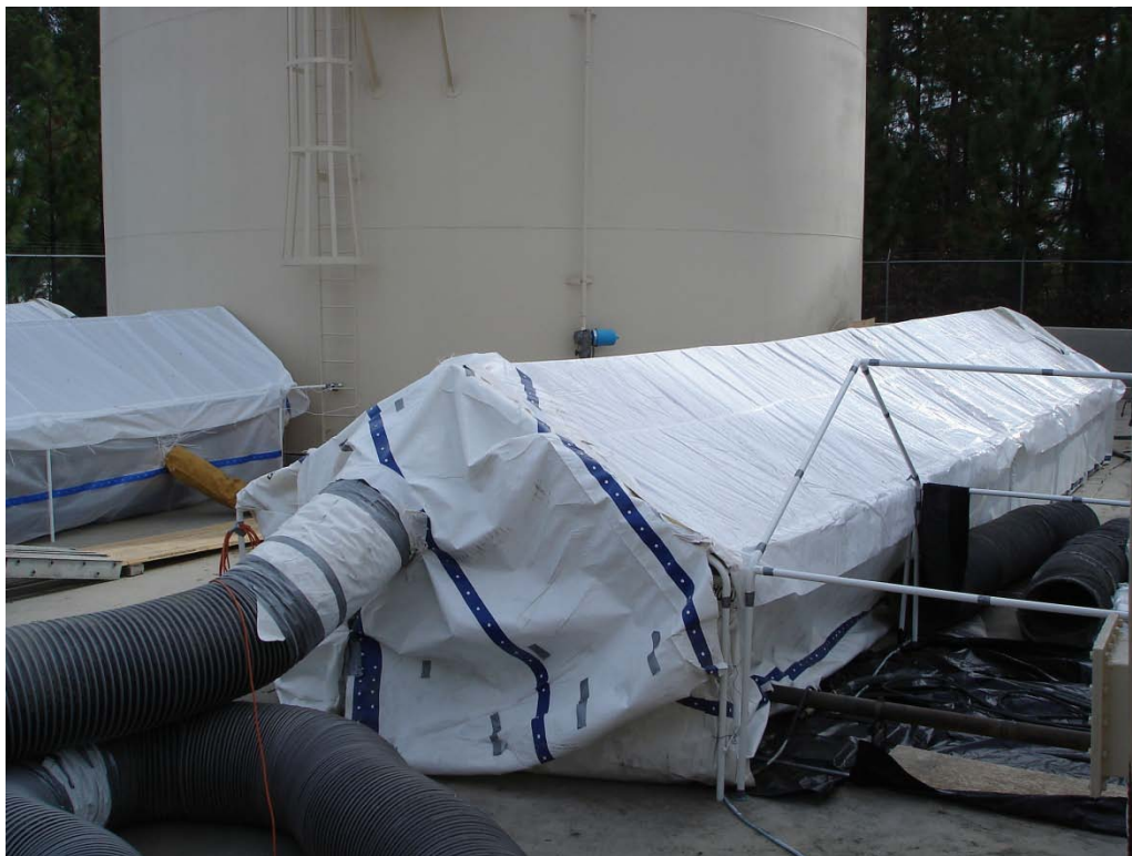
Figure 13. Piping containment with environmental controls.
