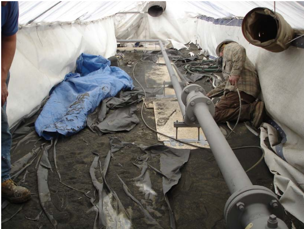
Figure 14. Abrasive blasting of piping.
