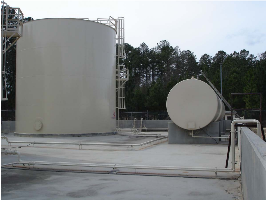
Figure 18. Completed fuel oil tank #2 and piping.
