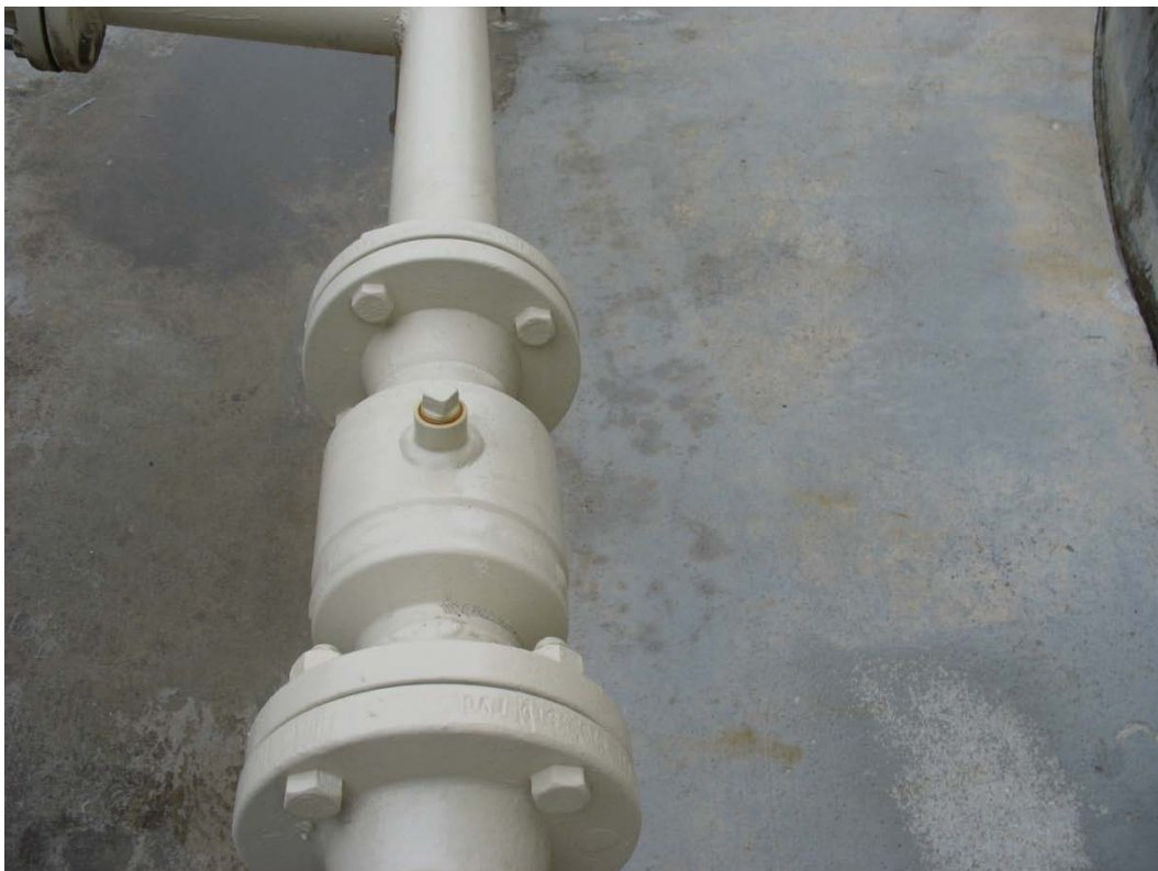
Figure 17. Finished piping with MIL-PRF-85285 polyurethane topcoat.
