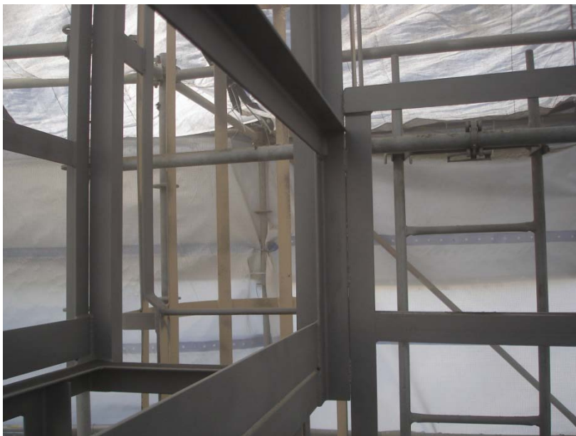
Figure 7. Abrasive blast-cleaned tank ladder.
