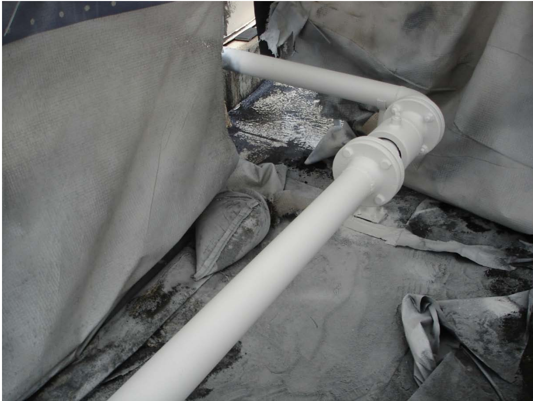
Figure 16. Intermediate epoxy primer on piping.
