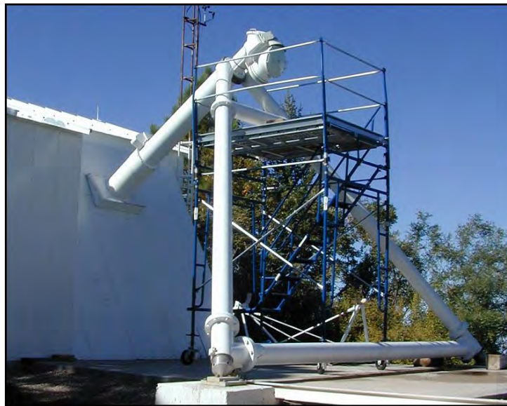
Fig. 2. Photograph of the ISOON prototype facility at the NSO, Sacramento Peak campus.
