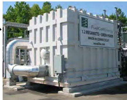
Four-Stack Module
