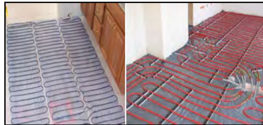
Electric and Hydronic Radiant Floor Heating Systems
