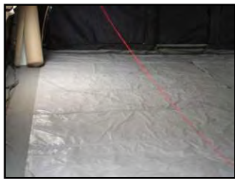
Radiant Floor Heating Prototype
