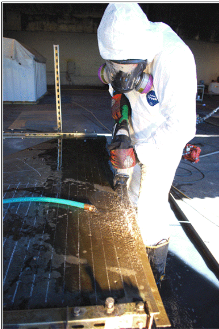
Figure 9. Reciprocating Saw Being Used to Cut F-16 Composite Sheets
