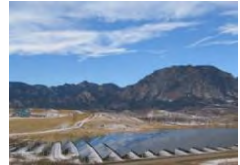
Fort Carson Photovoltaic Array
