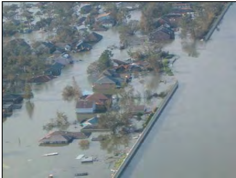
Figure 2.6. Floodwall failure on 17th Street Canal from Hurricane Katrina in New Orleans.
