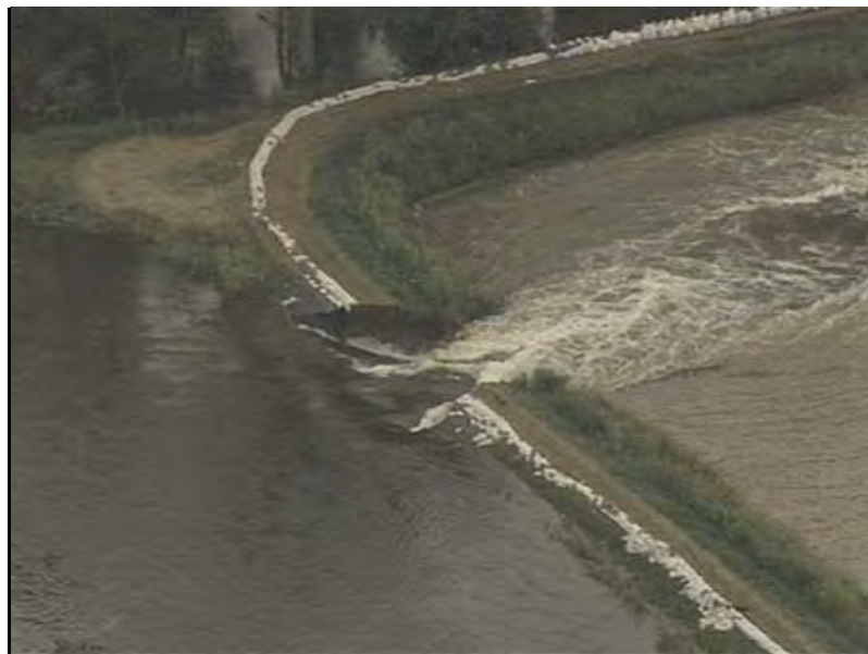
Figure 2.3. Failure of the Pin Oak levee in the Midwest. Note sand bags atop levee used to fight rising water levels.
