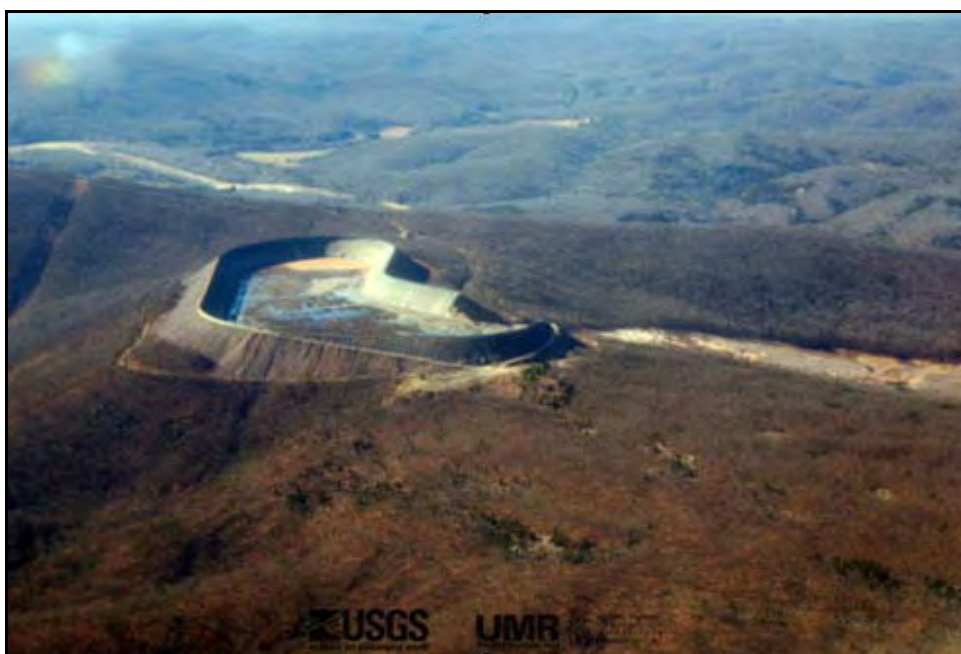
Figure 2.17. Aerial photo of the Taum Sauk Upper Reservoir just after breach in December 2005.
