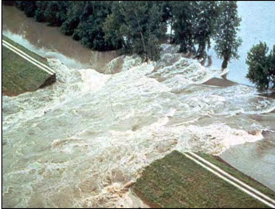
Figure 2.14. Kaskaskia River levee breach at location of sand boil.
