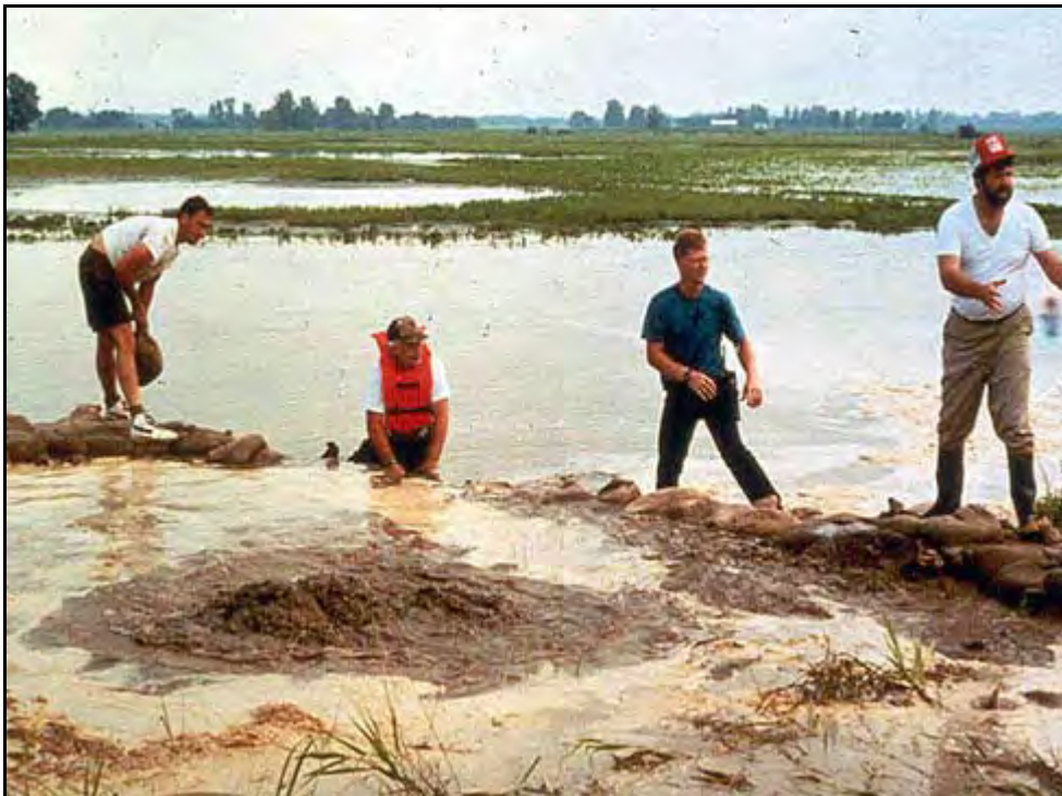
Figure 2.13. Sand bag levee around sand boil on Kaskaskia River.
