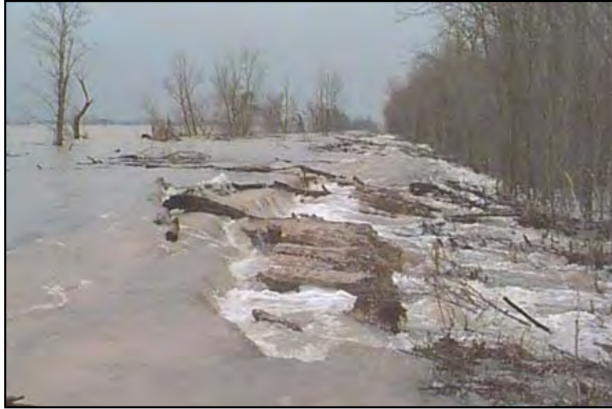
Figure 2.11. Overtopping of a levee over a wide area with a potential breach growing in foreground.
