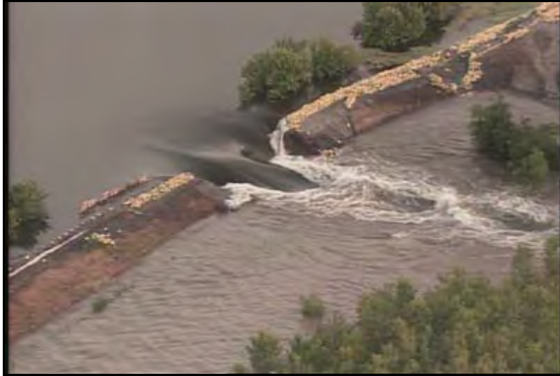
Figure 2.4. Failure of the Elm Point levee in the Midwest.
