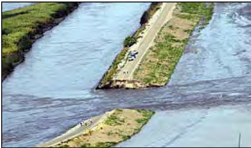
Figure 2.5. Upper Jones Tract levee breach in the Sacramento-San Joaquin River Delta.
