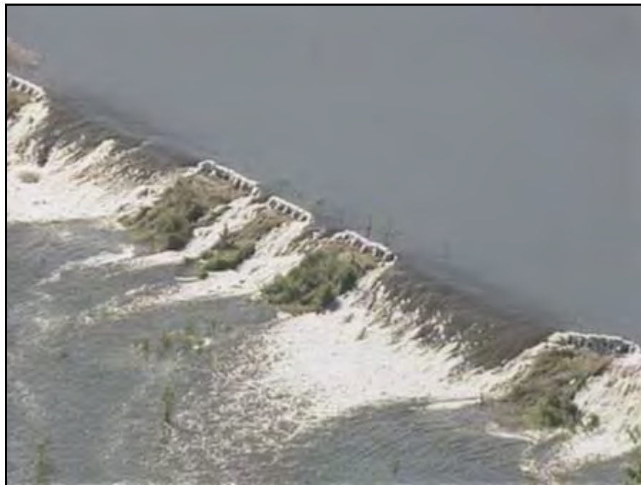
Figure 2.12. Overtopping of the Foley levee in the Midwest.
