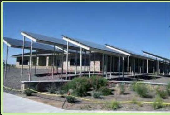
Fort Bliss solar panels
