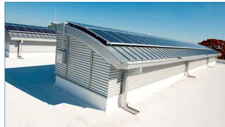
Reflective roof with solar panels, Tyndall AFB, FL
