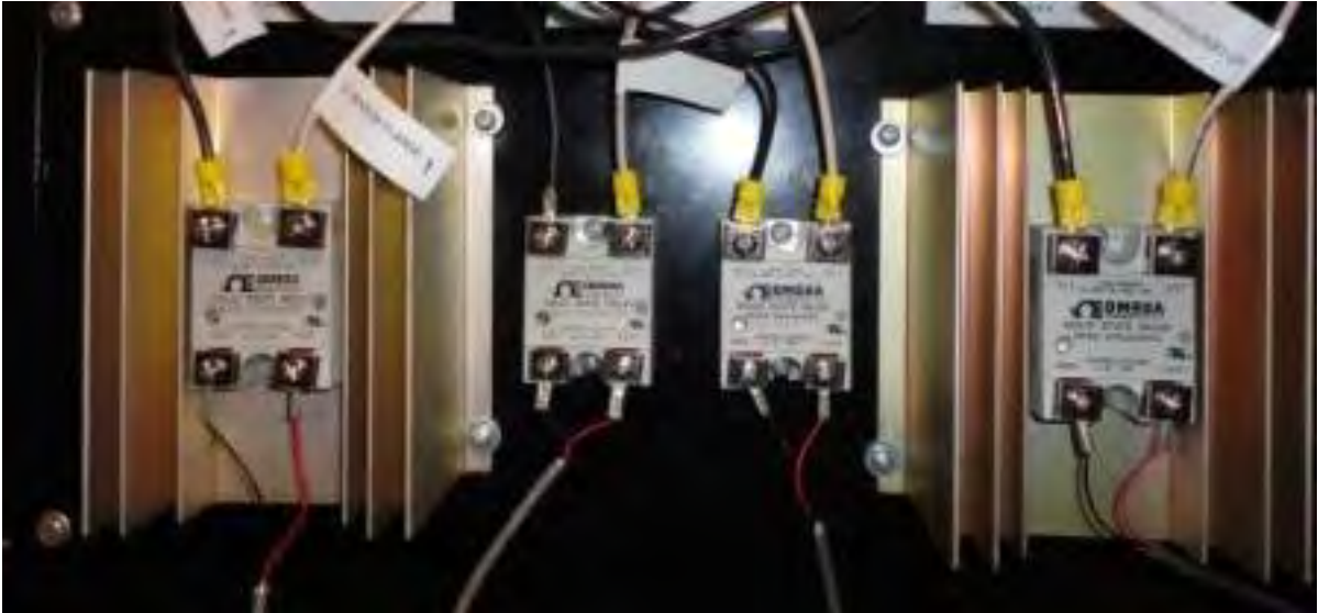
Figure 28. Solid State Relays and Finned Heat Sinks
