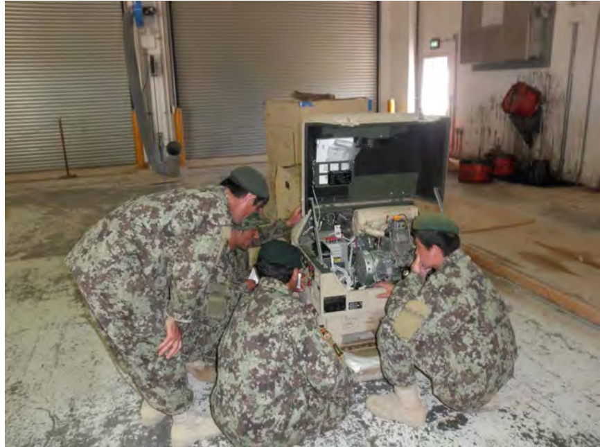
Figure 12. ANA Mechanics Repair Generator
