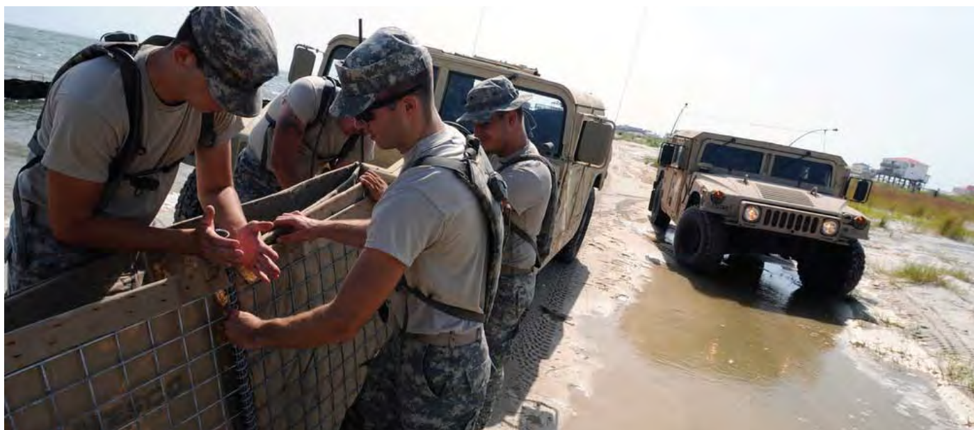
Building and maintaining miles of HESCO barriers to protect Dauphin Island, Ala., beaches. Photo by Staff Sgt. Jim Greenhill
