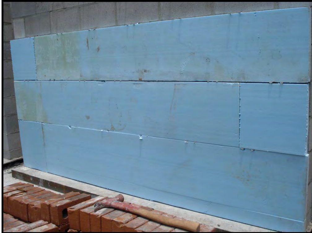
Figure B-35. Insulation foam positioned for the cavity wall construction
