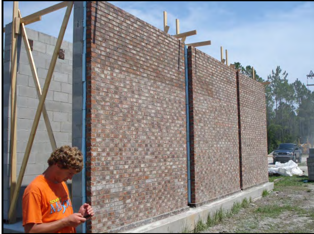
Figure B-45. Wall panel construction complete
