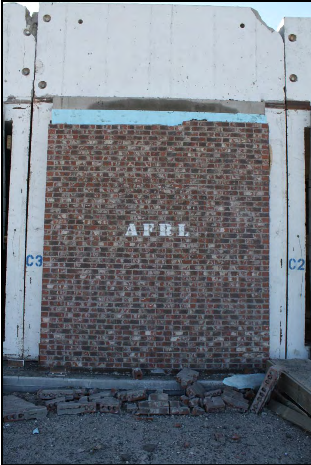
Figure C-15. Experiment 1 cavity wall front view
