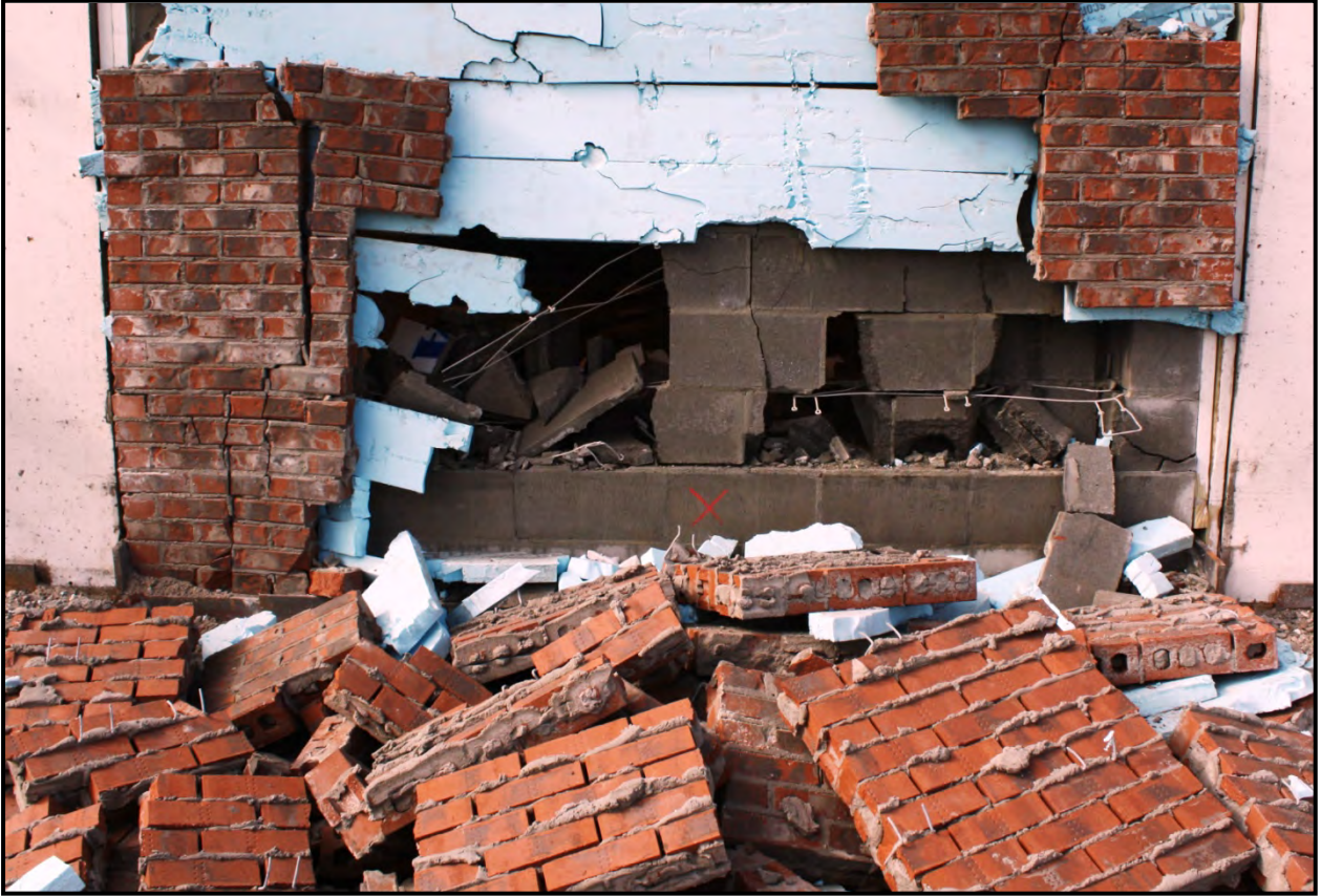
Figure C-60. Experiment 3 cavity wall panel lower exterior view
