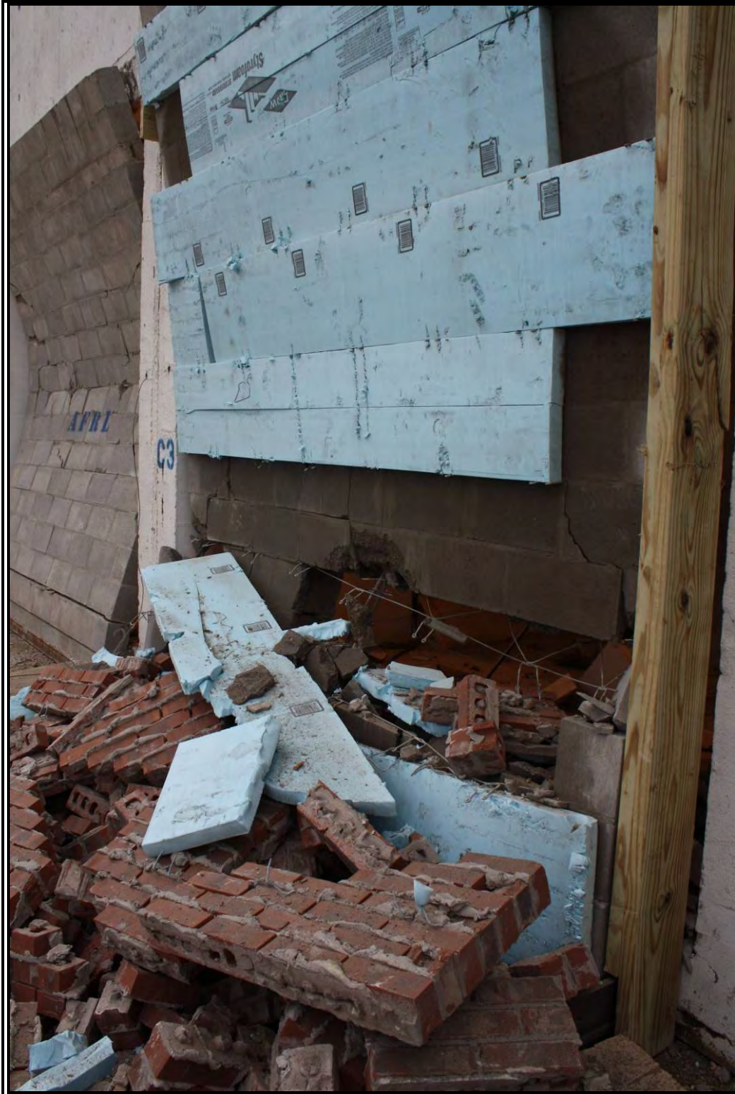
Figure C-37. Experiment 2 cavity wall panel exterior view
