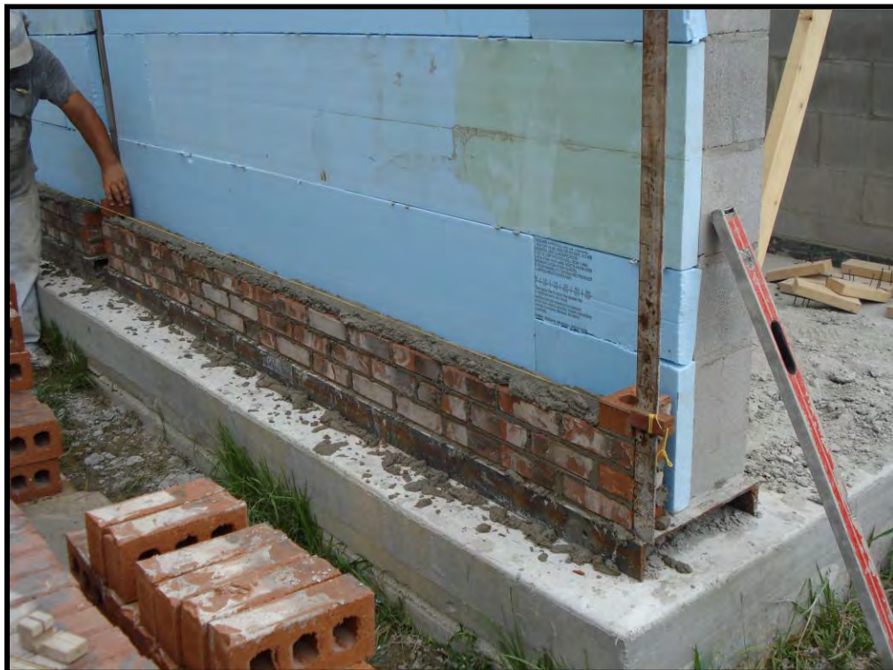
Figure B-36. Beginning of cavity wall veneer construction
