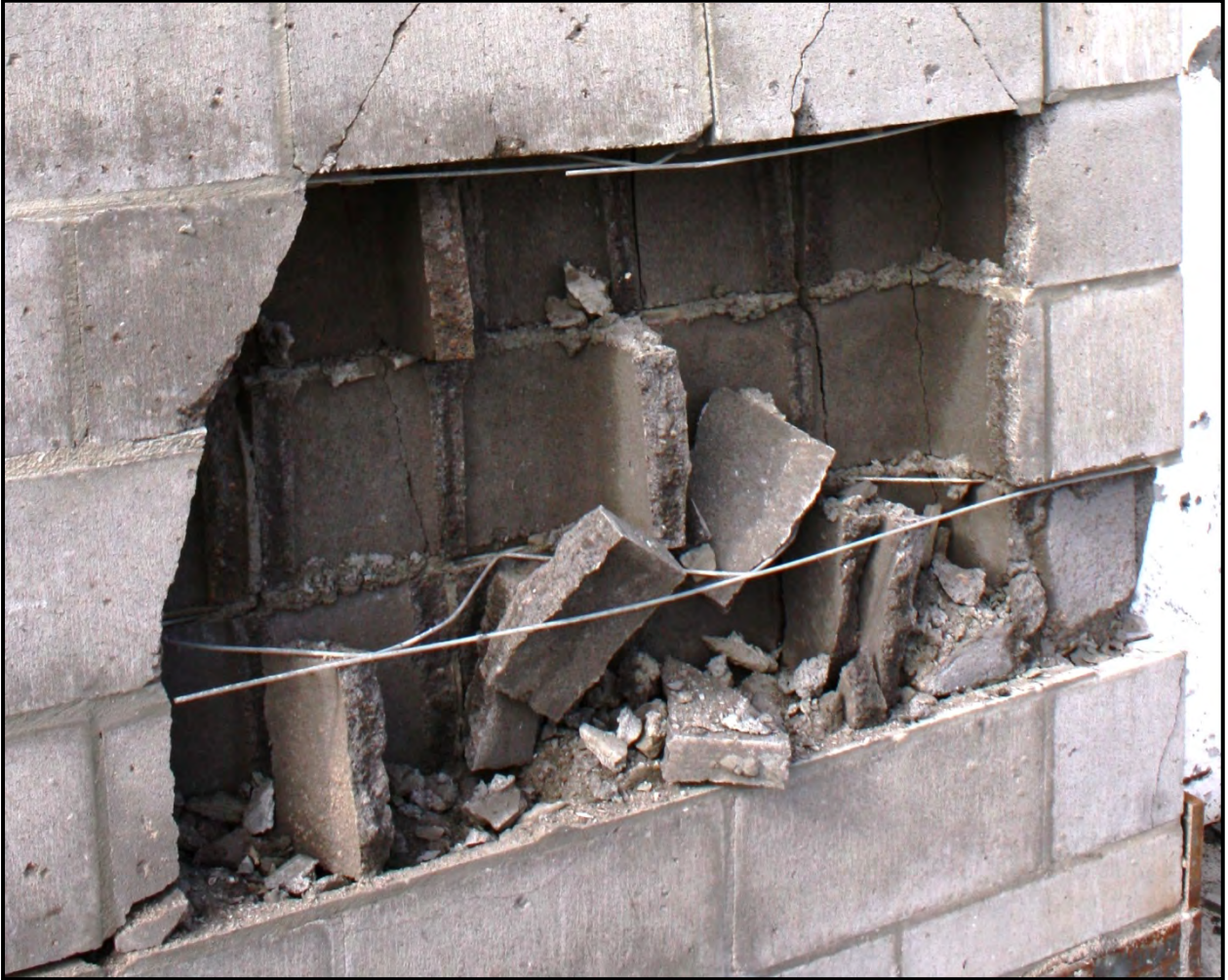
Figure C-52. Experiment 3 8-inch CMU panel close-up exterior view
