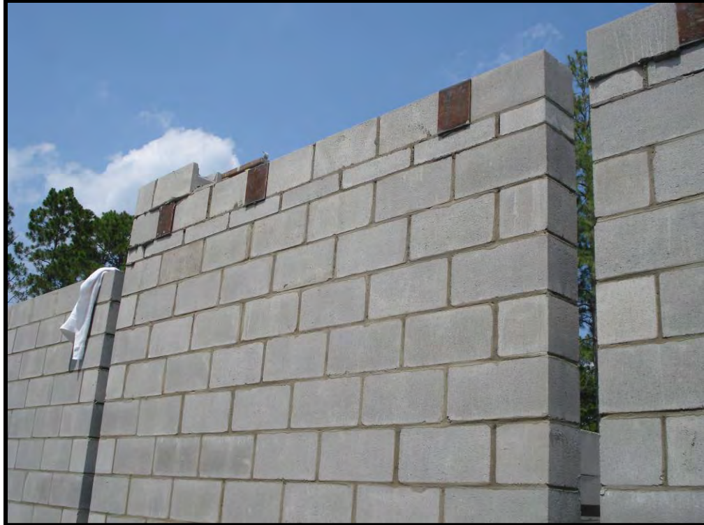
Figure B-27. Top bond beam complete
