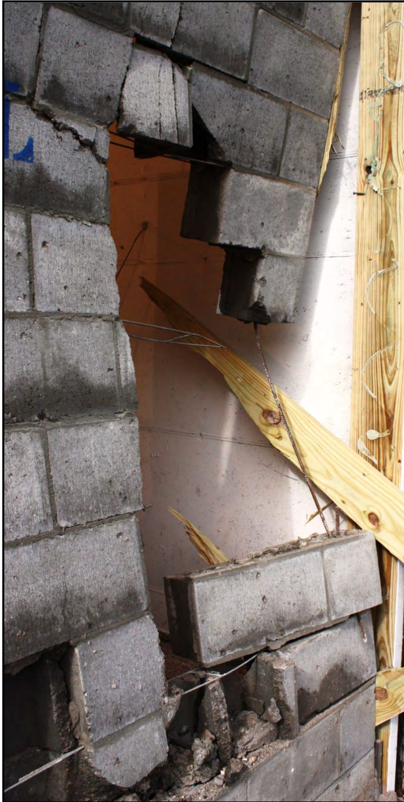
Figure C-46. Experiment 3 6-inch CMU panel close-up breaching exterior view
