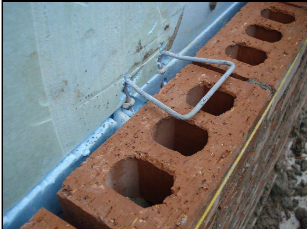
Figure B-37. Close-up of veneer tie
