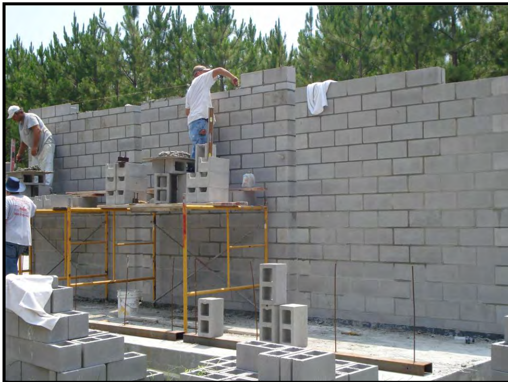
Figure B-22. Construction wide view
