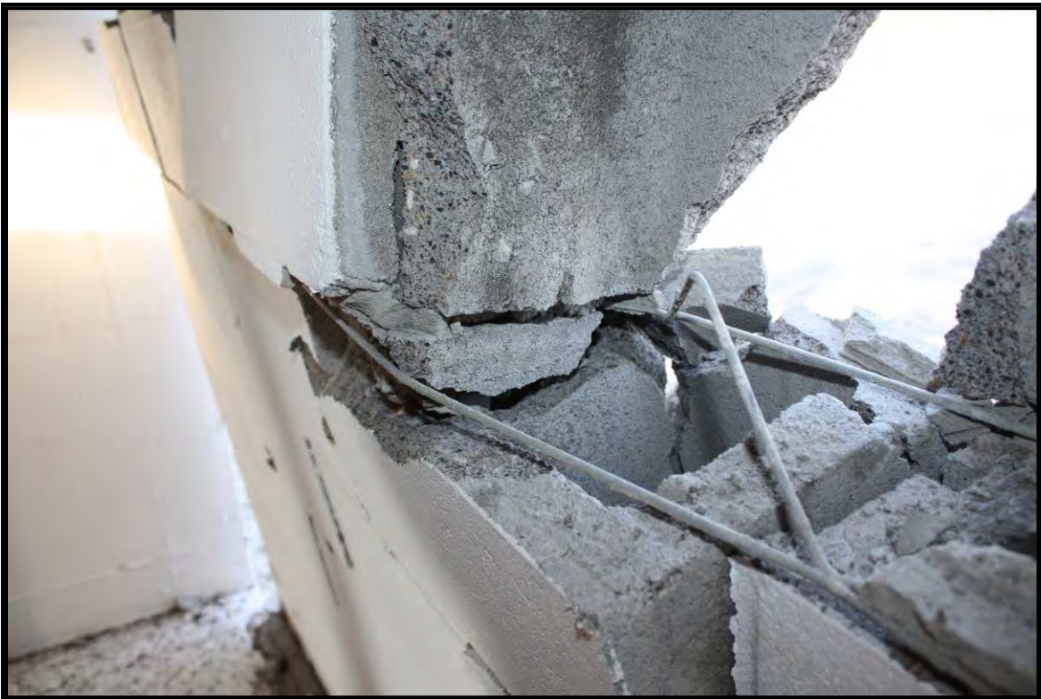
Figure C-14. Experiment 1 8-inch CMU panel close-up interior view
