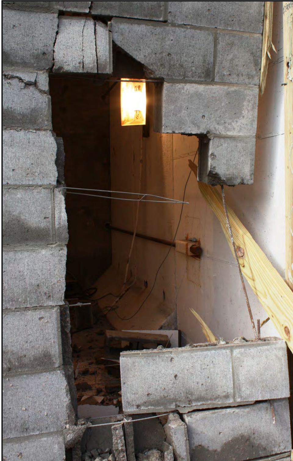
Figure C-45. Experiment 3 6-inch CMU panel close-up breaching exterior view
