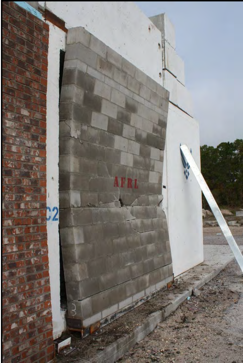
Figure C-10. Experiment 1 8-inch panel left side view
