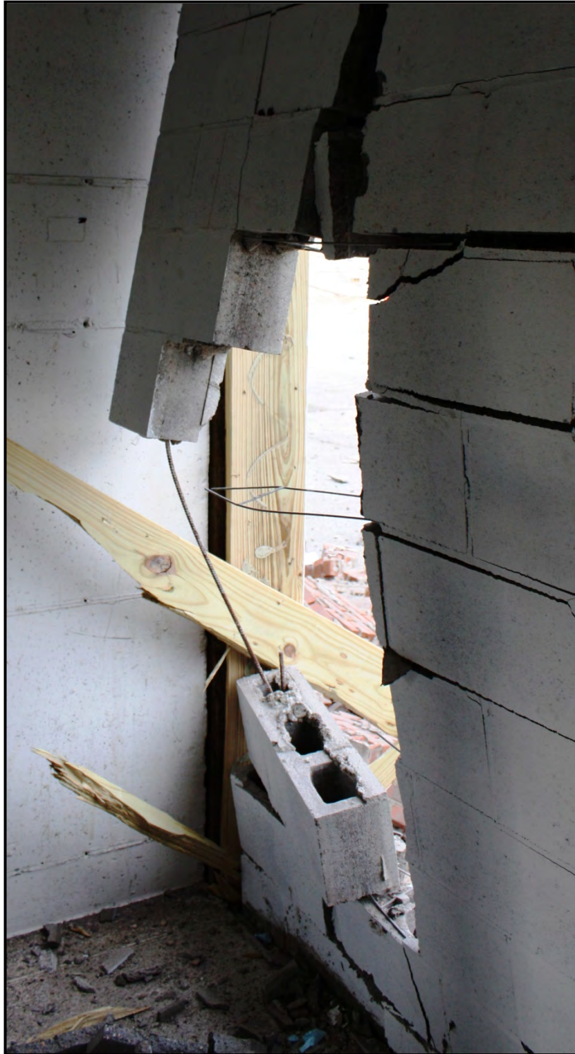
Figure C-49. Experiment 3 6-inch CMU panel breaching interior view
