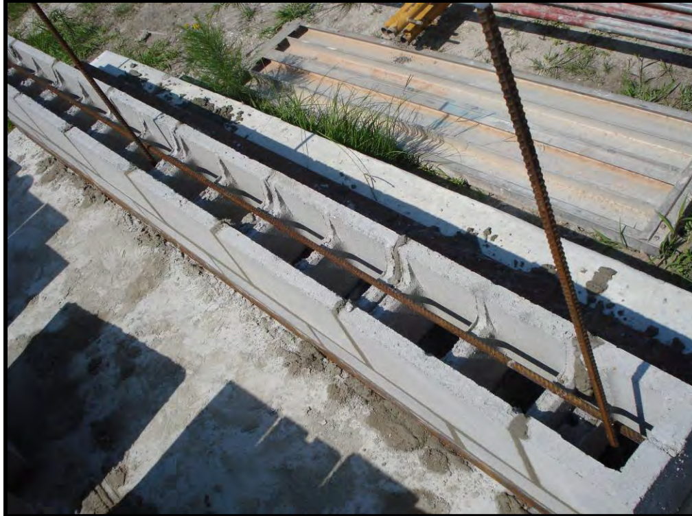
Figure B-11. Bottom bond beam top view
