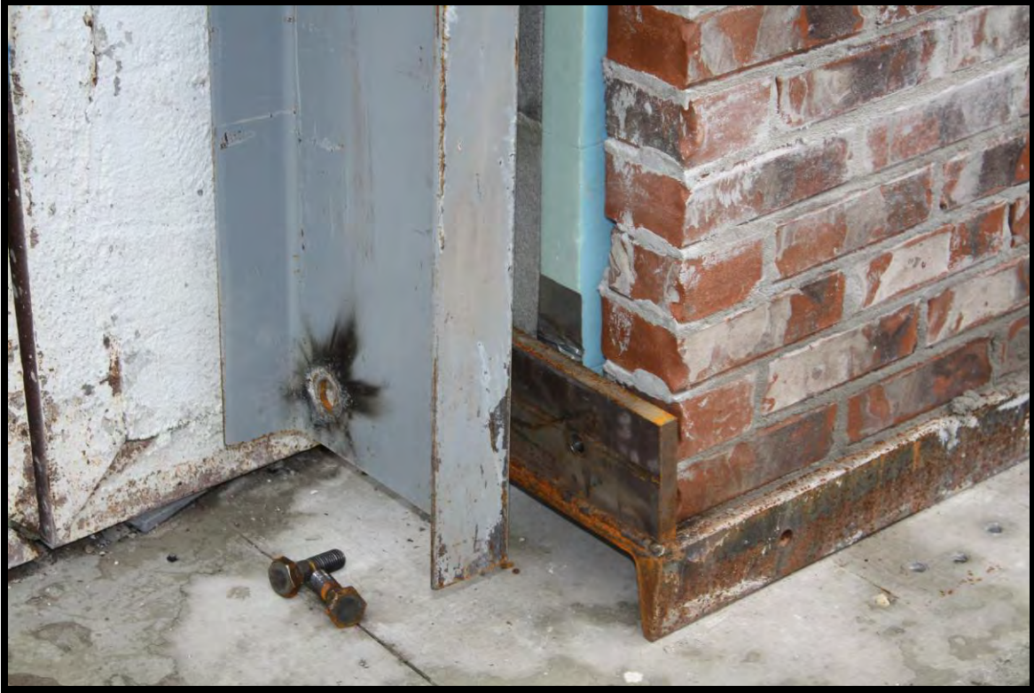
Figure B-55. Base of cavity wall being positioned for testing
