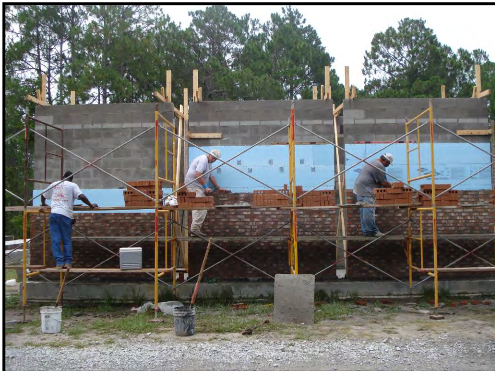
Figure B-42. Cavity wall panel construction
