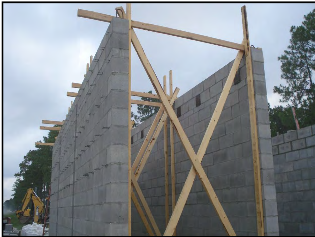
Figure B-34. Positioning wind stability bracing
