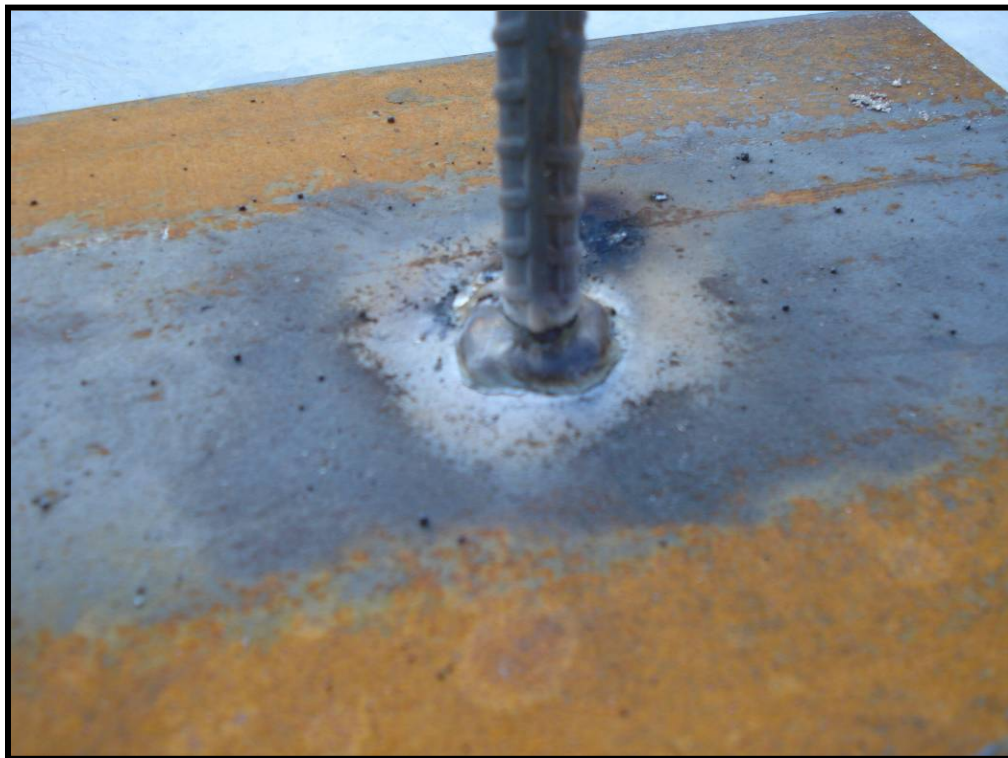
Figure B-8. Base of the welded dowel
