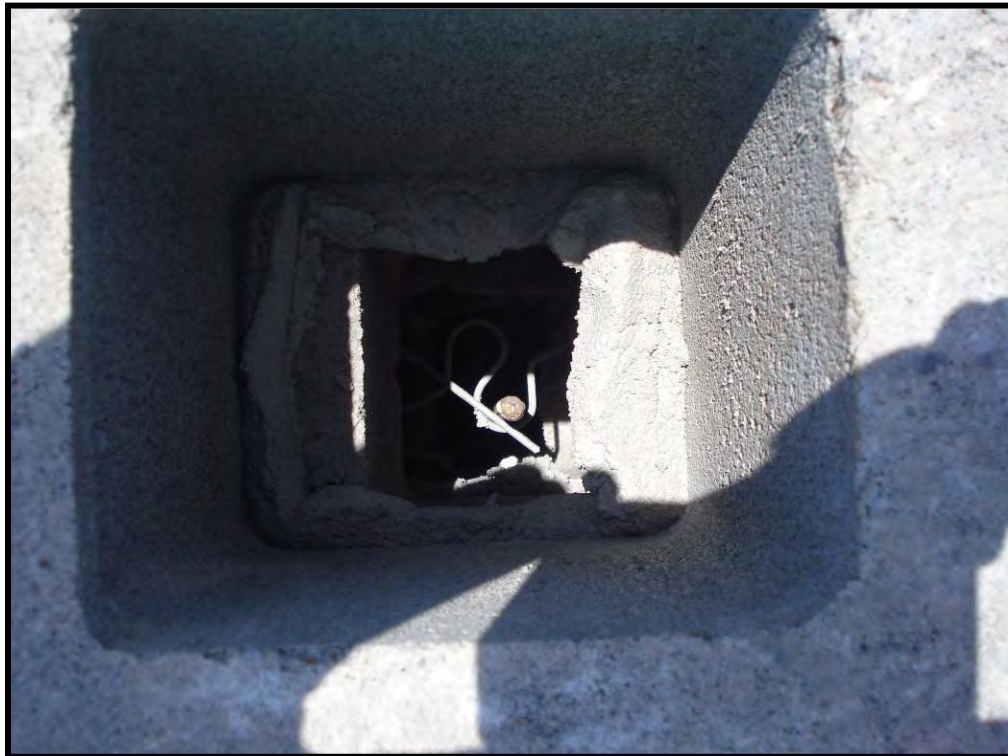
Figure B-18. Top view of dowel rebar positioned
