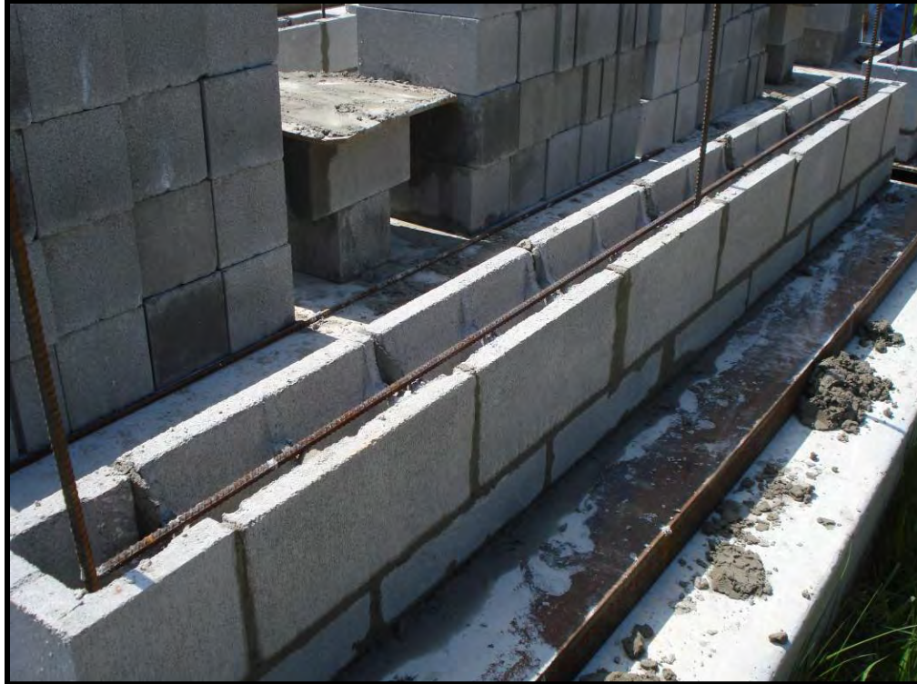
Figure B-13. Bottom bond beam rebar in position
