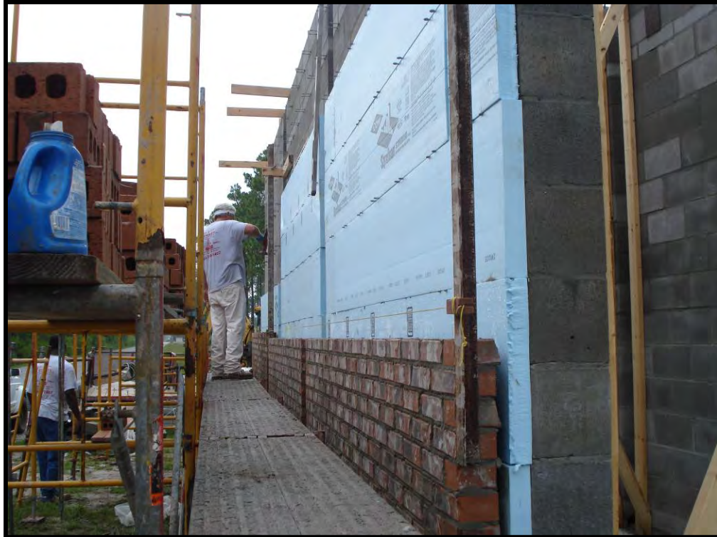
Figure B-41. Cavity wall panel construction
