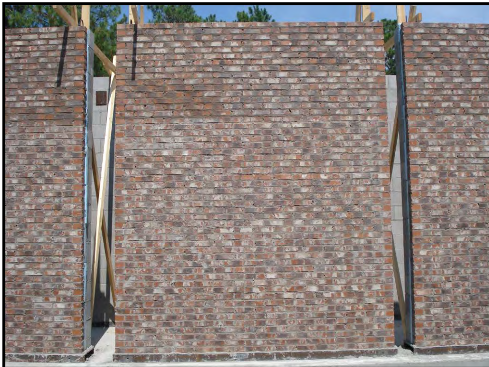
Figure B-44. Cavity wall panel construction complete
