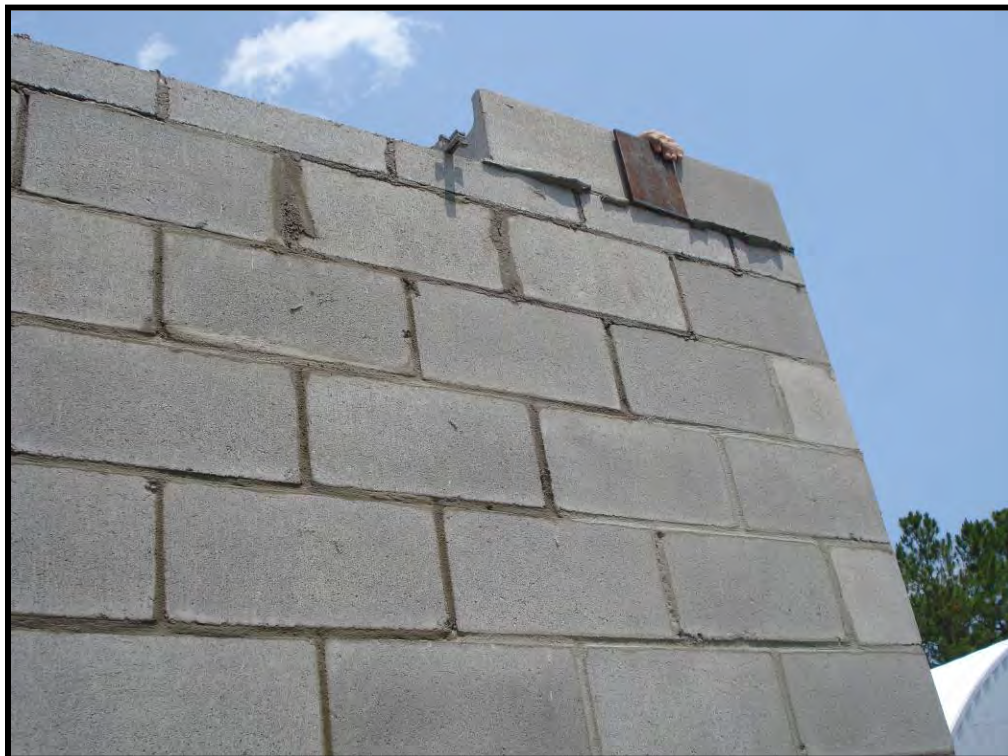
Figure B-20. First embed positioned
