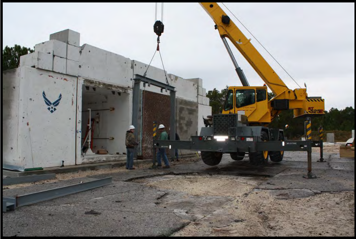
Figure B-57. Removing the stability frame
