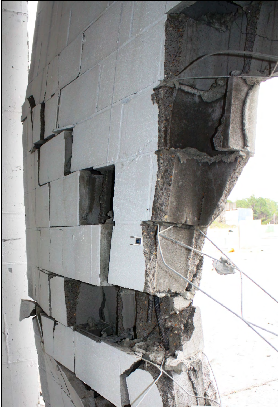
Figure C-58. Experiment 3 8-inch CMU panel breaching interior close-up view
