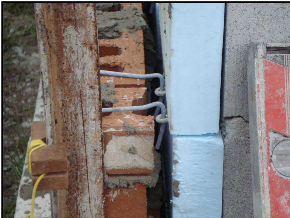
Figure B-38. Side view of veneer tie
