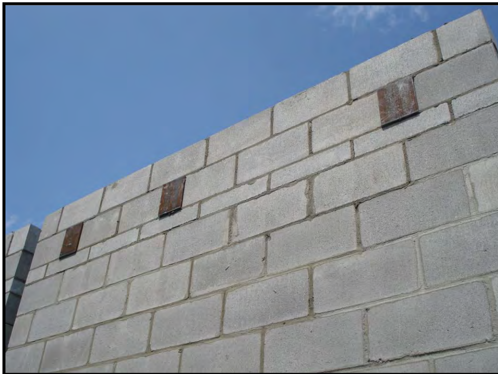
Figure B-28. 8-inch CMU panel complete
