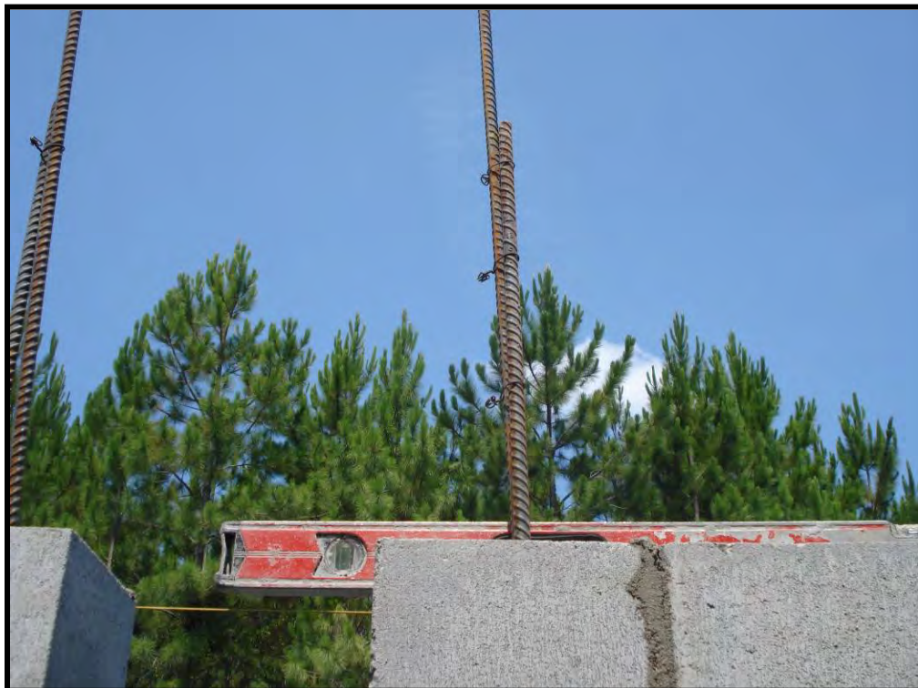
Figure B-32. Rebar splice
