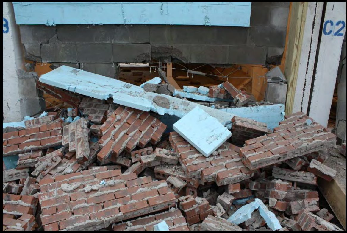
Figure C-39. Experiment 2 cavity wall panel veneer failure
