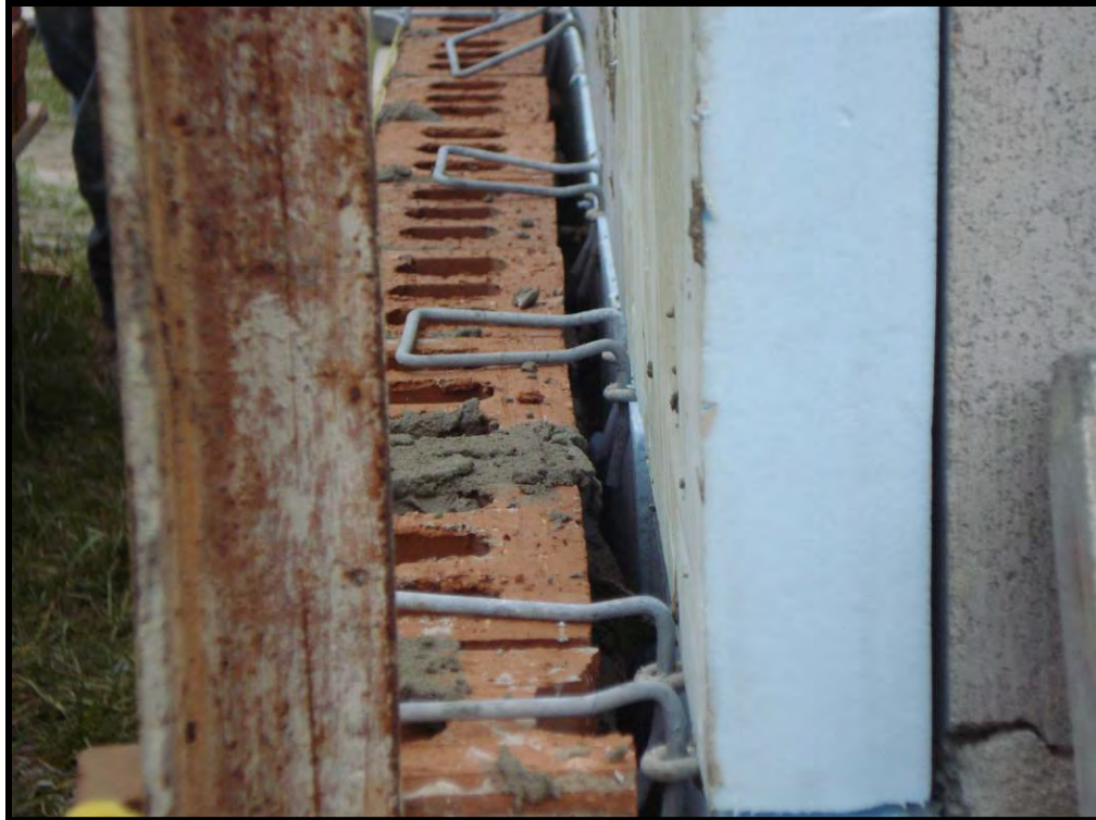
Figure B-39. Side view of veneer tie
