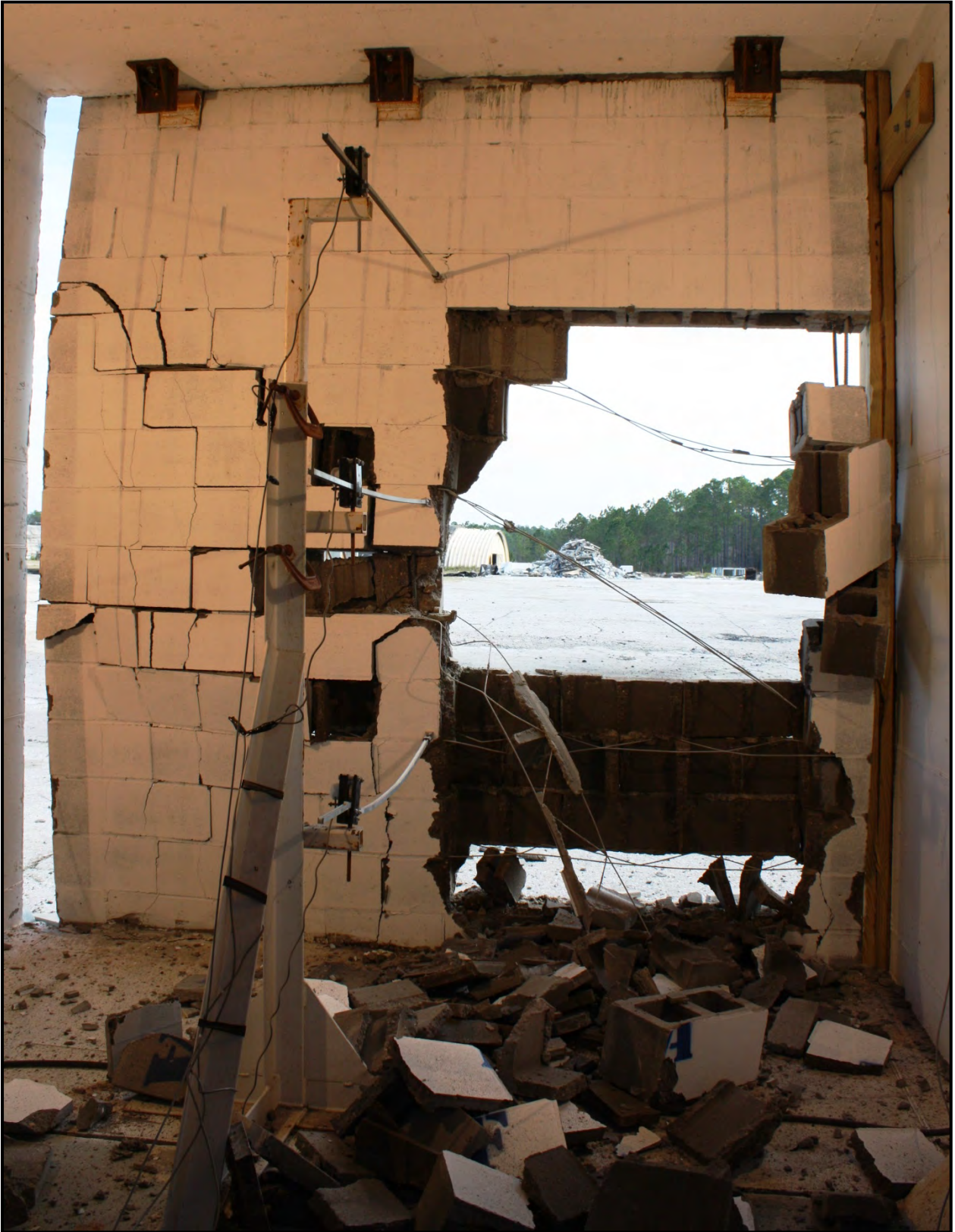
Figure C-54. Experiment 3 8-inch CMU panel full interior view
