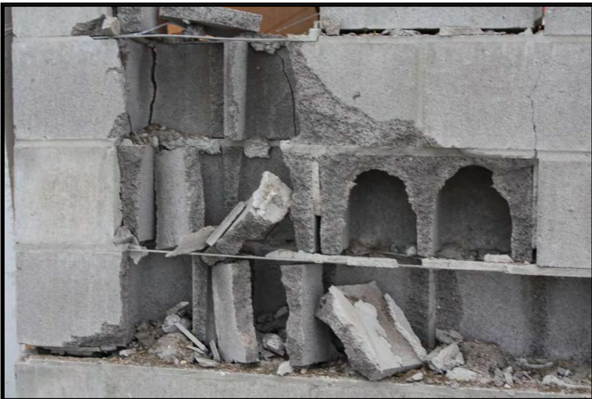
Figure C-30. Experiment 2 8-inch CMU panel exterior close-up view
