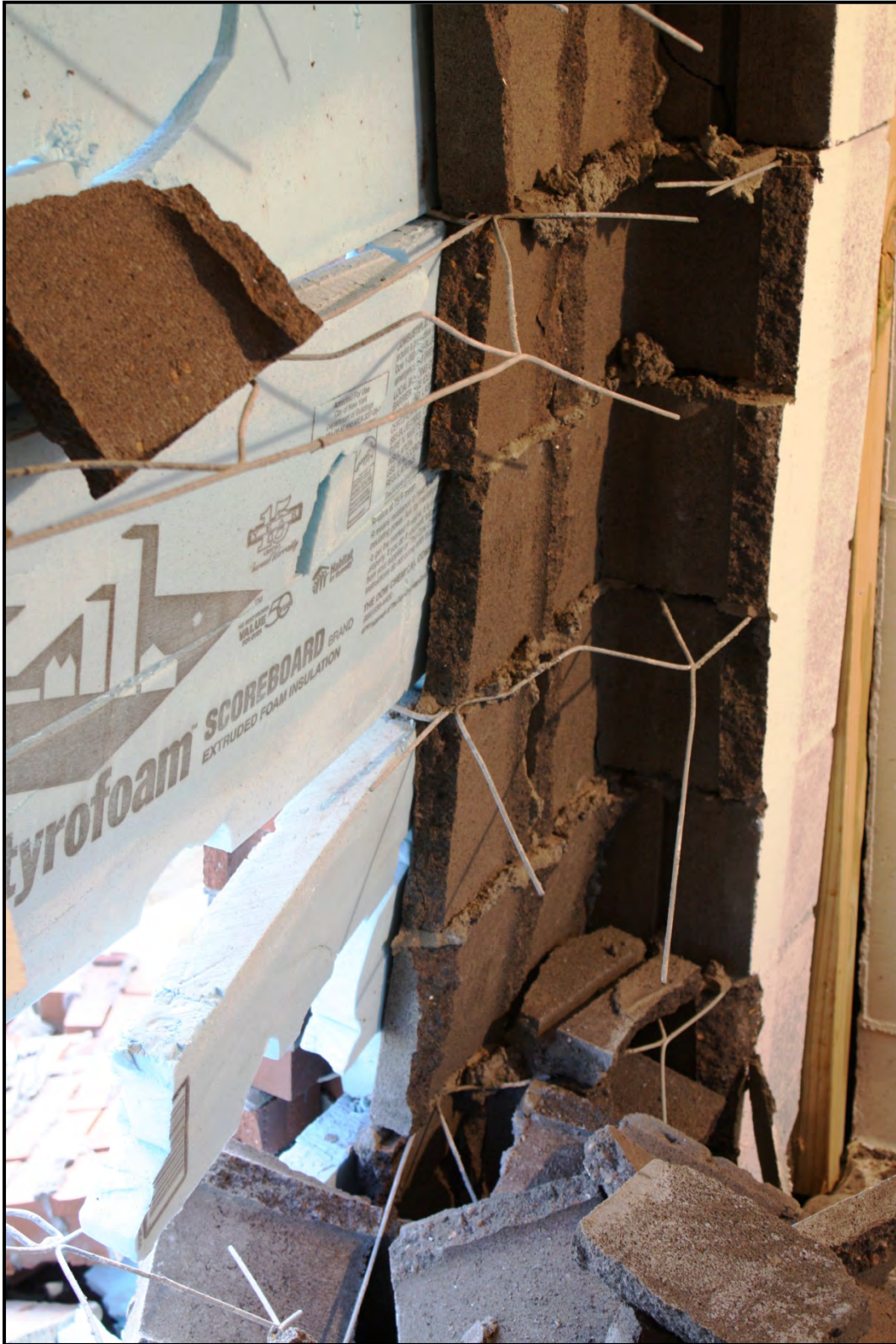
Figure C-66. Experiment 3 cavity wall panel interior close-up view
