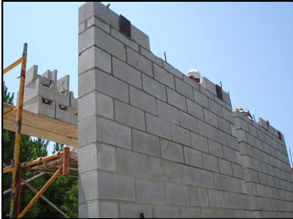
Figure B-33. Setting top bond beam
