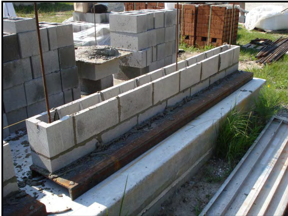
Figure B-10. Bottom bond beam
