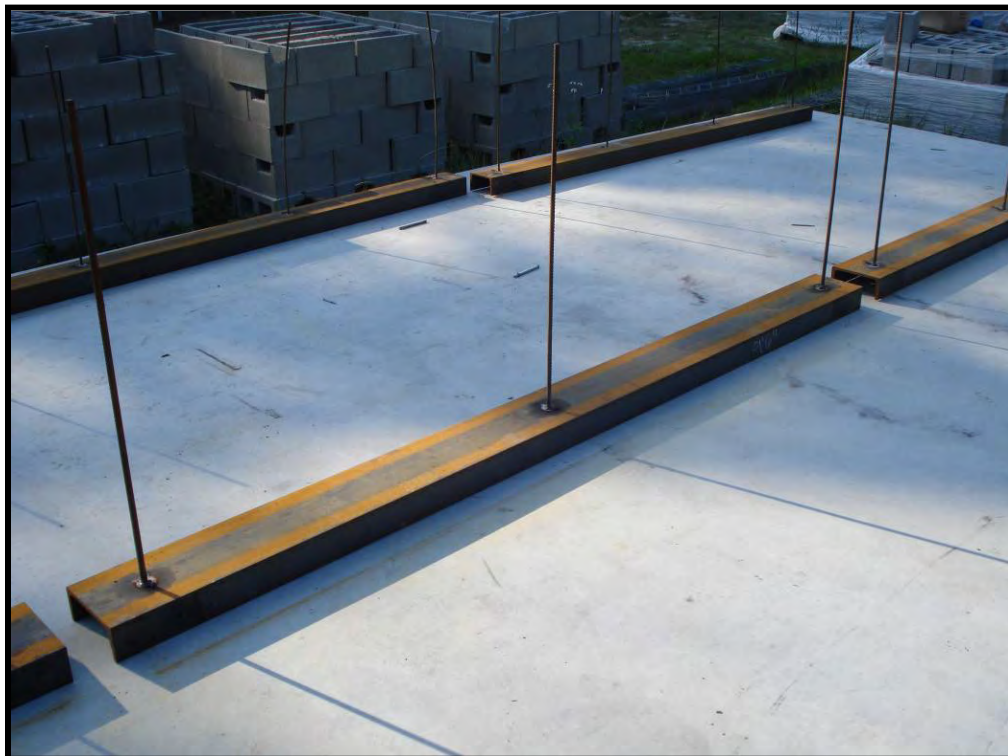
Figure B-6. Base channels with welded dowels
