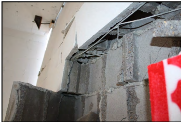
Figure 25. Experiment 1 Breaching Failure of the 8-inch CMU Panel
