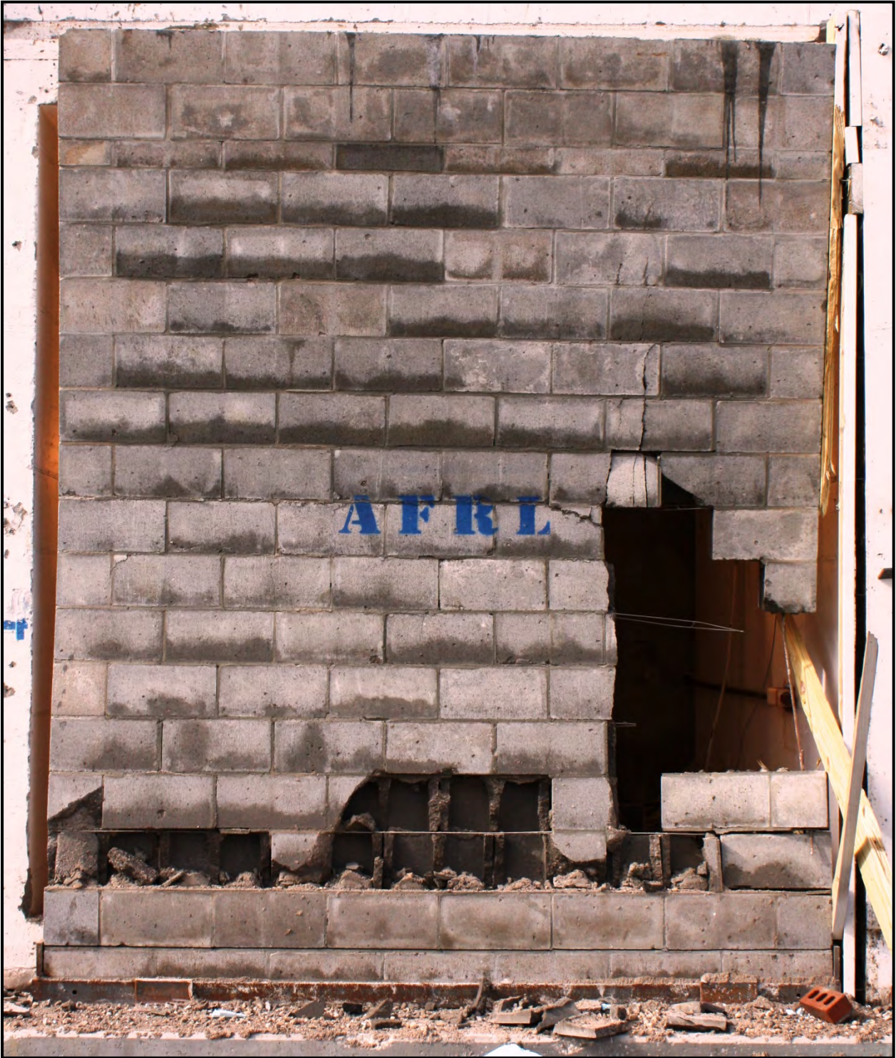
Figure C-44. Experiment 3 6-inch CMU panel exterior view
