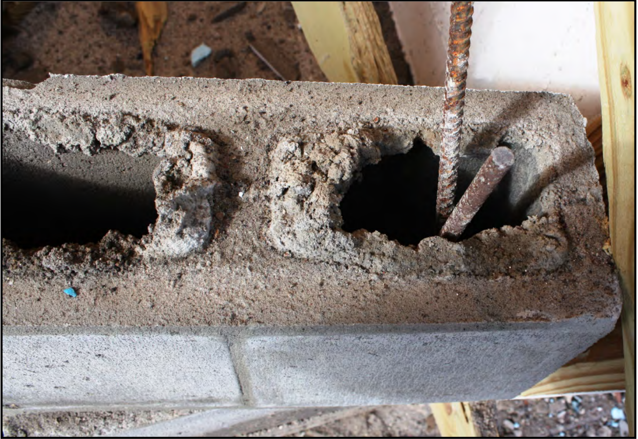
Figure C-47. Experiment 3 6-inch CMU panel close-up reinforced cells not grouted properly
