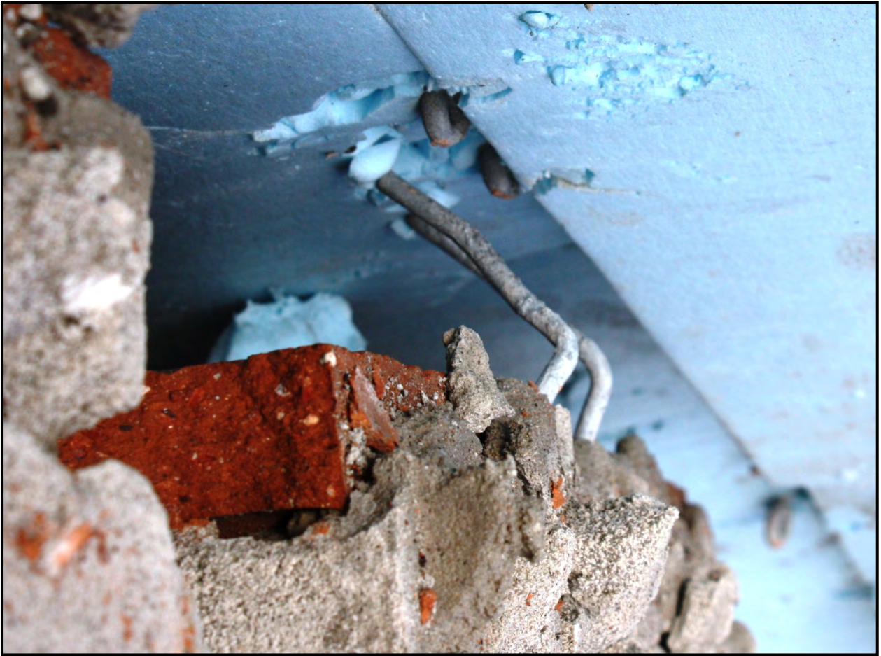
Figure C-61. Experiment 3 cavity wall panel veneer tie close-up
