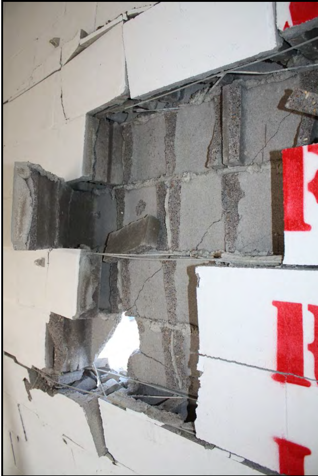
Figure C-12. Experiment 1 8-inch CMU panel close-up interior view
