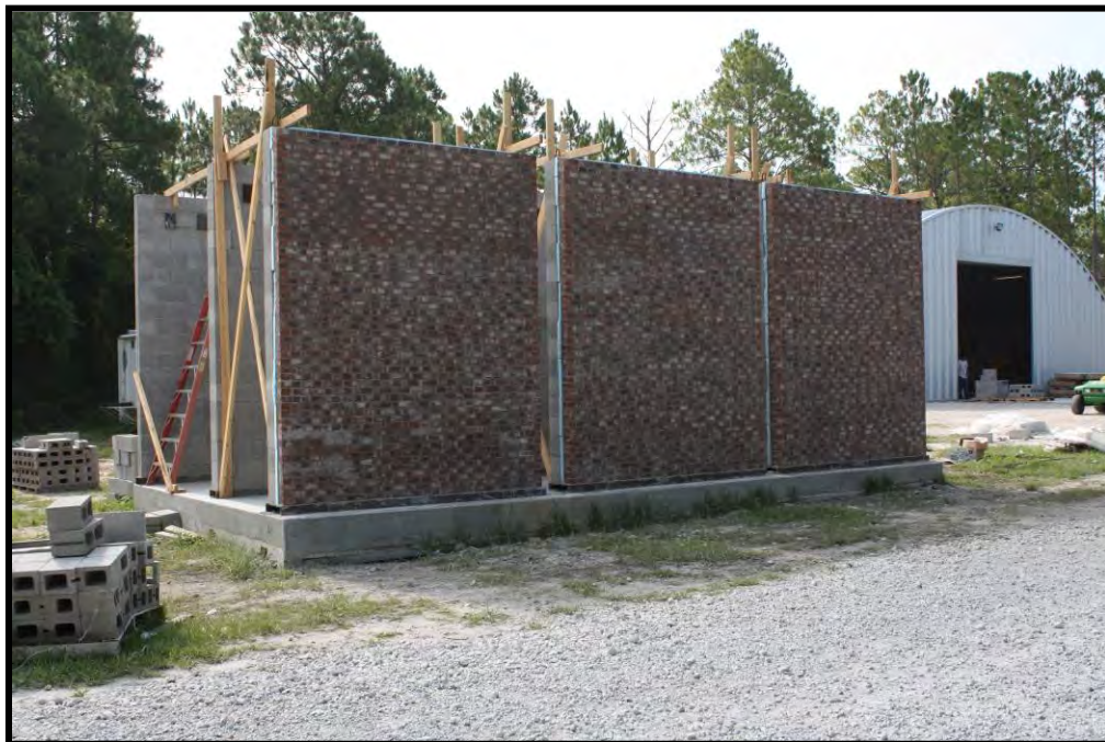
Figure B-46. Wall panel construction complete
