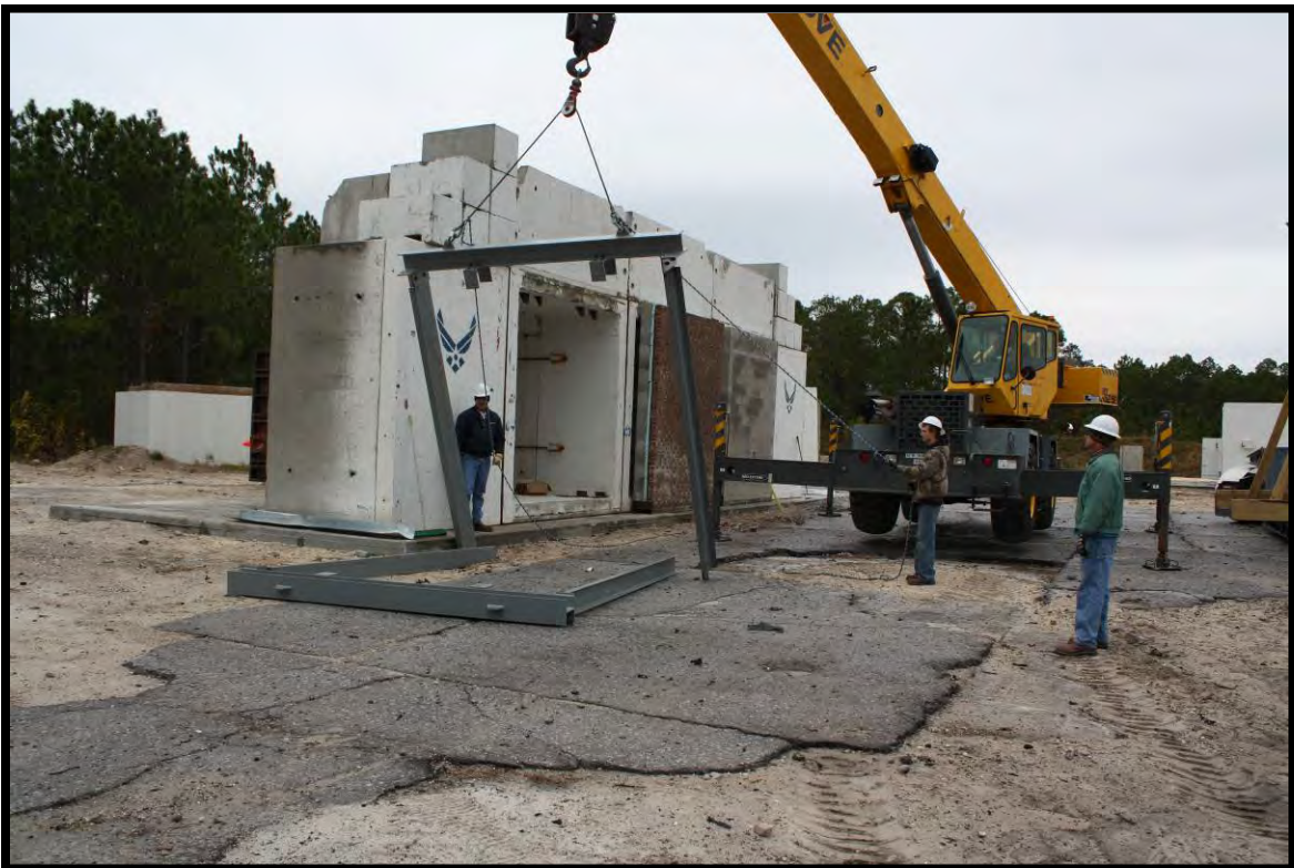
Figure B-58. Removing the stability frame
