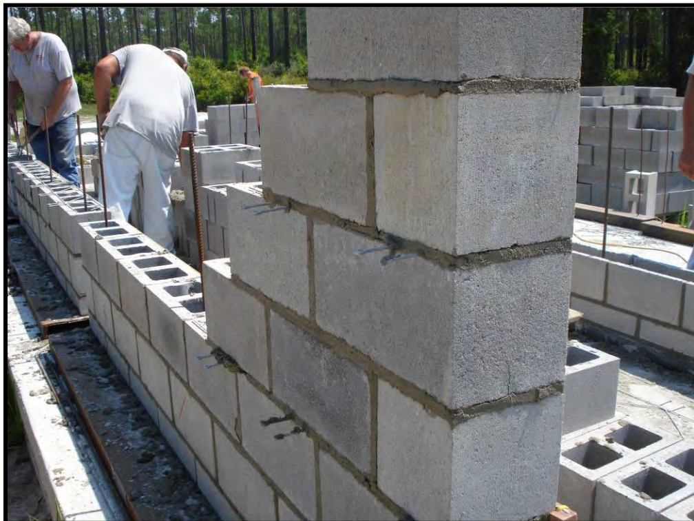
Figure B-16. Construction progressing
