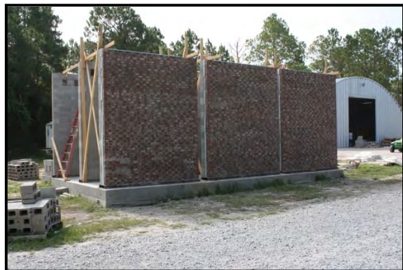
Figure 8. Construction of Test Panels (continued)
