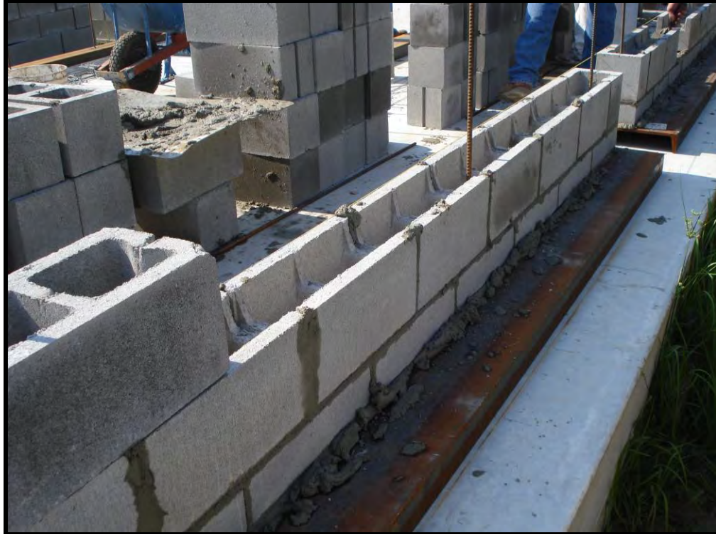
Figure B-9. Bottom bond beam
