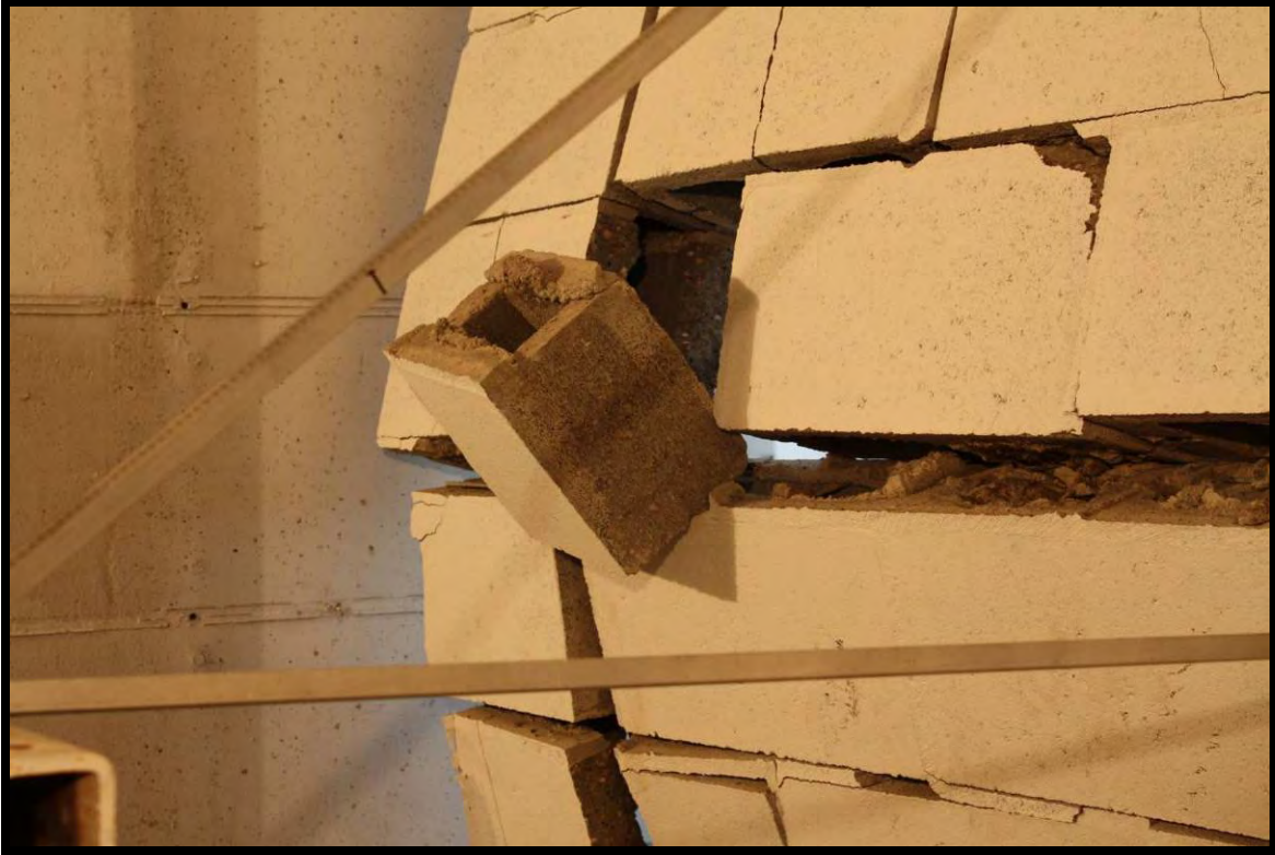
Figure C-27. Experiment 2 6-inch CMU panel interior close-up view
