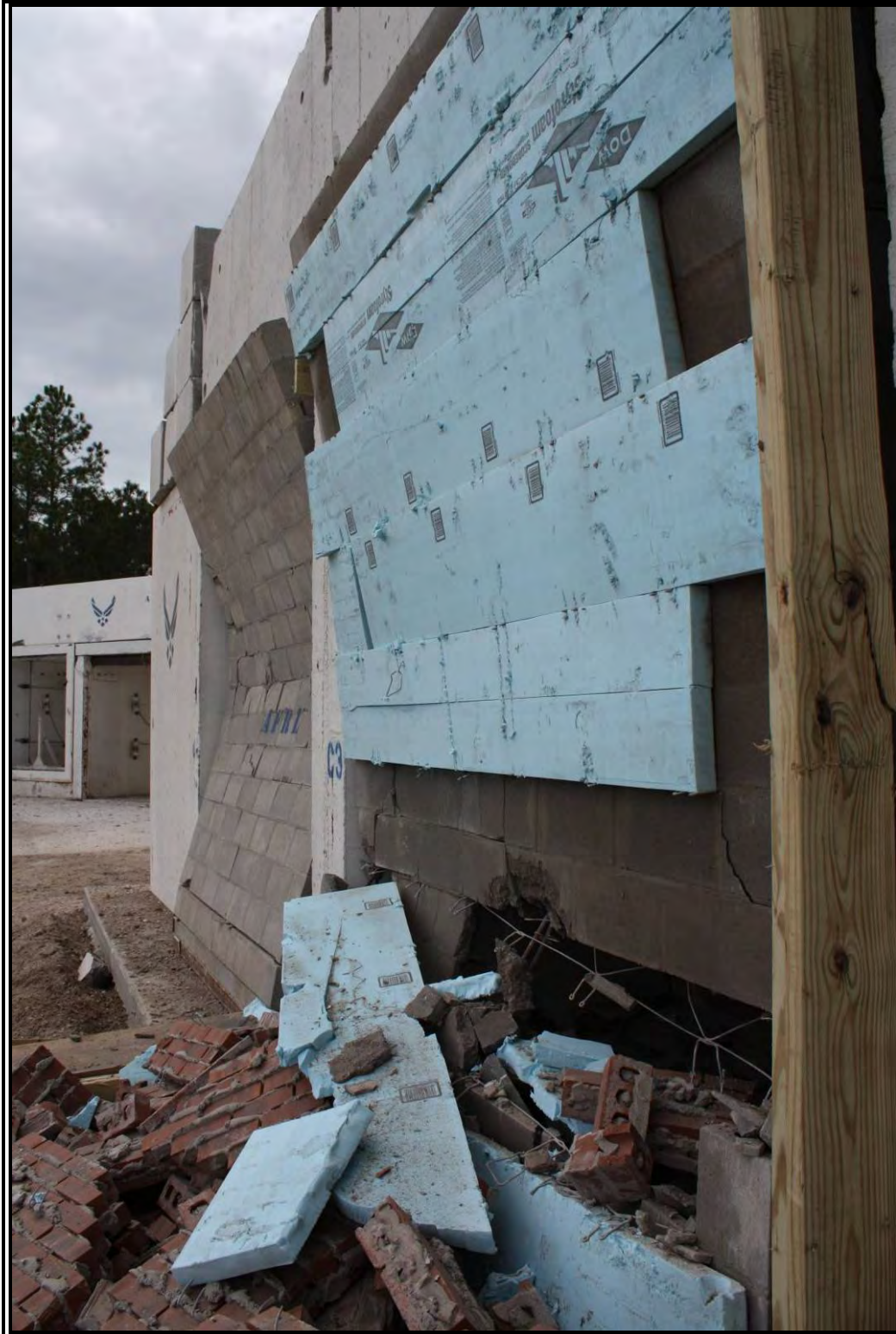
Figure C-38. Experiment 2 cavity wall panel exterior view
