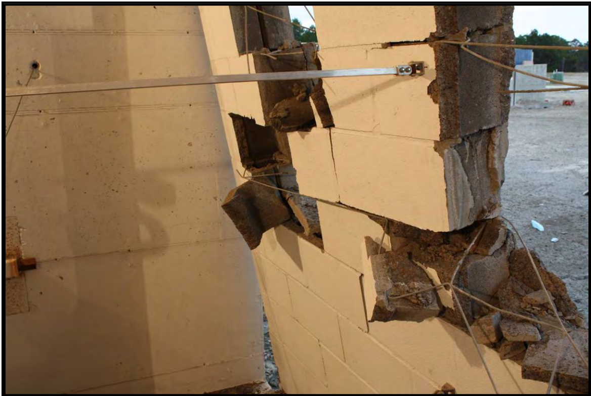
Figure C-34. Experiment 2 8-inch CMU panel interior close-up view
