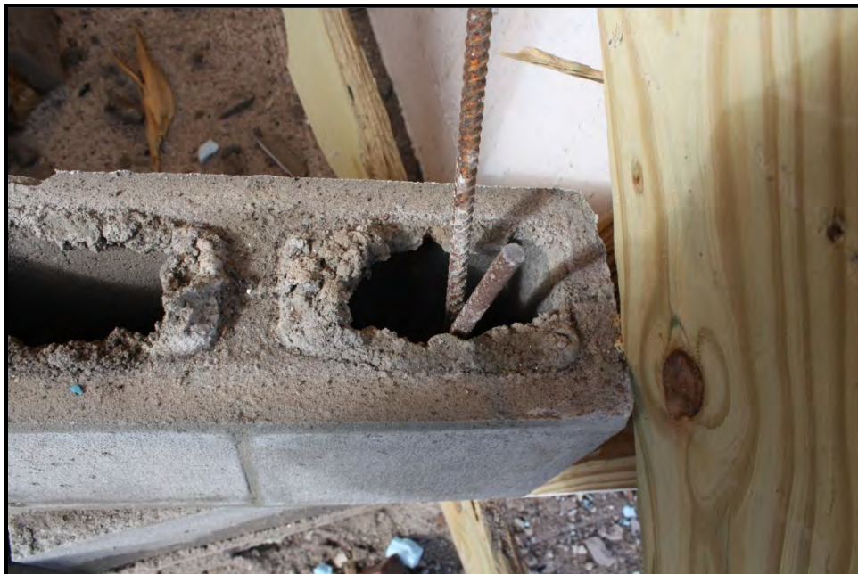
Figure 49. Experiment 3 Post-detonation 6-inch CMU Panel Close-up Views
