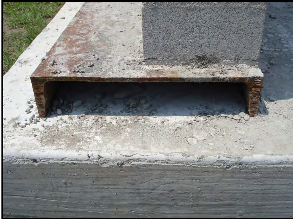
Figure B-21. Bottom view cavity wall base and channel
