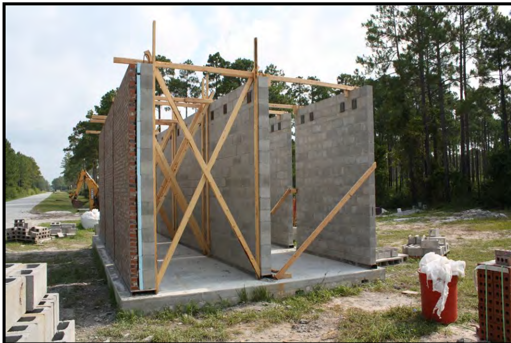
Figure B-48. Test panels complete with wind bracing
