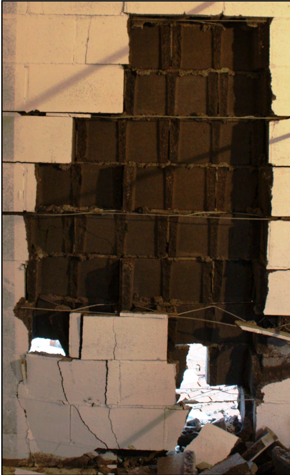
Figure C-68. Experiment 3 cavity wall panel interior view
