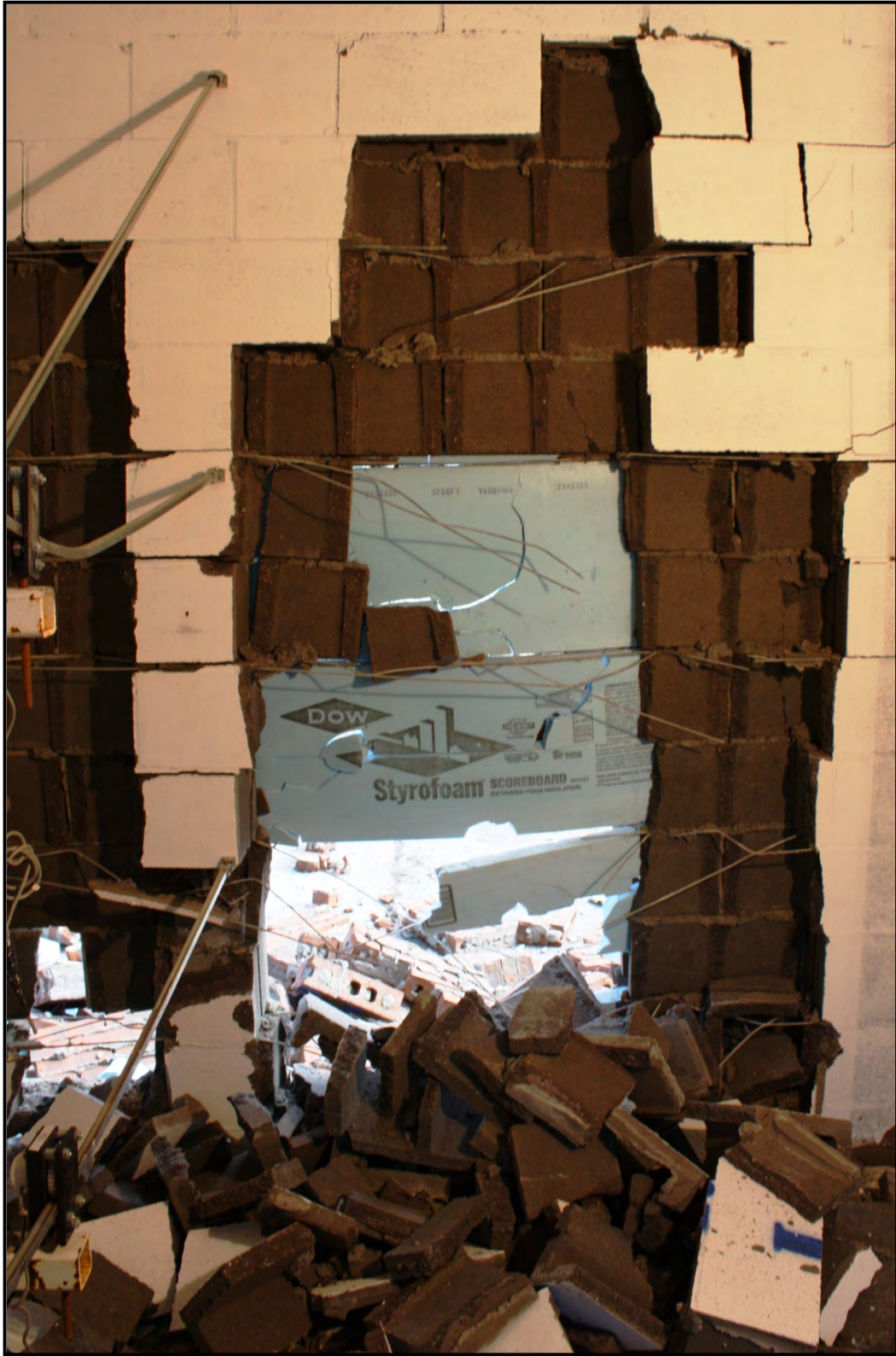
Figure C-67. Experiment 3 cavity wall panel interior view
