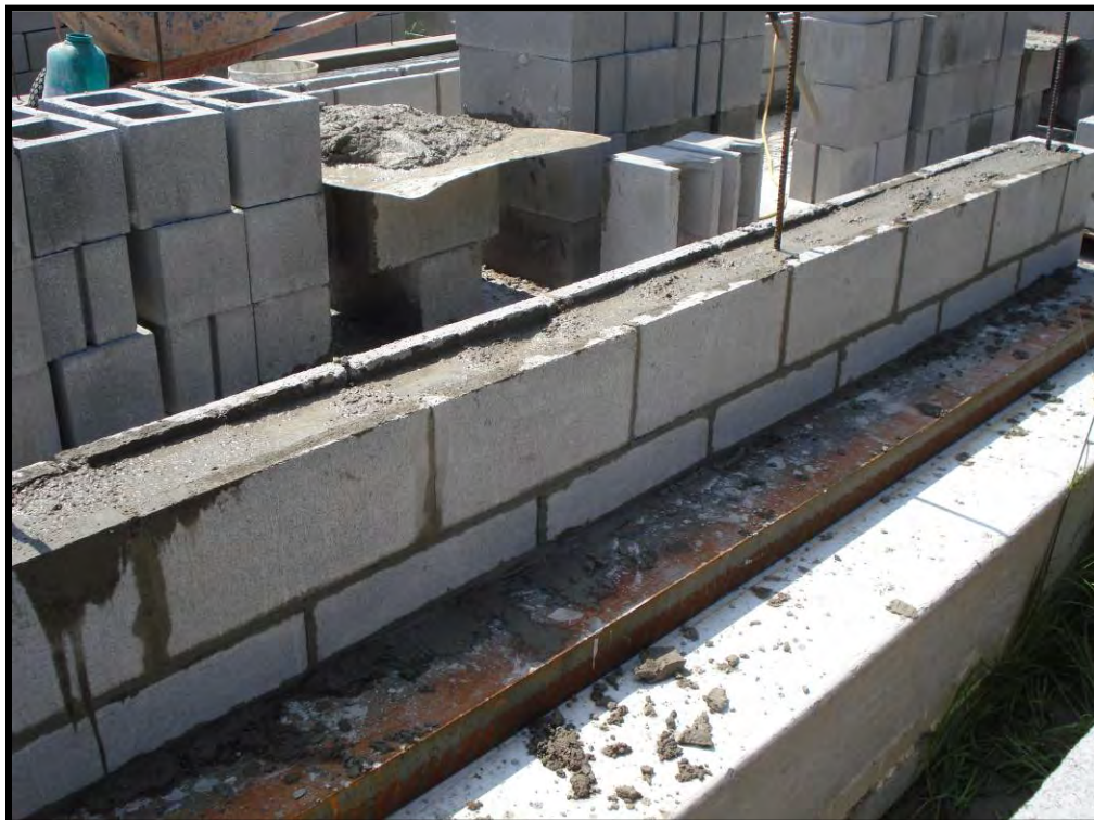
Figure B-12. Bottom bond beam grouted
