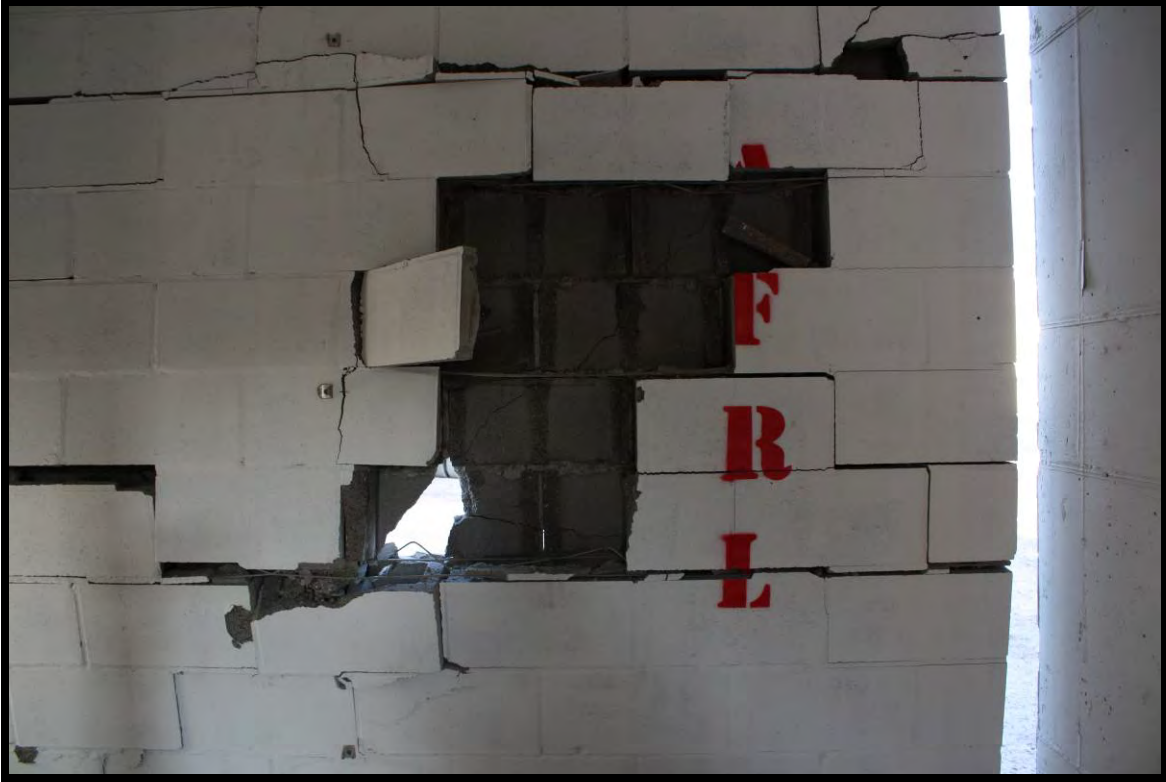
Figure C-13. Experiment 1 8-inch CMU panel partial interior view
