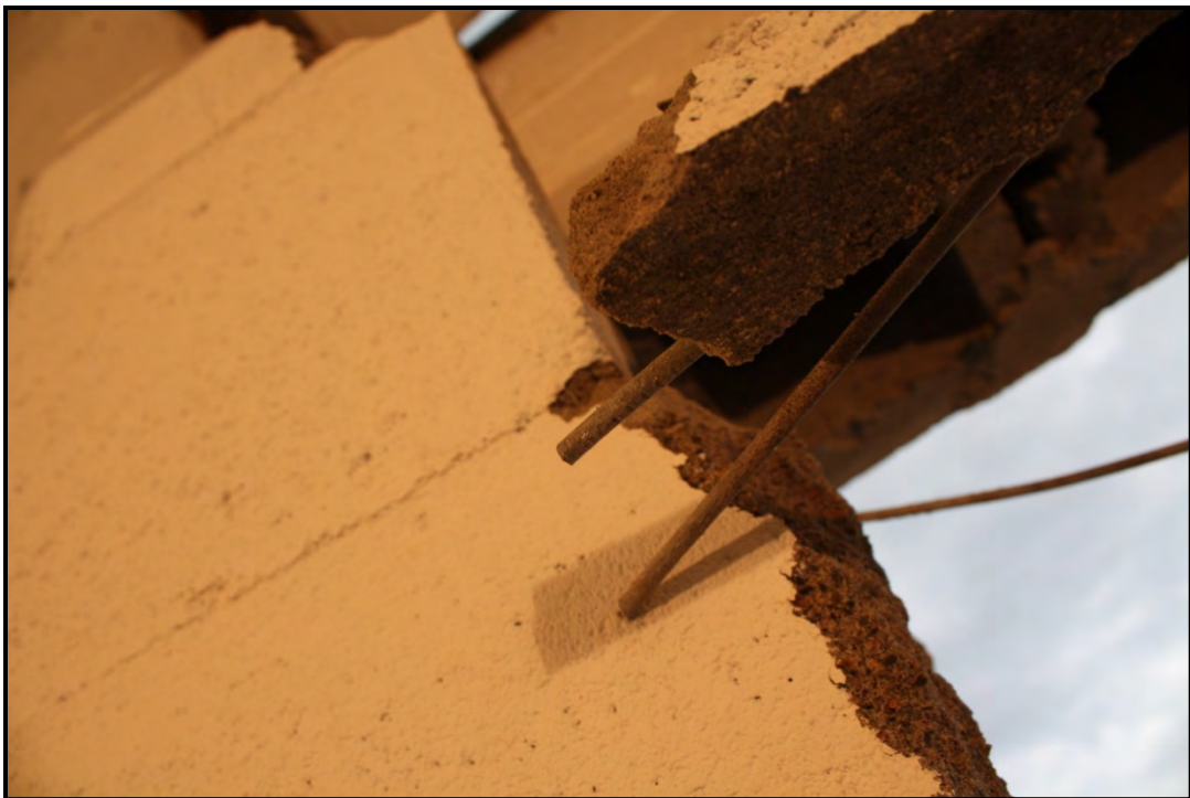
Figure 39. Experiment 2 Post-detonation 8-inch CMU Panel CMU Damage
