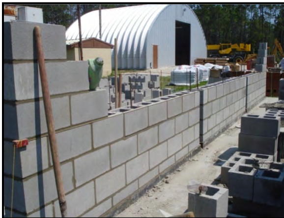
Figure 7. Construction of Test Panels
