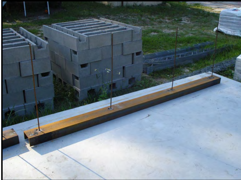
Figure B-7. Base channels with welded dowels
