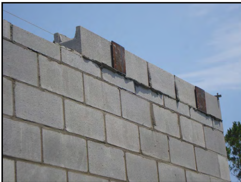
Figure B-26. Two embeds positioned
