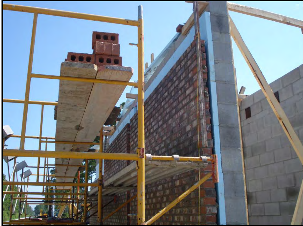
Figure B-43. Cavity wall panel construction
