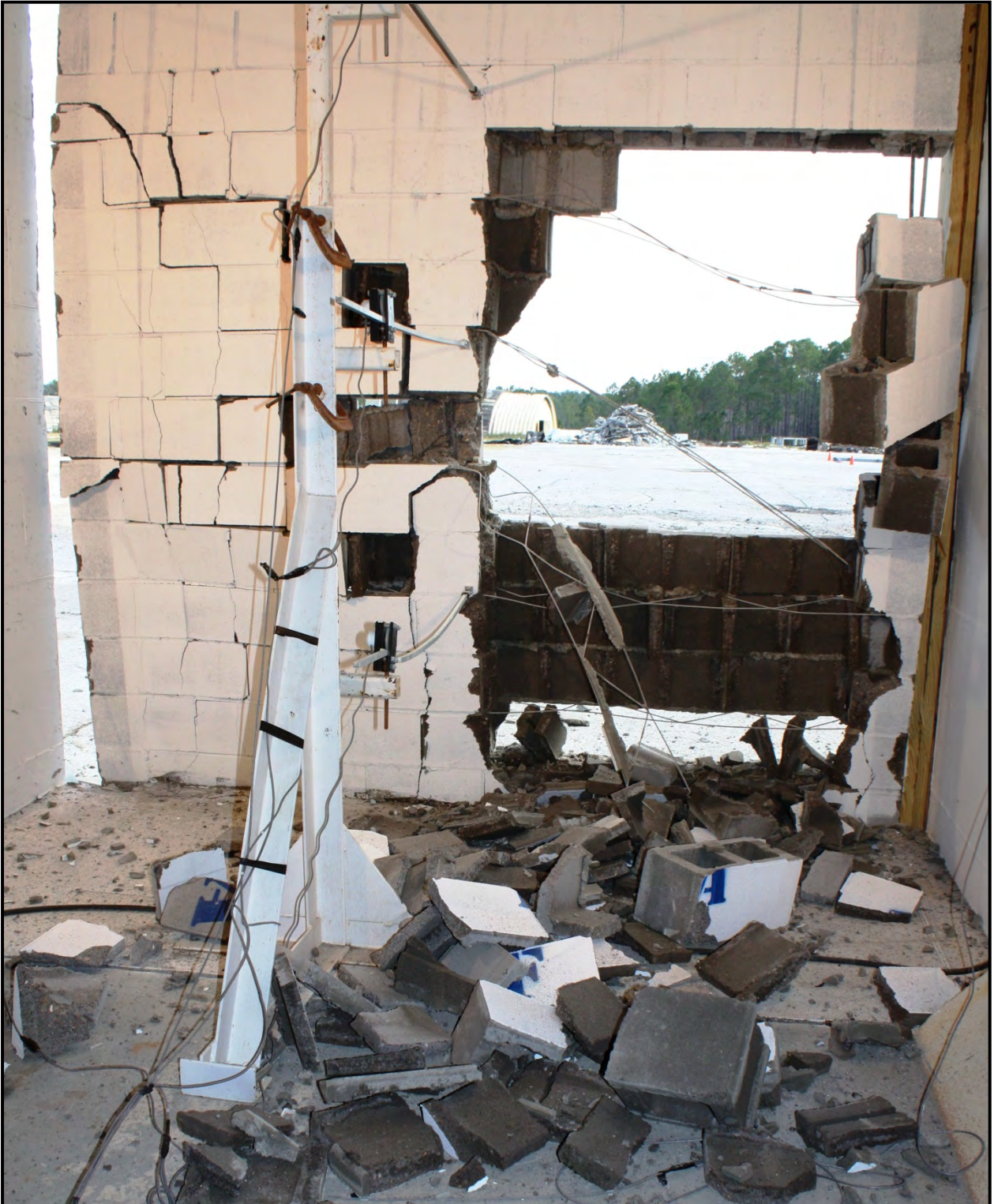
Figure C-55. Experiment 3 8-inch CMU panel full interior view
