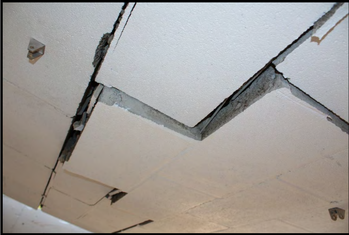
Figure C-18. Experiment 1 cavity wall panel close-up interior view
