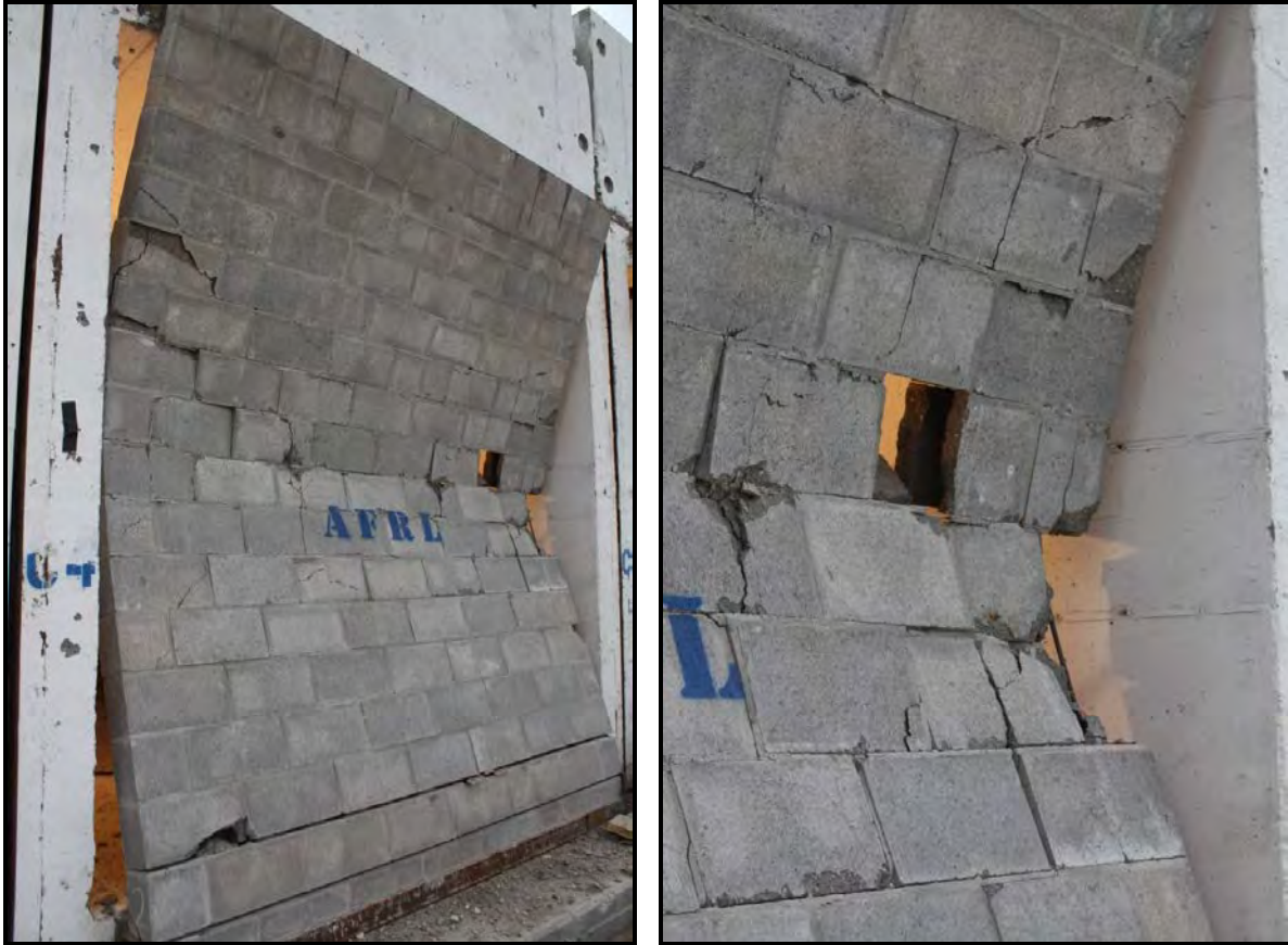
Figure 34. Experiment 2 Post-detonation 6-inch CMU Panel Closer Outside Views
