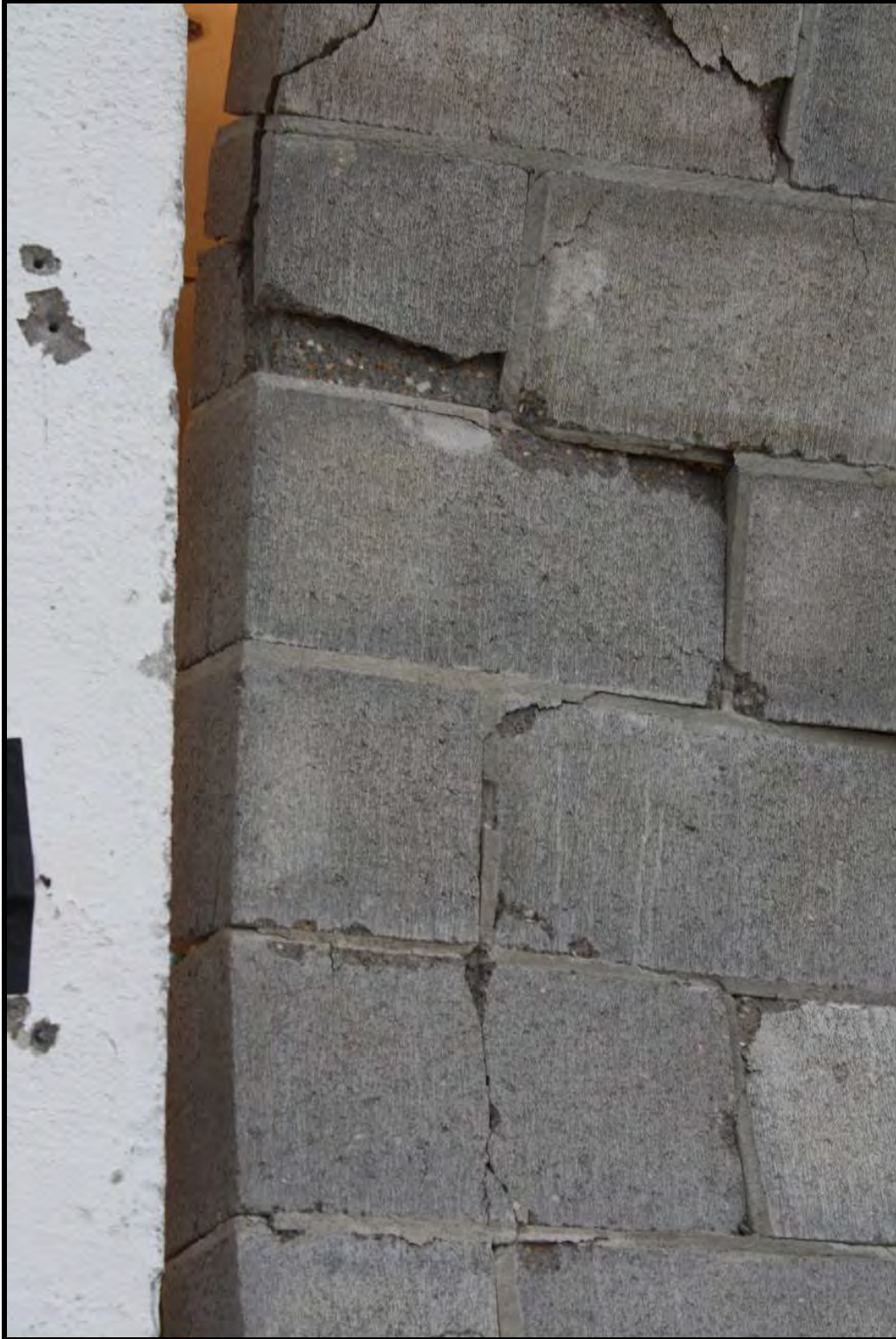
Figure C-23. Experiment 2 6-inch CMU panel left side exterior close-up view
