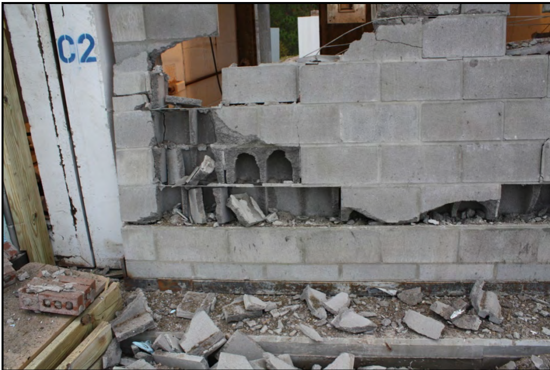
Figure 38. Experiment 2 Post-detonation 8-inch CMU Panel CMU Damage
