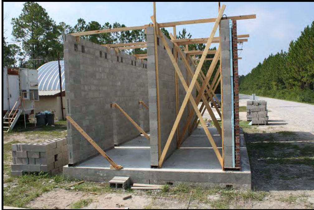
Figure B-47. Test panels complete with wind bracing
