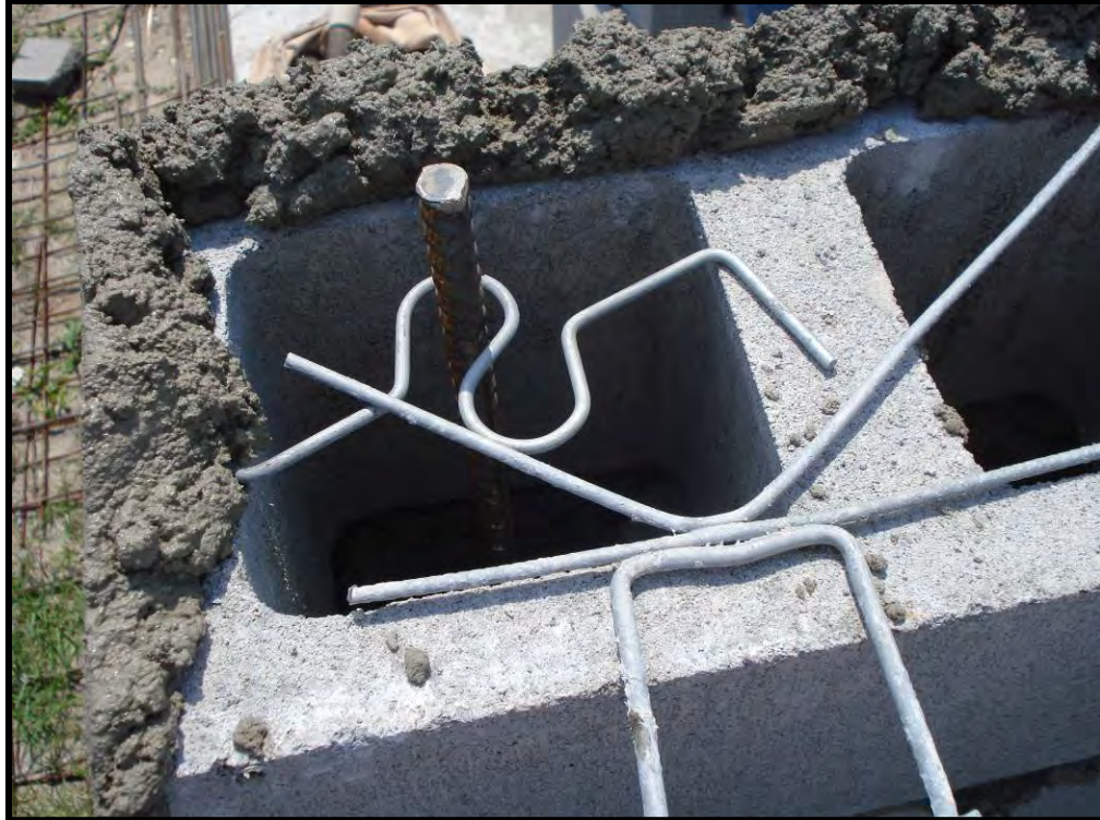
Figure B-15. Rebar positioned at end cell
