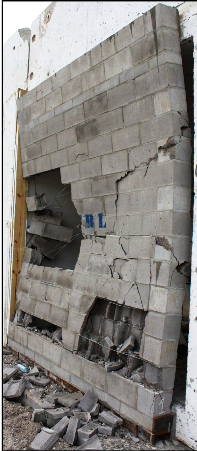
Figure C-53. Experiment 3 8-inch CMU panel right exterior view
