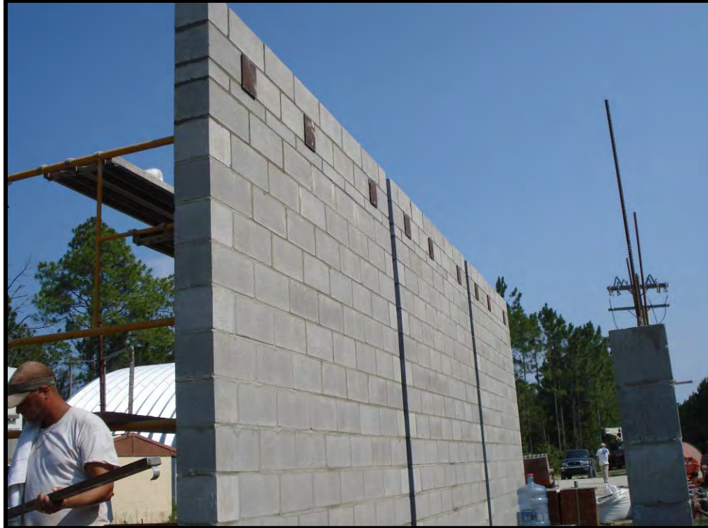
Figure B-29. Three 8-inch CMU panels complete
