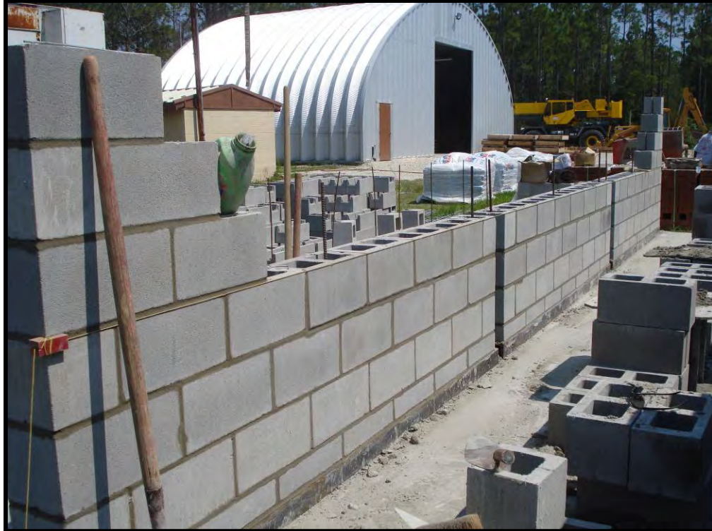
Figure B-17. Construction progressing
