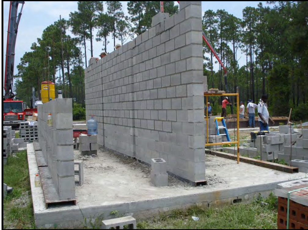
Figure B-19. 8-inch CMU panels almost complete
