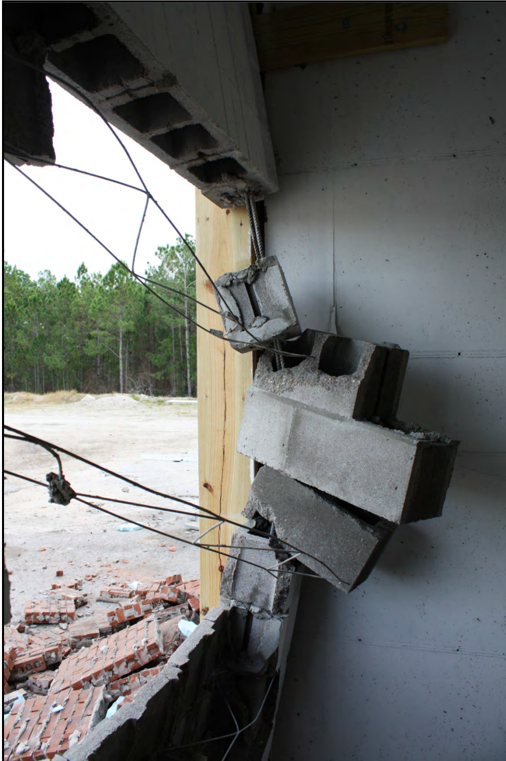
Figure C-56. Experiment 3 8-inch CMU panel breaching interior view, improperly grouted reinforced cells
