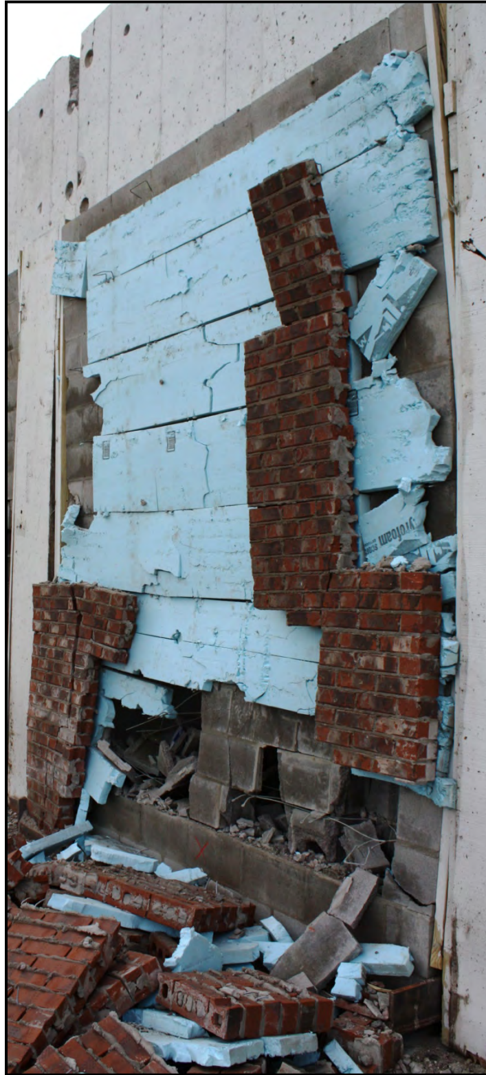
Figure C-63. Experiment 3 cavity wall panel right side exterior view
