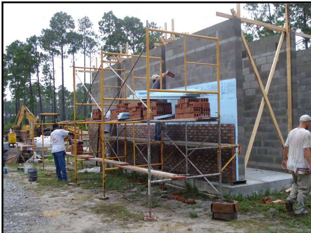
Figure B-40. Cavity wall panel construction
