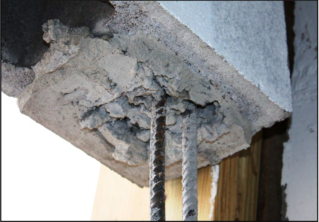
Figure C-57. Experiment 3 8-inch CMU panel breaching interior view, improperly grouted reinforced cells
