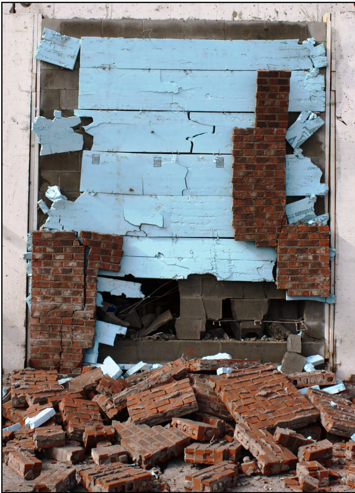
Figure C-59. Experiment 3 cavity wall panel full exterior view
