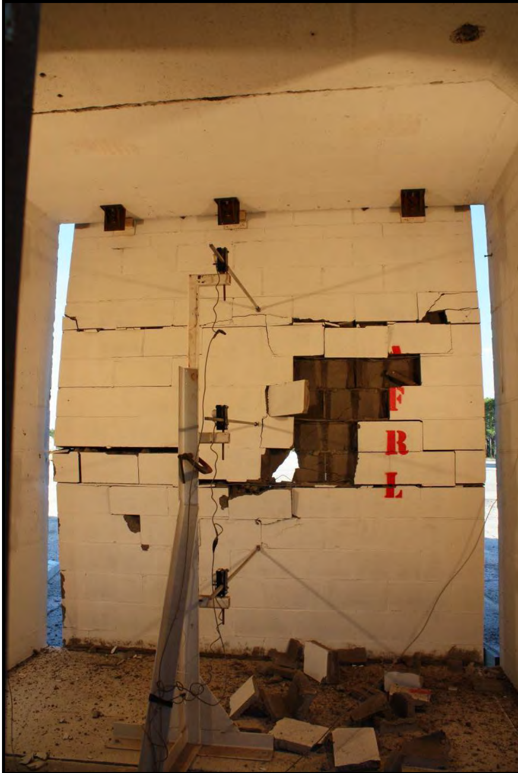
Figure C-11. Experiment 1 8-inch CMU panel full interior view
