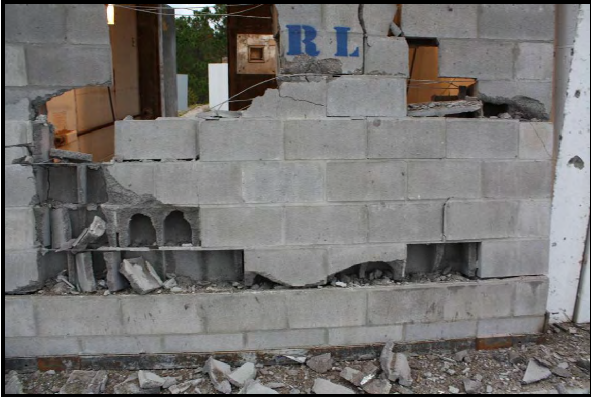
Figure C-29. Experiment 2 8-inch CMU panel exterior close-up view
