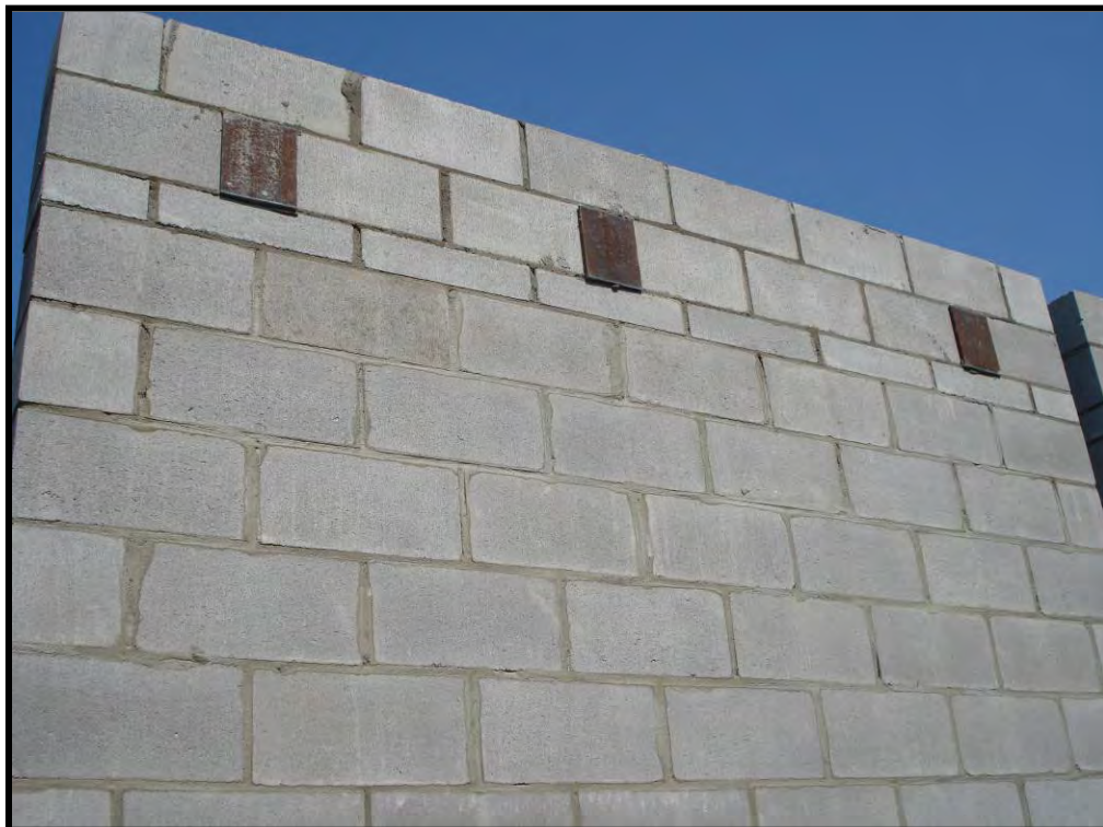
Figure B-30. 8-inch CMU panel complete
