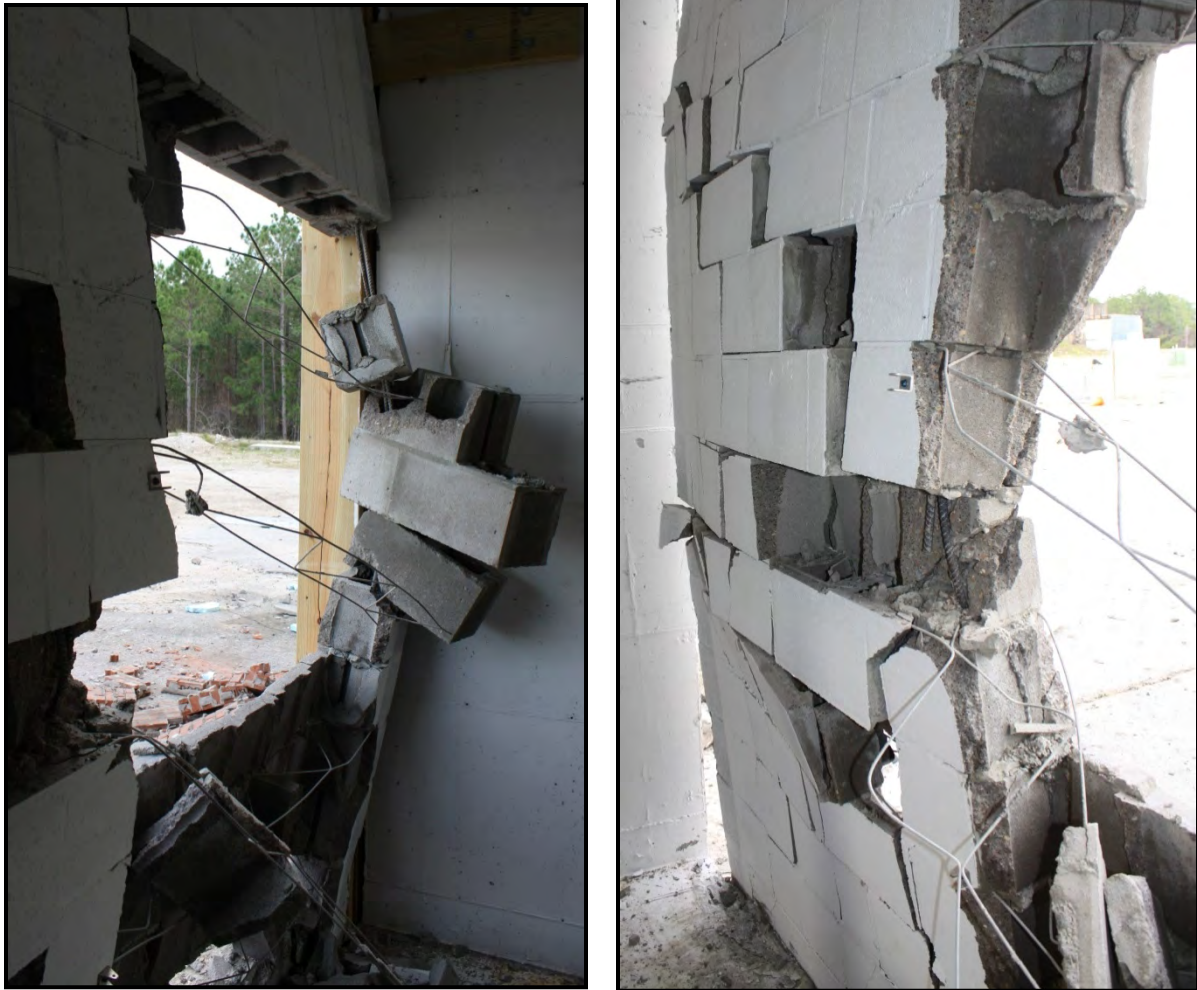
Figure 54. Experiment 3 Post-detonation 8-inch CMU Panel Close-up Interior Views
