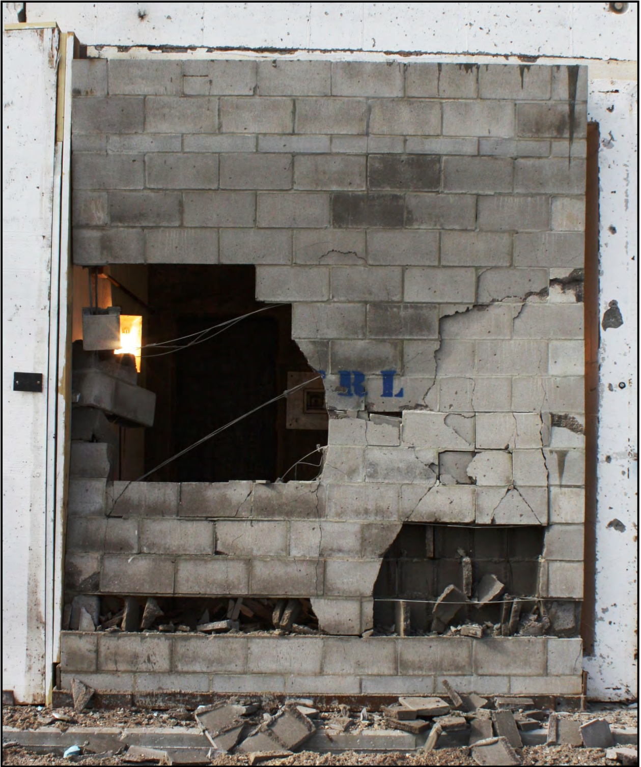
Figure C-50. Experiment 3 8-inch CMU panel full exterior view
