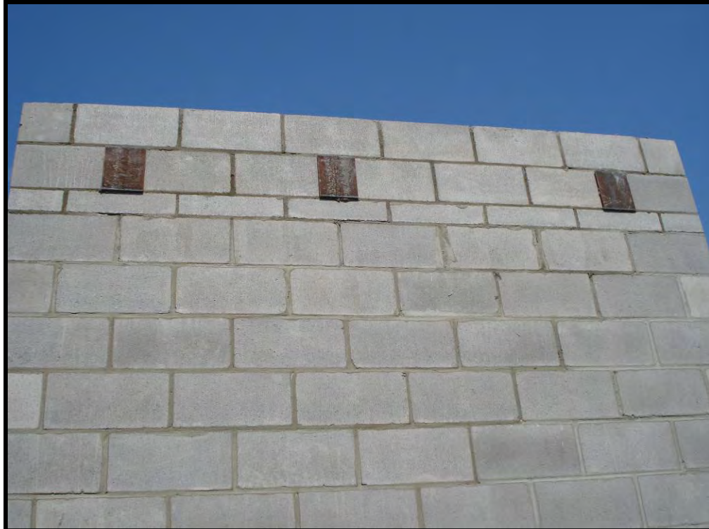
Figure B-31. 8-inch CMU panel complete
