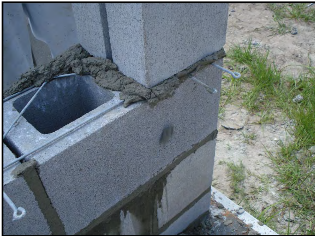
Figure B-14. End bed joint
