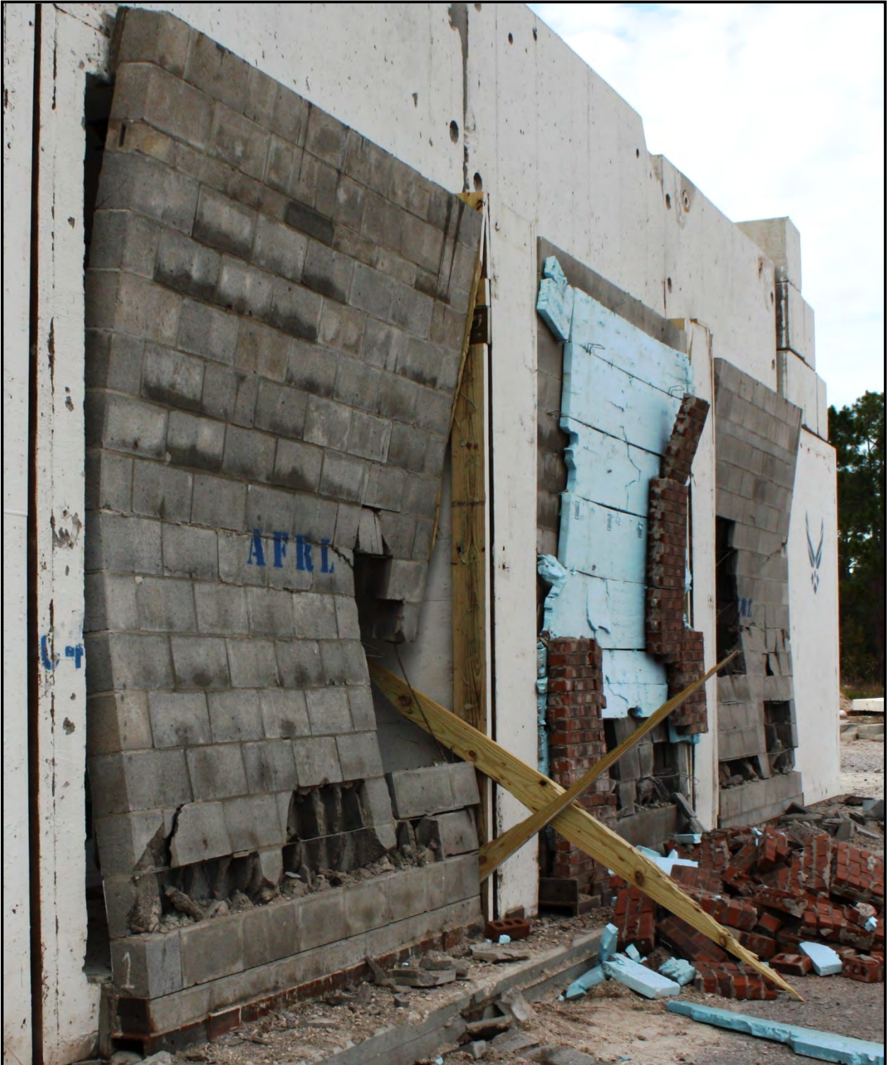
Figure C-43. Experiment 3 full exterior left side view
