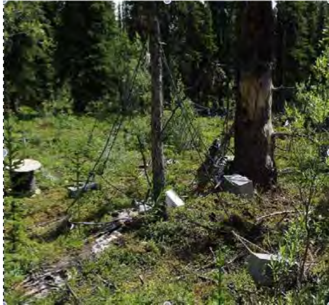
Figure 7: Photograph of ELF/VLF receiver as installed at Paradise, Alaska to detect the ELF/VLF signals generated by the HAARP HF
