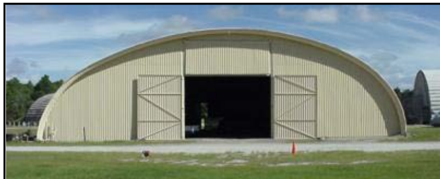
Figure 1. Fire Hangar at Tyndall Air Force Base
