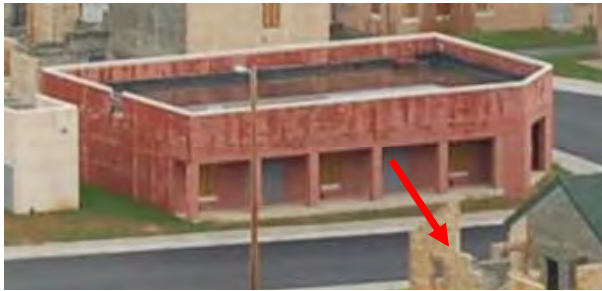
Runs 125-136 (Level Concrete x 3 Heights x 2 Landings)
