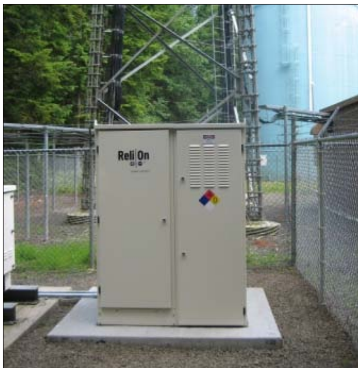
RELION FUEL CELL BACKUP POWER SYSTEM, SPRINT CELL PHONE TOWER COURTESY OF FUEL CELL AND HYDROGEN ENERGY ASSOCIATION
