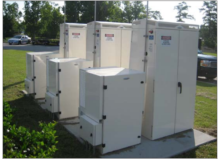
PLUG POWER FUEL CELL BACKUP POWER SYSTEM, FORT JACKSON, COLUMBIA, SC COURTESY OF LOGANENERGY
