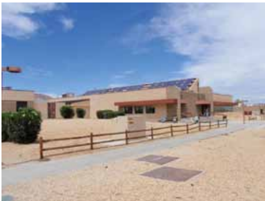
Figure 37. Dining Facility (Bldg 254).
