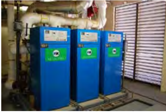
Figure 7. Patterson Kelley Boilers in Central Energy Plant 263.
