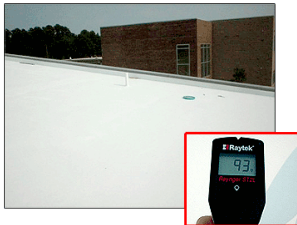
Figure 33. Decreased roof temperature with cool roof material.
