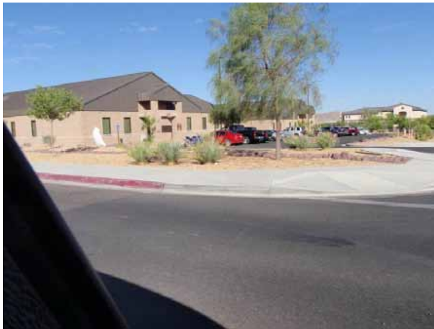
Figure 30. Building with brown roof.
