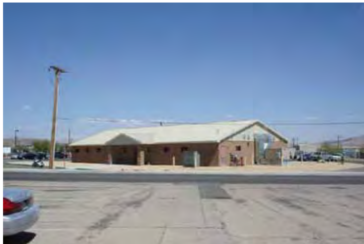
Figure 31. Building with light roof.
