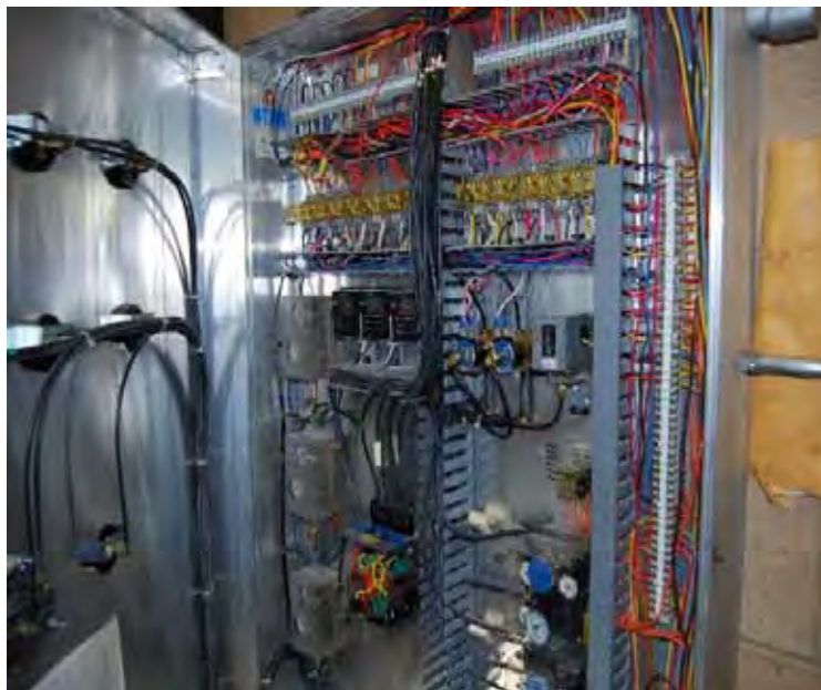
Figure 35. Controls for multi-zone AHU.
