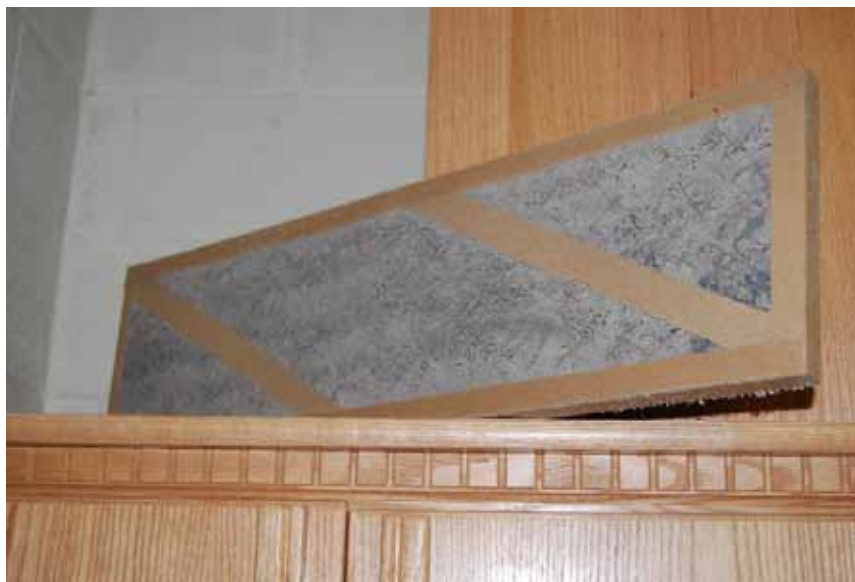
Figure 3. Dirty filter from fan coil unit at Bldg 264.
