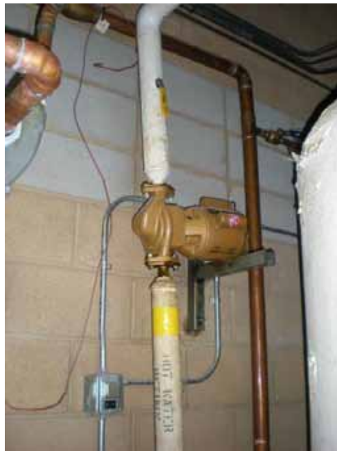
Figure 9. Hot water circulating pump.
