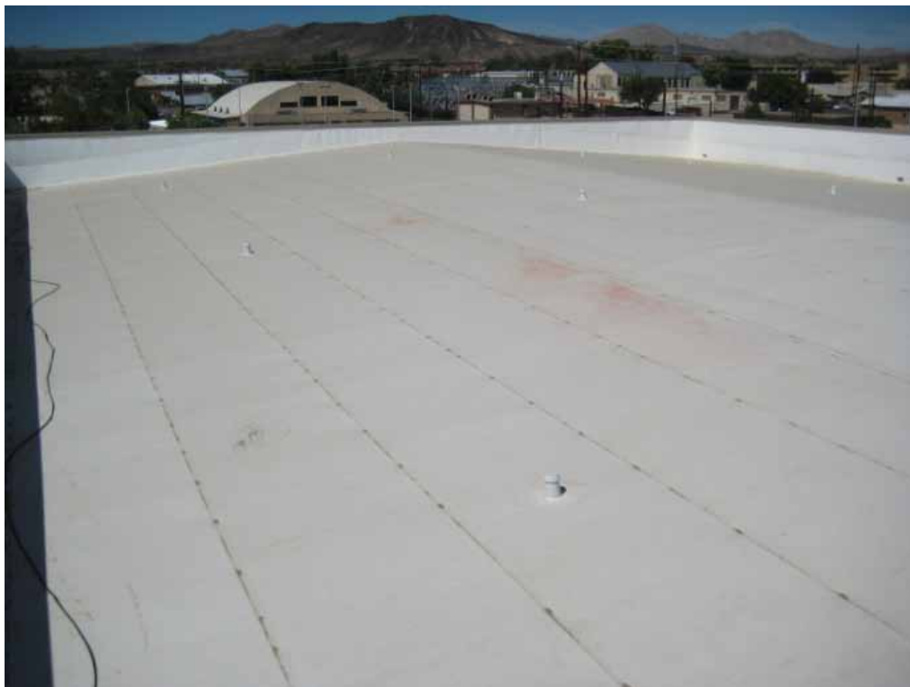
Figure 41. Roof of Bldg 362.
