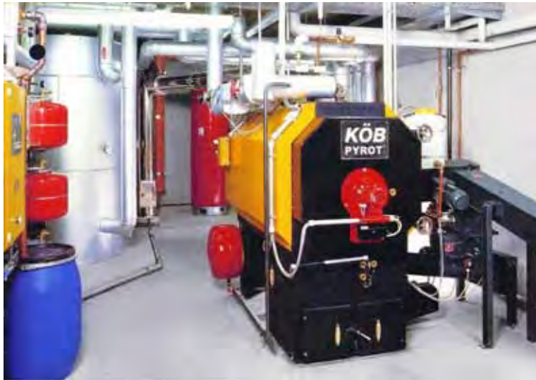
Figure 21. Example biomass system mechanical room.
