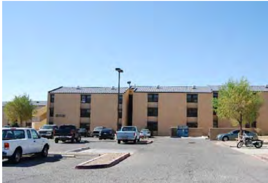
Figure 1. Bldg 265 (identical to Bldg 264).
