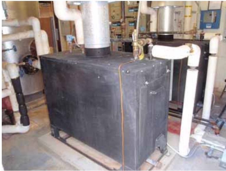
Figure 36. Boiler with 140 °F sides and top (Bldg 254).
