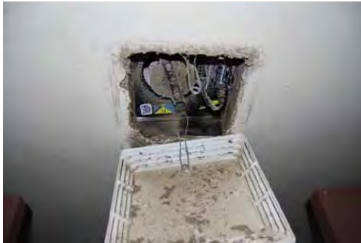
Figure 4. Bathroom exhaust fan at Bldg 264.
