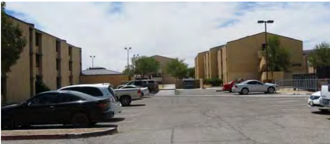
Figure 11. Building Cluster (Bldgs 261–267, 271).
