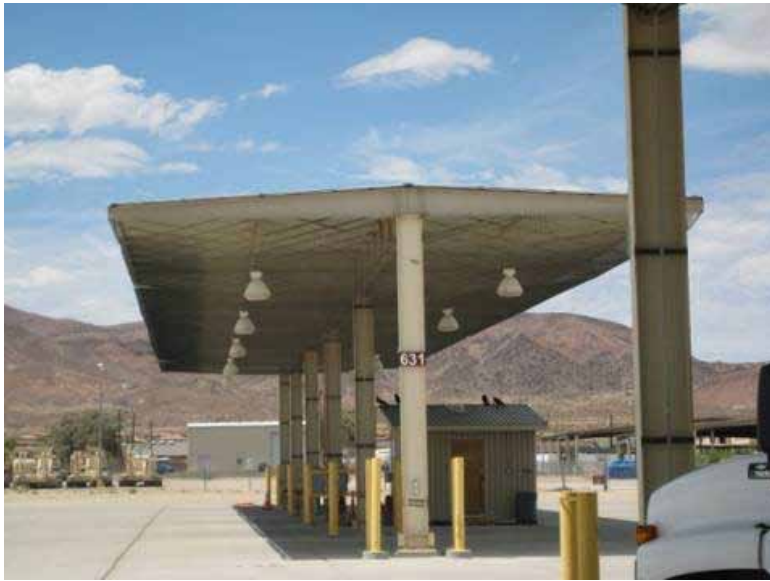
Figure 49. RUFMA shading structure.
