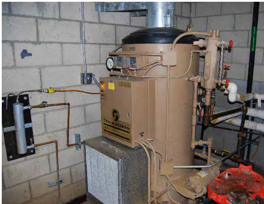
Figure 6. Steam boiler at Dining Facility 271.
