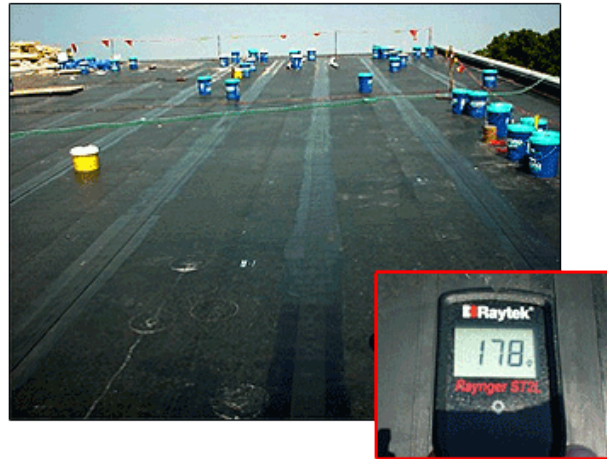
Figure 32. Roof before treatment; thermometer reads 178 °F.
