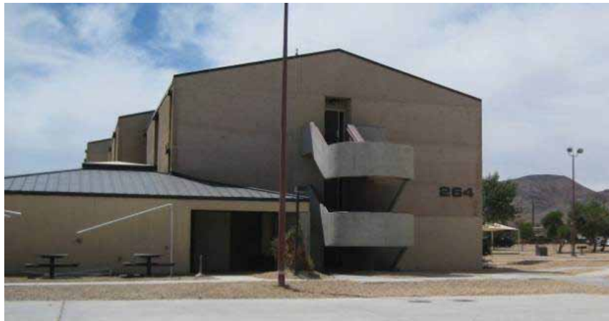
Figure 28. Typical Barracks (Bldg 264).
