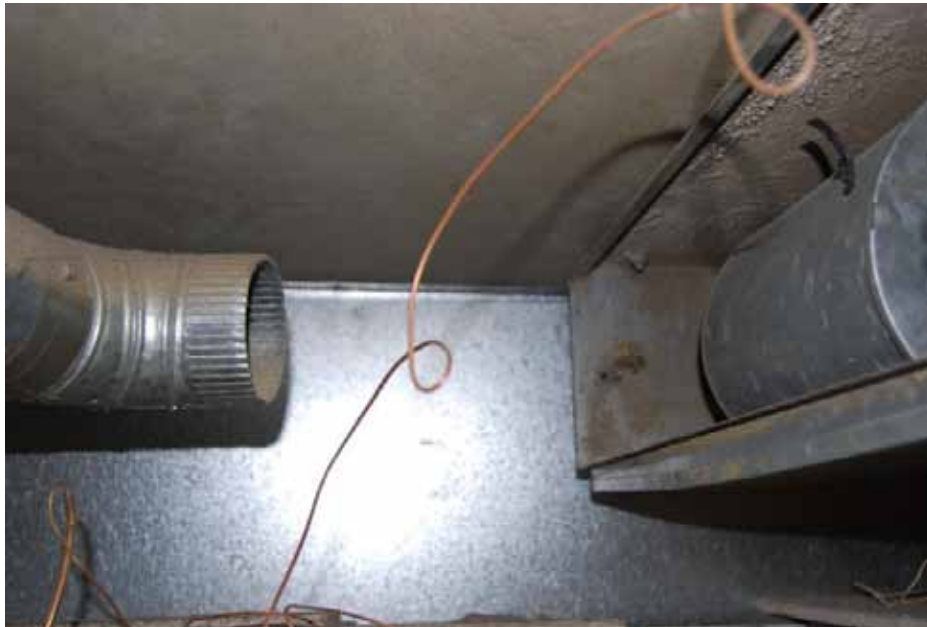
Figure 2. Fan coil return air plenum at Bldg 265.
