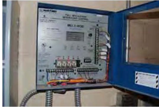
Figure 8. Central Energy Plant 263 — heater timer for temperature control.
