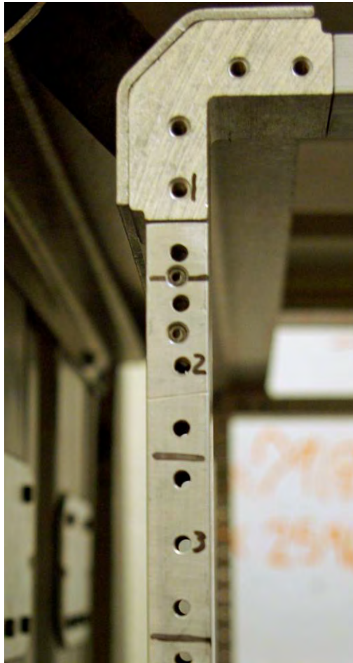
Figure 35. Horizontal Markings with Easy to Reference Numbers Every 1 U
