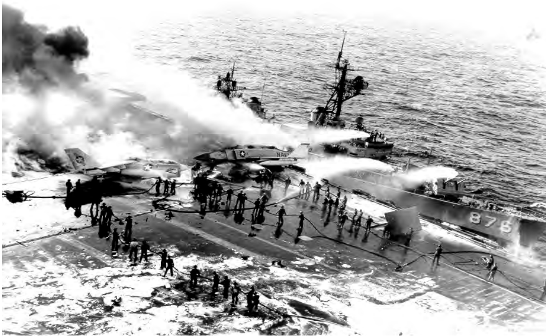
Figure 8. Firefighting Efforts aboard the USS Enterprise (From Leonhardt, 1969)
