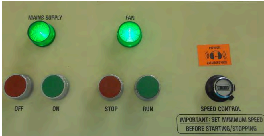
Figure 23. Wind Tunnel Control Panel
