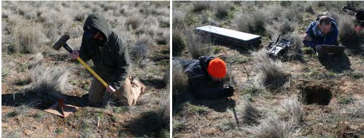
Figure 7. Rut Formation and Down-Hole Magnetic Susceptibility Measurements as Part of the Field Compaction Tests
