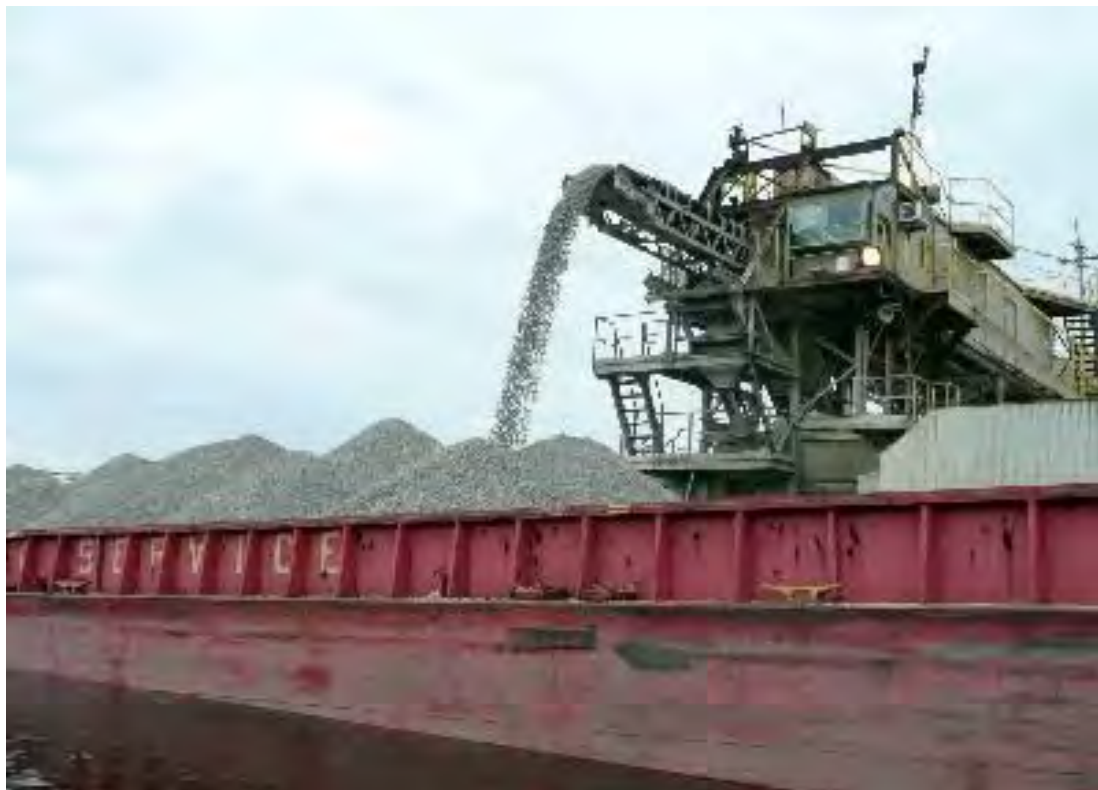
Figure B-2. Interior of empty hopper barge (upper). Loading hopper barge (lower).
