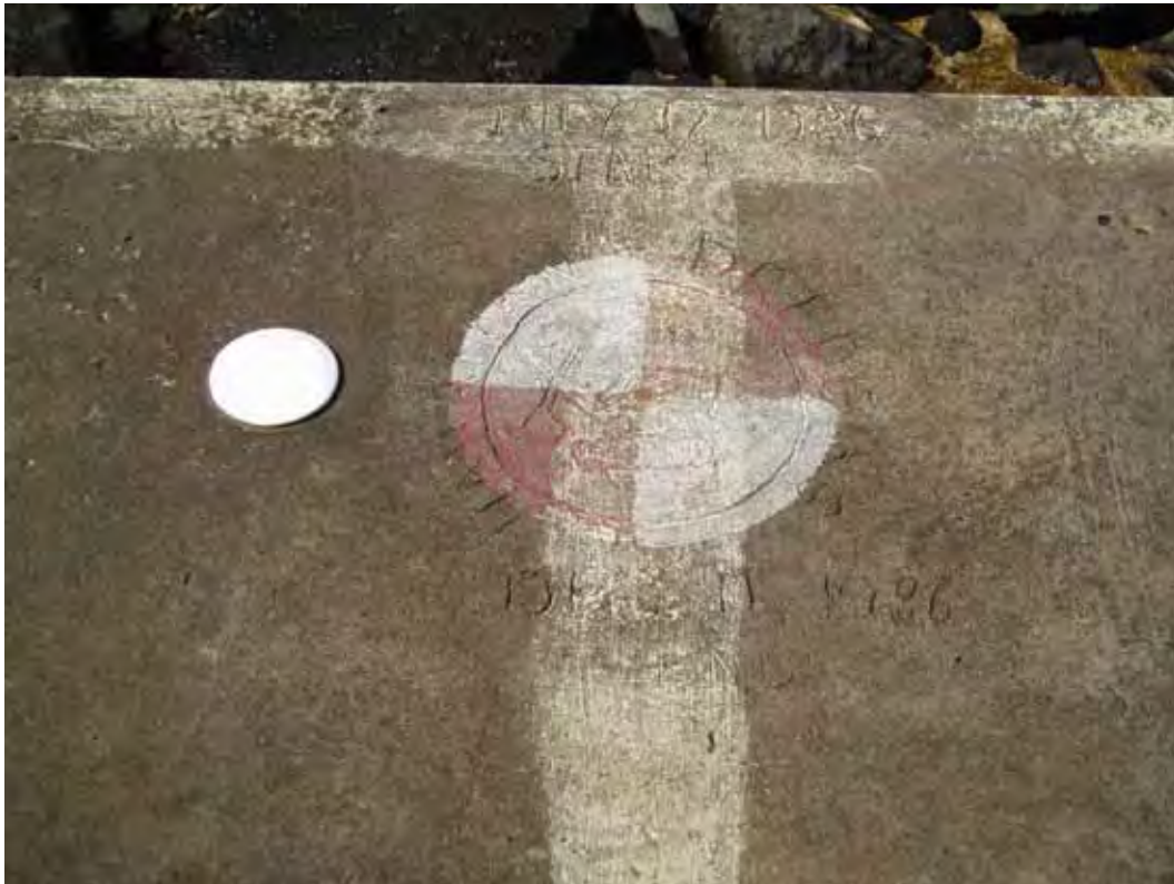
Figure D24. Sta 12+00, rib cap begins (Note: Centerline to centerline of rib dimension = 6 ft).
