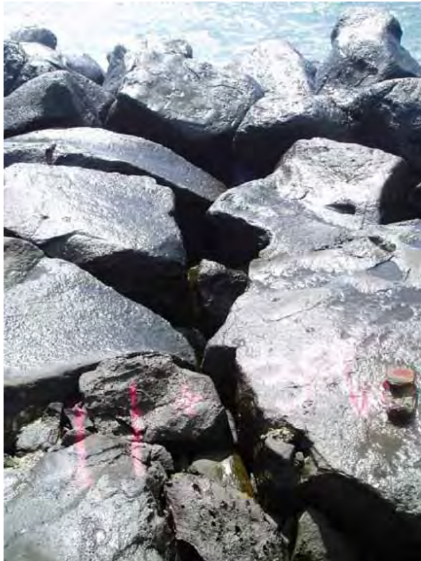
Figure D23. Damage location 25, sta 11+39, ocean side, depression/settling of crest, 5 ft x 4 ft void on crest.
