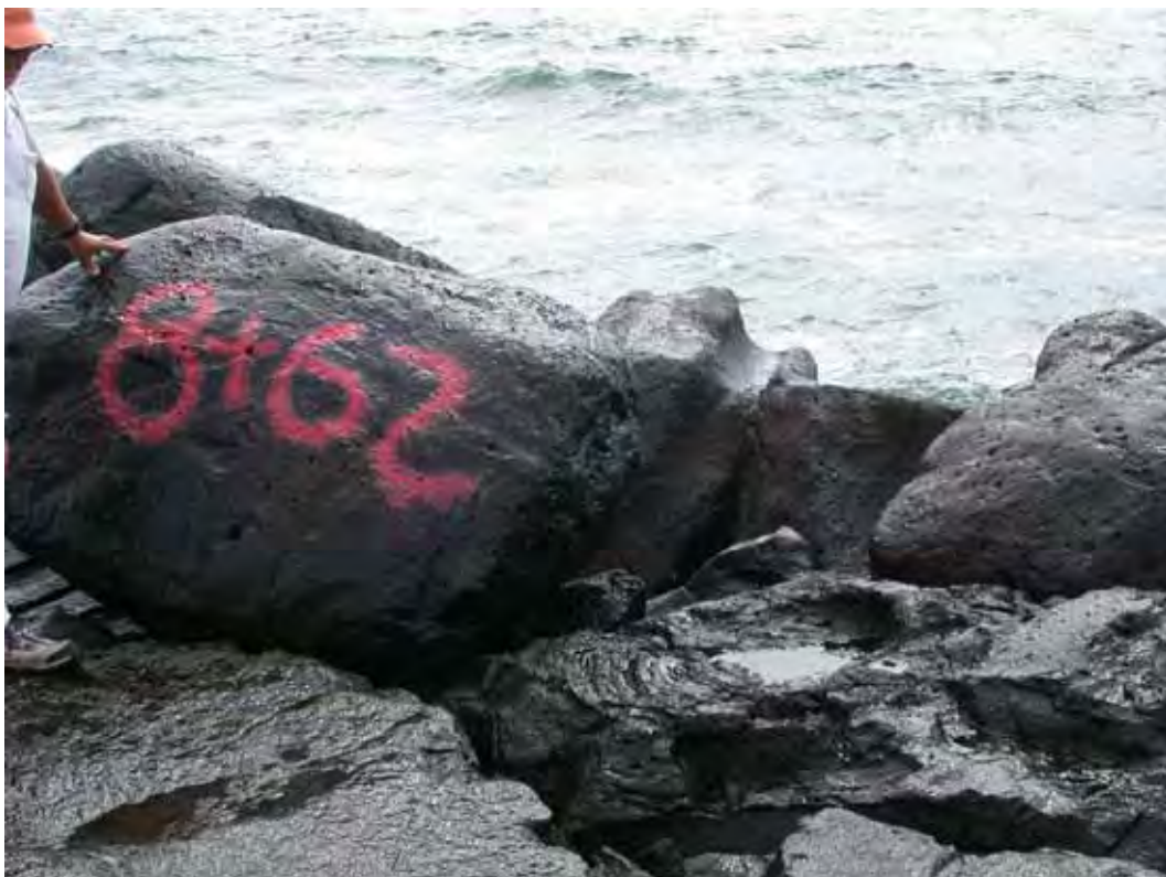
Figure D12. Damage location 11, sta 8+62, ocean side, perched armor stone with void.
