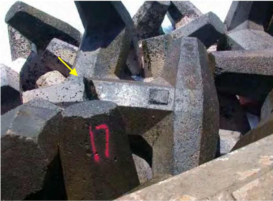
Figure D40. Damage location 49, sta 14+88, ocean side, rib #49, dolosse with fluke-shank break.
