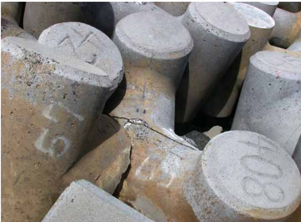
Figure D31. Damage location 34, sta 12+90, harbor side, rib #16, tribar with leg broken at center.
