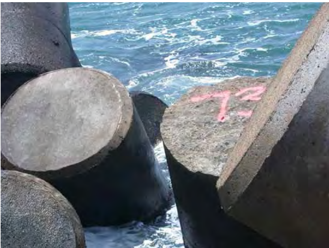
Figure B82. Damage location 51, sta 22+98, harbor side, tribar with broken can.
