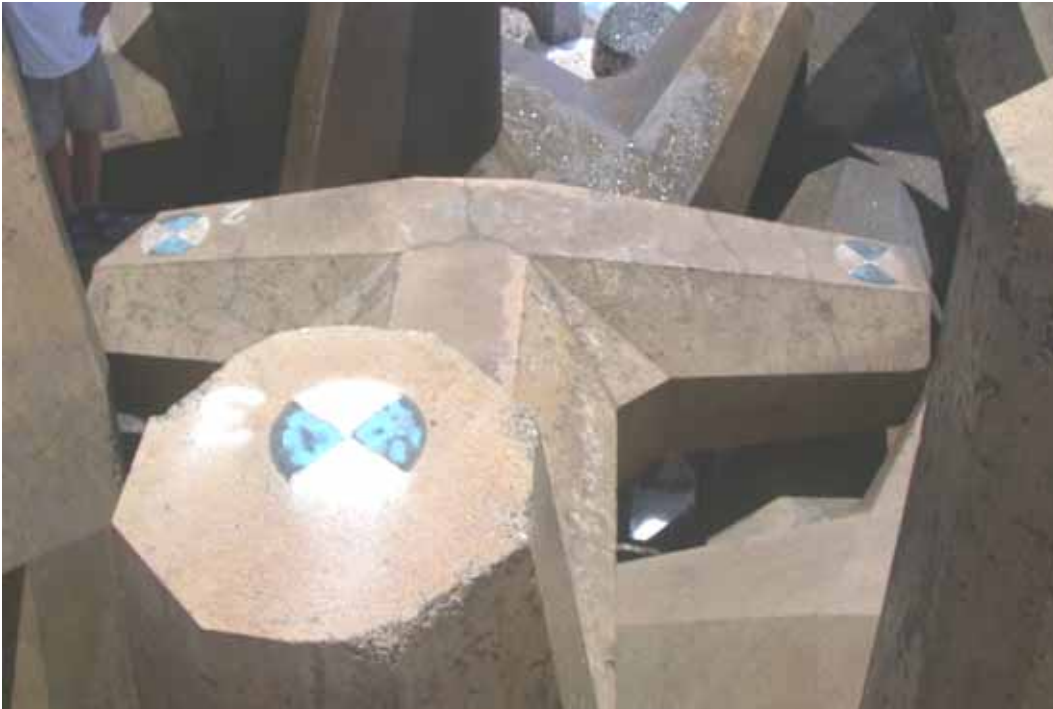
Figure 22. Example of a targeted 11-ton dolosse.
