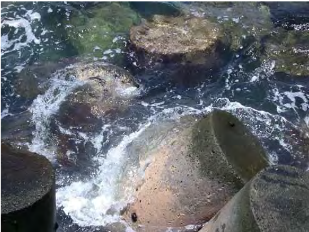
Figure A14. Damage location 16, sta 17+40, ocean side, broken tri-bar at waterline.
