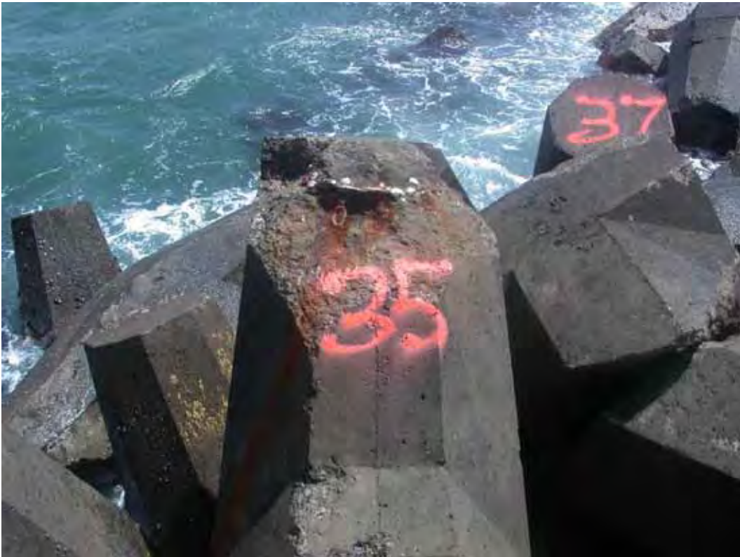
Figure B77. Damage location 46, sta 22+88, ocean side, dolosse with fluke tip break.
