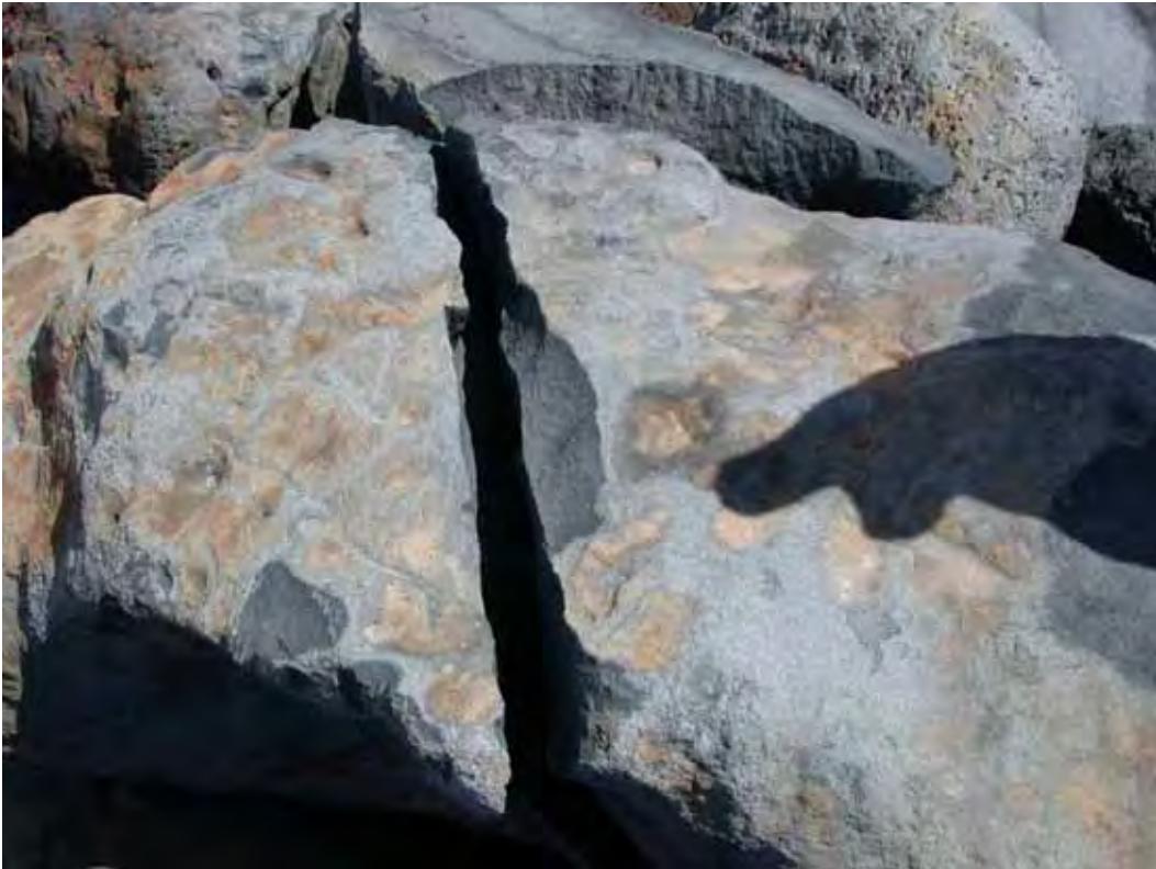
Figure B1. Damage location 1, sta 3+08, harbor side, broken armor stone.
