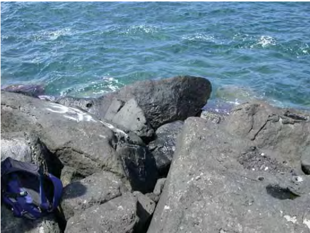
Figure A35. Damage location 37, sta 33+00, ocean side, void with dislodged hinge stone.
