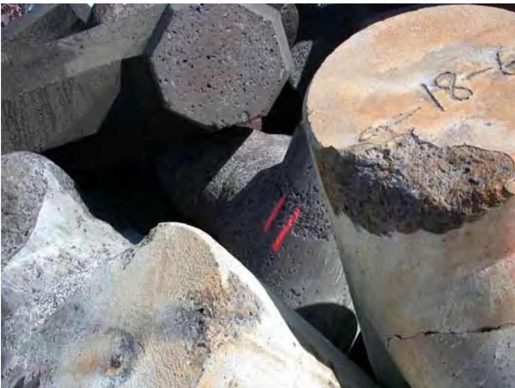
Figure B56. Damage location 18, sta 21+54, ocean side, rib #48, tribar with can missing.
