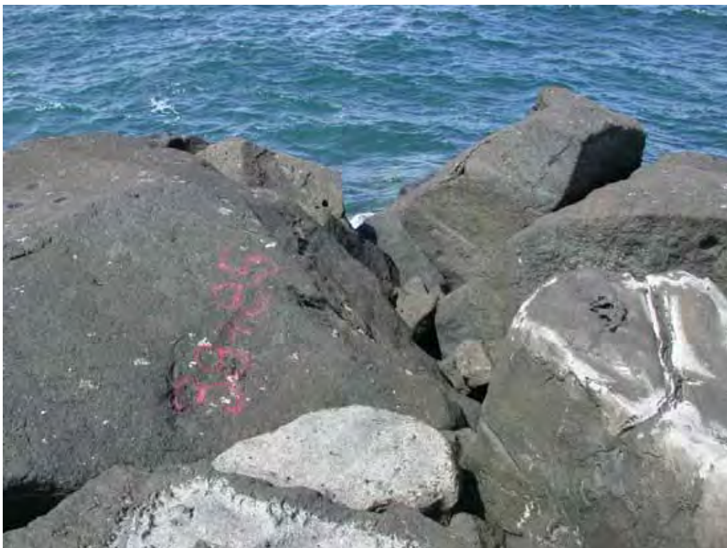
Figure A42. Damage location 44, sta 38+85, two perched armor stones.
