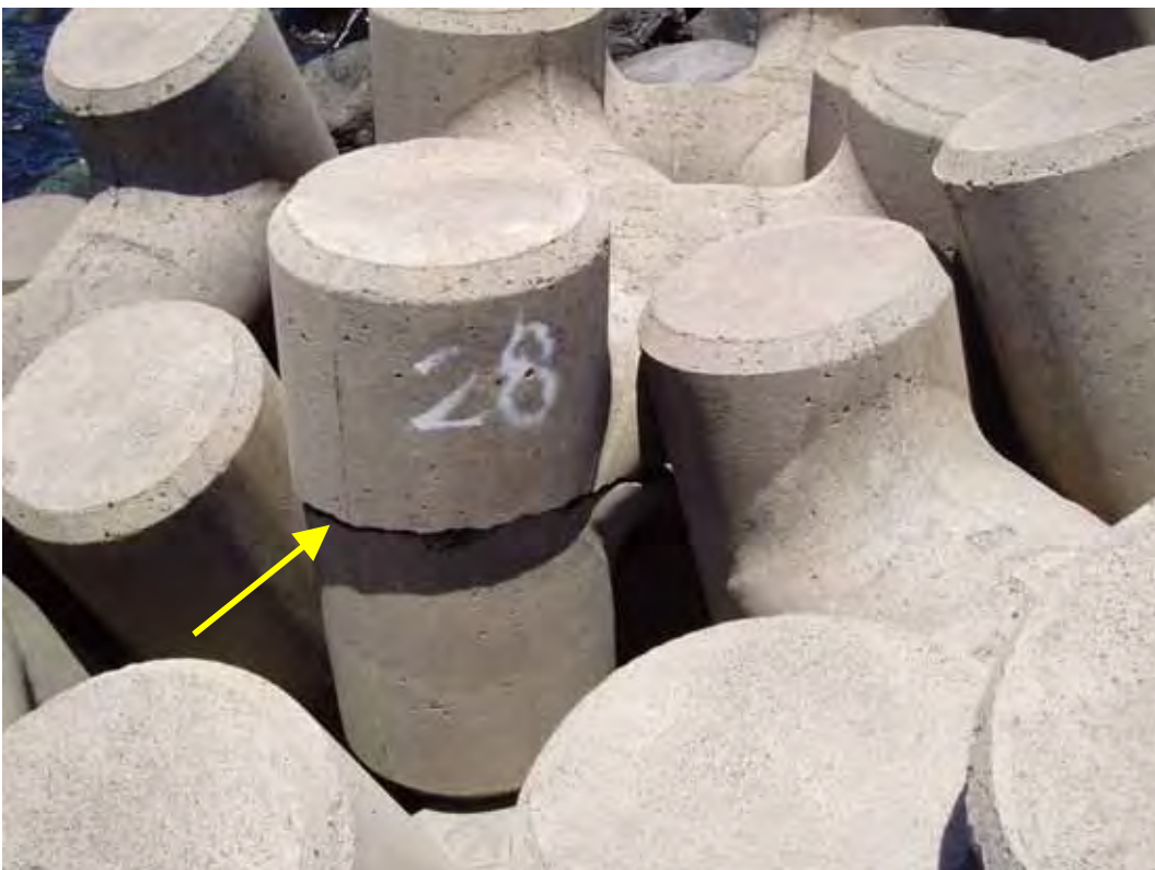
Figure B45. Damage location 2, sta 18+08, harbor side, rib #6, tribar with broken can.
