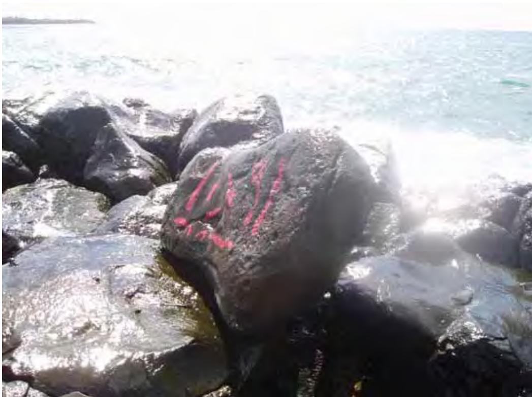
Figure D22. Damage location 24, sta 10+91, ocean side, flipped armor stone, settling, bridging, void.
