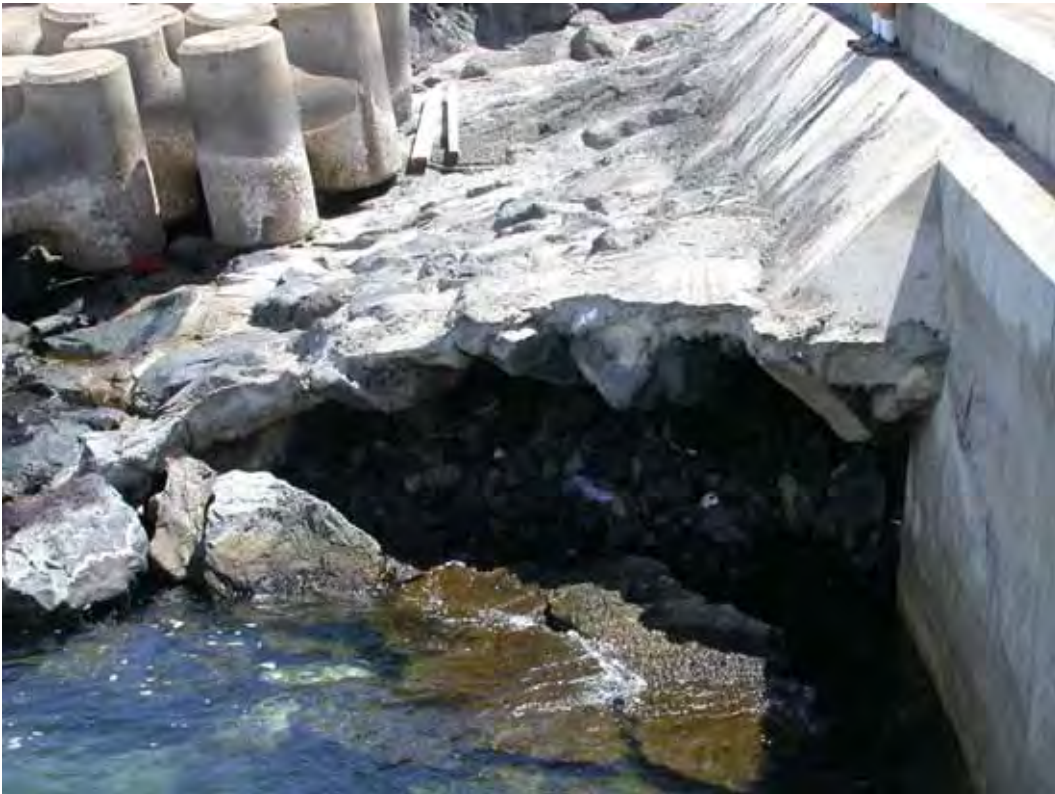
Figure B10. Damage location 13, sta 26+26, harbor side, eroded side slope.
