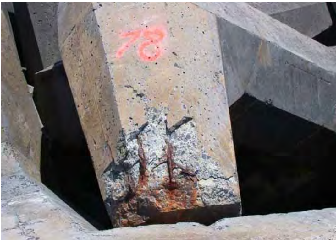
Figure B74. Damage location 40, sta 22+70, ocean side, dolosse with spalling and exposed rebar on fluke tip.
