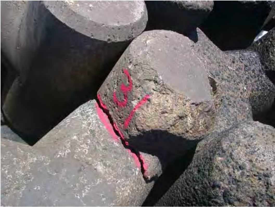
Figure 27. Typical tribar leg break.
