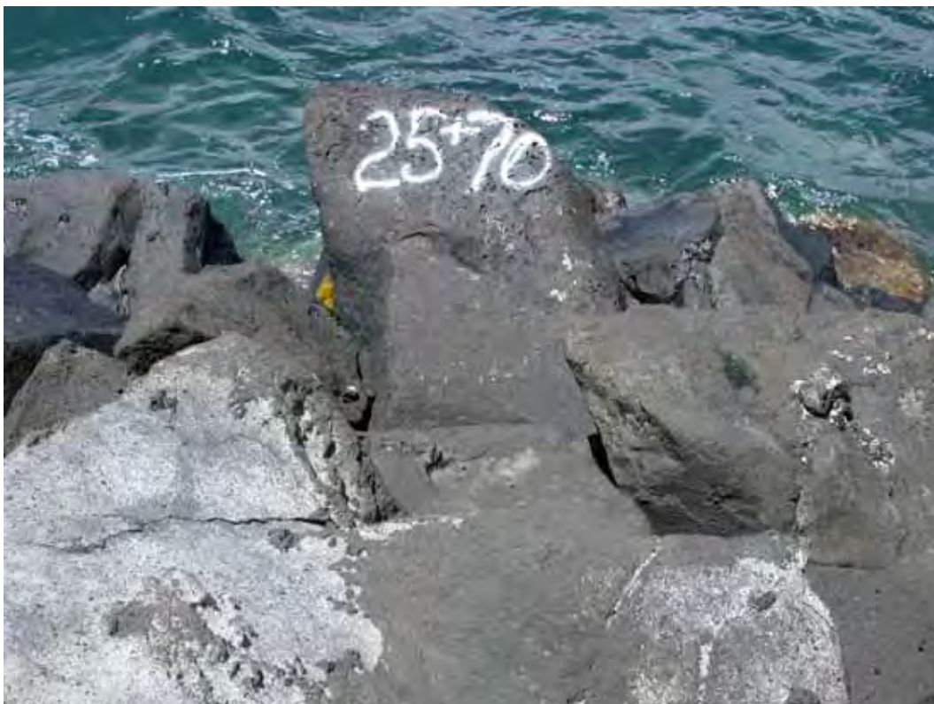
Figure A27. Damage location 26, sta 25+70, ocean side, dislodged stone.
