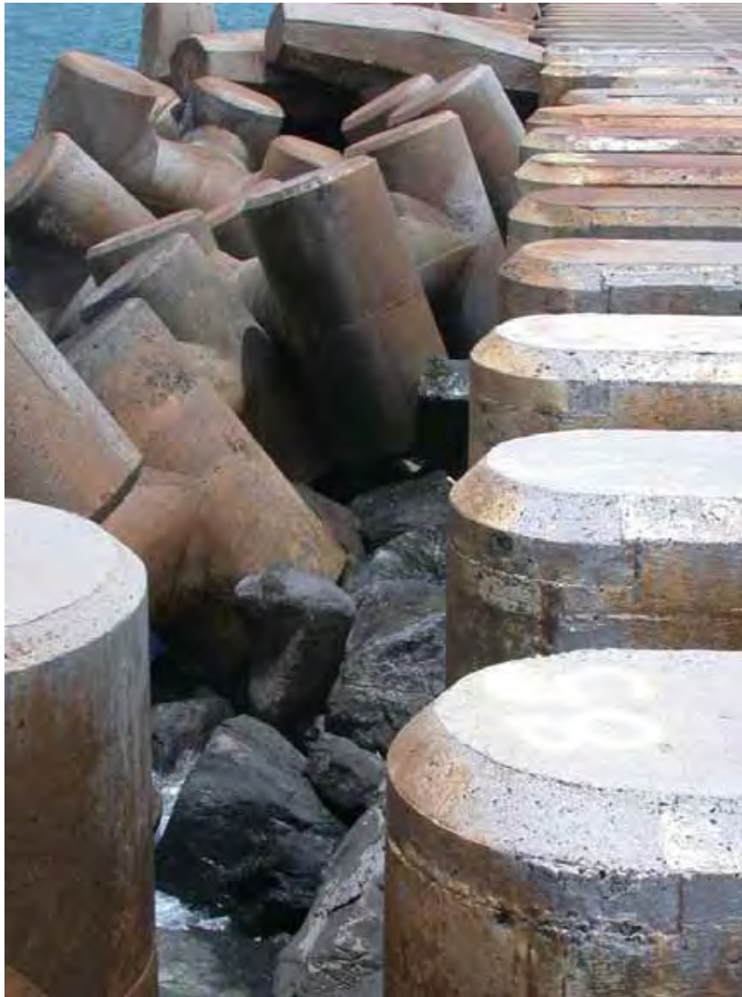
Figure B31. Damage location 40, sta 31+54 - 32+04, ocean side, rib #88 - 97, 8 ft separation of tribar from ribcap.
