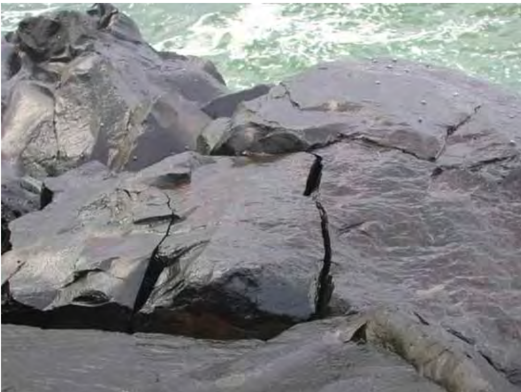
Figure A69. Damage location 82, sta 92+20, ocean side, broken armor stone and bridging.
