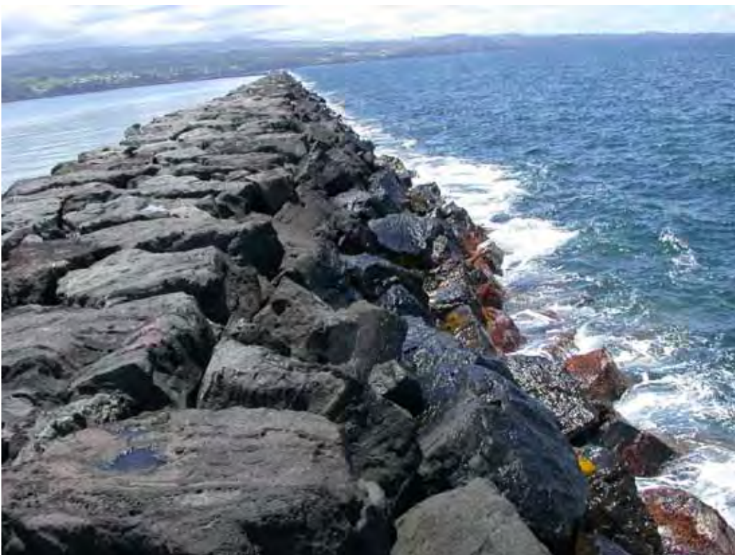
Figure A24. Damage location 23, sta 23+90-24+15, ocean side, void and settling.
