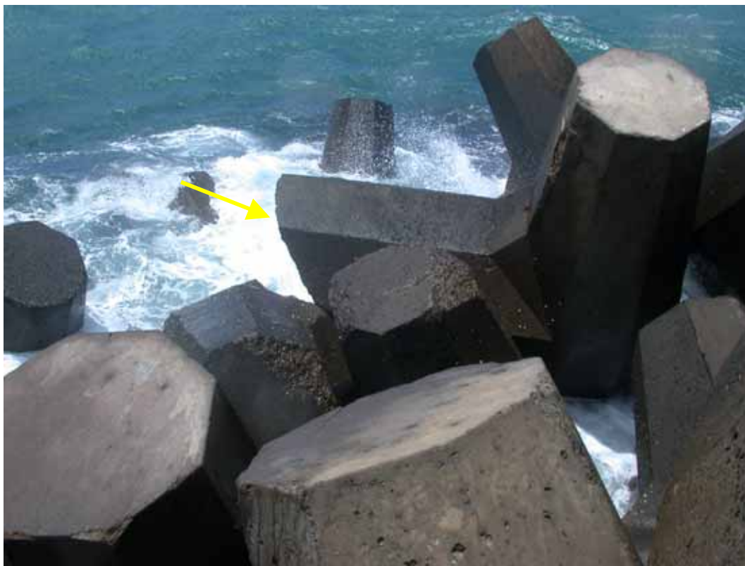
Figure B42. Damage location 57, head, 0 deg, dolosse with fluke break.
