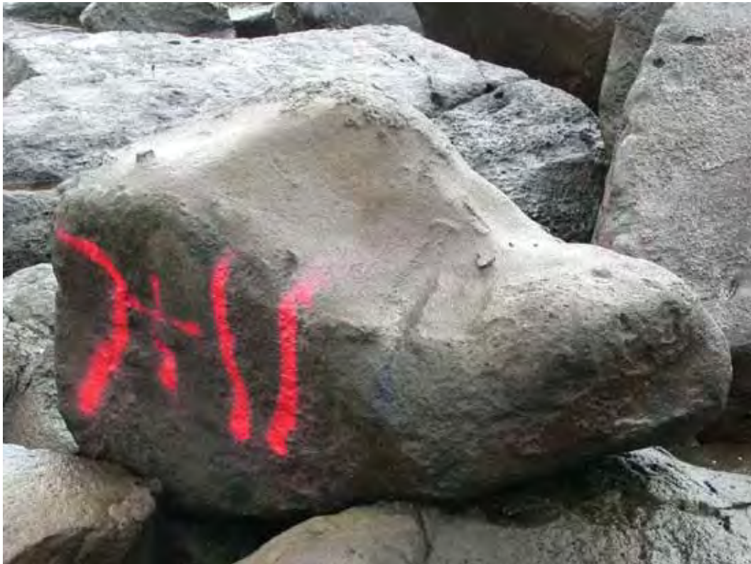
Figure D9. Damage location 8, sta 7+11, perched armor stone on crest.
