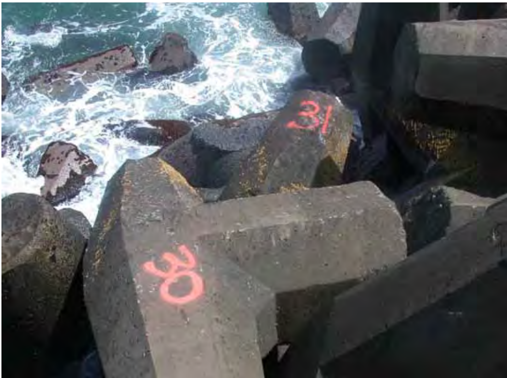
Figure B76. Damage locations 42 & 43, sta 22+74, ocean side, two dolosse with shank-fluke breaks.
