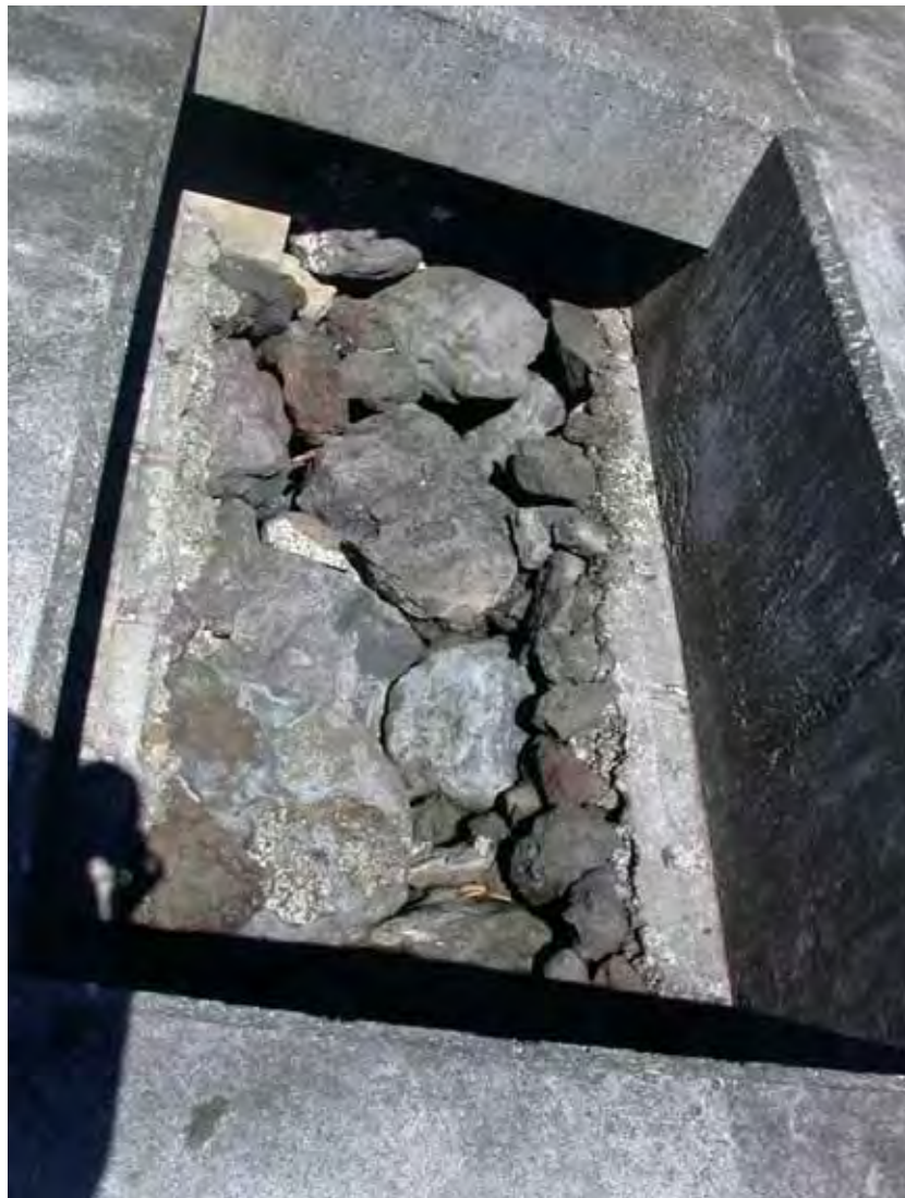
Figure C8. Shifting of stones between ribs.
