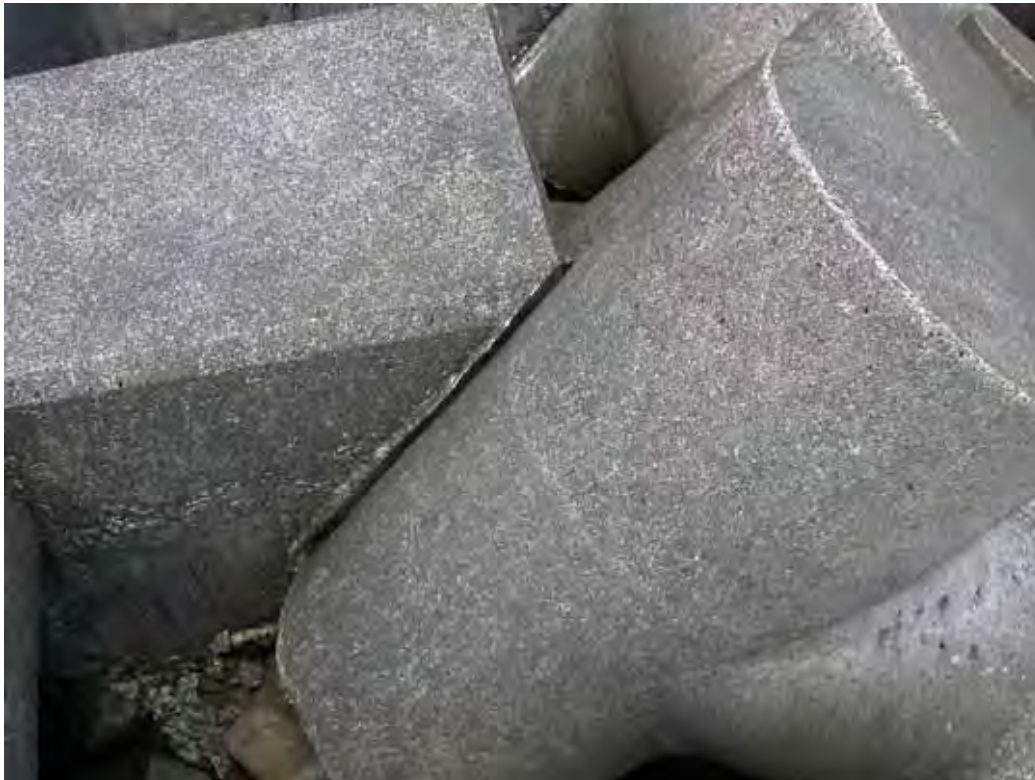
Figure A9. Damage location 8, sta 11+18, tribars separating from rib cap, side slope steepening.
