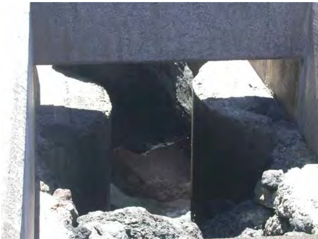
Figure C16. Underlayer loss and shifting of stones between ribs.
