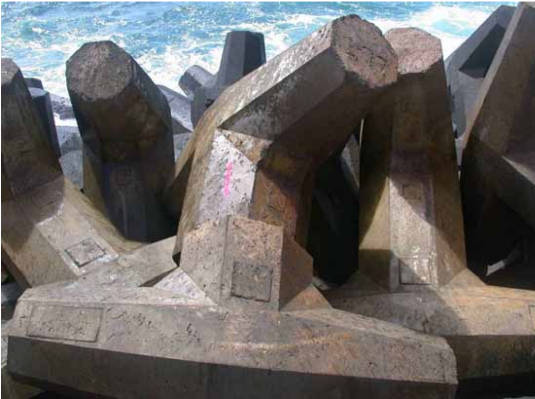
Figure D26. Damage location 27, sta 12+24, ocean side, rib #5, dolosse with mid-shank break.
