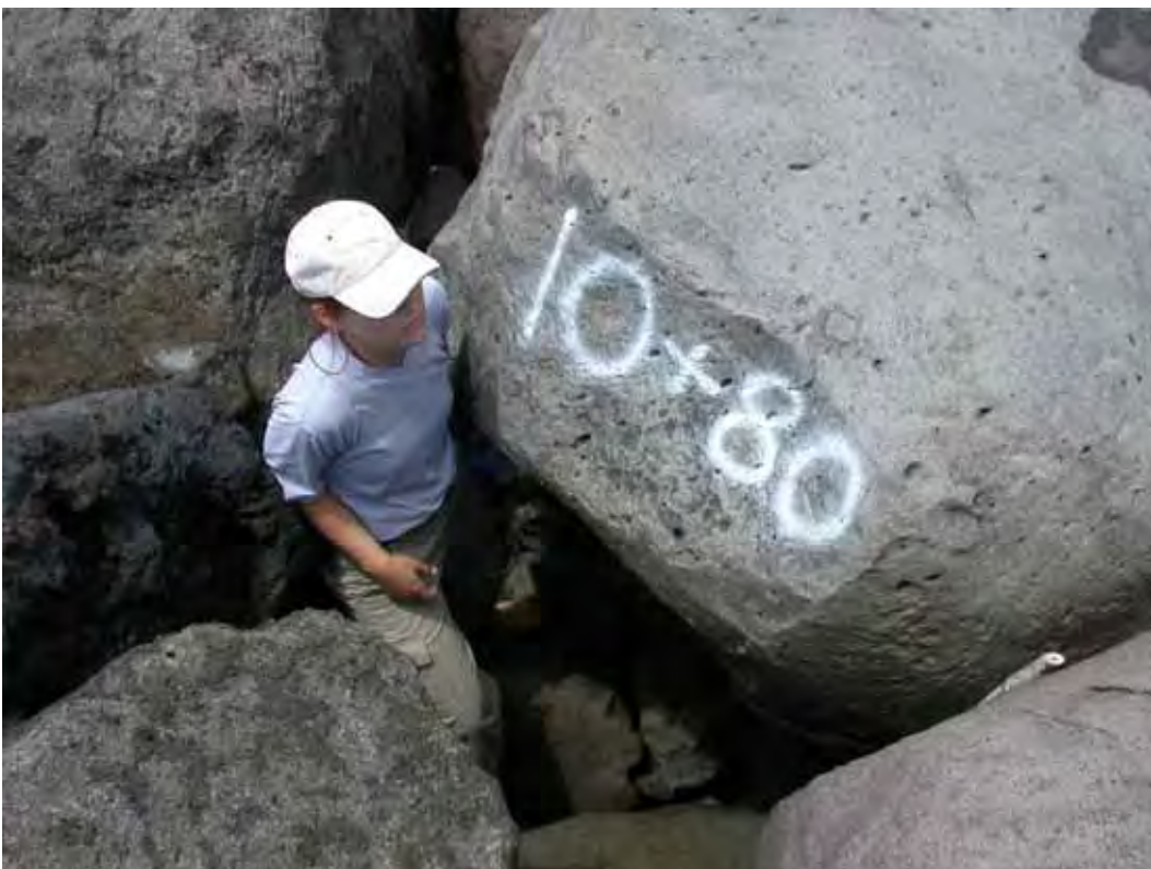
Figure A8. Damage location 7, sta 10+80, harbor side, void approximately 5 ft deep.
