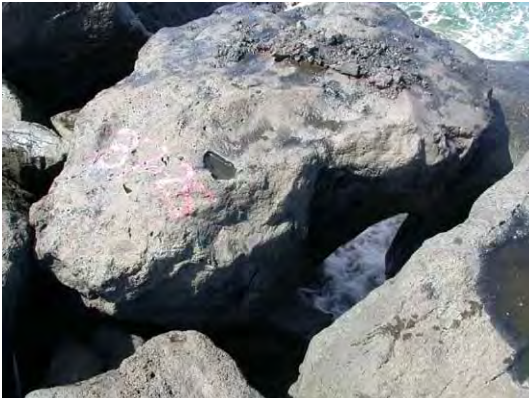
Figure A41. Damage location 43, sta 37+25, ocean side, bridging at crest.
