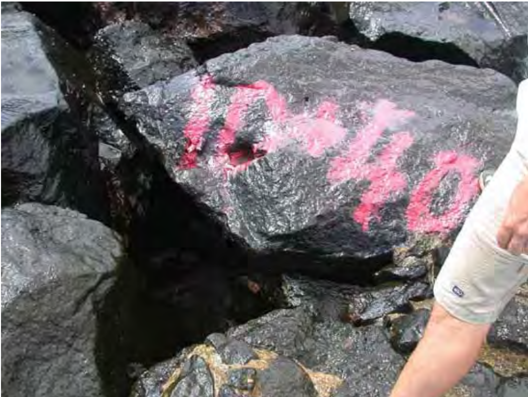
Figure D21. Damage location 20, sta 10+40, void (depth to waterline) at centerline of crest.
