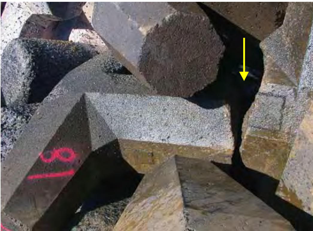
Figure D41. Damage location 50, sta 14+94, ocean side, rib #50, dolosse with shank-fluke break.
