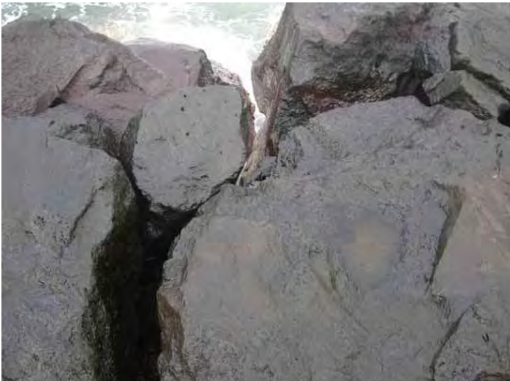
Figure A73. Damage location 87, sta 98+50, ocean side, 2-ft-wide fissure extending from crest down to waterline.
