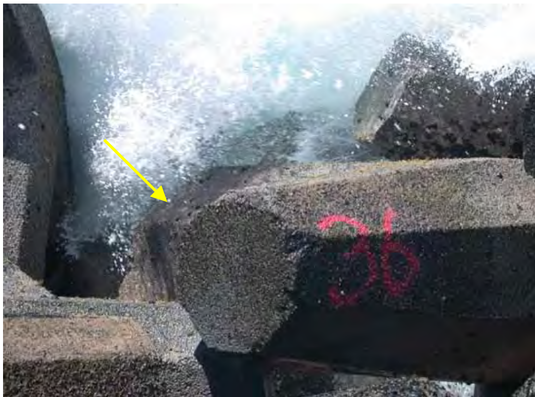
Figure D52. Damage location 68, sta 16+80, ocean side, rib #81, dolosse with shank-fluke break.
