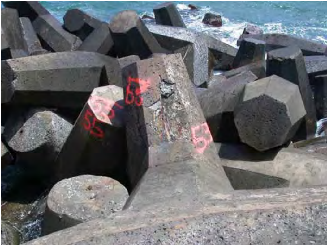
Figure B91. Damage location 67, 45 deg ocean side of head, dolosse with spalling.
