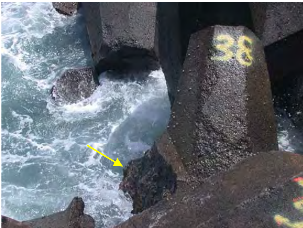
Figure B84. Damage location 53, sta 23+00, ocean side, dolosse with shank-fluke break.
