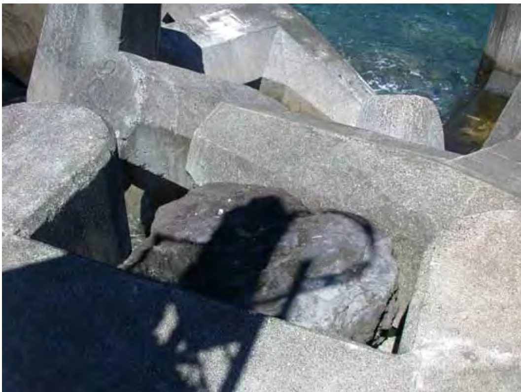
Figure C12. Displaced armor stone, tossed onto dolosse.
