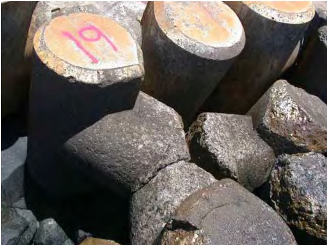
Figure D42. Damage location 51, sta 15+00, ocean side, rib #51, tribar with 3-way split.
