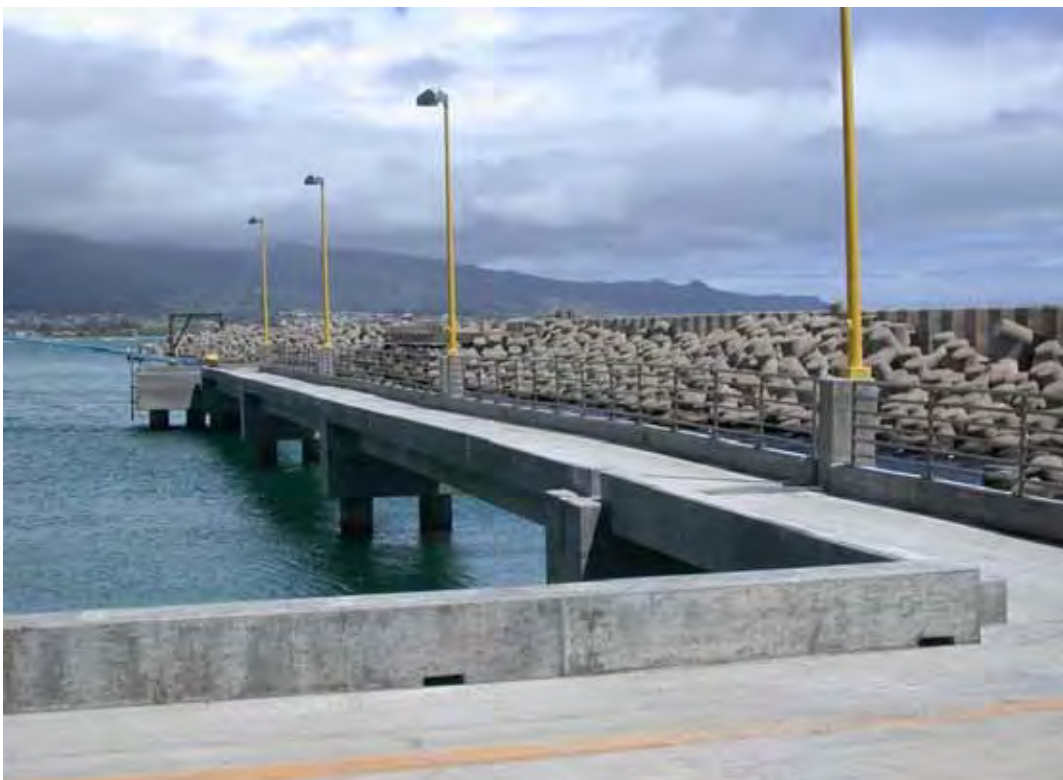
Figure B9. Sta 26+26, harbor side, New Dolphin and walkway adjacent to breakwater; built 2005.
