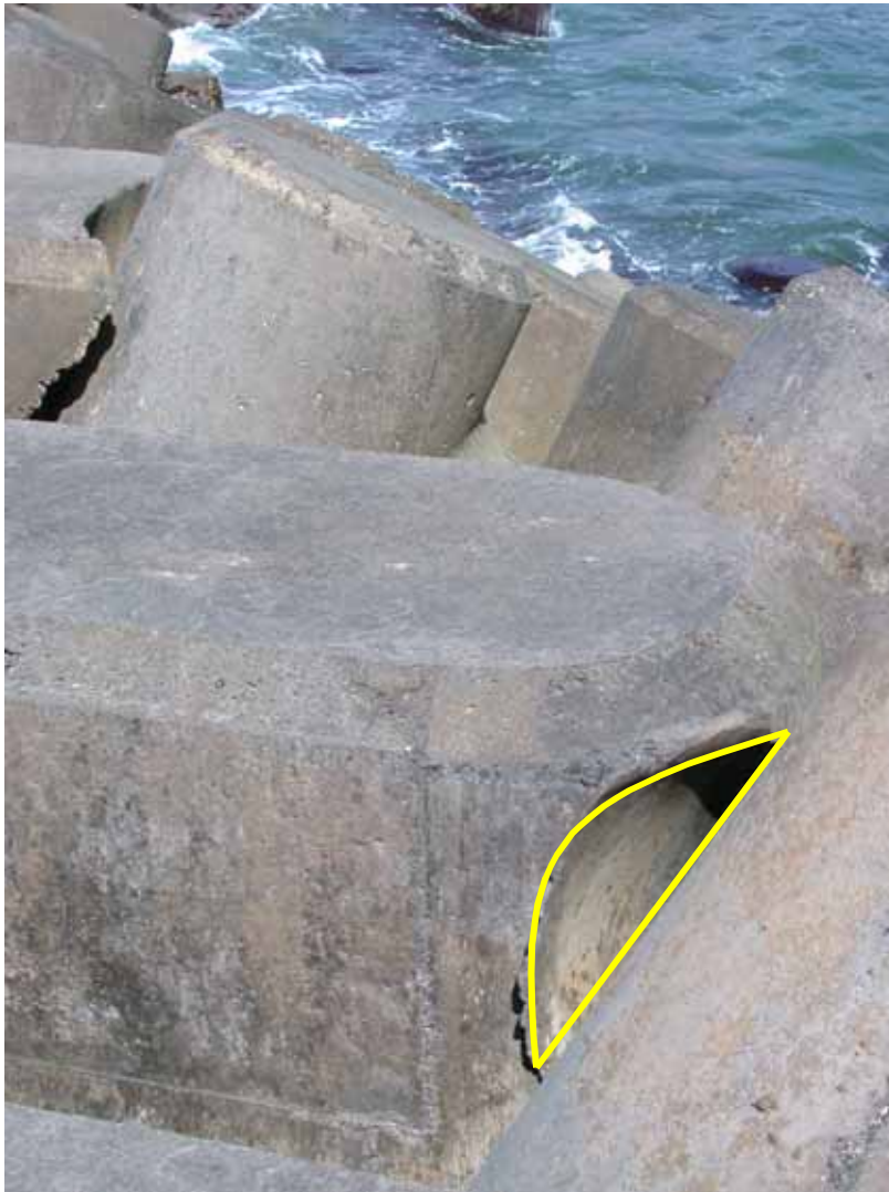
Figure B46. Damage location 3, sta 18+74, ocean side, rib #13, 8" separation of tribar from rib cap.
