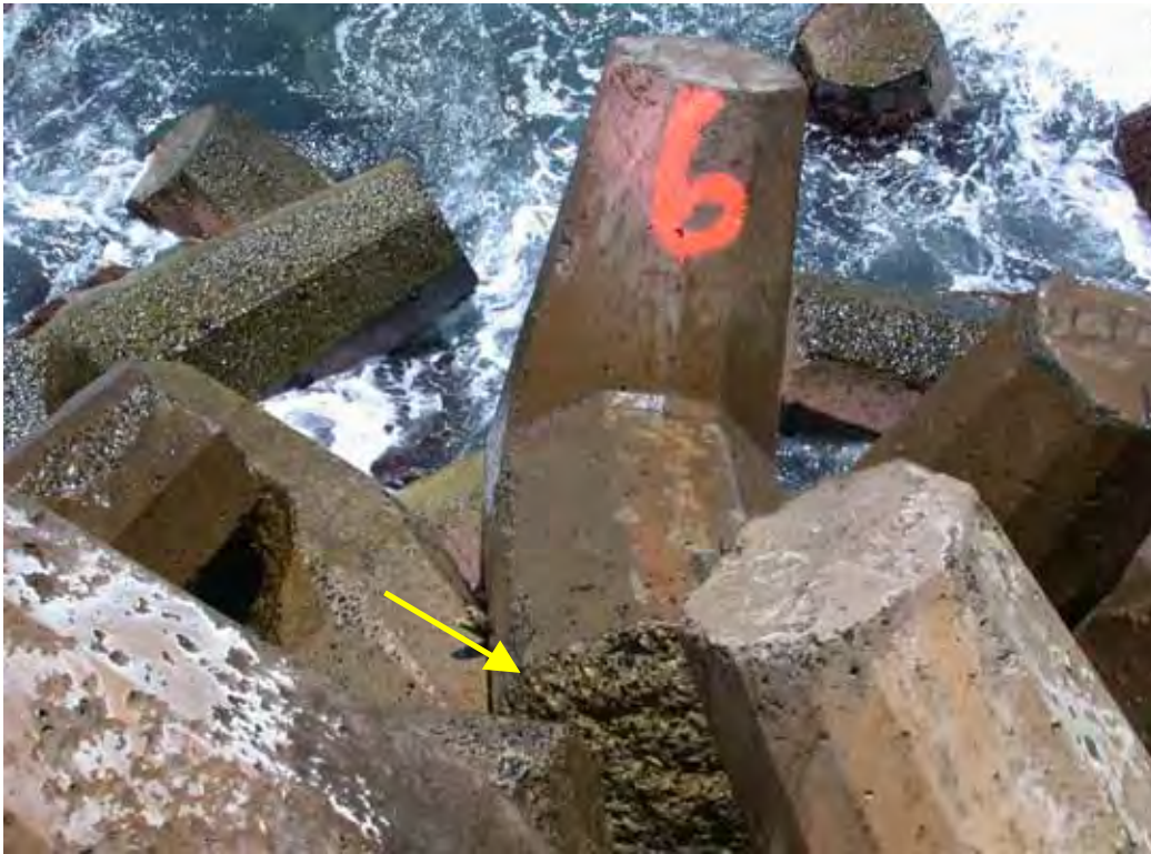
Figure B16. Damage location 19, sta 27+09, ocean side, rib #15, dolosse with shank-fluke break.
