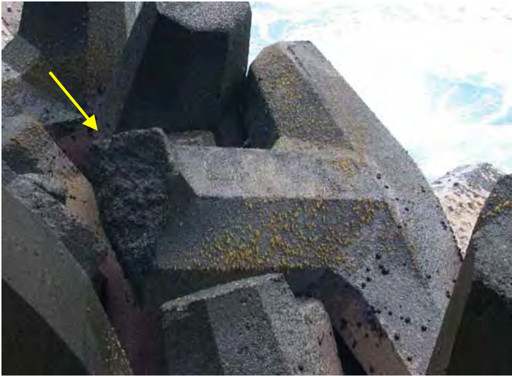
Figure D30. Damage location 33, sta 12+72, ocean side, rib #13, dolosse with shank-fluke break at waterline, ocean side of target NA.
