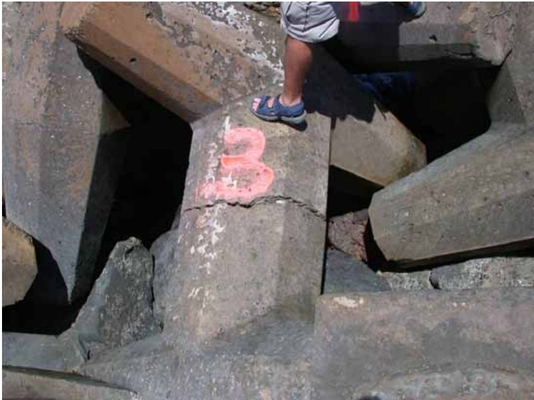
Figure 23. Typical dolosse mid-shank crack/break.
