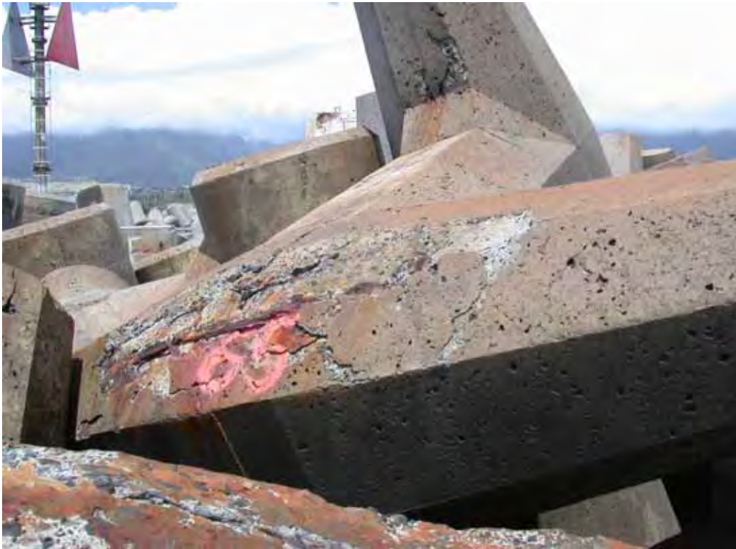
Figure B97. Damage location 79, 6 deg harbor side of head, dolosse with spalling and exposed rebar on fluke.
