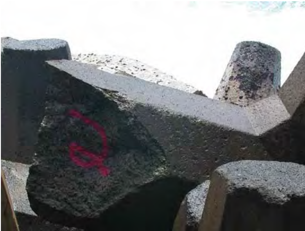
Figure D28. Damage location 29, sta 12+36, ocean side, rib #7, dolosse with mid-shank and shank-fluke breaks.
