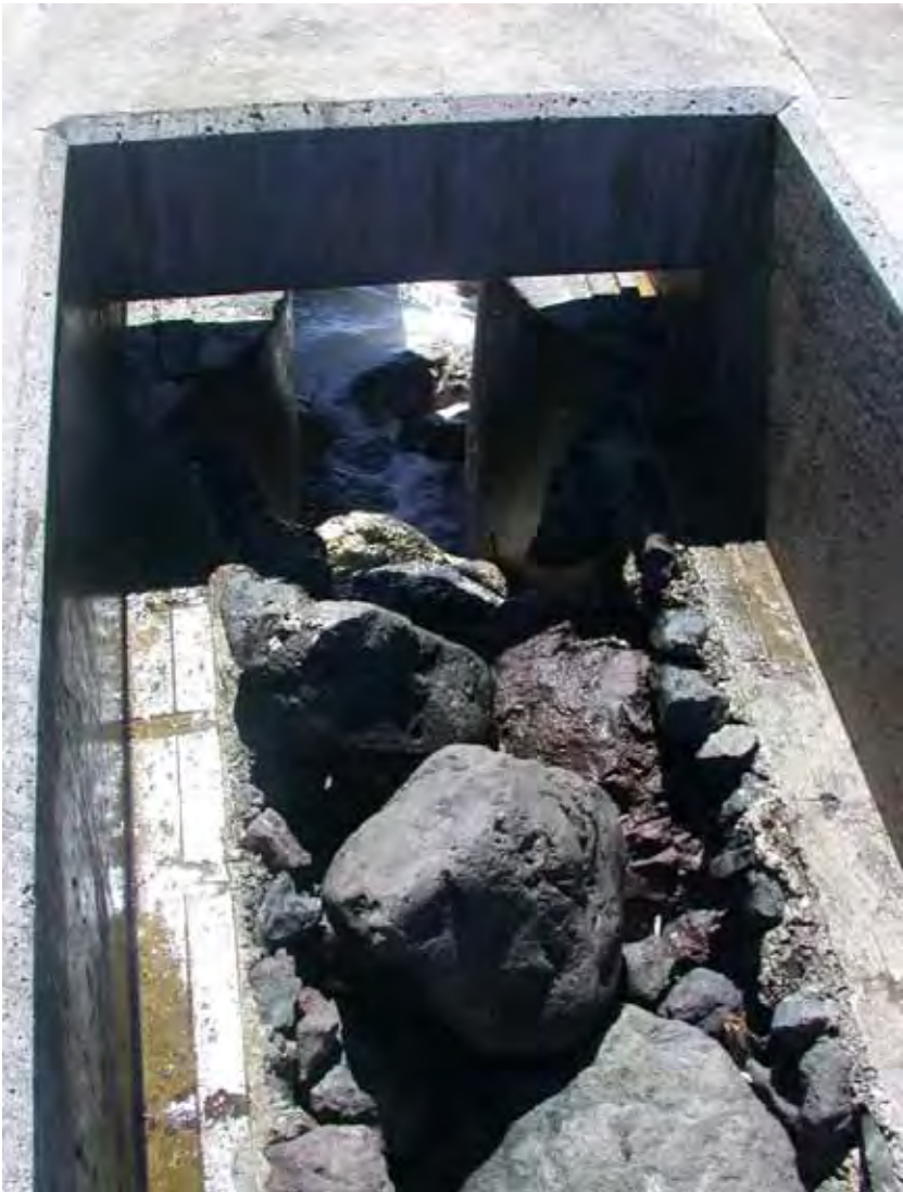
Figure C10. Underlayer loss and shifting of stones between ribs.
