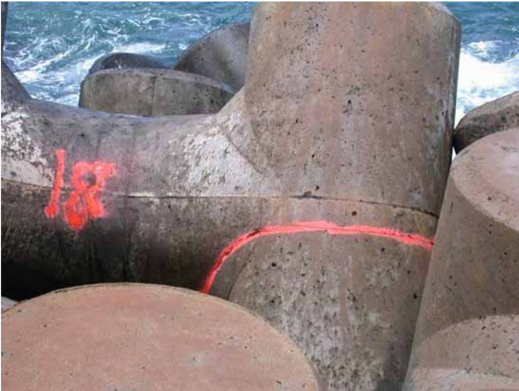
Figure B29. Damage location 38, sta 31+54, ocean side, rib #88, tribar with leg crack.
