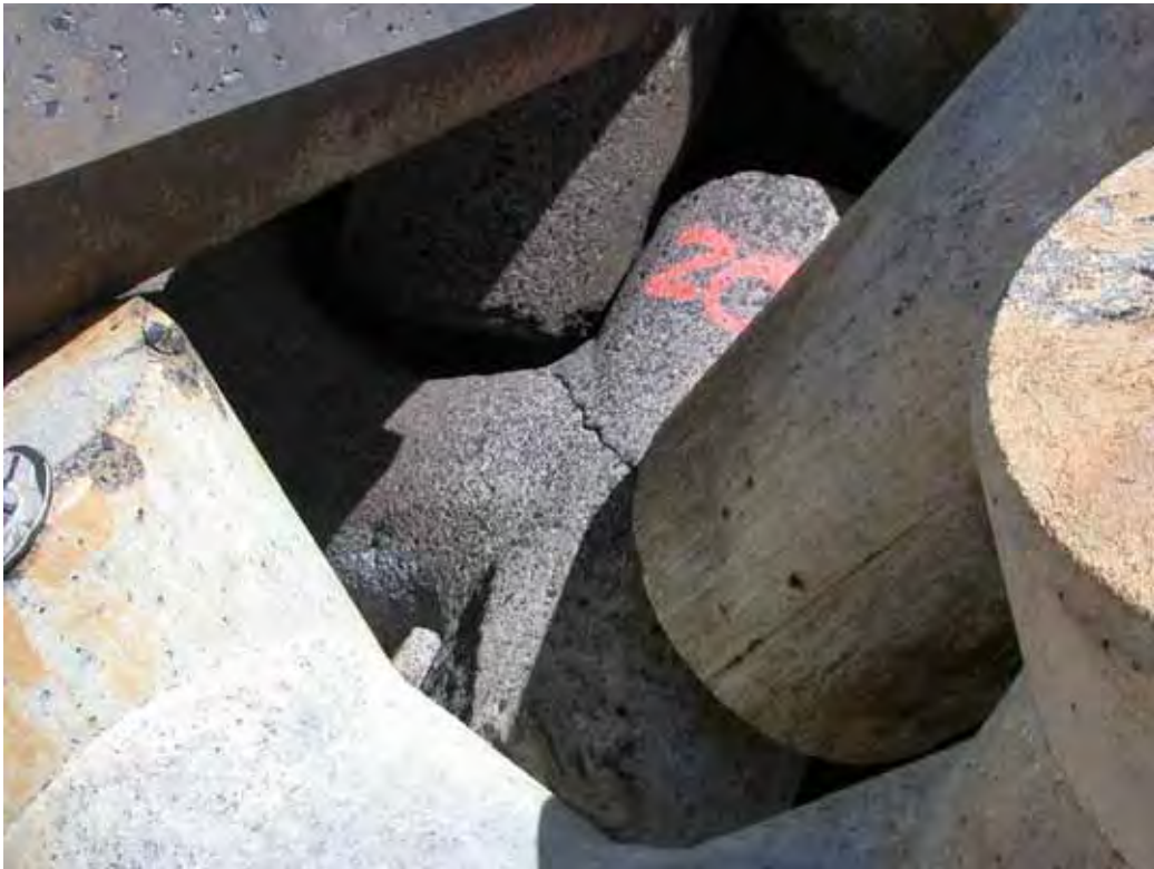
Figure B63. Damage location 26, sta 22+10, ocean side, tribar with crack held together by rebar.
