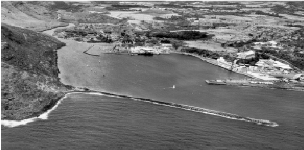
Figure 17. Aerial photograph of Nawiliwili Harbor.
