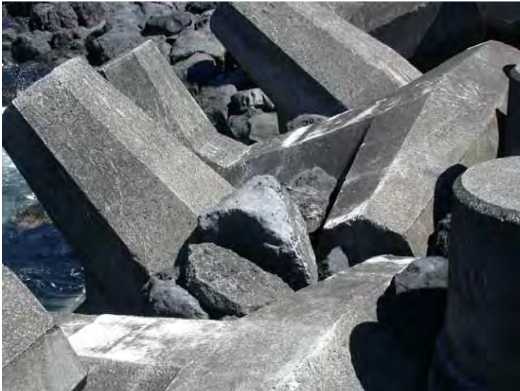
Figure C11. Displaced armor stone, tossed onto dolosse.
