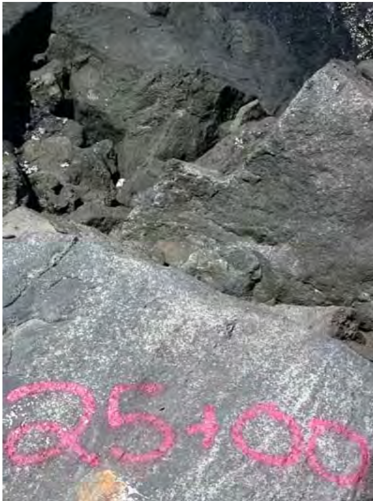
Figure A25. Damage location 24, sta 25+00, hinge stone breaking apart.
