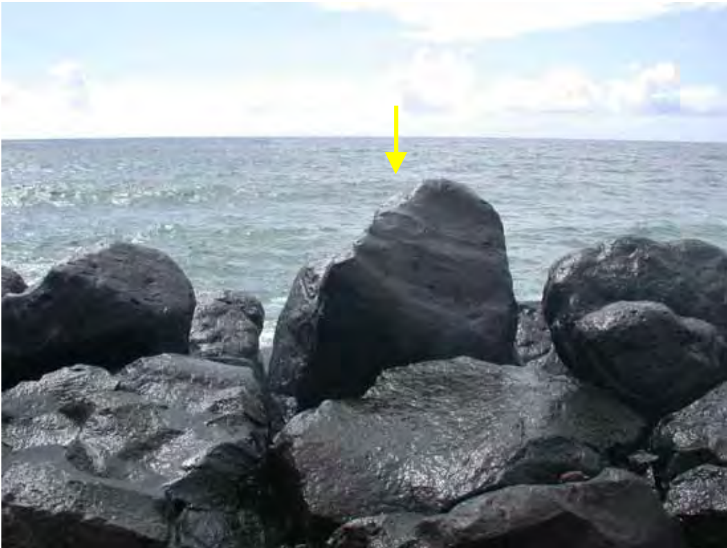
Figure D15. Damage location 14, sta 9+20, ocean side, flipped armor stone and void.
