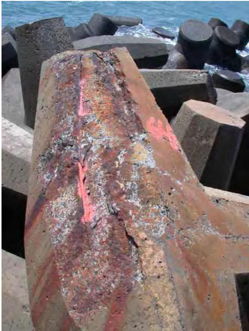
Figure B96. Damage location 78, 5 deg harbor side of head, dolosse with spalling, exposed rebar, and fracturing on fluke tip.
