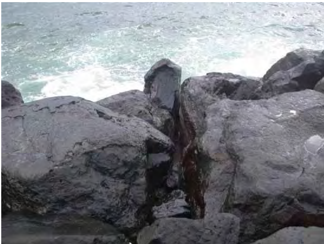
Figure A71. Damage location 85, sta 95+50, ocean side, separation of slope, flipped stone.
