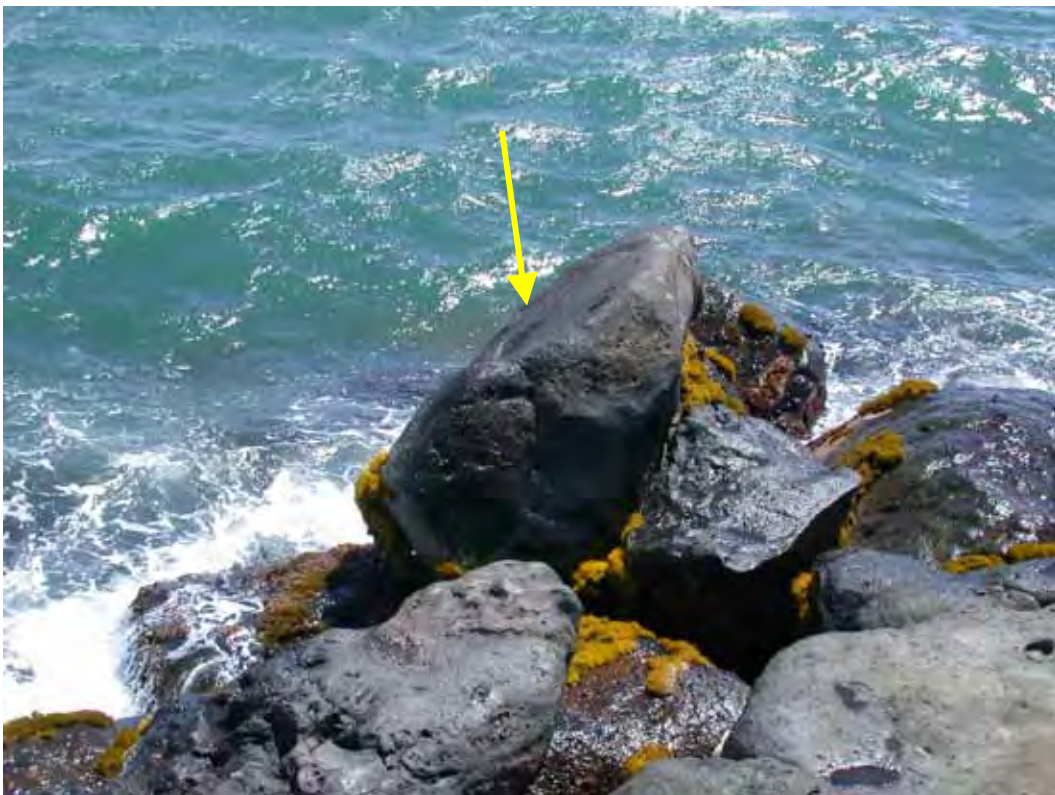
Figure B7. Damage location 12, sta 24+50, ocean side, flipped armor stone.
