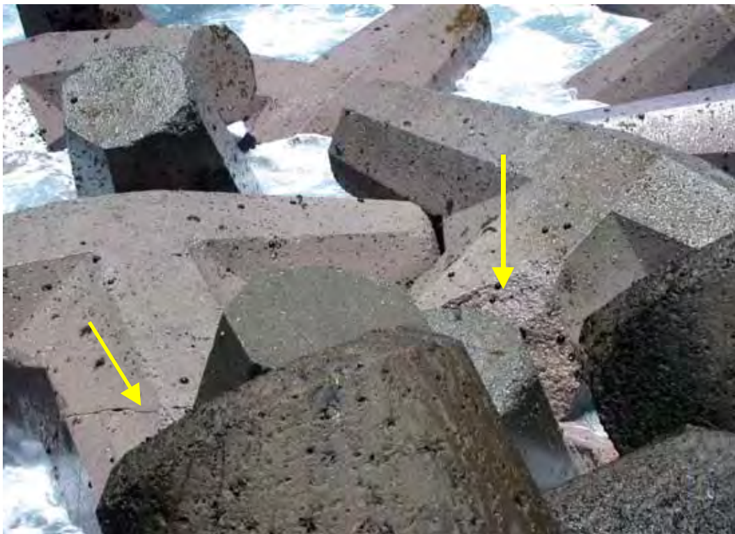
Figure D79. Damage locations 109 & 110, 25 deg harbor side of head, dolosse with shank crack and dolosse with shank break.
