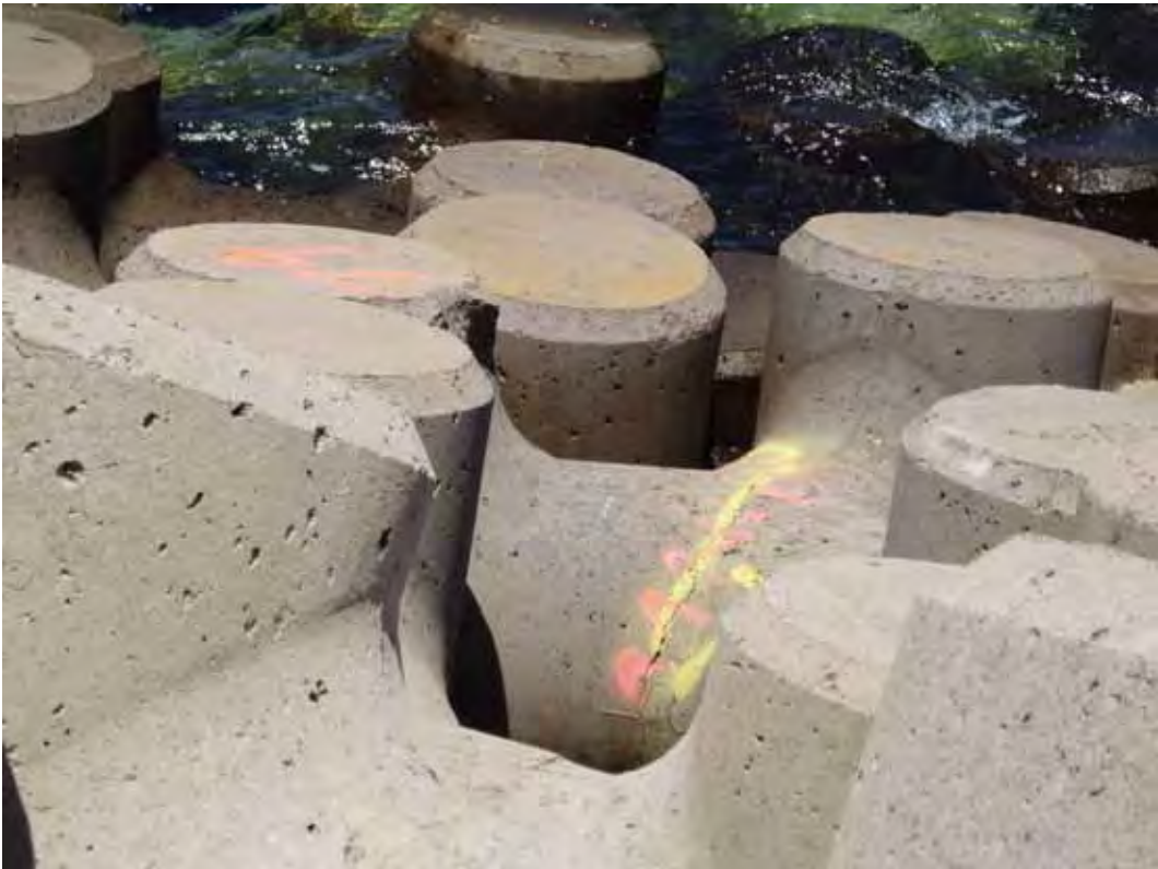
Figure B52. Damage location 10, sta 20+74, ocean side, rib #38, tribar with broken leg.
