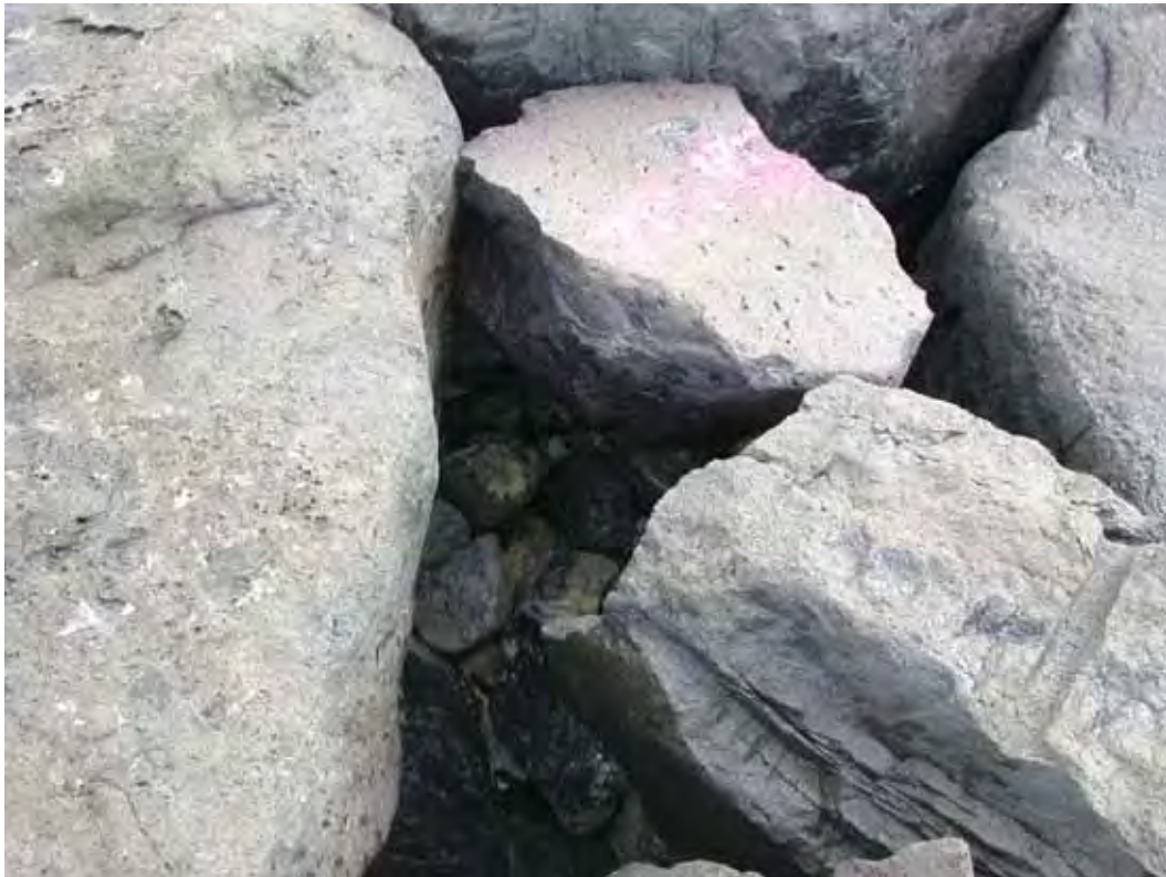
Figure A64. Damage location 75, sta 75+95, void.
