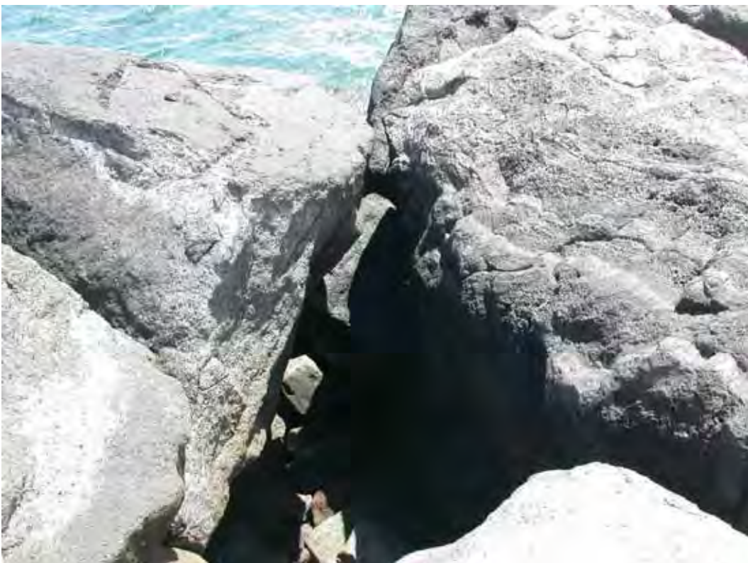
Figure A4. Damage location 3, sta 8+15, ocean side, 4-ft-wide void, 6.5 ft deep, slight sinking.
