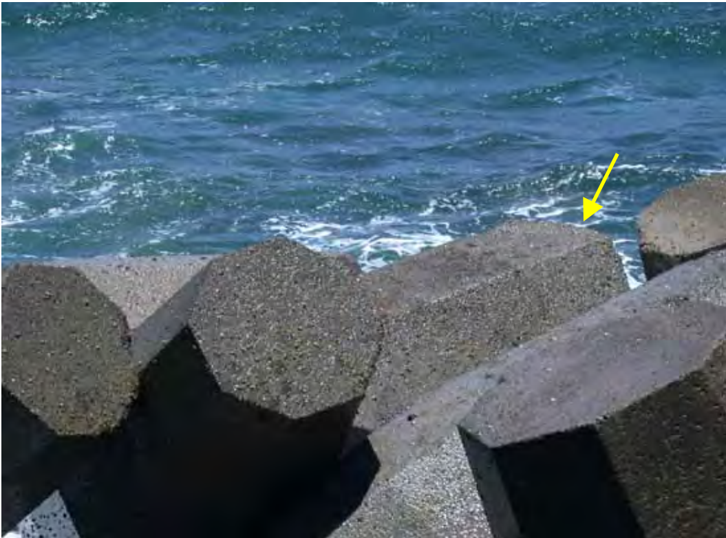
Figure D78. Damage location 108, 70 deg ocean side of head, dolosse with shank-fluke break at waterline.
