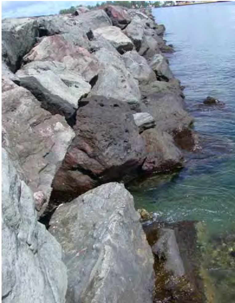
Figure 30. Example of a breakwater void.
