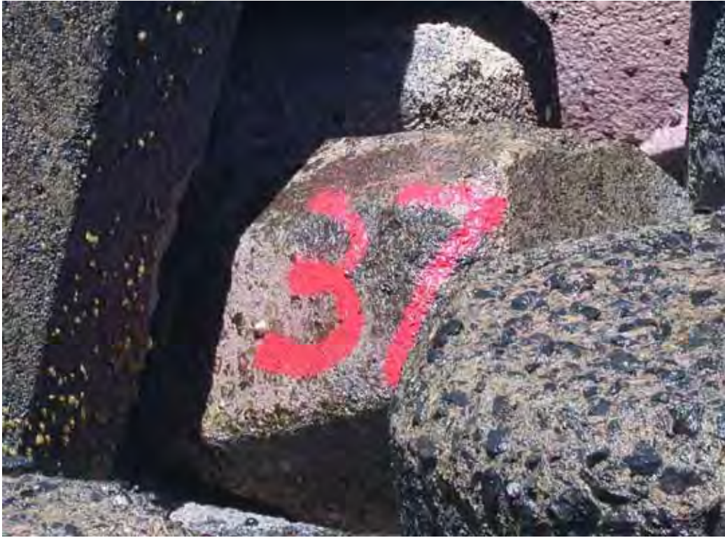
Figure D53. Damage location 69, sta 16+98, ocean side, rib #84, detached dolosse fluke tip, origin unknown.
