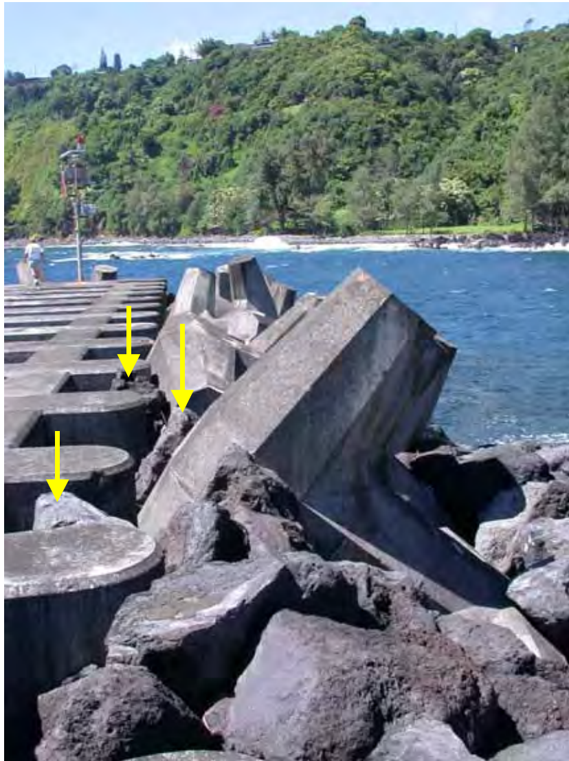
Figure C9. Displaced armor stone, tossed onto dolosse.
