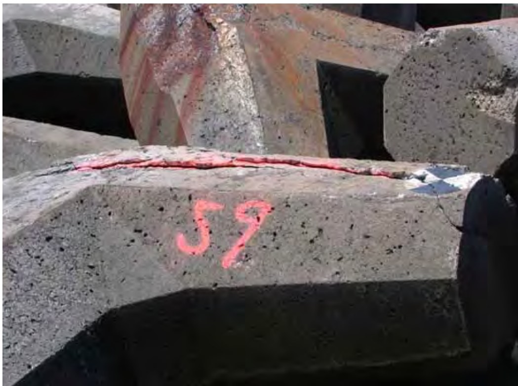
Figure B95. Damage location 75, head, 0 deg, dolosse with longitudinal fluke crack and spalling.
