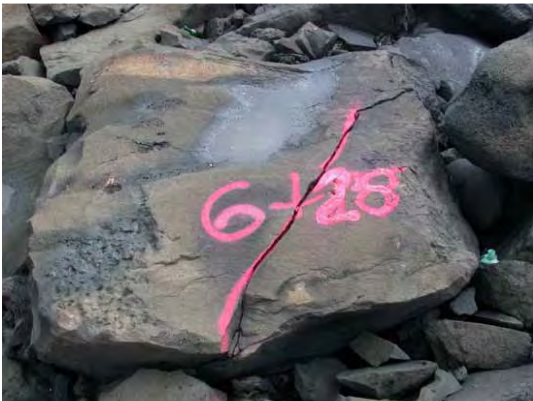
Figure D6. Damage location 5, sta 6+28, cracked armor stone on crest.
