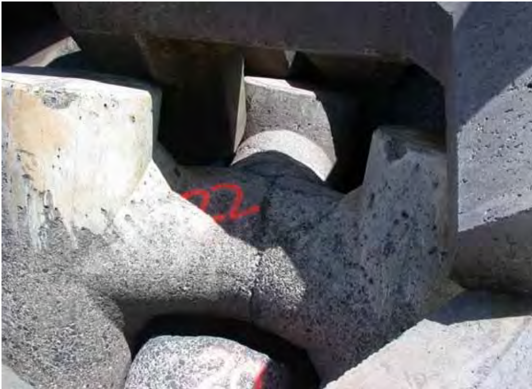
Figure B65. Damage location 28, sta 22+14, ocean side, tribar with broken can held together by rebar.
