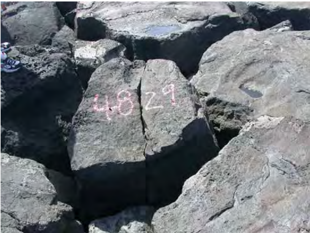
Figure A45. Damage location 48, sta 48+29, broken stone on crest.
