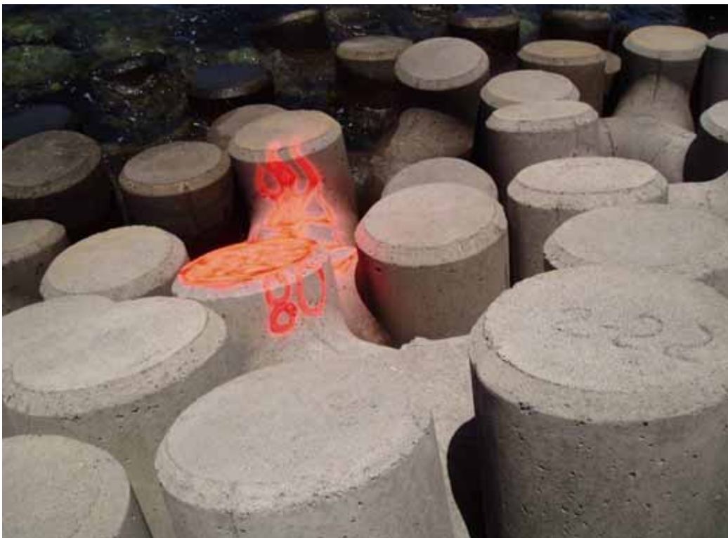
Figure B48. Damage location 5, sta 18+90, harbor side rib #15, tribar with crack through center.
