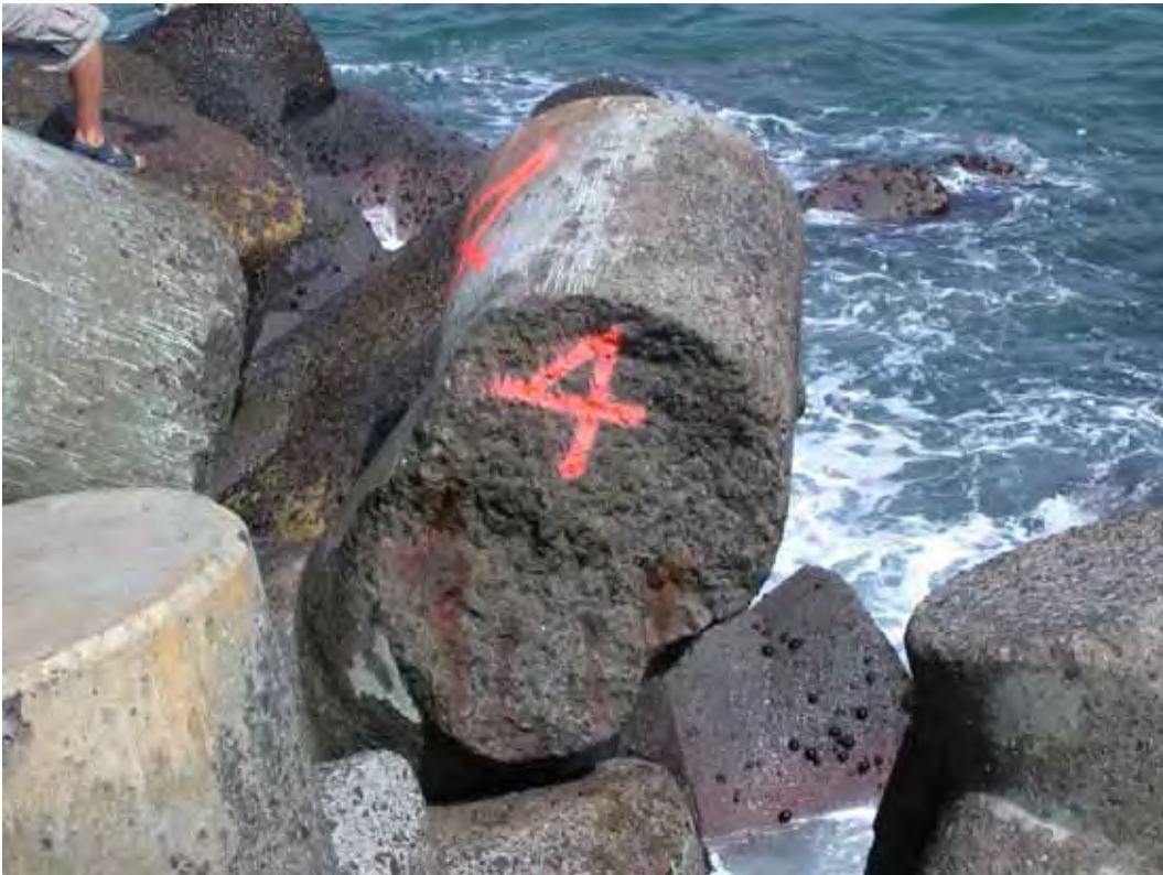
Figure B53. Damage location 13, sta 20+90, ocean side, rib #40, tribar with can missing.
