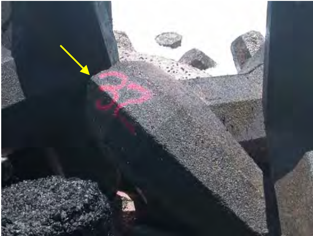
Figure D48. Damage location 64, sta 16+32, ocean side, rib #73, dolosse with fluke tip break.
