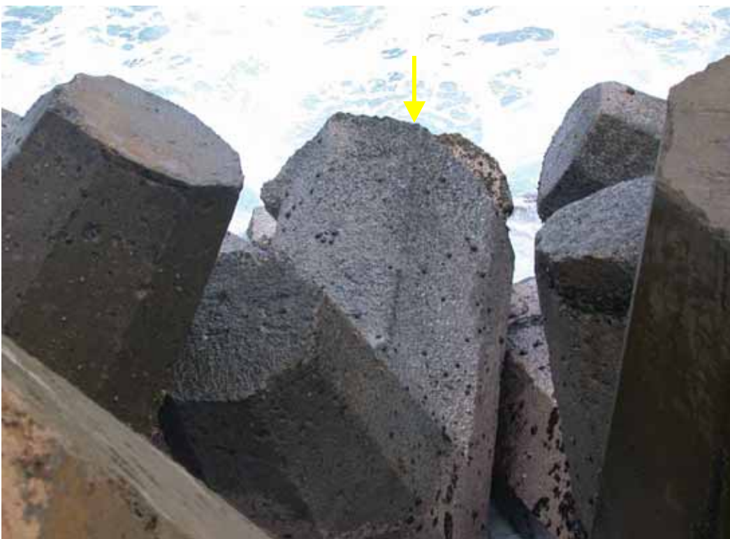
Figure D35. Damage location 40, sta 13+80, ocean side, rib #31, dolosse with shank-fluke break at waterline.
