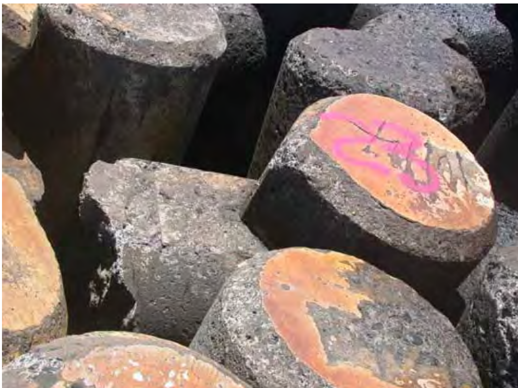
Figure D43. Damage location 55, sta 15+60, ocean side, rib #61, tribar with 3-way break at center.
