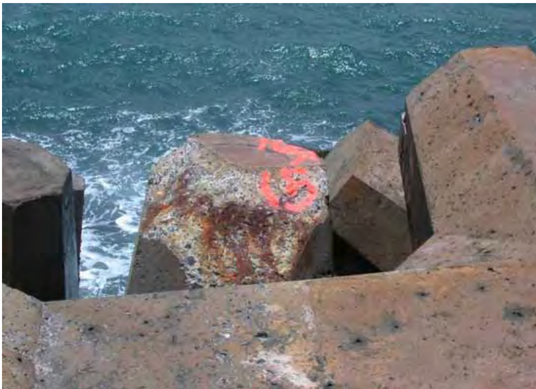
Figure B26. Damage locations 32 and 33, sta 30+04, ocean side, rib #63, two dolosse with tip chips (one visible in photograph).
