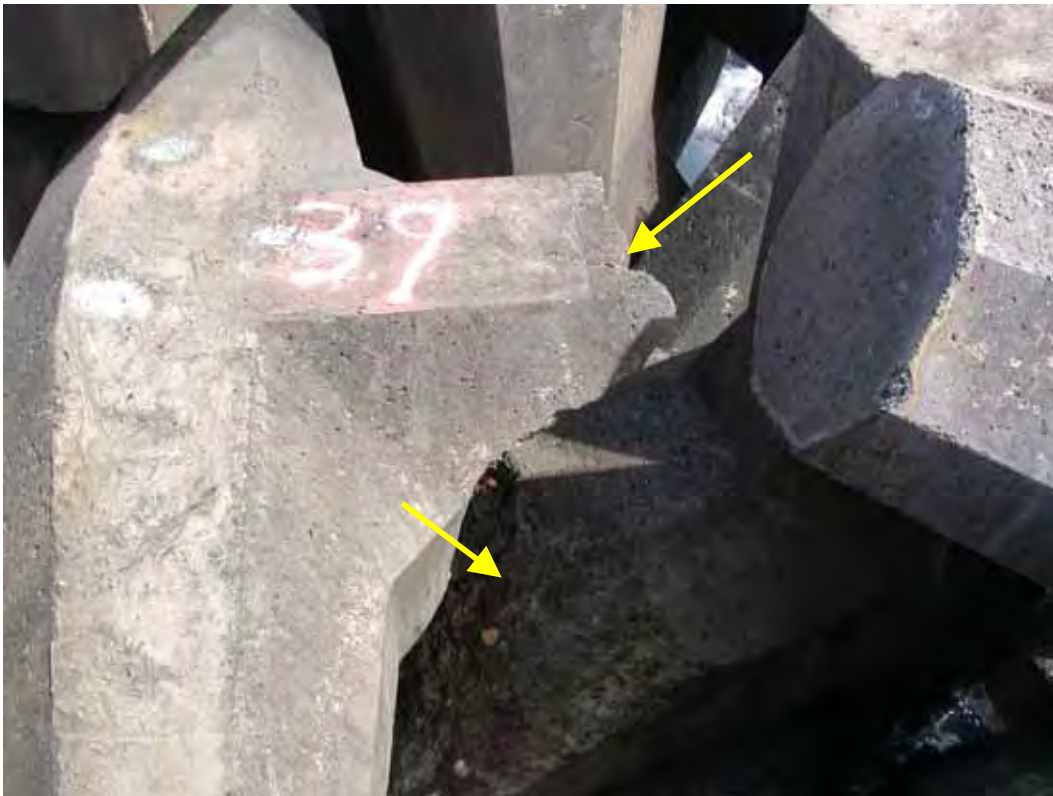
Figure B85. Damage location 54, sta 23+05, ocean side, dolosse with mid shank break.
