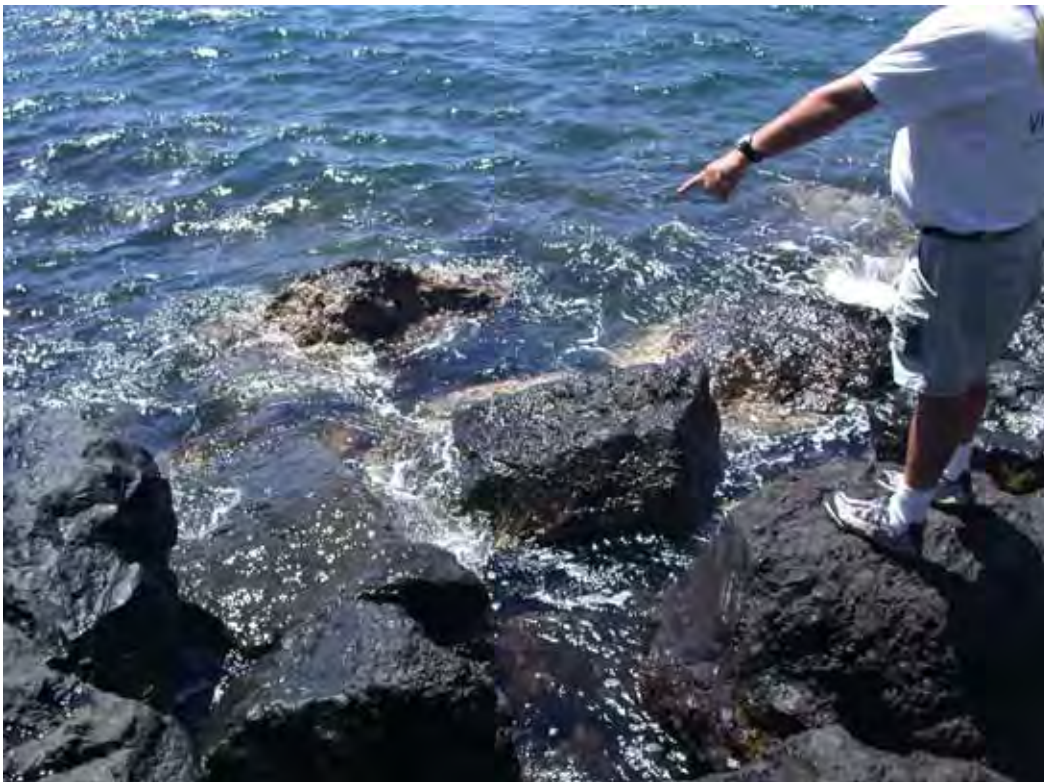
Figure C21. Displaced armor stones at wave absorber along shoreline, harbor side of breakwater.
