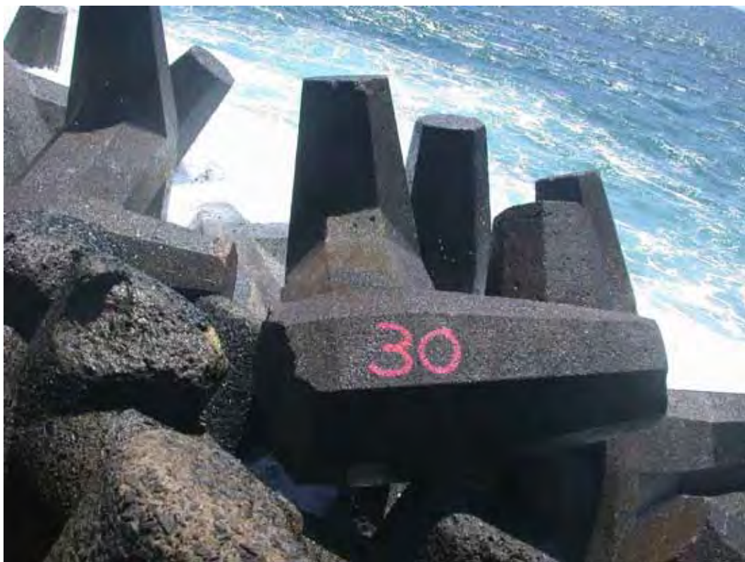
Figure 24. Typical dolosse fluke-shank break.
