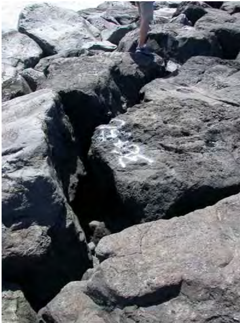
Figure A40. Damage location 42, sta 36+50, void at crest.
