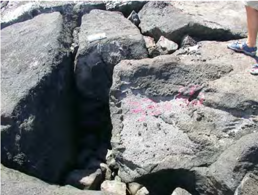
Figure A36. Damage location 38, sta 33+65, void at crest (3 ft x 6 ft x 4.5 ft).
