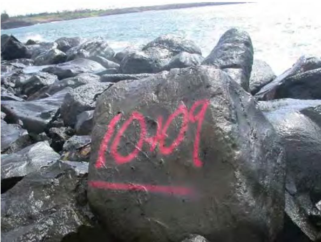
Figure D19. Damage location 18, sta 10+09, perched armor stone with void on crest.
