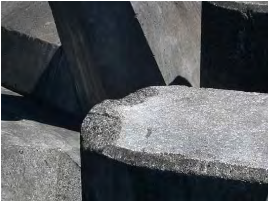
Figure C19. Rib damage possibly caused by displaced armor stones.
