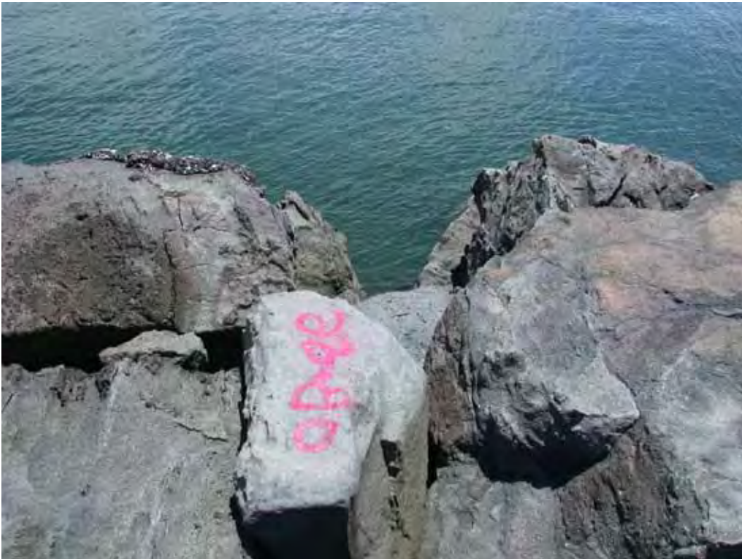
Figure A21. Damage location 20, sta 22+80, harbor side, missing armor stone at hinge.
