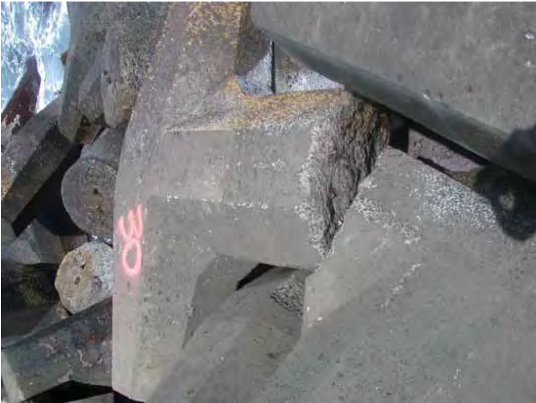
Figure B75. Damage location 41, sta 22+72, ocean side, dolosse with shank-fluke break.
