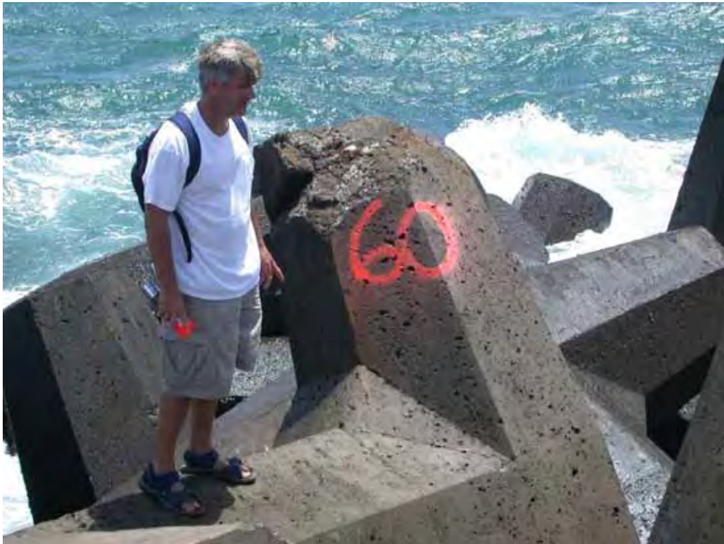
Figure B94. Damage location 72, 30 deg ocean side of head, dolosse with fluke tip chip.
