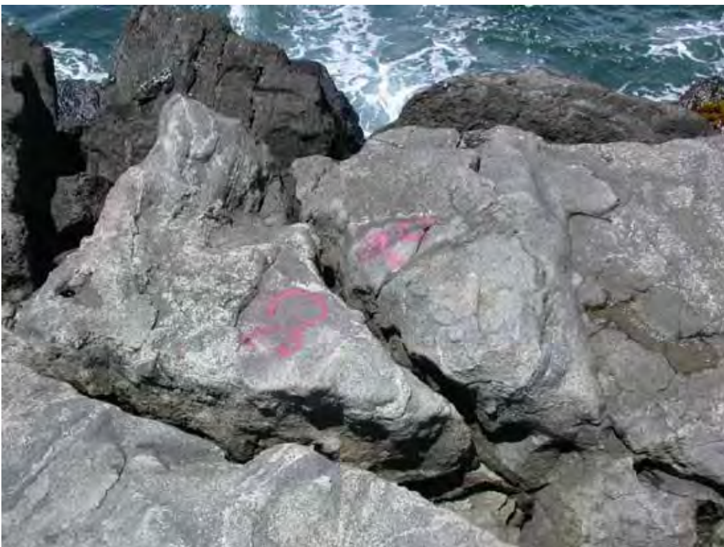
Figure A22. Damage location 21, sta 22+90, ocean side, cracked armor stone.
