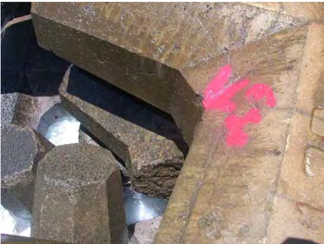
Figure D71. Damage location 96, sta 19+90, ocean side, rib #131, dolosse with shank break.
