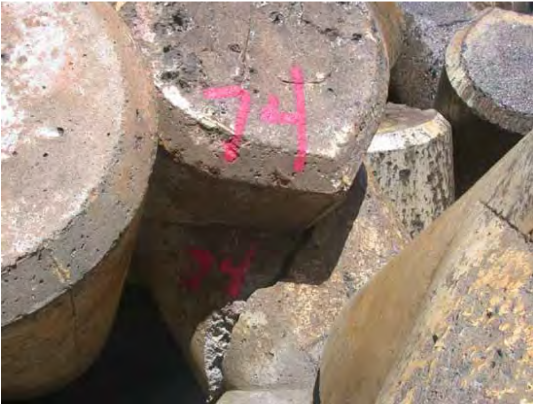
Figure D76. Damage location 107, sta 20+32, ocean side, rib #138, tribar with broken leg.
