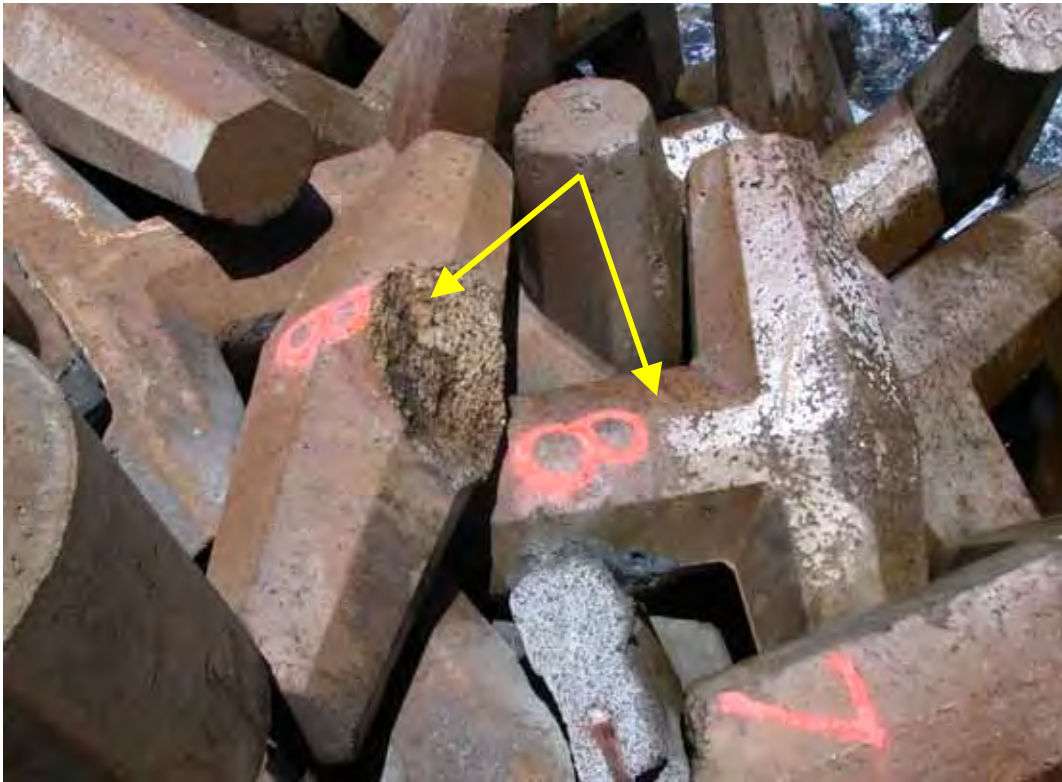
Figure B18. Damage location 22, sta 27+19, ocean side, rib #17, dolosse with straight shank-fluke break.
