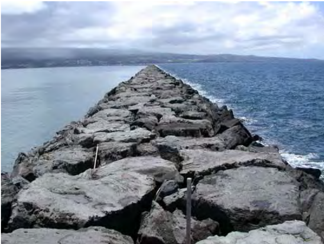
Figure 6. Photograph of Hilo breakwater viewed to the northwest.
