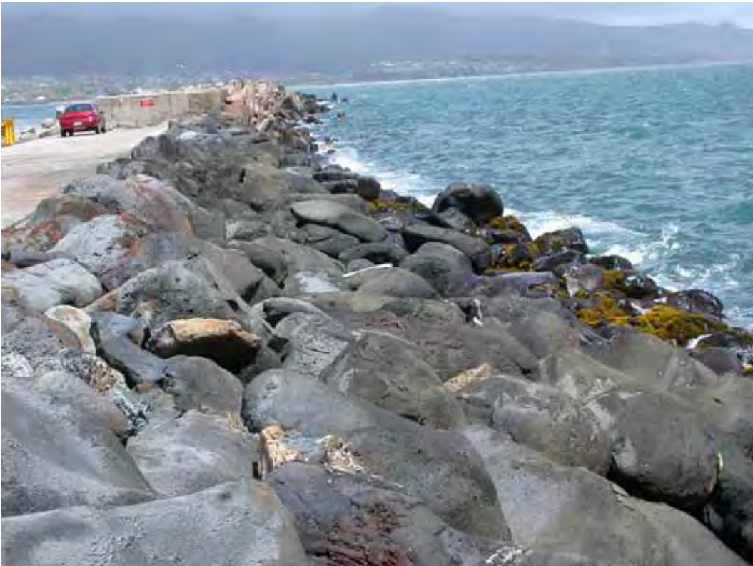
Figure B6. Damage location 11, sta 23+20, ocean side, slight settling.
