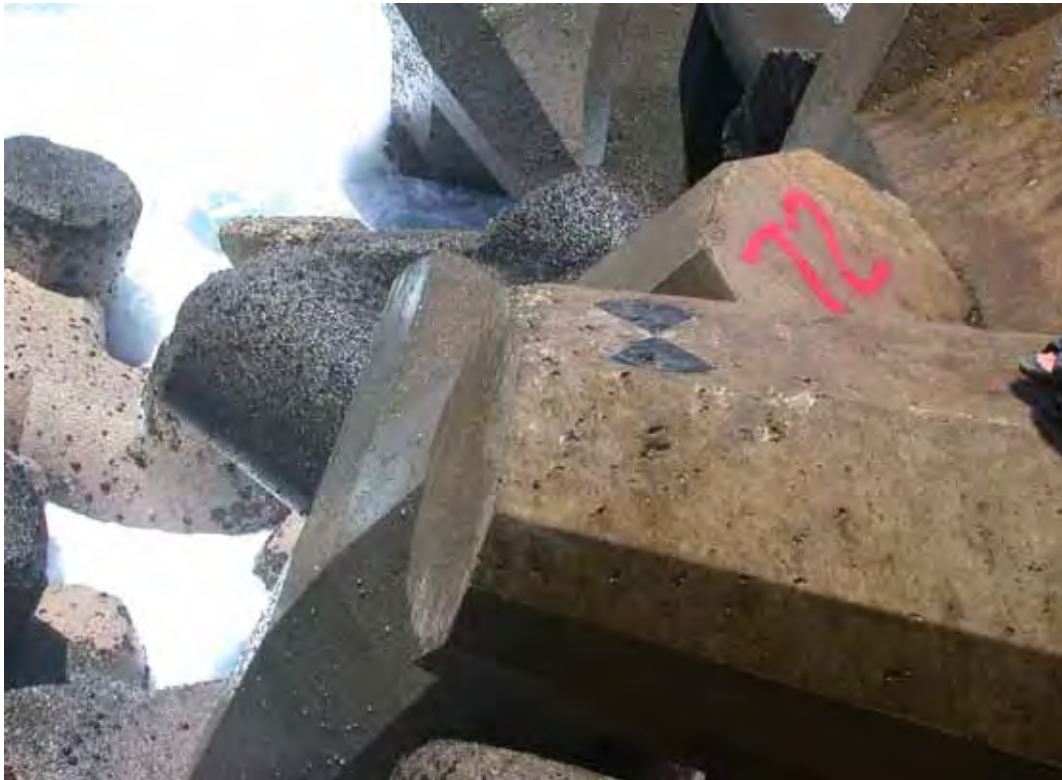
Figure D74. Damage location 105, sta 20+26, ocean side, rib #137, dolosse with multiple breaks.
