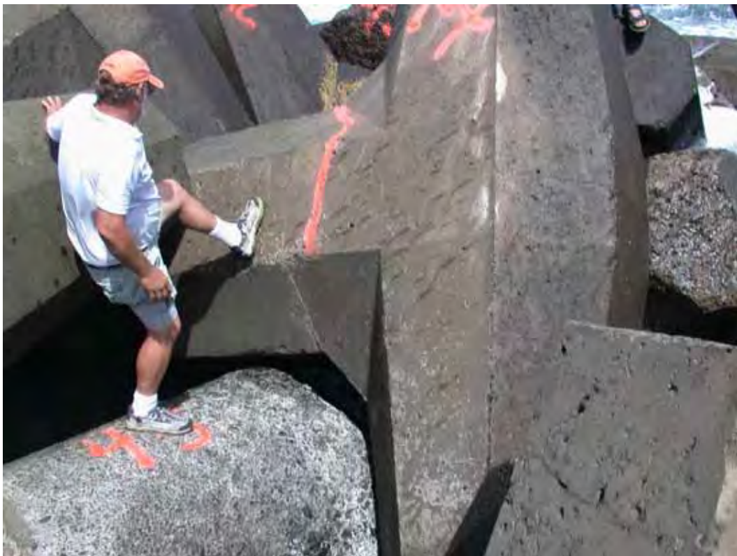
Figure B88. Damage location 58, sta 23+25, ocean side, dolosse with shank-fluke crack.
