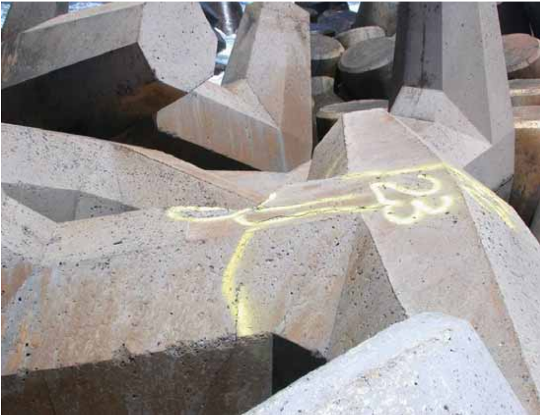
Figure B39. Damage location 54, sta 34+15, ocean side, rib #130, dolosse with crack through shank.
