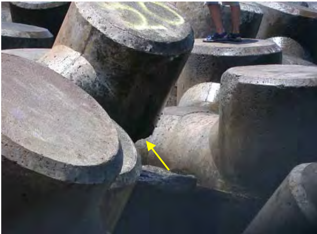
Figure B33. Damage location 44, sta 32+62, ocean side, rib #106, tribar with broken leg.
