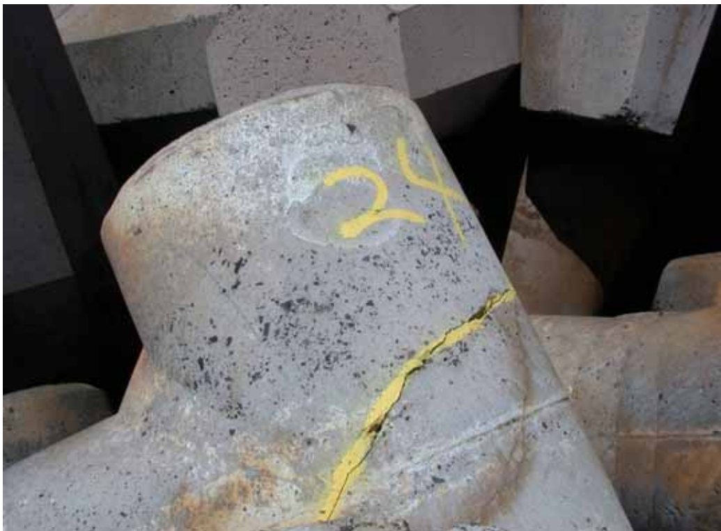
Figure B40. Damage location 55, sta 34+27, ocean side, rib #132, tribar with mid leg break.
