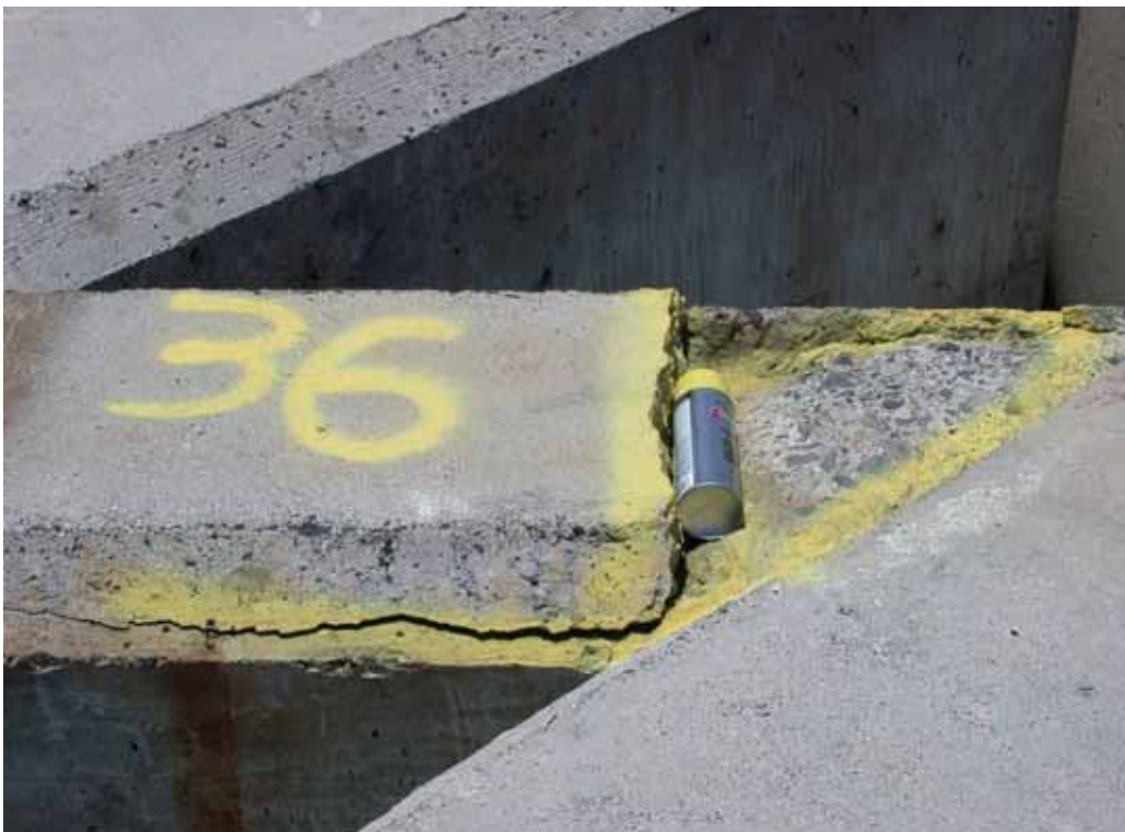
Figure B50. Damage location 8, sta 20+58, rib #36, red cross painted on rib cap (not visible in photograph) and spalling.
