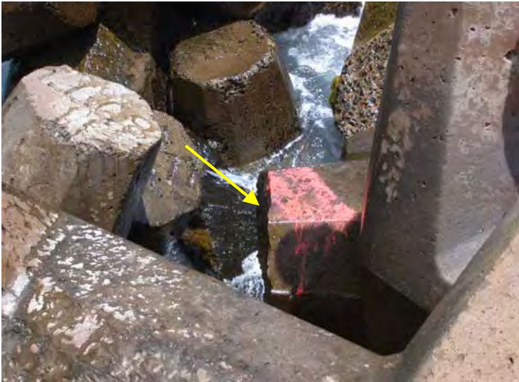
Figure B20. Damage location 25, sta 27+69, ocean side, rib #23, dolosse with shank-fluke break.
