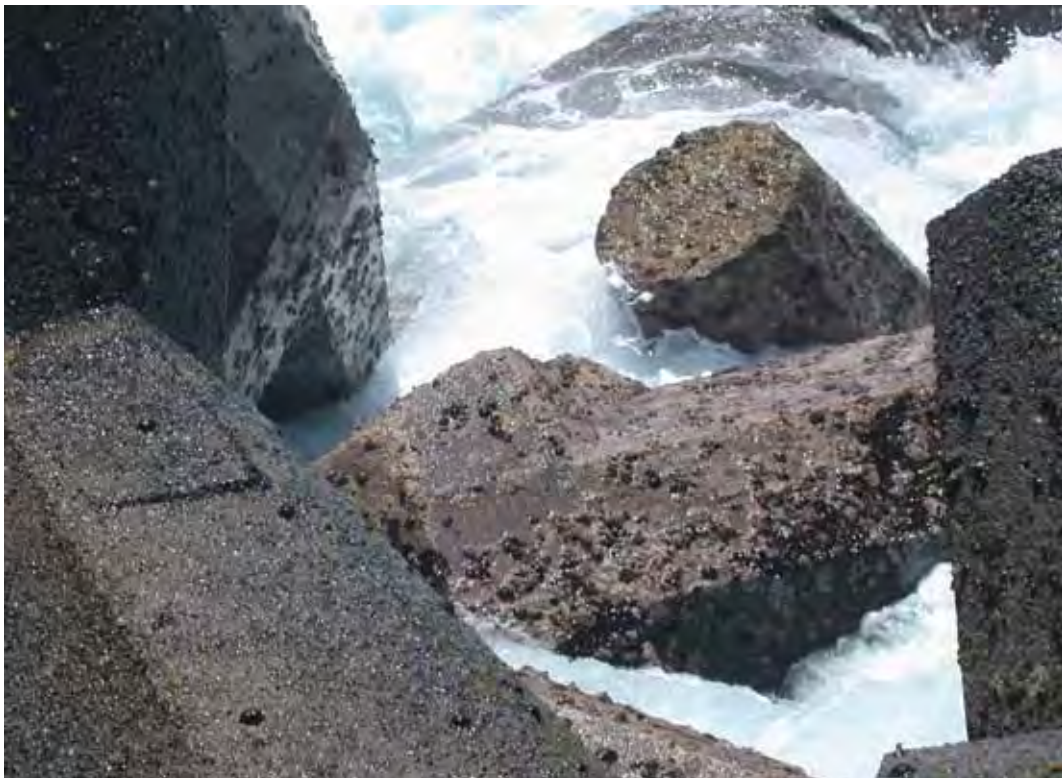
Figure D54. Damage location 71, sta 17+22, ocean side, rib #88, dolosse with multiple breaks at waterline.
