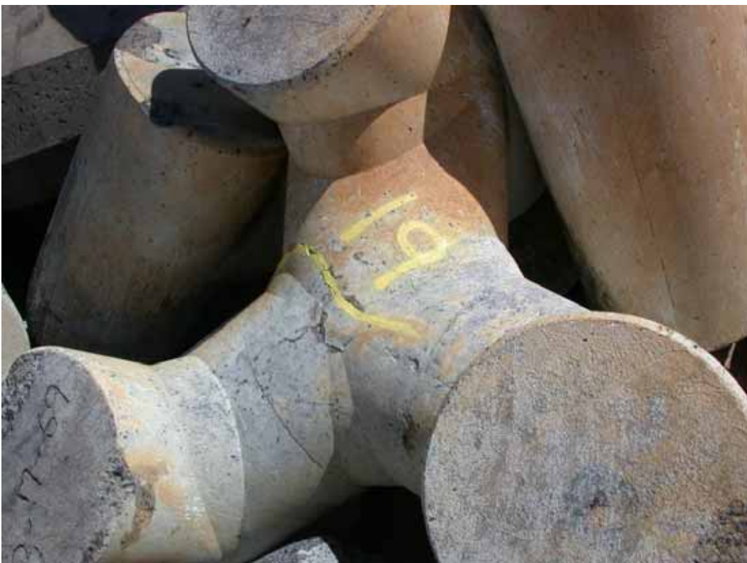
Figure B62. Damage location 25, sta 21+95, ocean side, tribar with crack.
