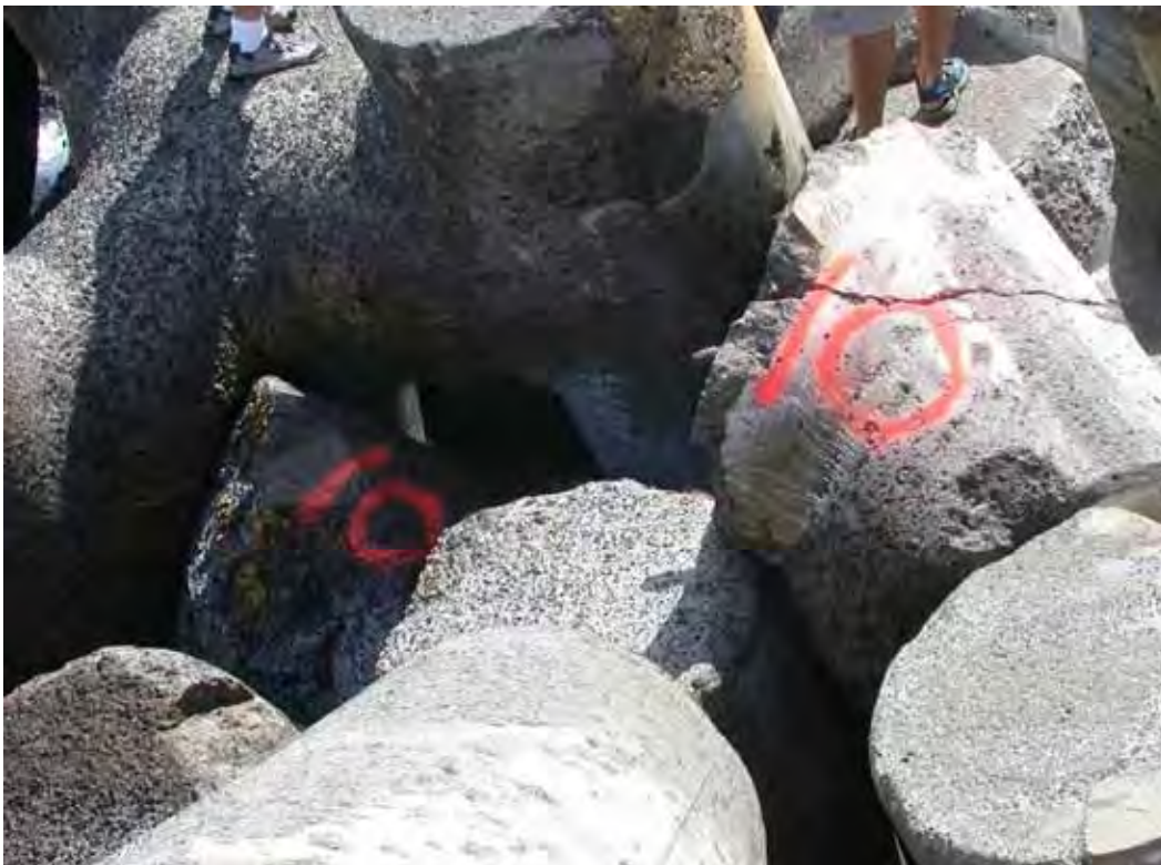
Figure B54. Damage location 15, sta 21+22, ocean side, rib #44, tribar broken into three pieces.
