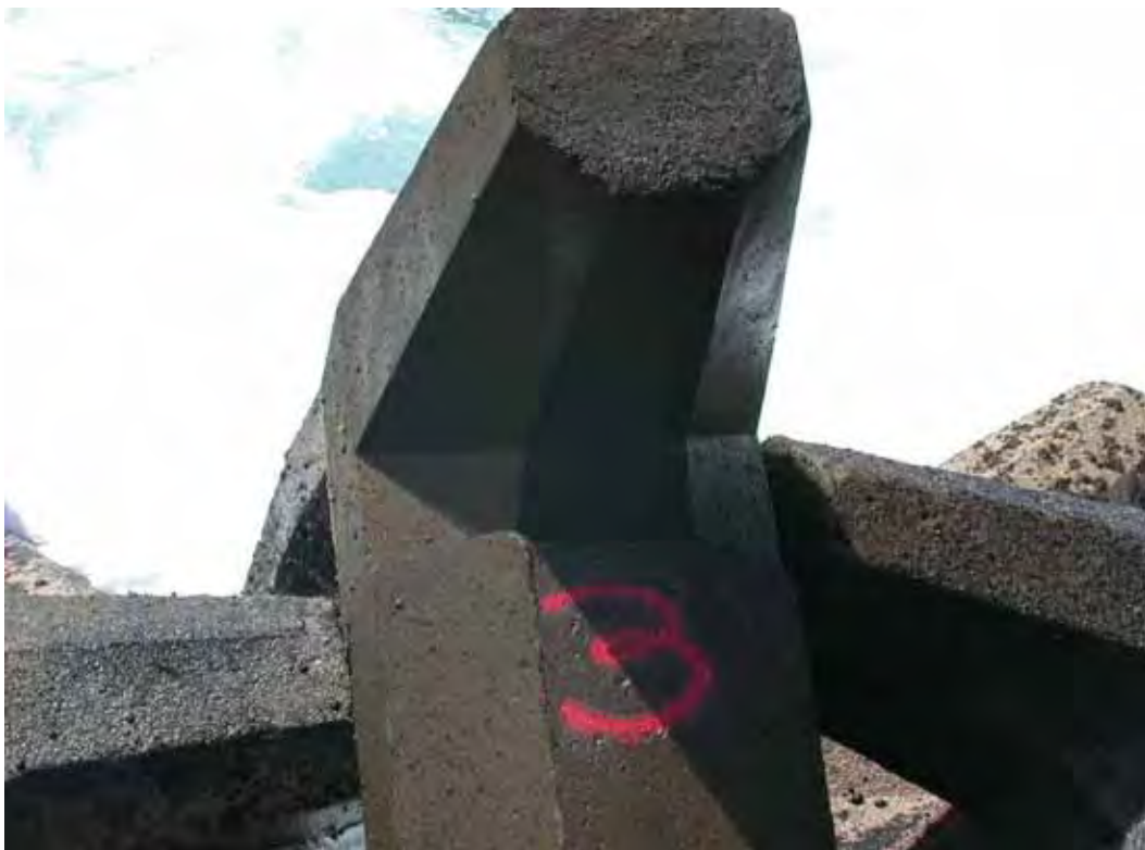
Figure D25. Damage location 26, sta 12+06, ocean side, rib #2, dolosse with shank-fluke break.
