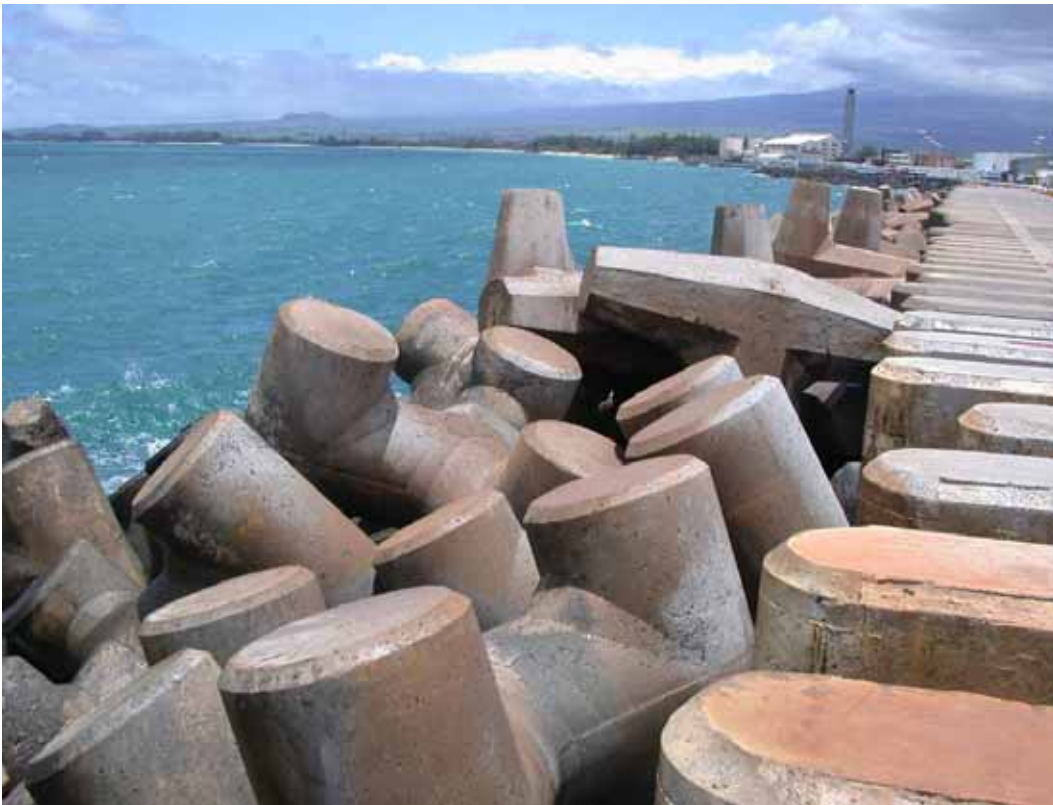
Figure B27. Sta 30+64 – 30+70, ocean side, ribs #73 - #74, transition of dolosse to tribar.
