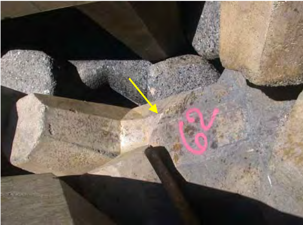
Figure D70. Damage location 94, sta 19+78, ocean side, rib #129, dolosse with mid-shank break.
