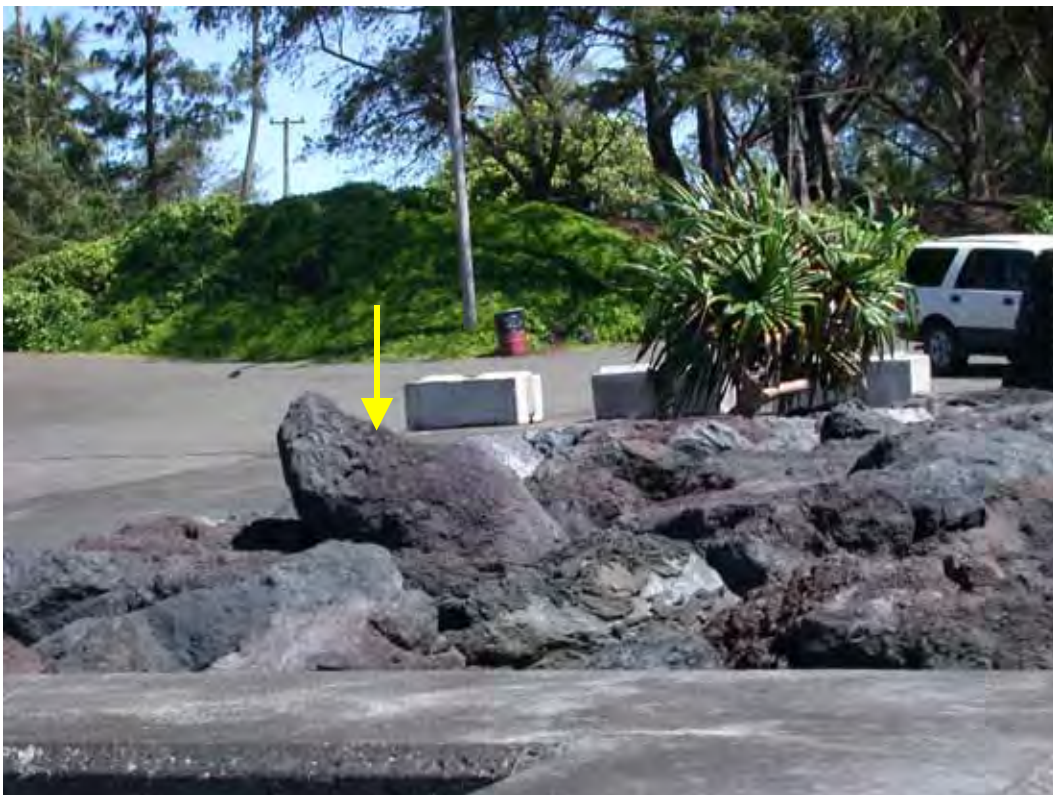
Figure C7. Harbor side, perched armor stone.
