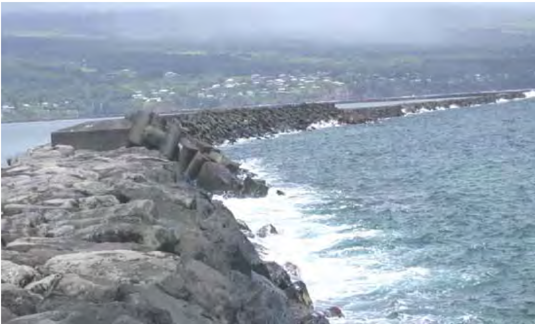
Figure 5. Photograph of Hilo breakwater 1981 repair section viewed east to west.
