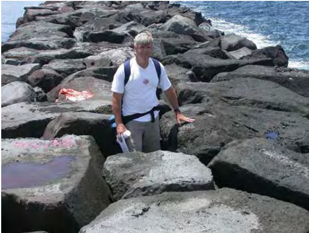
Figure A28. Damage location 27, sta 25+85, void at crest.
