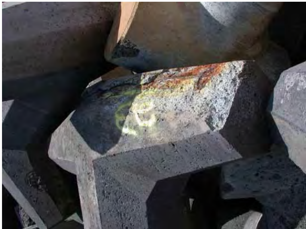
Figure B66. Damage location 29, sta 22+14, ocean side, dolosse with spalling.
