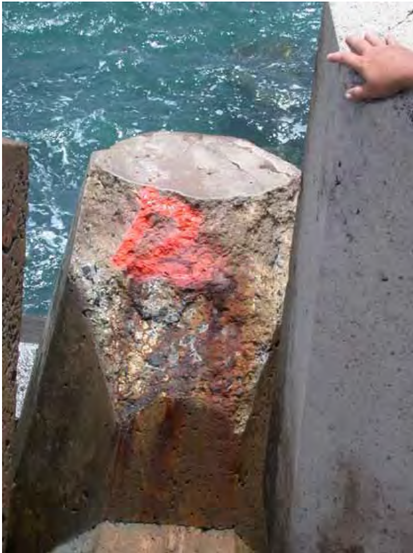
Figure B21. Damage location 26, sta 28+04, ocean side, rib #30, dolosse with tip chip.
