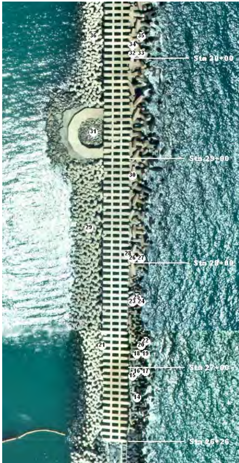
Figure 32. Approximate damage locations on Kahului East Breakwater, photograph 2.
