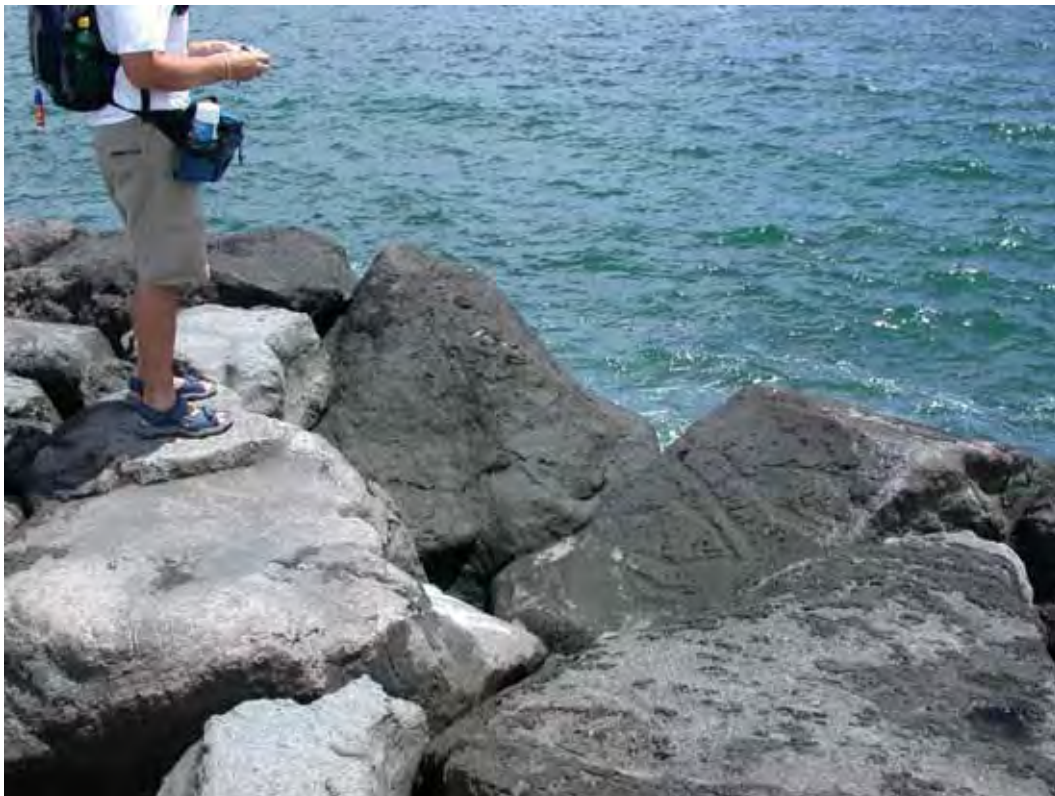
Figure A5. Damage location 4, sta 9+08, ocean side, void.
