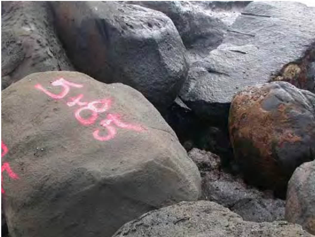
Figure D5. Damage location 4, sta 5+85, ocean side, void on side slope.
