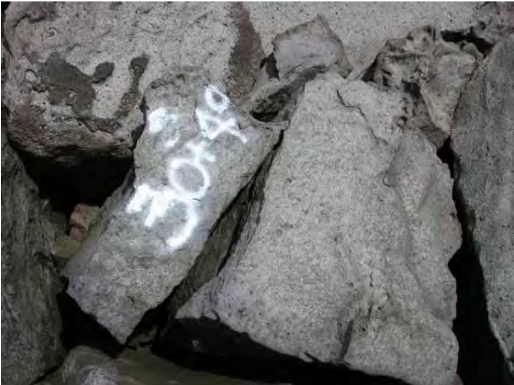
Figure A32. Damage location 34, sta 30+40, broken stone on crest.
