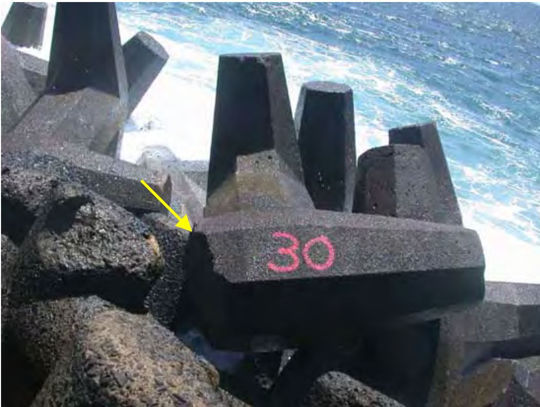
Figure D46. Damage location 63, sta 16+14, ocean side, rib #70, dolosse with fluke tip break.
