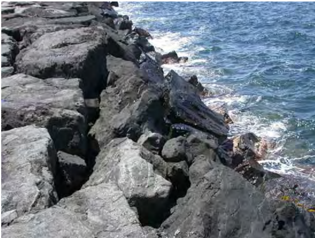
Figure A26. Damage location 25, sta 25+30, hinge stone separating.
