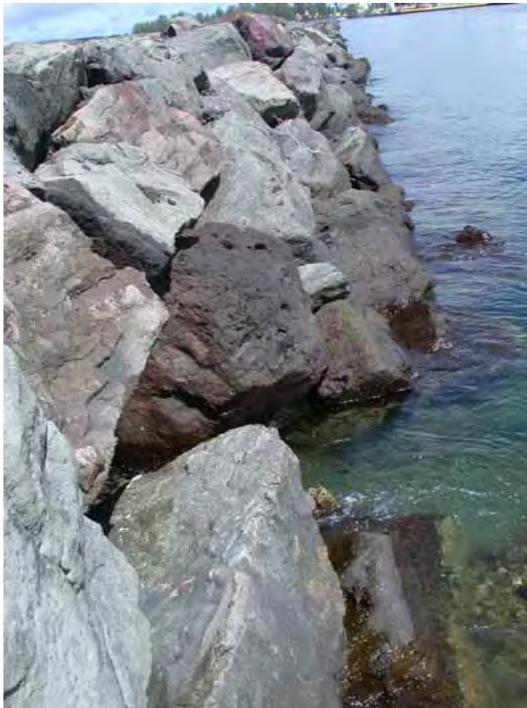
Figure A39. Damage location 41, sta 36+10, large void at crest from centerline to harbor side, missing toe stone, two large rock separations.
