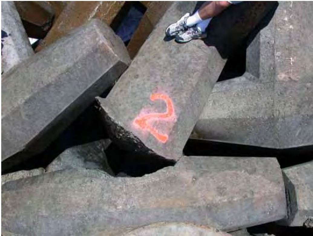
Figure B12. Damage location 15, sta 26+92, ocean side, rib #12, dolosse with straight shank-fluke break.
