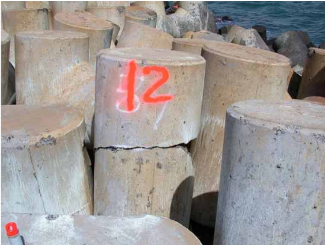
Figure B55. Damage location 17, sta 21+38, ocean side, rib #46, tribar with broken leg.
