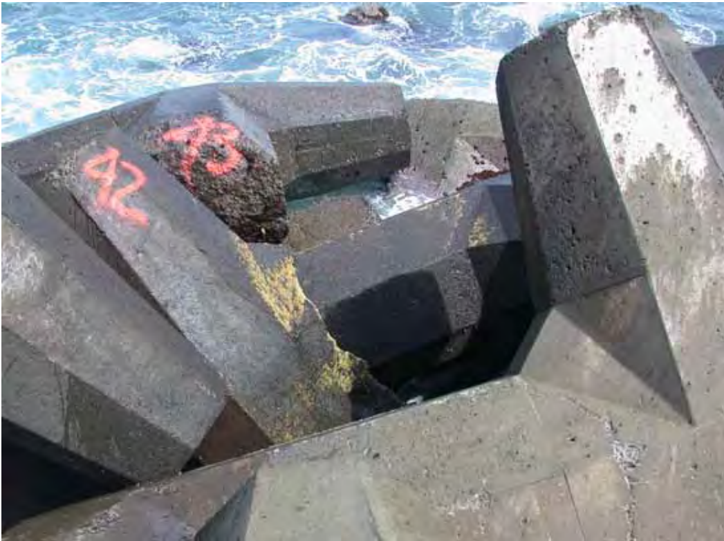
Figure B87. Damage locations 56 & 57, sta 23+19, ocean side, two dolosse with shank-fluke breaks.
