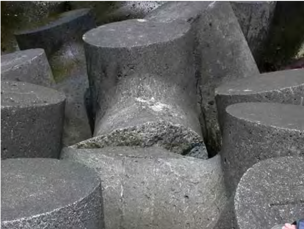
Figure A13. Damage location 15, sta 16+00, rib #85, tri-bar broken through center.
