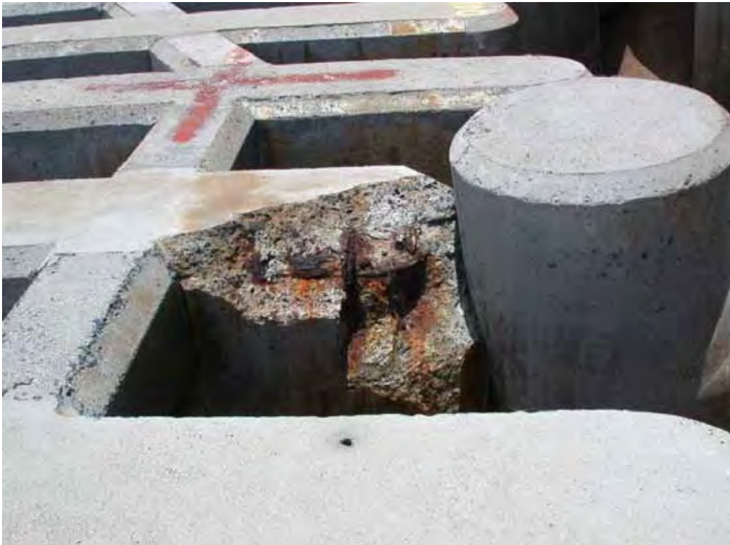
Figure B32. Damage location 42, sta 32+16, ocean side, rib #98, cracked and spalling rib cap, red cross painted on rib cap.
