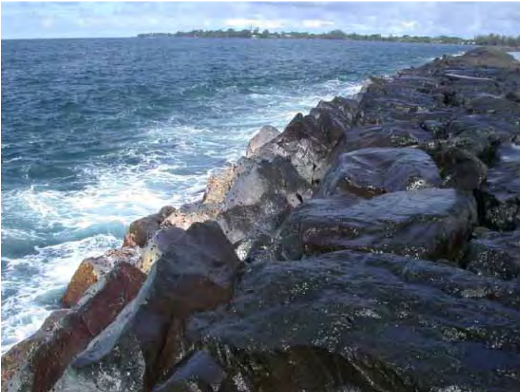
Figure A53. Damage location 57, sta 55+56 and 59+30, ocean side, settling at crest.
