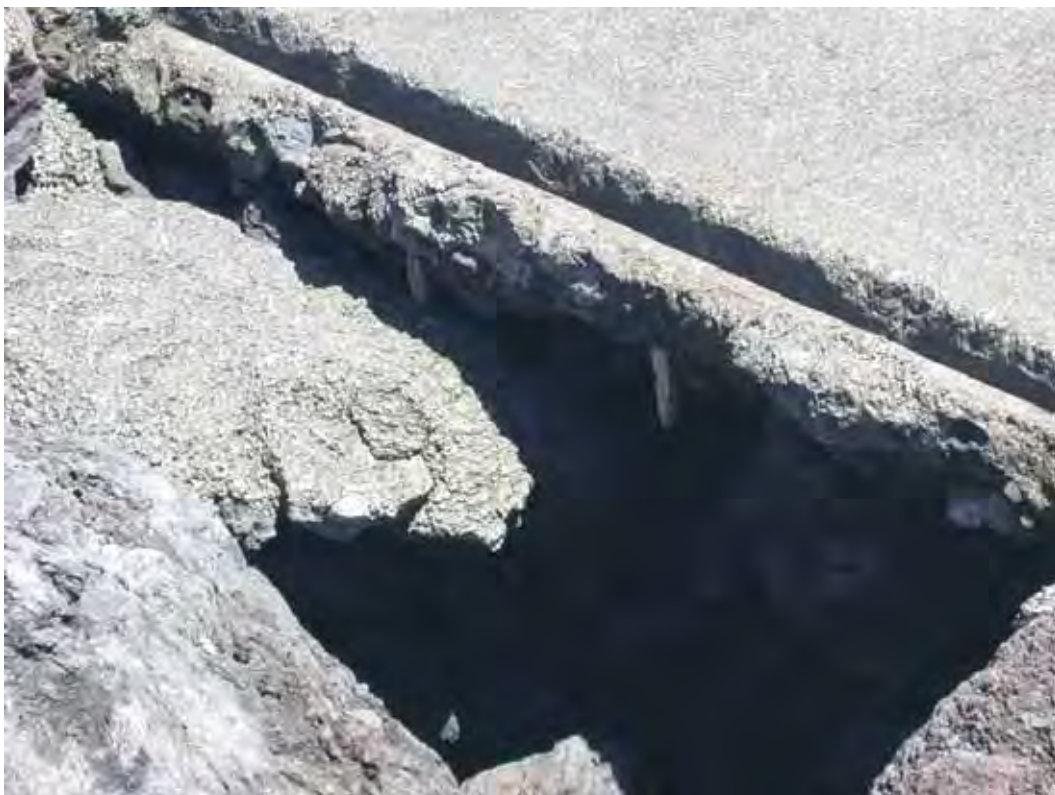
Figure C20. Undermining of concrete slab adjacent to breakwater and boat launch.
