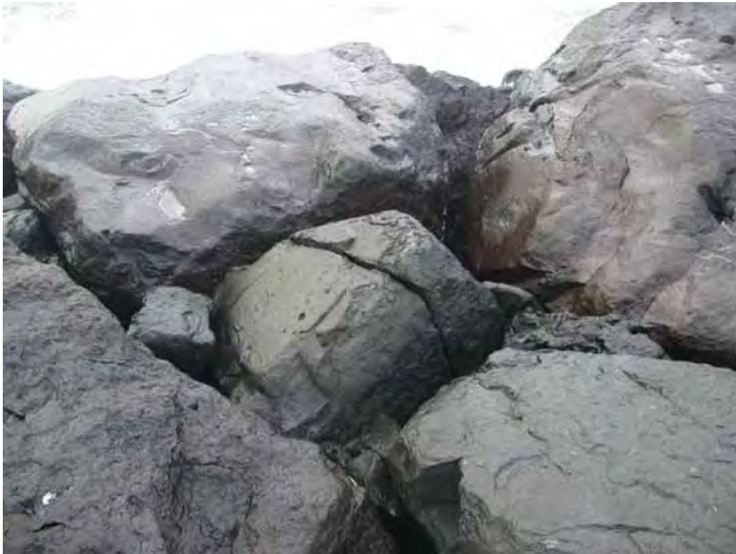
Figure A66. Damage location 77, sta 77+80, cracked armor stone on centerline of crest.
