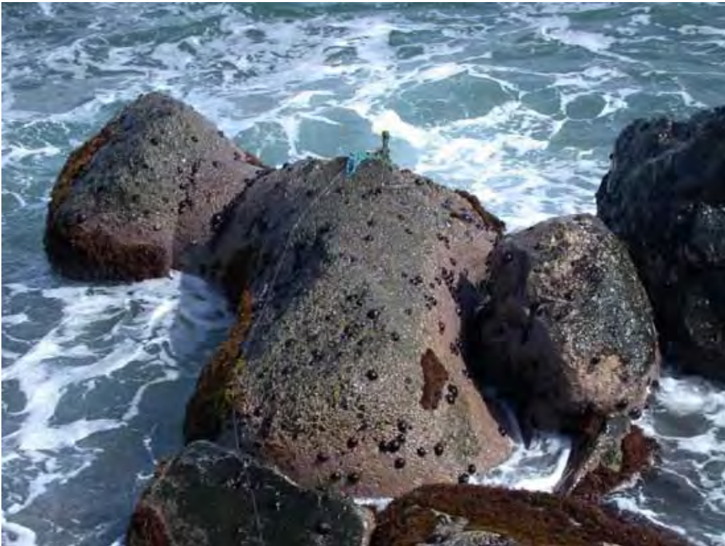
Figure B44. Damage location 1, sta 17+10, ocean side, tribar out of place at waterline.
