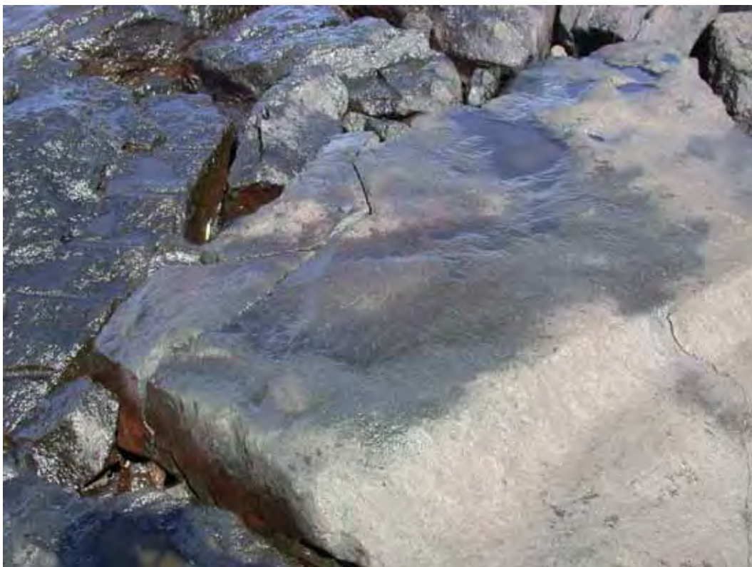
Figure A49. Damage location 53, sta 54+30, broken stone on crest.
