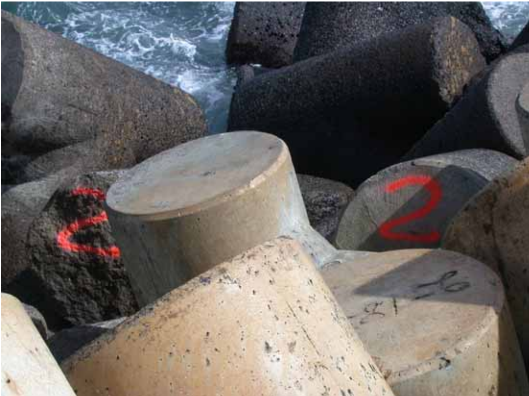
Figure B51. Damage location 9, sta 20+66, ocean side, rib #37, tribar with can break.
