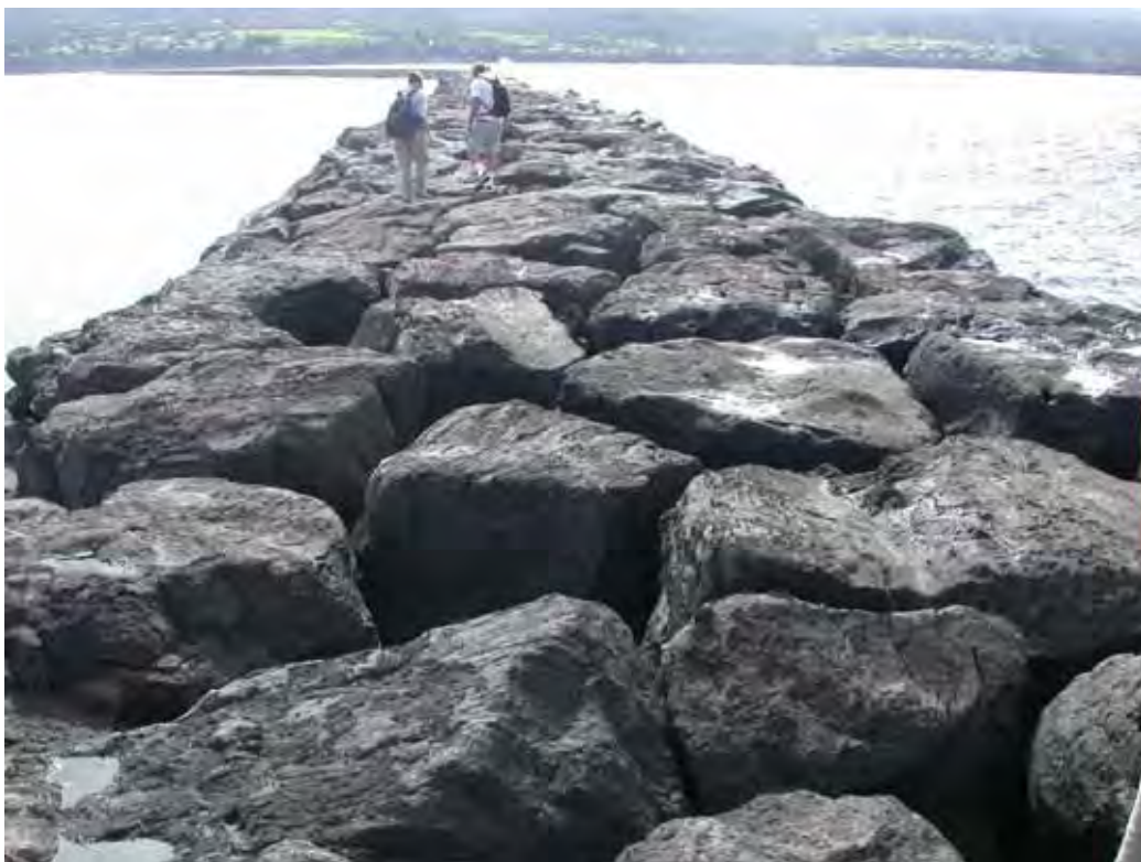
Figure A56. Damage location 60, sta 61+13-and 61+50, numerous armor stone separations and voids.
