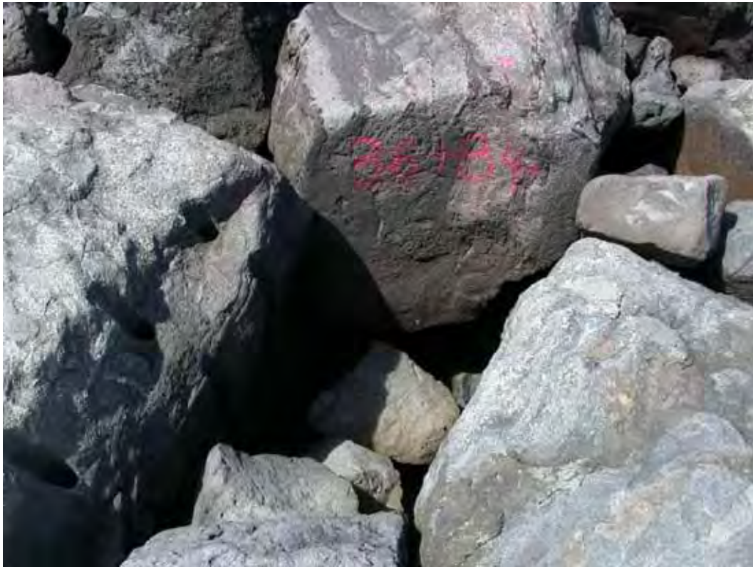
Figure A38. Damage location 40, sta 35+84, void at crest.
