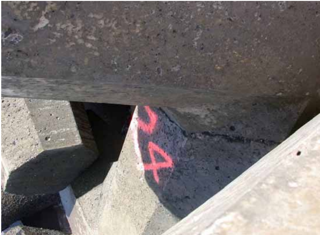
Figure B67. Damage location 30, sta 22+20, ocean side, dolosse with shank-fluke break held together by rebar.
