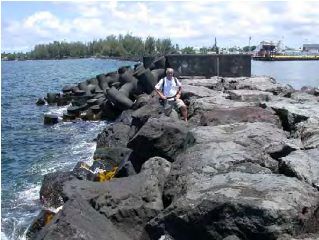
Figure A19. Damage location 18, sta 20+30, ocean side, void.
