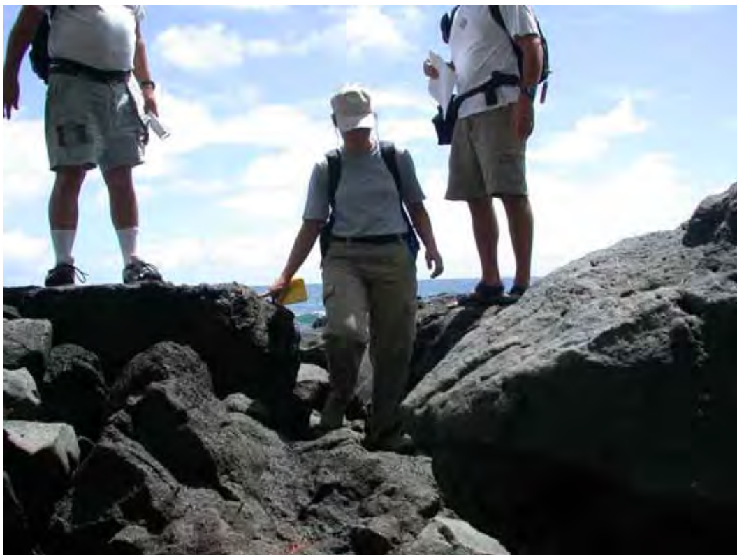
Figure A2. Damage location 1, sta 2+60, harbor side, missing armor stone, 8-ft x 4-ft void.
