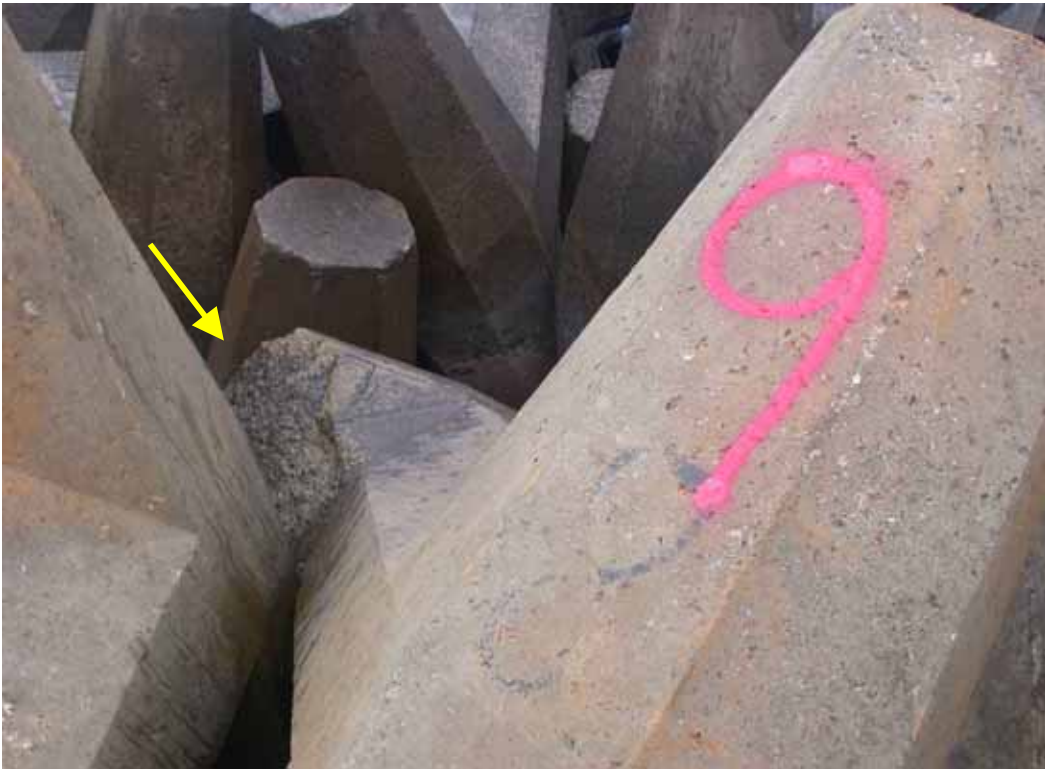
Figure D34. Damage location 39, sta 13+62, ocean side, rib #28, dolosse with fluke-shank break.
