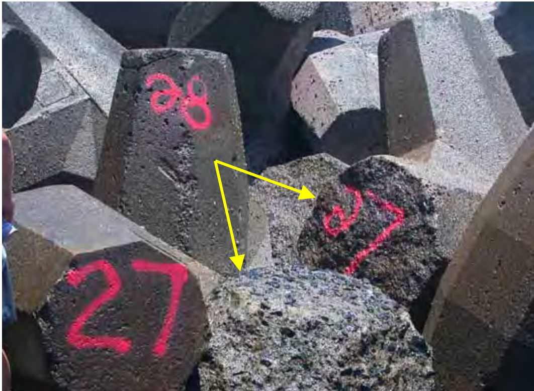
Figure D44. Damage locations 59 & 60, sta 15+96 - 16+02, ocean side, rib #67 & 68, two dolosse with mid-shank breaks.
