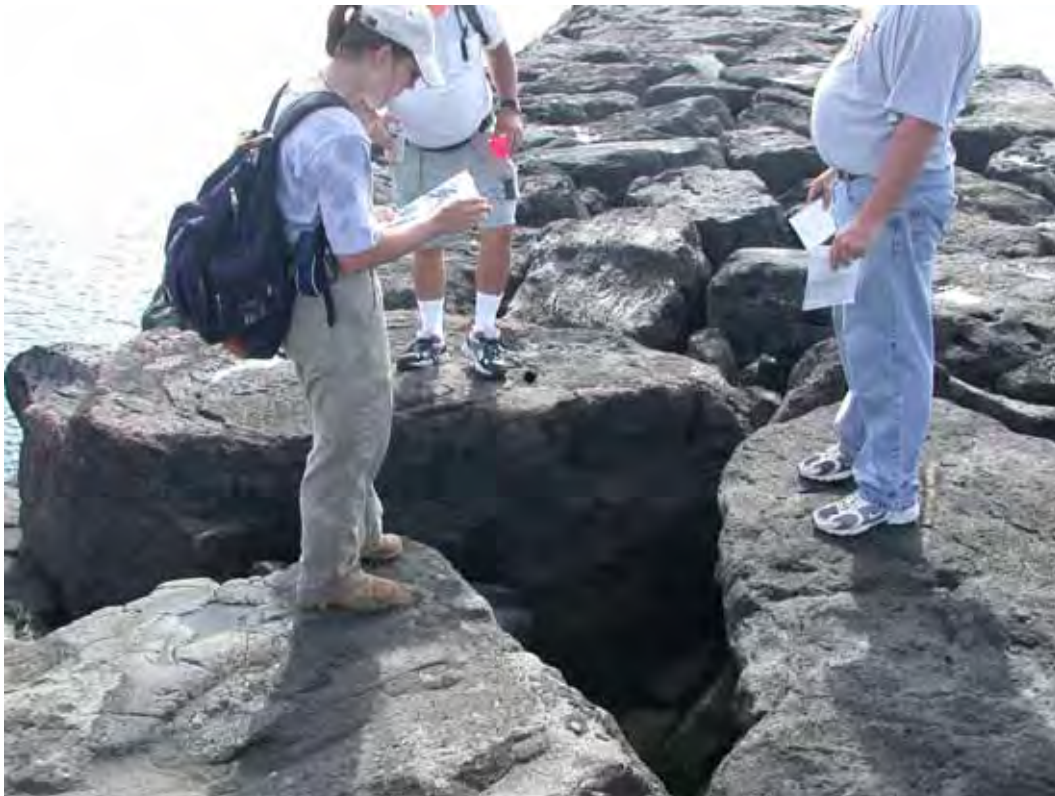
Figure A55. Damage location 59, sta 60+80, harbor side, void at crest (2 ft x 4 ft x 4 ft).
