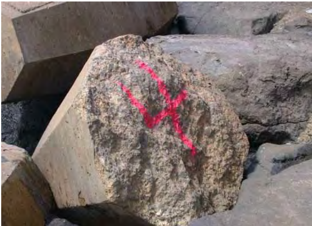
Figure D27. Damage location 28, sta 12+30, ocean side, rib #6, detached dolosse fluke tip, origin unknown.
