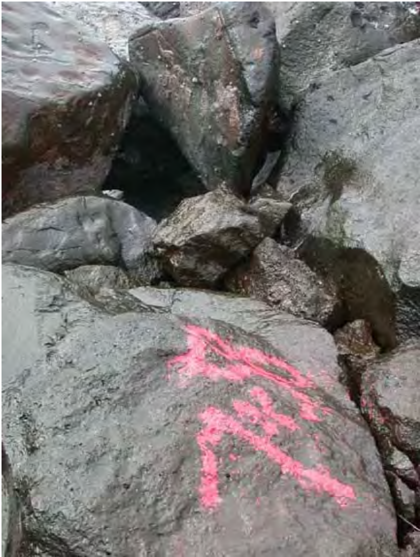
Figure D10. Damage location 9, sta 7+58, settling of crest.
