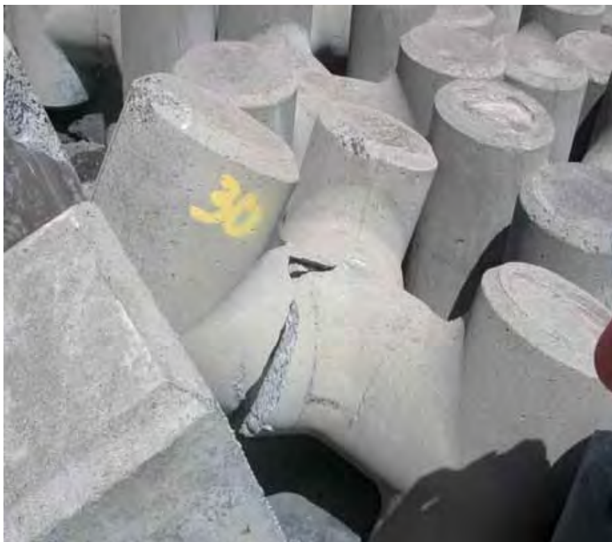
Figure B24. Damage location 29, sta 28+30, harbor side, rib #34, tribar with break through center.
