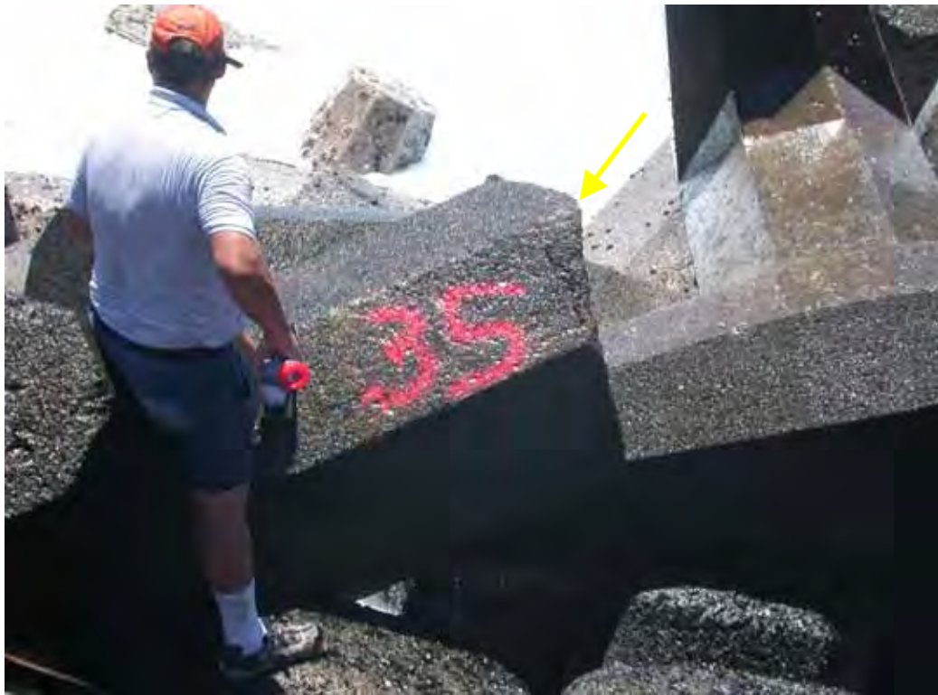
Figure D51. Damage location 67, sta 16+74, ocean side, rib #80, dolosse with shank-fluke break.
