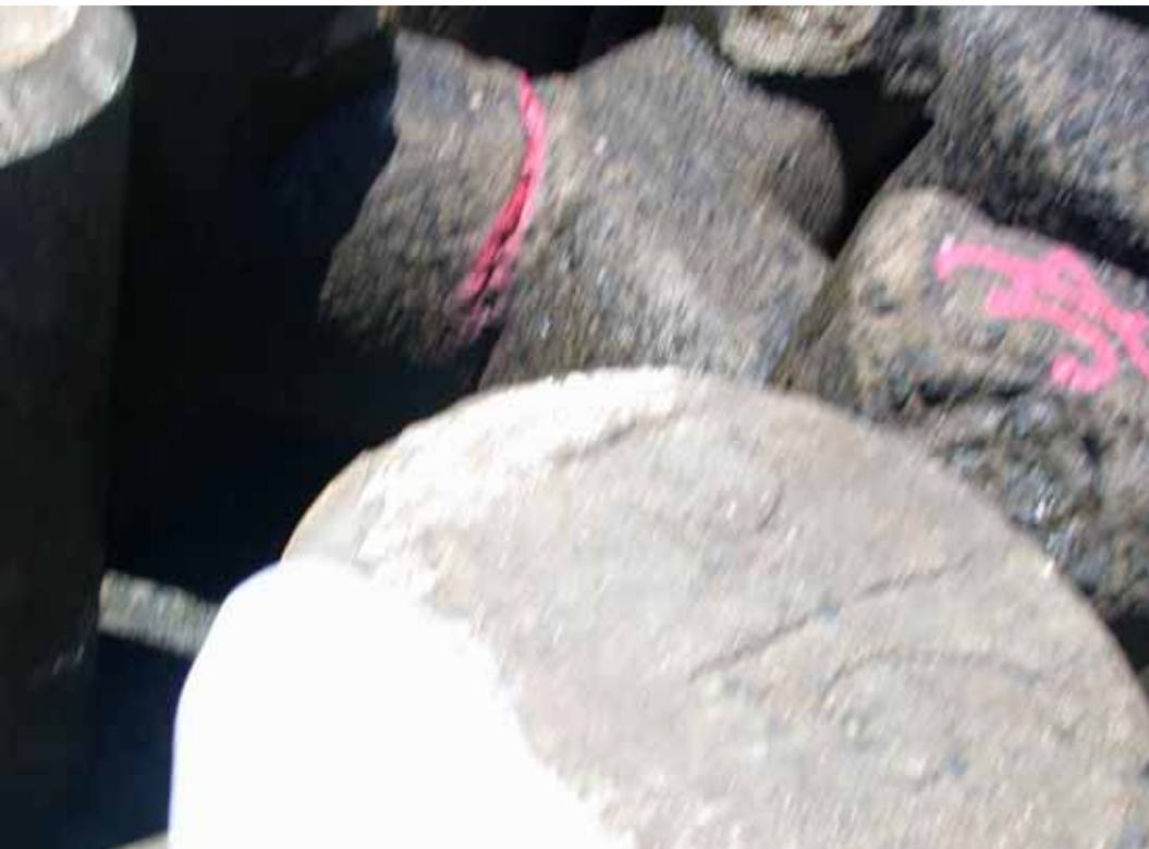
Figure D50. Damage location 66, sta 16+68, ocean side, rib #79, tribar broken through center-no separation.
