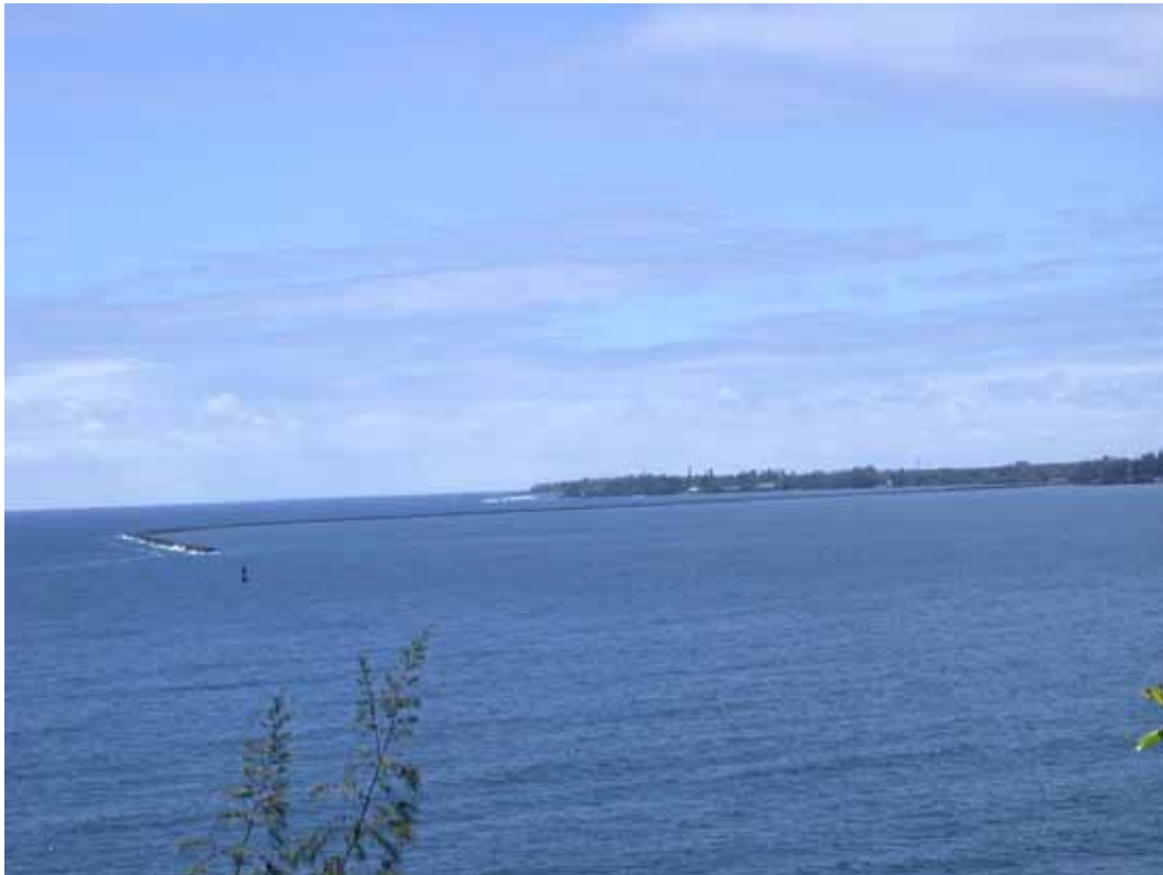
Figure A1. Overview of structure.
