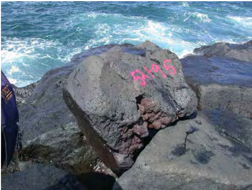
Figure A48. Damage location 52, sta 52+95, ocean side, perched armor stone.
