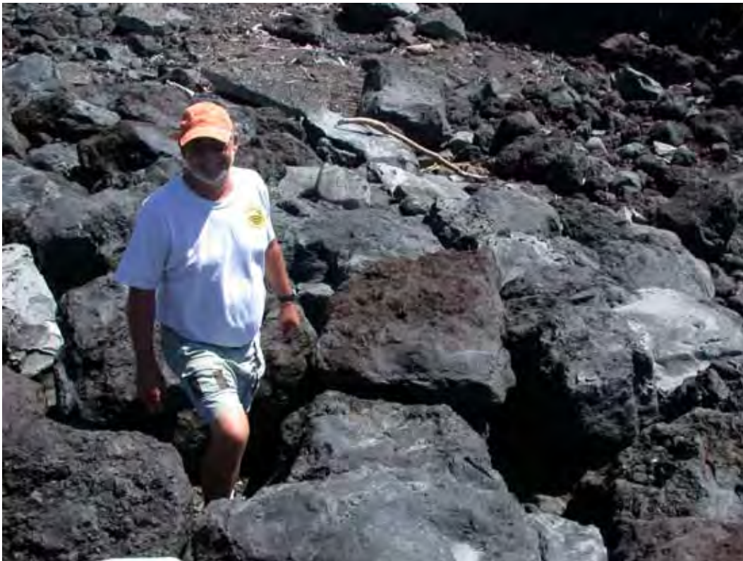
Figure C1. Sta 0+25 - 0+28, voids and missing armor stones.
