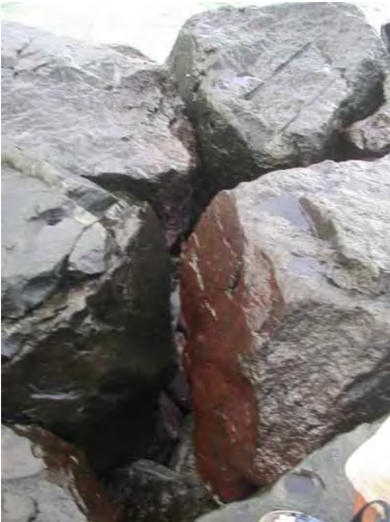
Figure A67. Damage location 80, sta 89+30, bridging.
