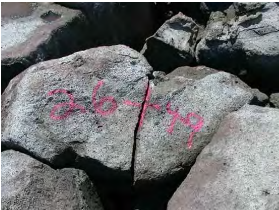
Figure A29. Damage location 29, sta 26+49, harbor side, broken armor stone.
