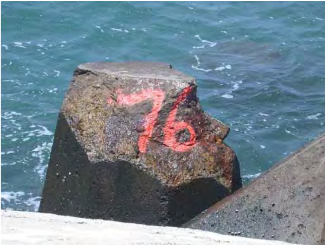
Figure B71. Damage location 36, sta 22+48, harbor side, dolosse with fluke tip break.
