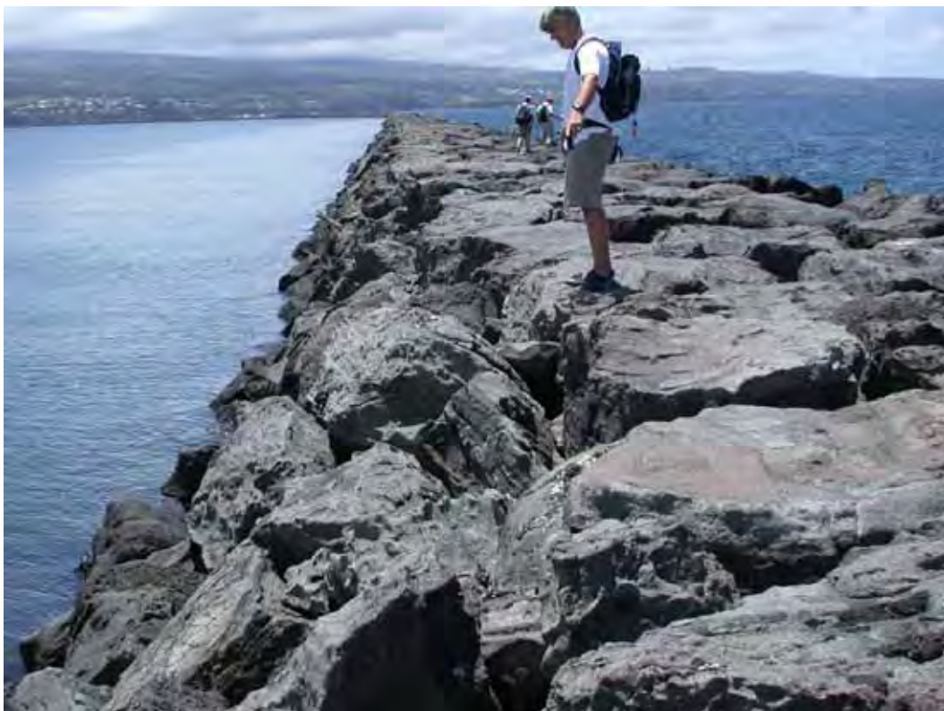
Figure A20. Damage location 19, sta 22+10, harbor side, sloped crest.
