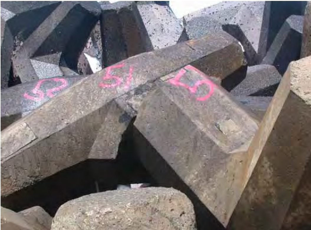
Figure D62. Damage location 83, sta 19+08, ocean side, rib #119, dolosse with shank-fluke break.
