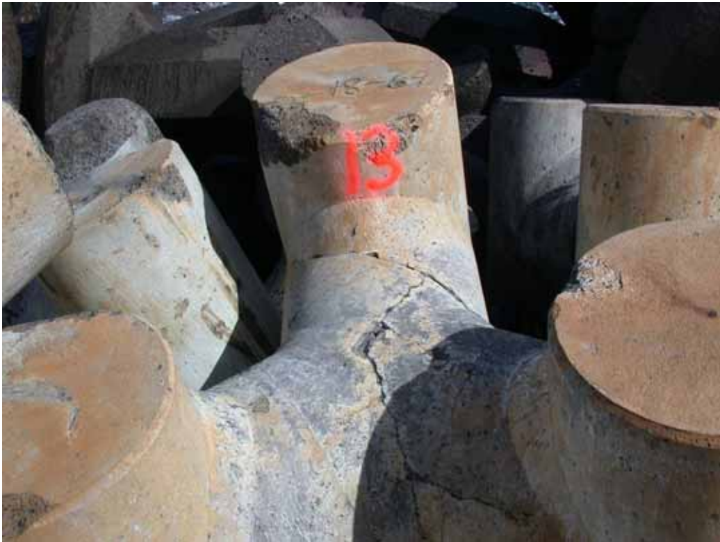
Figure B57. Damage location 19, sta 21+54, ocean side, rib #48, tribar with multiple cracks through center.
