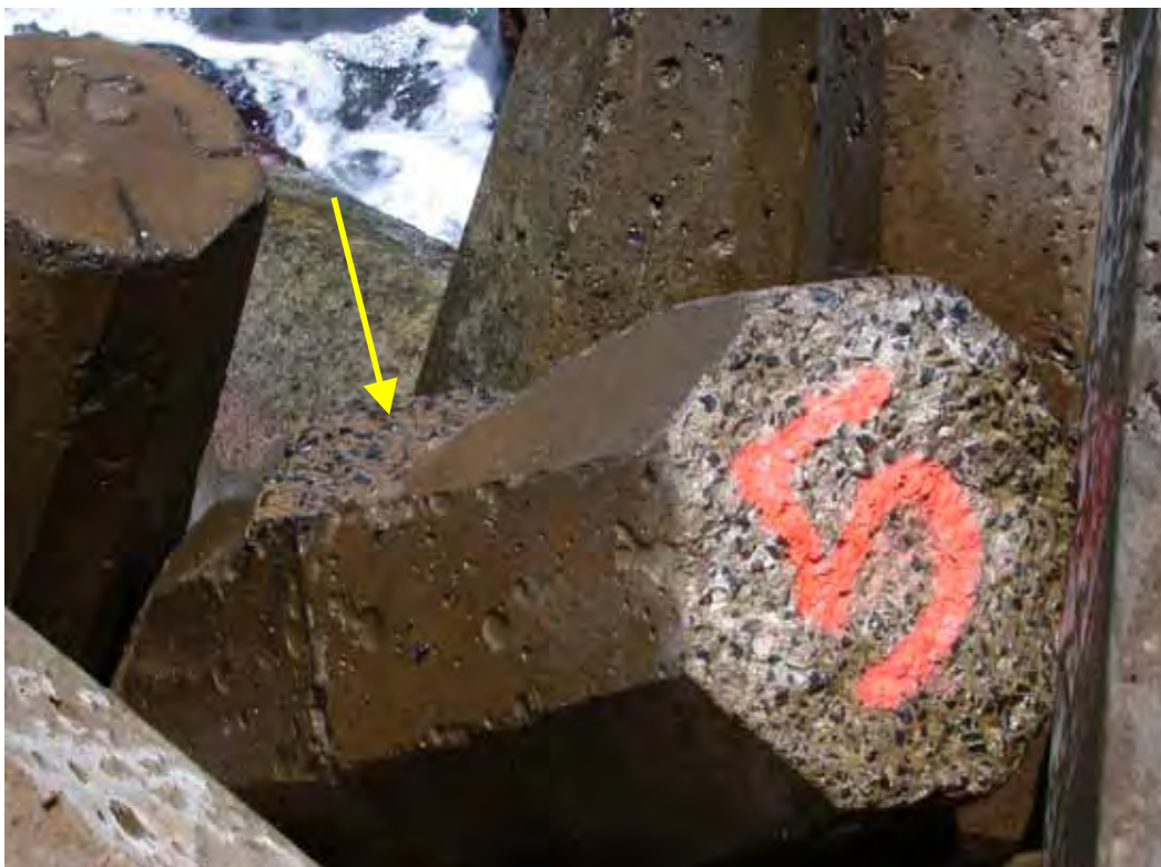
Figure B15. Damage location 18, sta 27+09, ocean side, rib #15, dolosse with shank-fluke break.
