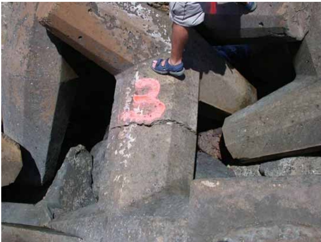
Figure B13. Damage location 16, sta 26+97, ocean side, dolosse with mid-shank break.
