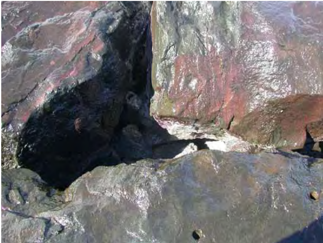
Figure A51. Damage location 55, sta 57+35, void at crest (10 ft x 2 ft x 4 ft).
