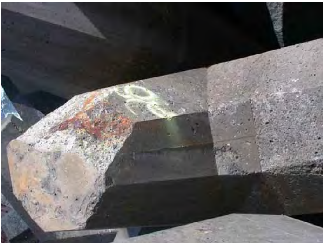
Figure B70. Damage location 35, sta 22+38, ocean side, dolosse with tip break.
