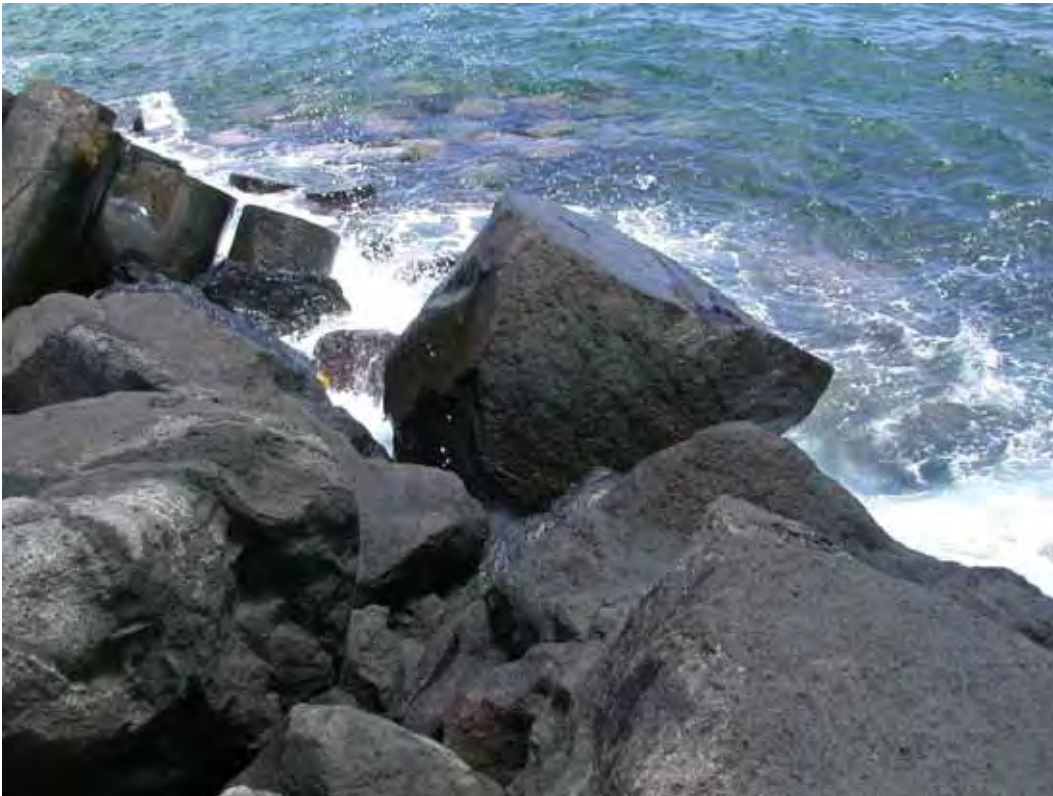
Figure A7. Damage location 6, sta 10+80, ocean side, dislodged stone.
