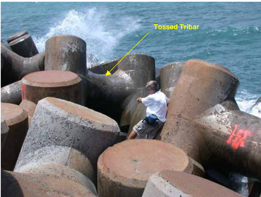
Figure B30. Damage location 39, sta 31+54, ocean side, rib #88, tossed 9-ton tribar.
