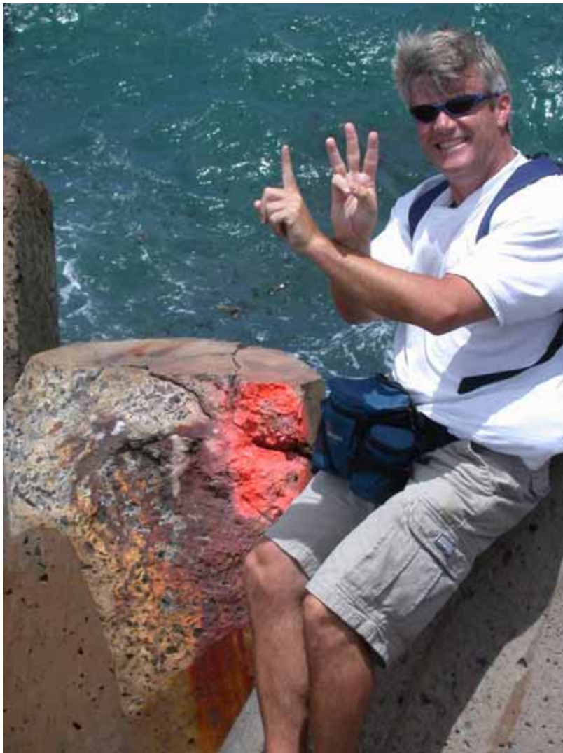
Figure B22. Damage location 27, sta 28+04, ocean side, rib #30, dolosse with tip chip.
