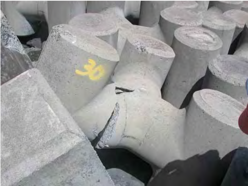
Figure 26. Typical tribar center section break.
