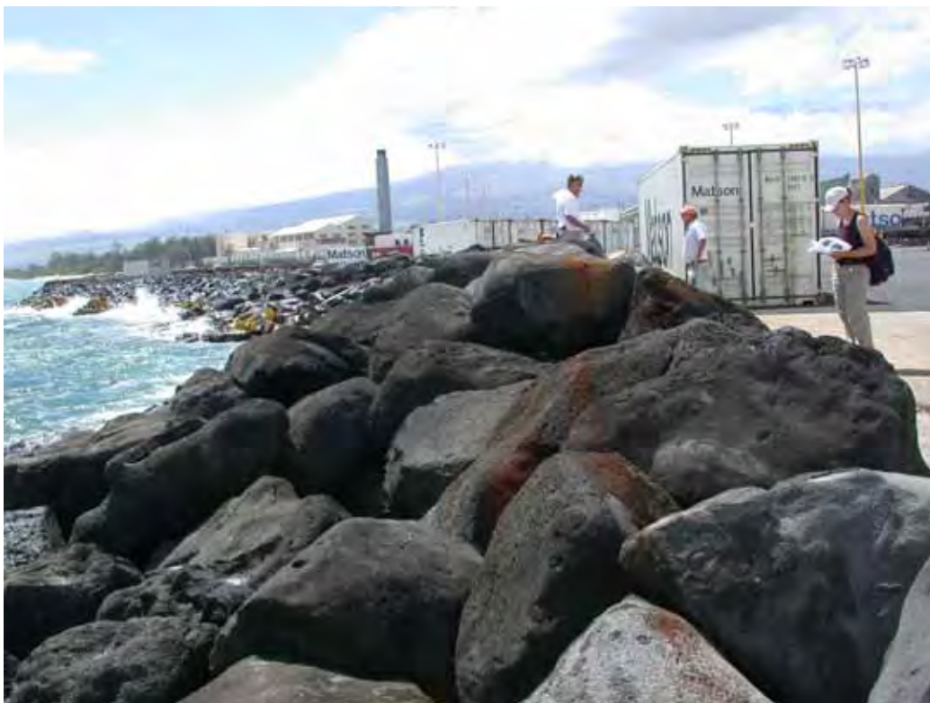
Figure B5. Damage location 10, sta 22+40, transition of repair zones, crest elevation drop, monitor side slope settling.
