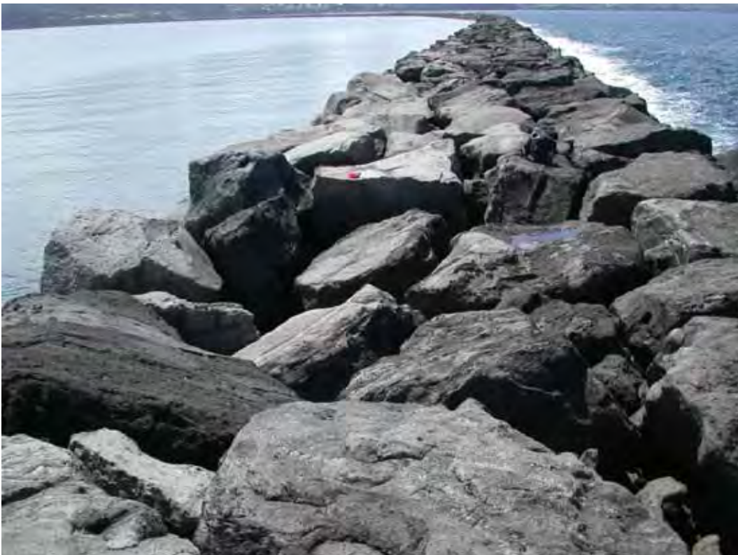
Figure A37. Damage location 39, sta 34+40, ocean side, settled hinge stone, void at crest.
