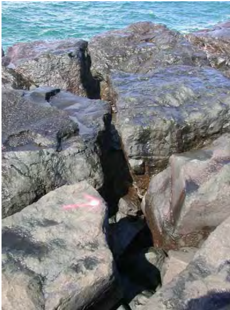
Figure A50. Damage location 54, sta 56+10, ocean side, void at crest.
