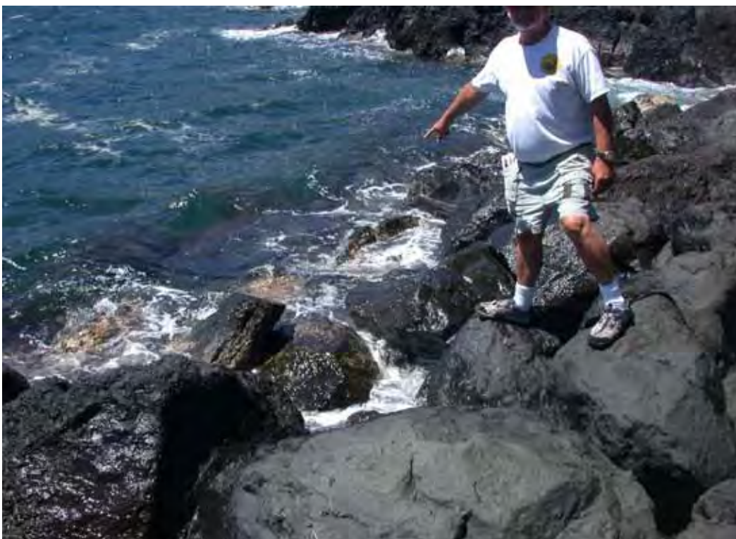
Figure C22. Displaced armor stones at wave absorber along shoreline, harbor side of breakwater.
