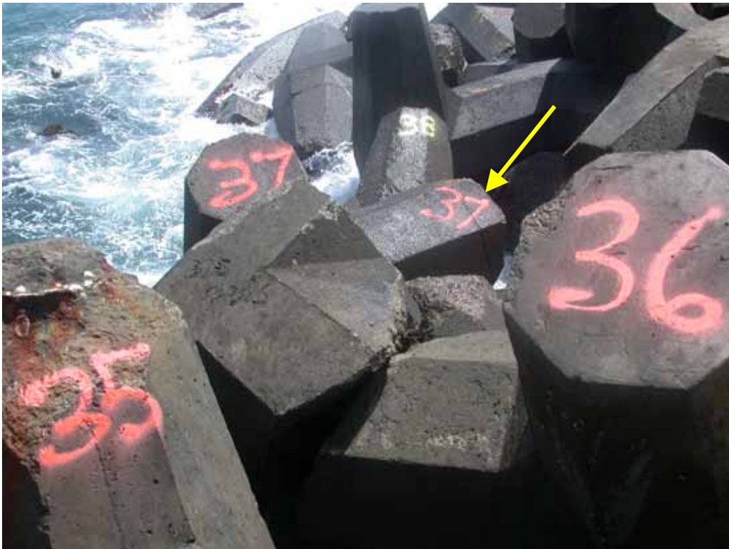
Figure B81. Damage location 50, sta 22+94, ocean side, dolosse with mid shank break.
