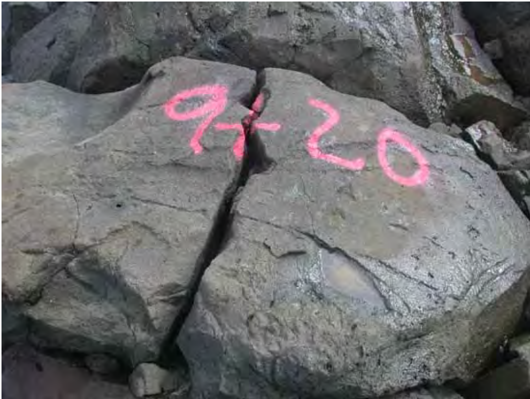
Figure 28. Typical armor stone break.
