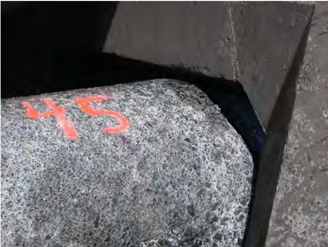
Figure B89. Damage location 59, sta 23+28, ocean side, tetrapod with missing top.
