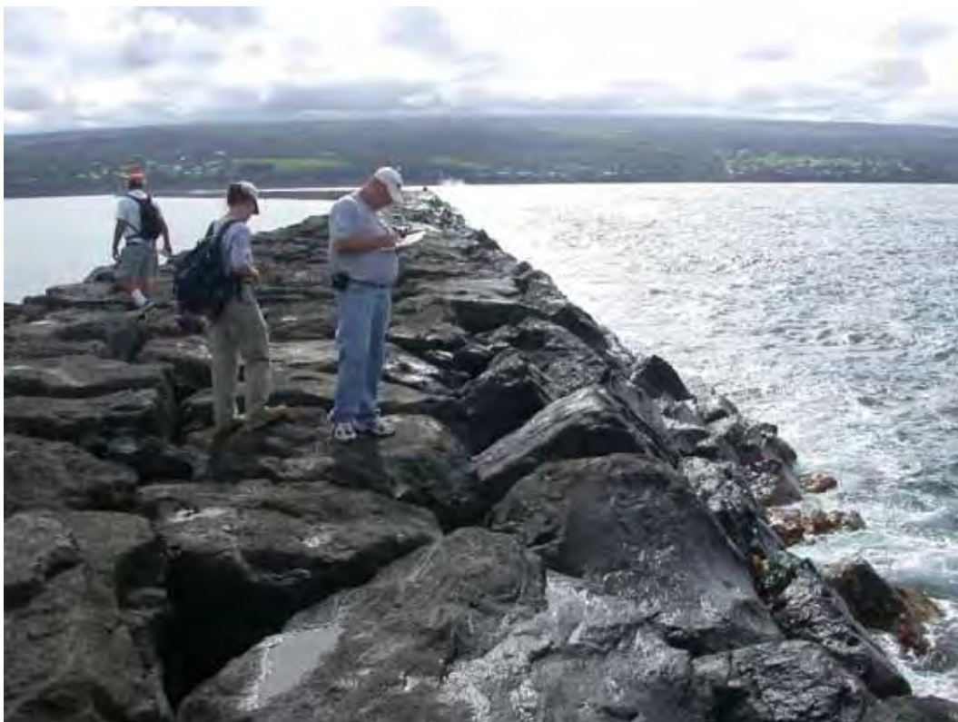
Figure A58. Damage location 62, sta 62+30 - 63+50, ocean side, hinge bowing out, bridging.
