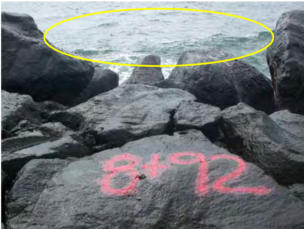
Figure D13. Damage location 12, sta 8+92, ocean side, void.
