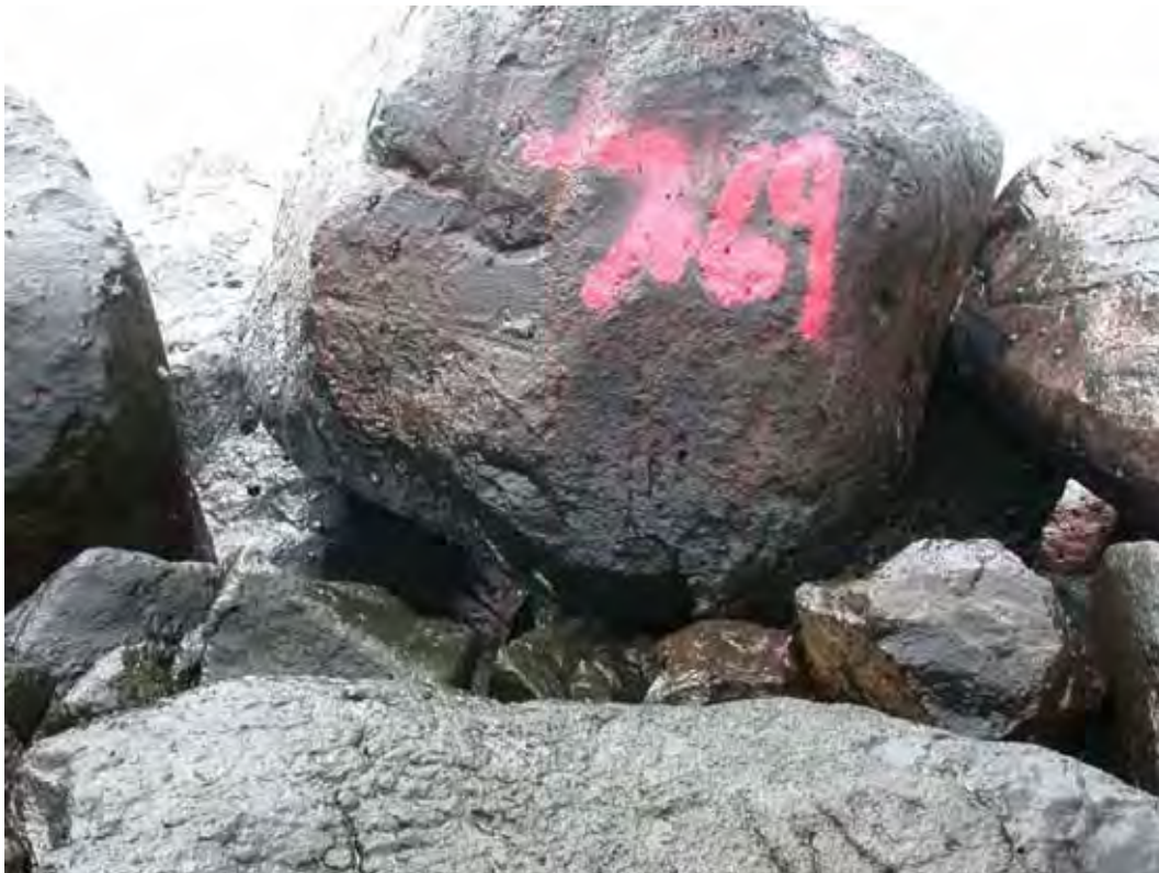
Figure D11. Damage location 10, sta 7+69, ocean side, bridging.
