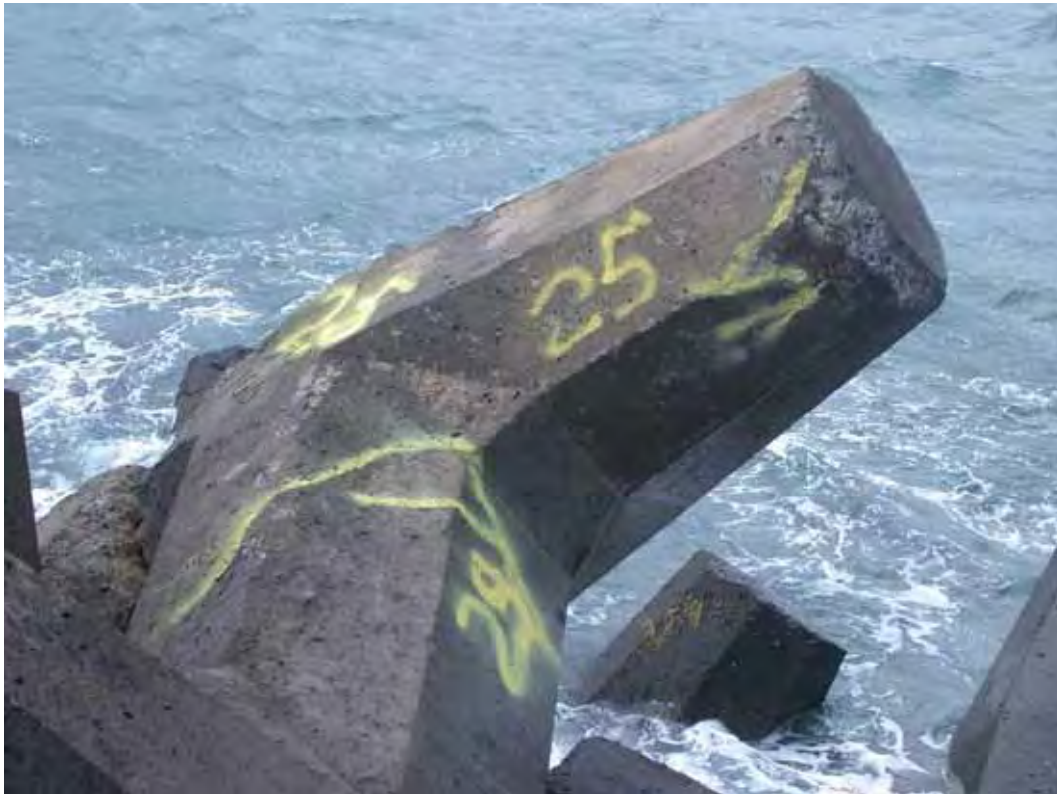
Figure B41. Damage location 56, head, 0 deg, dolosse with tip chip.
