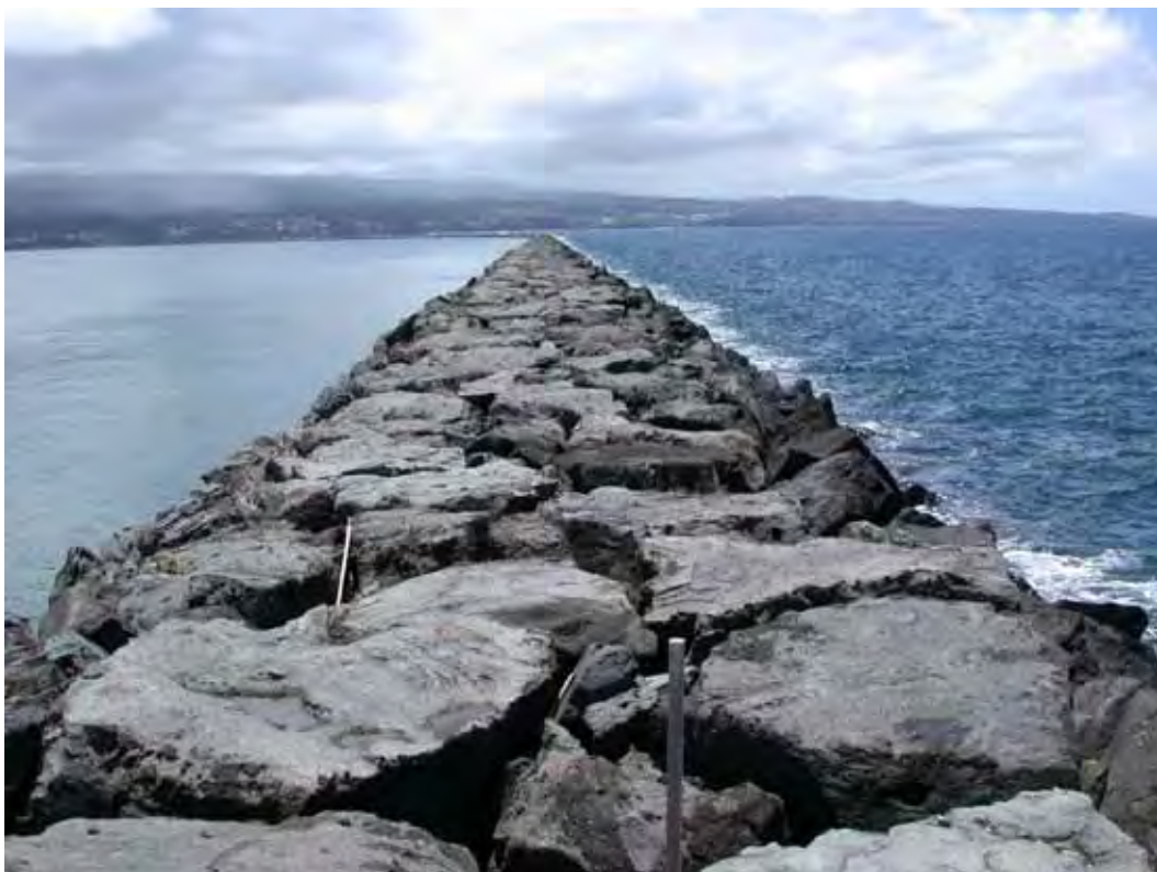
Figure A18. Sta 19+90, end of rib cap, overview looking north.
