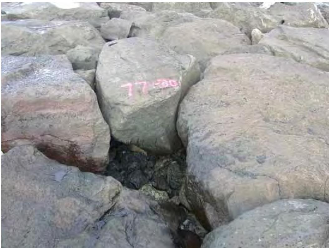
Figure A65. Damage location 76, sta 77+30, ocean side, bridging and settling.
