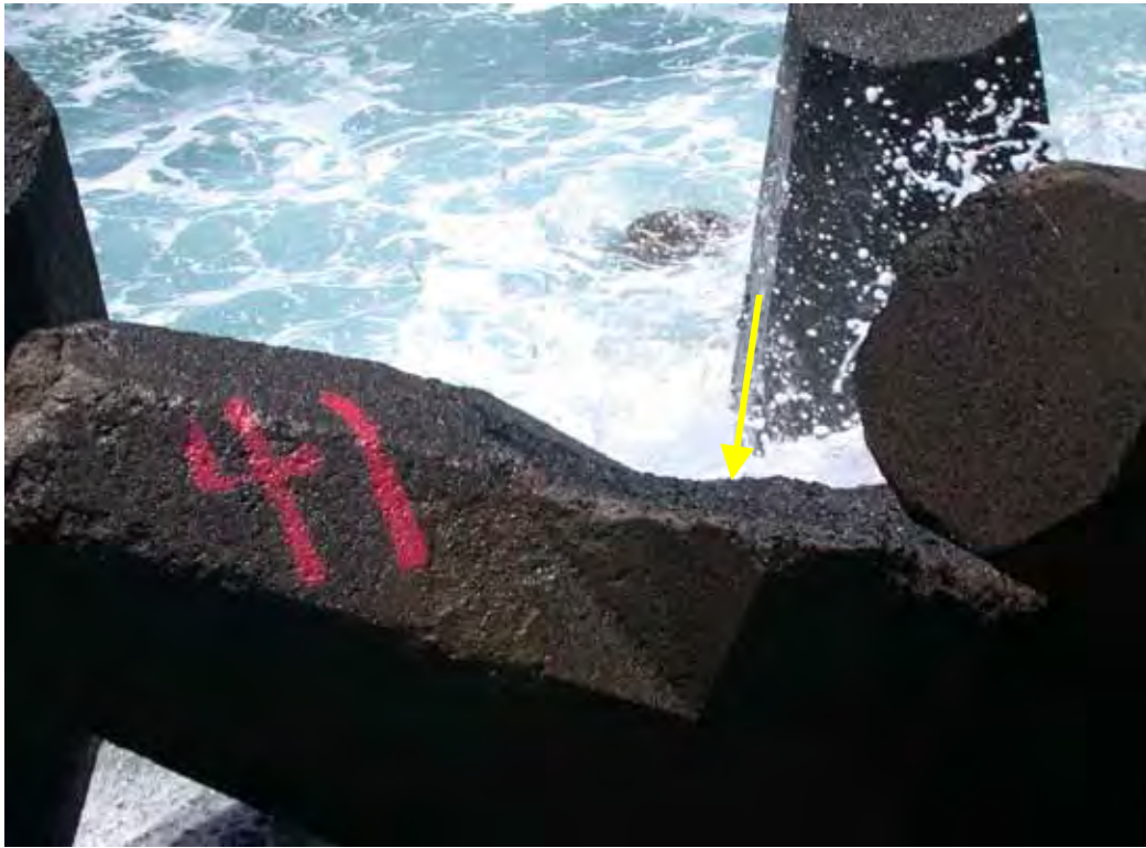
Figure D55. Damage location 73, sta 17+58, ocean side, rib #94, dolosse with shank-fluke break.
