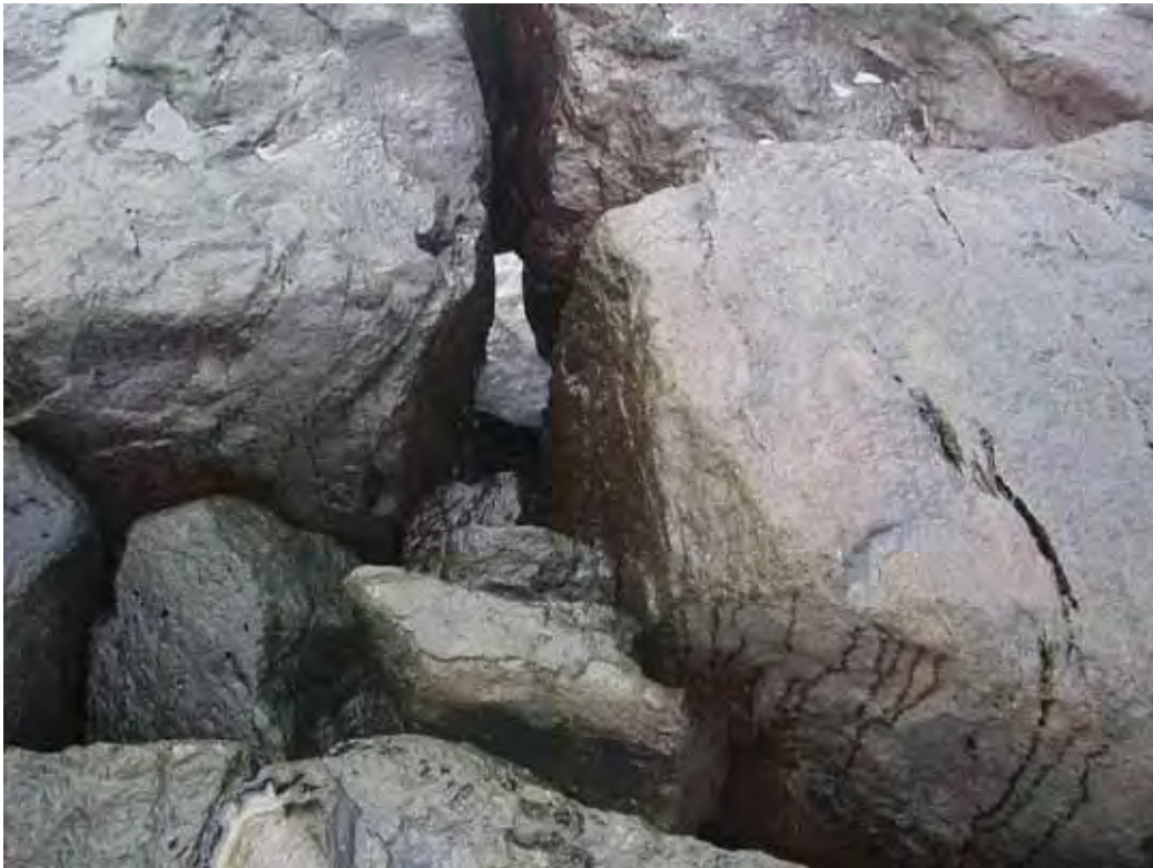
Figure A68. Damage location 81, sta 90+00, harbor side, aerial survey marker; settling at hinge; void at centerline of crest; bridging.
