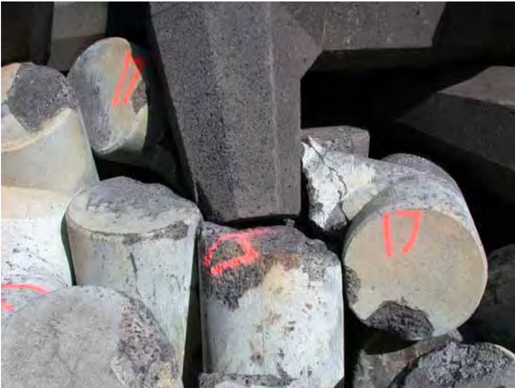
Figure B61. Damage location 24, sta 21+90, ocean side, tribar broken into three pieces.
