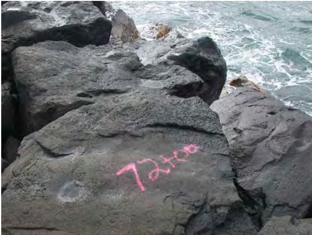
Figure A61. Damage location 70, sta 72+00, ocean side, hinge settling.
