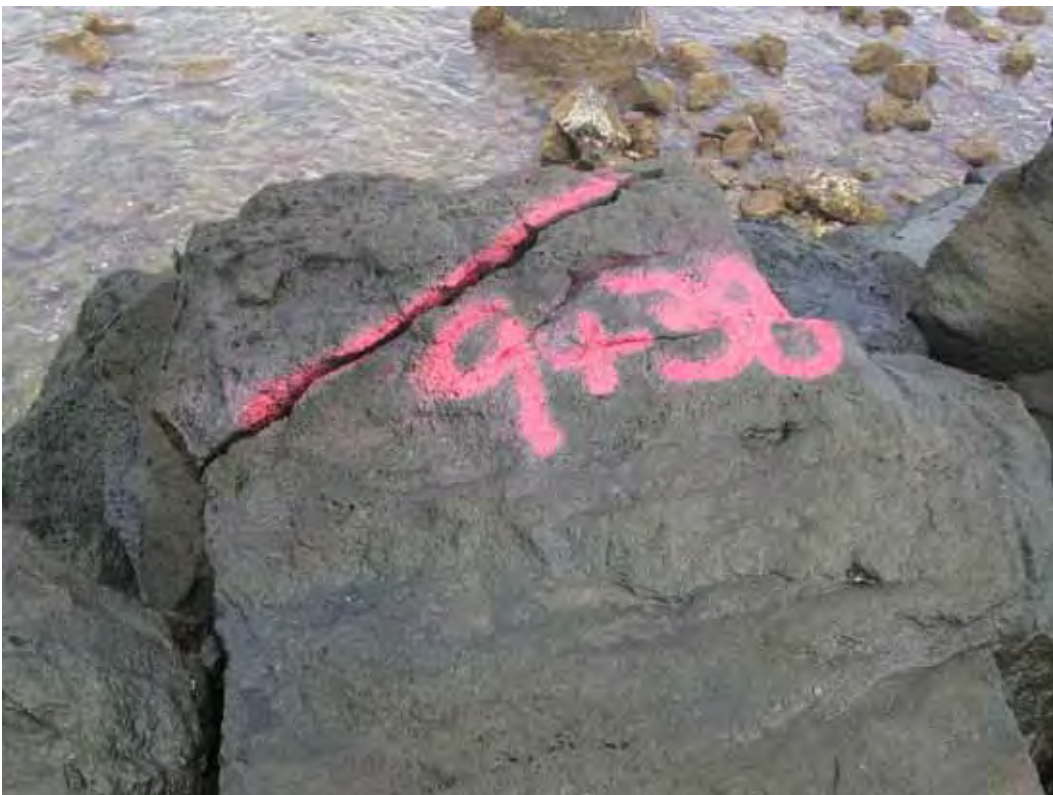
Figure D16. Damage location 15, sta 9+38, harbor side, cracked armor stone at hinge.
