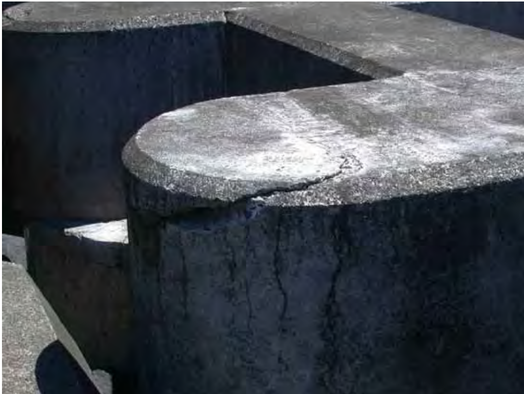
Figure C15. Rib #9, cracked.
