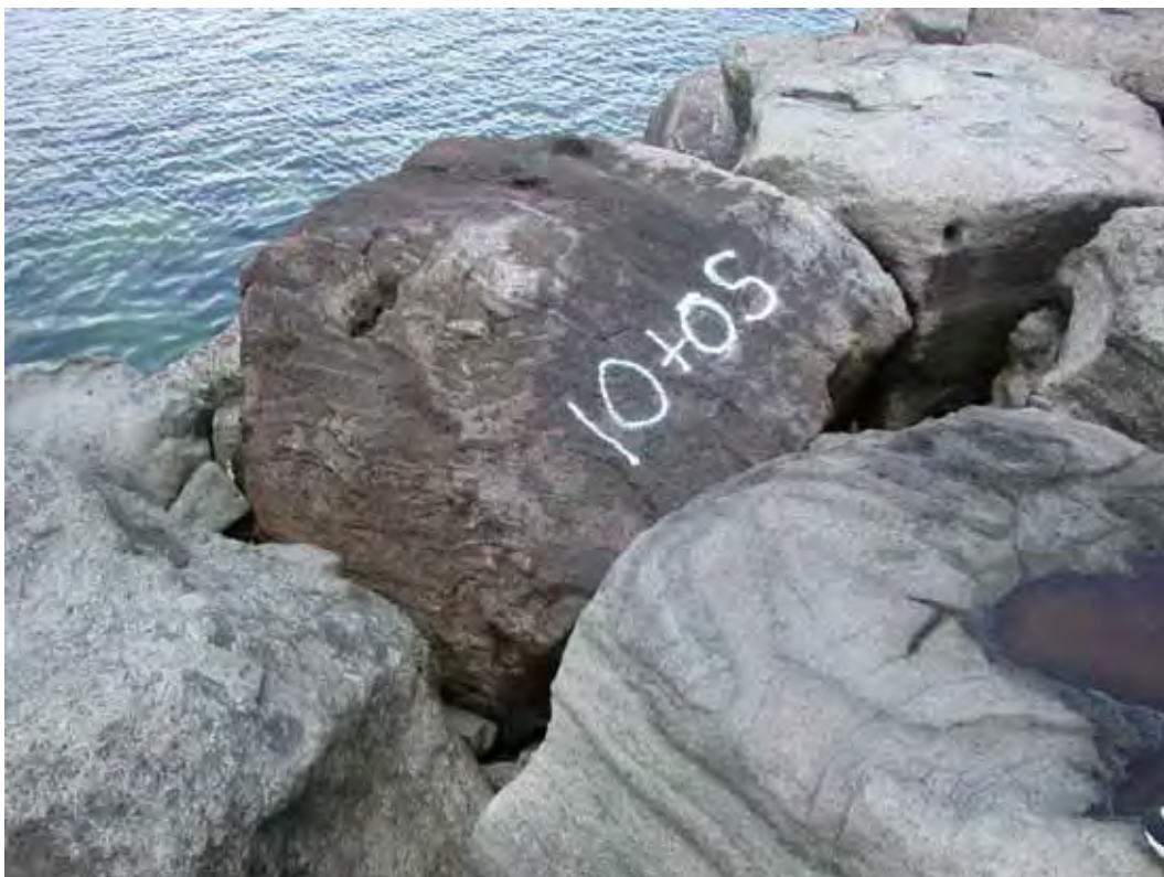
Figure A6. Damage location 5, sta 10+05, harbor side, void.
