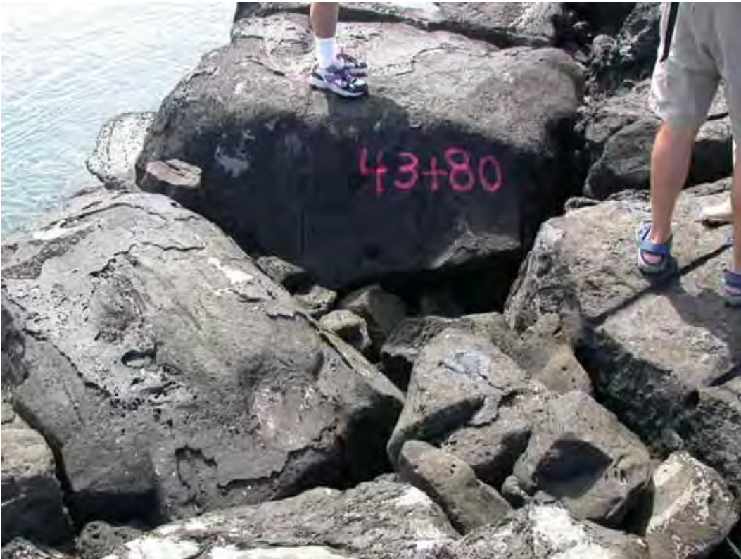
Figure A44. Damage location 46, sta 43+80, harbor side, void at crest (4 ft x 3 ft x 4 ft).
