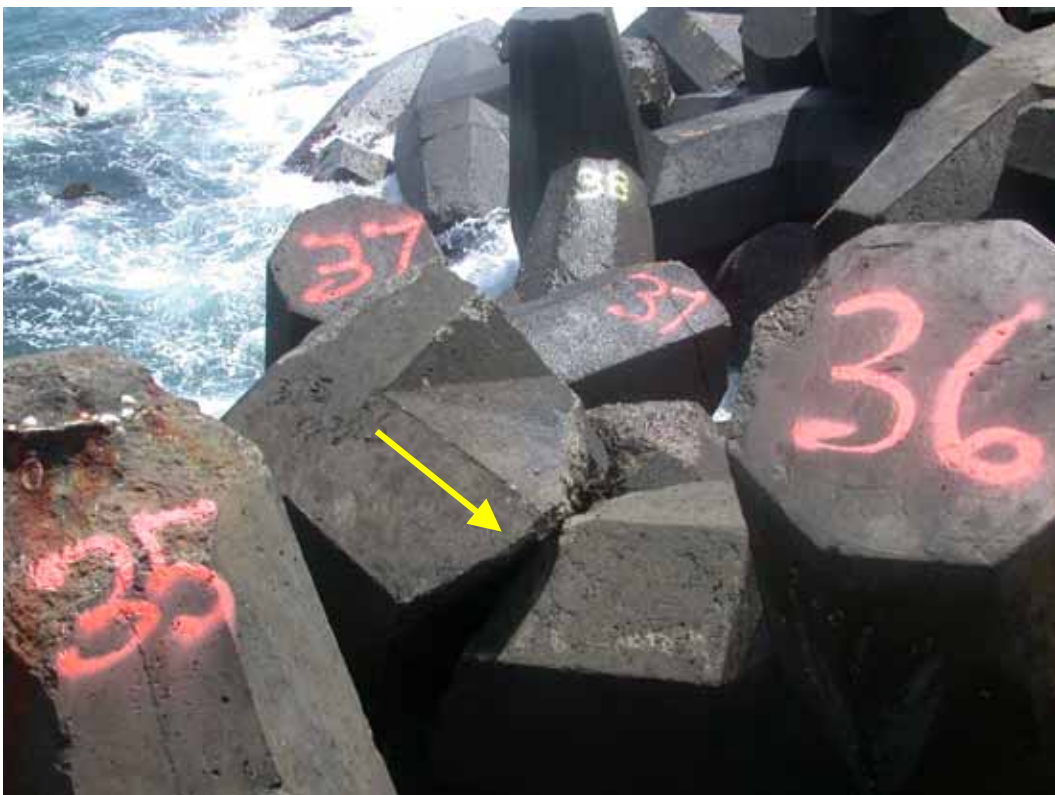
Figure B78. Damage location 47, sta 22+89, ocean side, dolosse with mid shank break.
