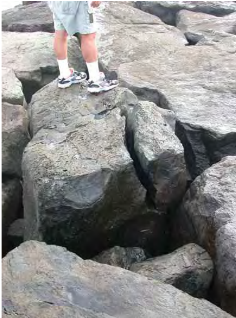
Figure A63. Damage location 72, sta 74+40, broken armor stones and bridging at crest.
