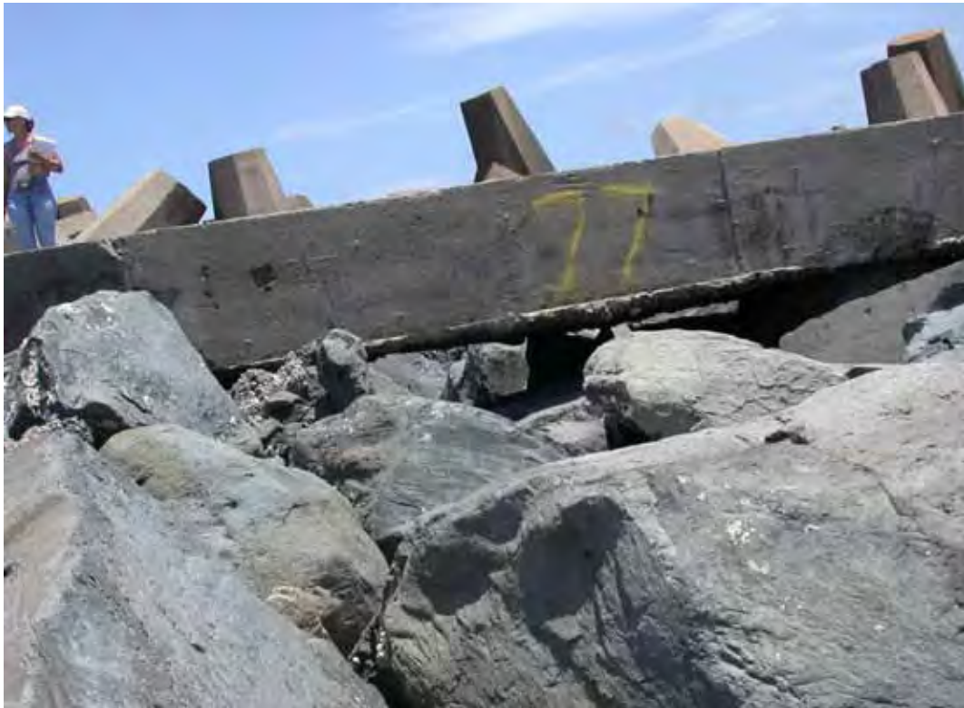
Figure B73. Damage location 38, sta 22+50, harbor side, center of turnaround, settling and unsupported rib cap.
