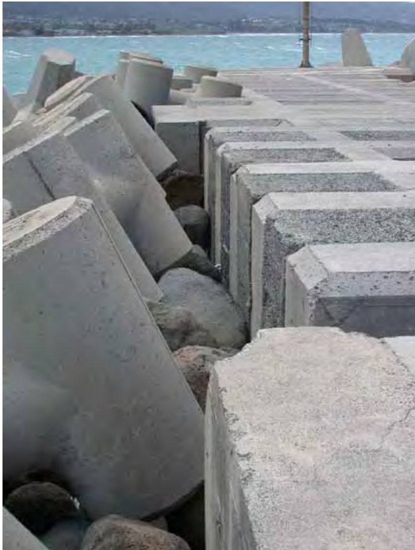
Figure B36. Damage location 48, sta 33+40 – 33+64, harbor side, rib #119 - 123, settling of tribar and separation from rib cap.
