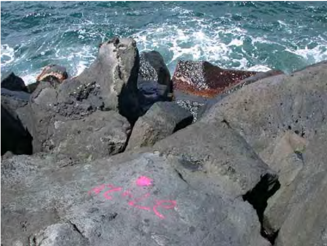
Figure A30. Damage location 30, sta 27+28, ocean side, hinge stone settling.
