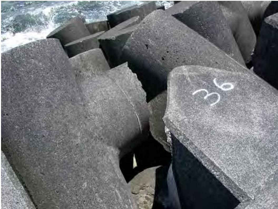
Figure A11. Damage location 13, sta 13+10, ocean side, rib #36, tribar with broken leg.
