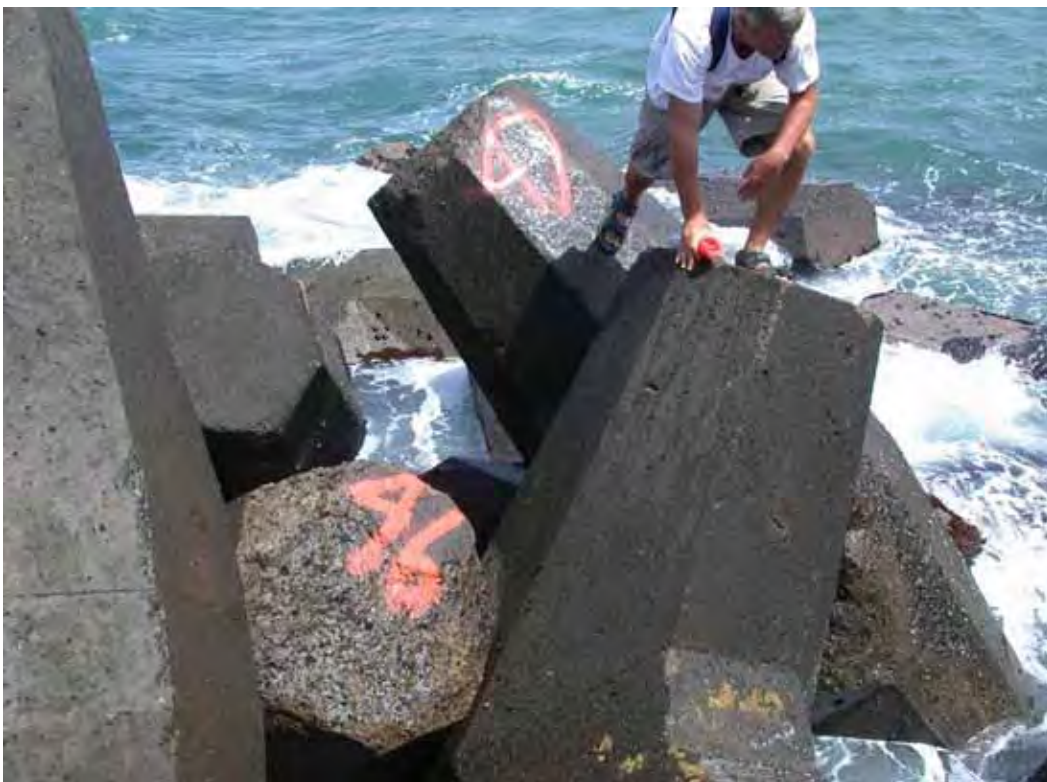
Figure B90. Damage locations 60 & 61, sta 23+30, ocean side, dolosse with mid-shank break and dolosse with shank-fluke break.
