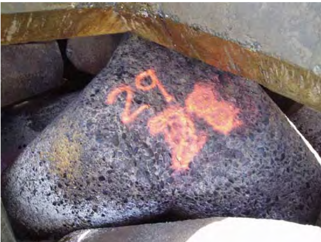
Figure B72. Damage location 37, sta 22+49, ocean side, tetrapod with broken top.
