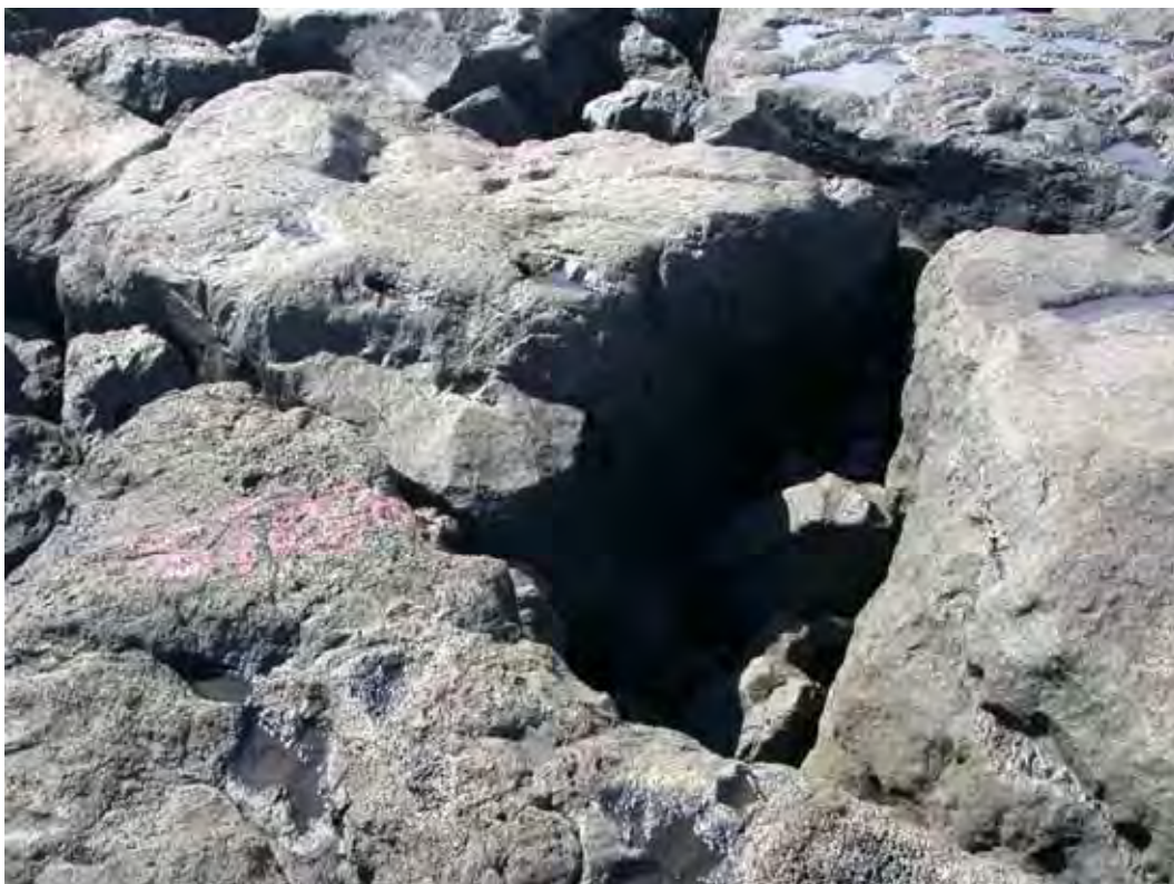
Figure A52. Damage location 56, sta 57+58, void at crest (2 ft x 4 ft x 3 ft).
