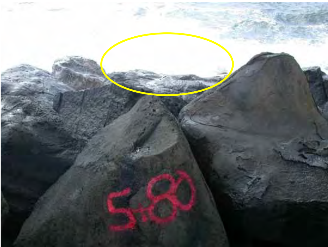
Figure D4. Damage location 3, sta 5+80, ocean side, void at toe.
