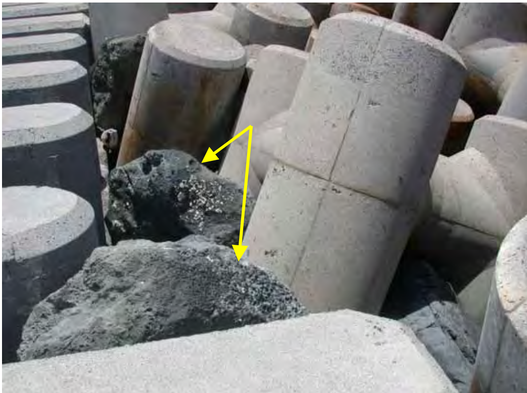
Figure B35. Damage location 46, sta 32+80 - 33+04, ocean side, rib #109 - 113, stones tossed up between ribs and tribars.
