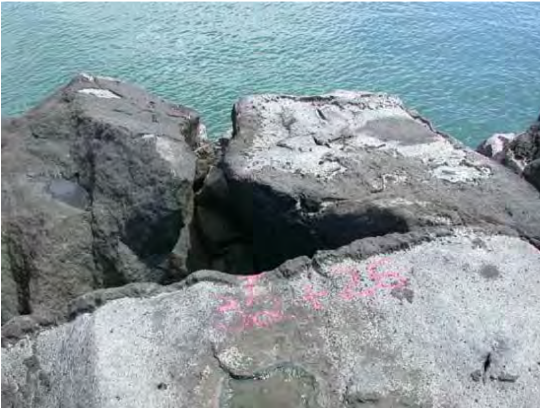
Figure A34. Damage location 36, sta 32+25, harbor side, void on edge of crest.
