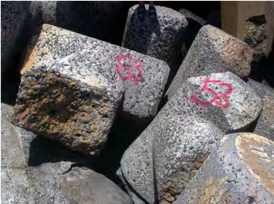
Figure D64. Damage location 85, sta 19+20, ocean side, rib #121, tribar broken through center.
