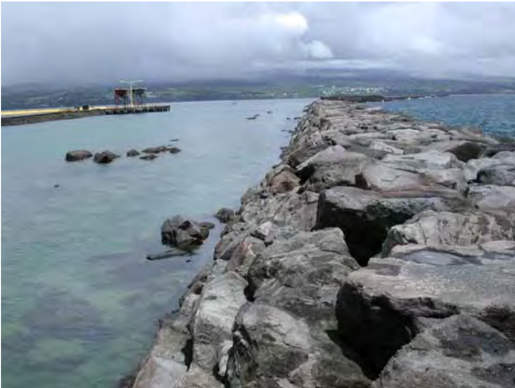
Figure A3. Damage location 2, sta 4+00, harbor side, minor settling on crest and side slope.
