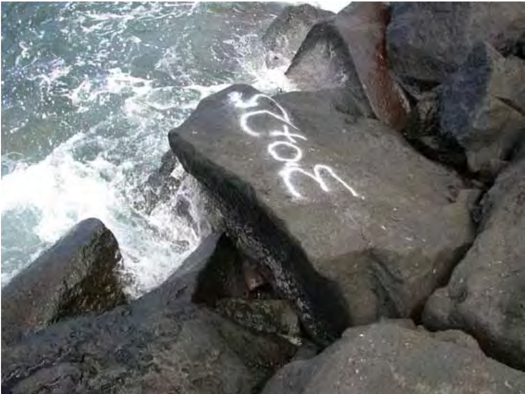
Figure A33. Damage location 35, sta 30+25, ocean side, overhanging hinge stone.
