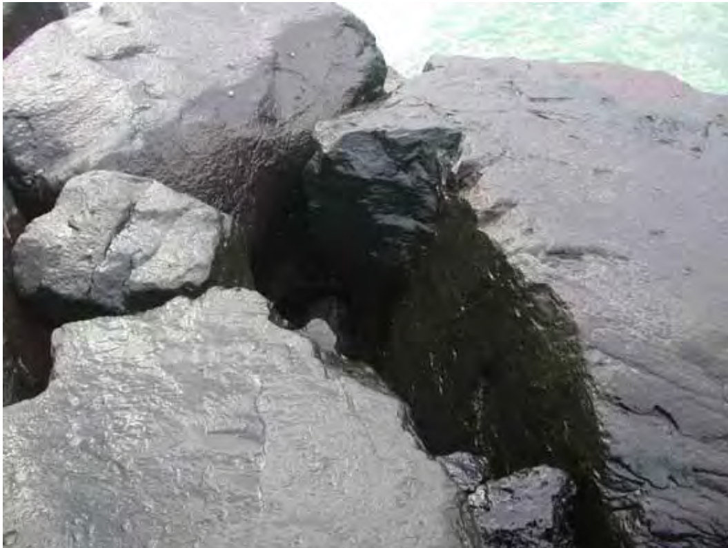
Figure A70. Damage location 84, sta 94+10, ocean side, void and bridging.
