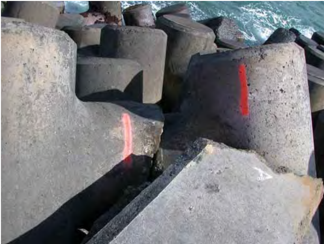
Figure B49. Damage location 6, sta 19+14, ocean side, rib #18, tribar with break through center and 4" separation from rib cap.
