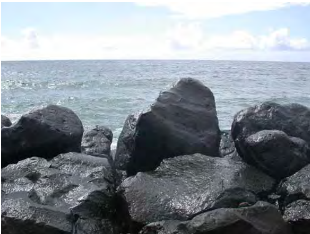
Figure 29. Example of perched armor stones.
