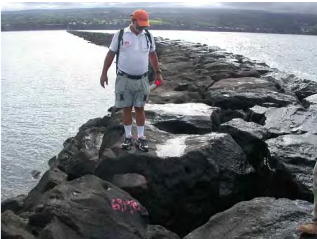
Figure A60. Damage location 68, sta 69+98, harbor side, void at crest (3 ft x 6 ft x 10 ft).
