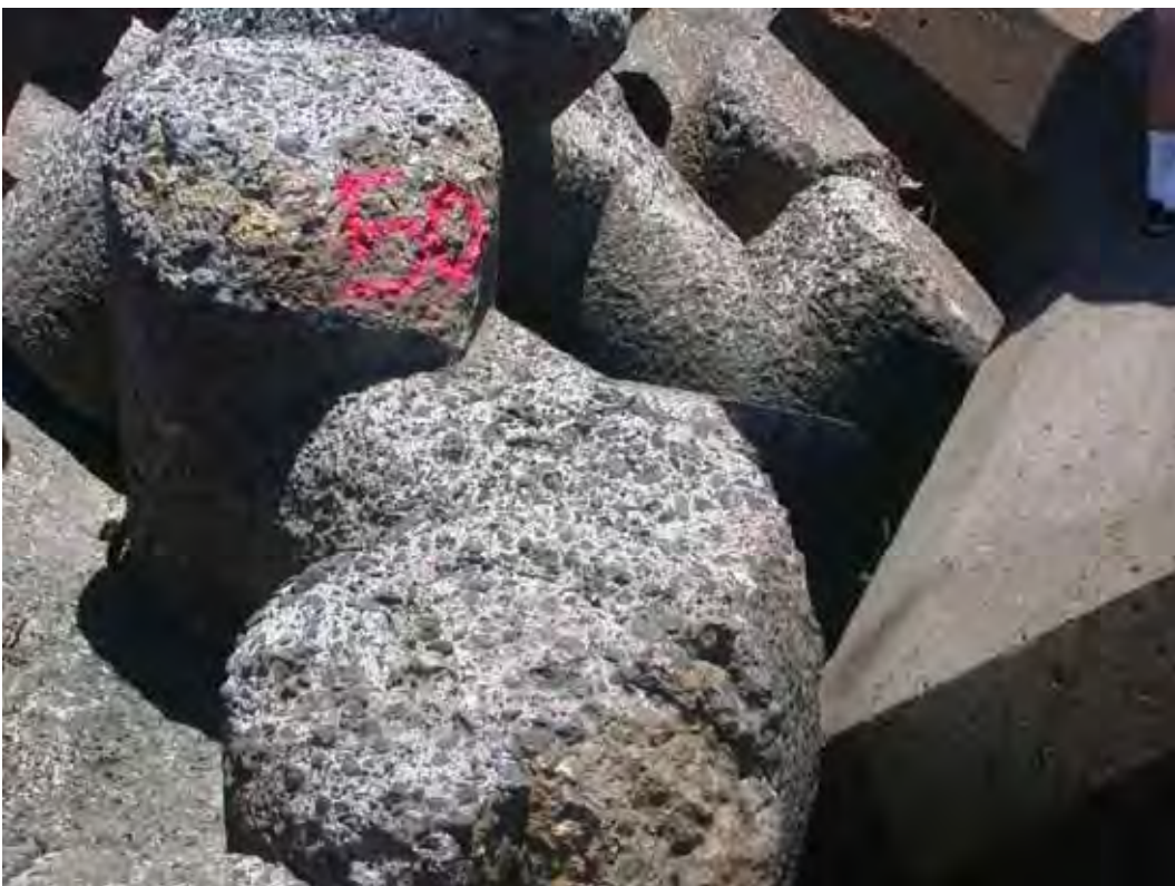
Figure D61. Damage location 82, sta 18+84, ocean side, rib #115, tribar with broken can.
