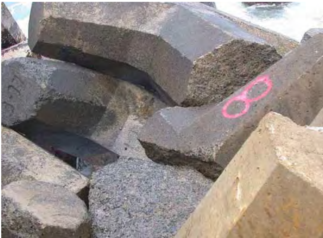
Figure D33. Damage location 38, sta 13+44 – 13+50, ocean side, rib #25 & 26, dolosse with mid-shank and fluke-shank breaks.
