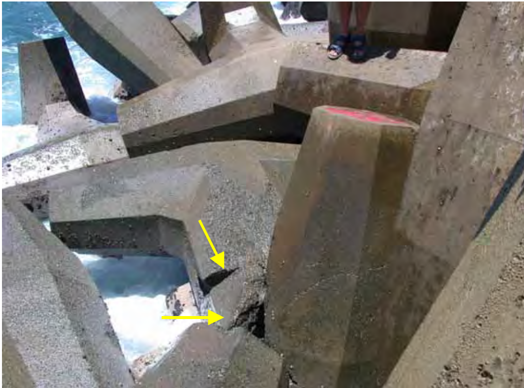
Figure D68. Damage location 91, sta 19+66, ocean side, rib #127, dolosse with multiple breaks.
