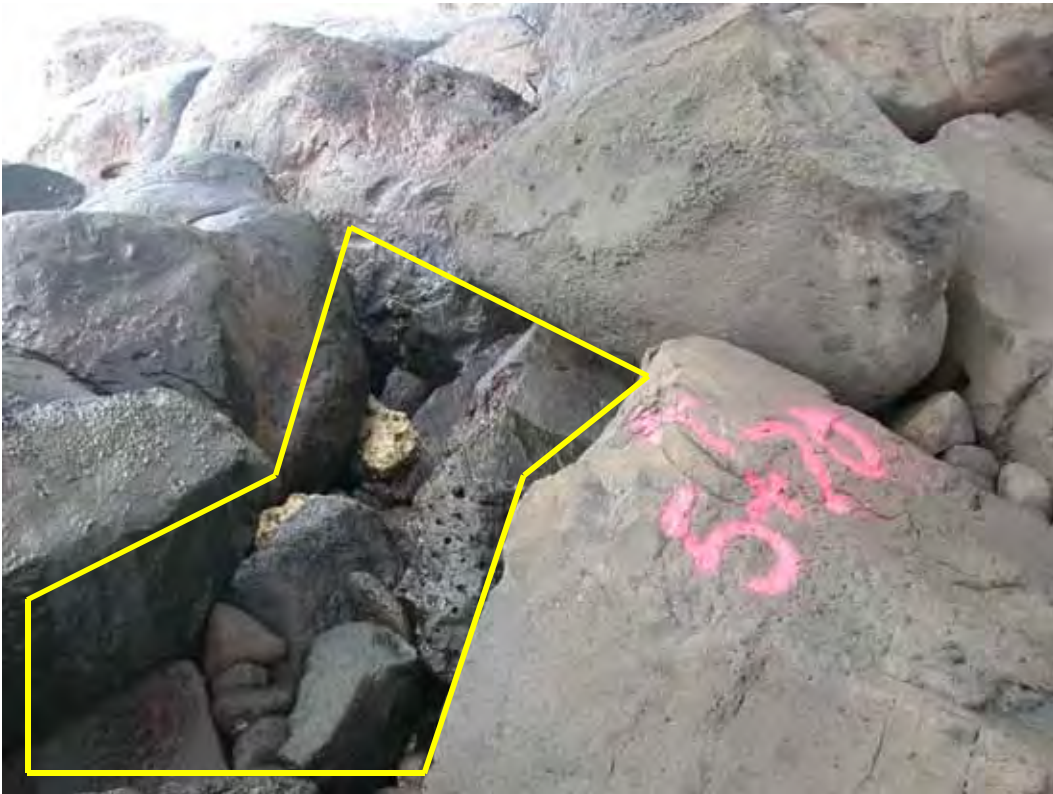
Figure D3. Damage location 2, sta 5+70, ocean side, void at hinge.
