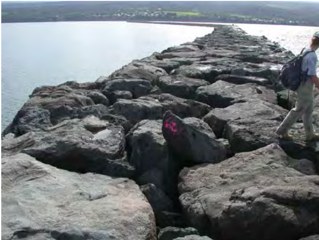
Figure A57. Damage location 61, sta 62+00, perched stone.
