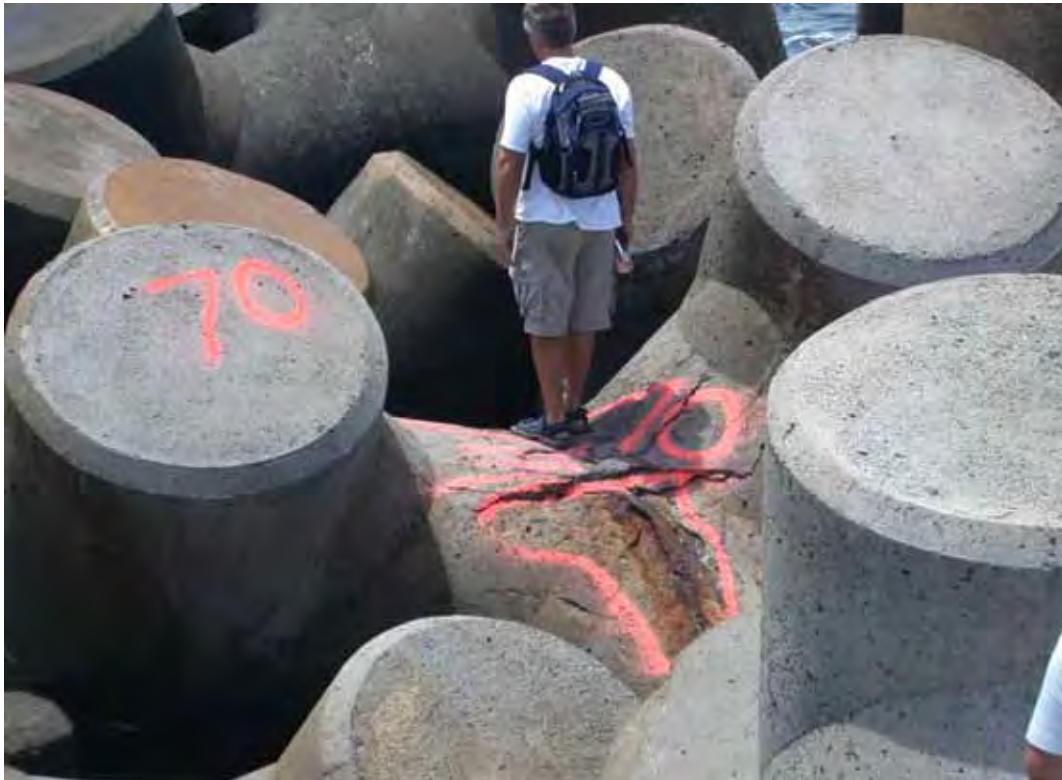
Figure B99. Damage location 84, 90 deg harbor side of head, tribar with exposed and rusted rebar at center.
