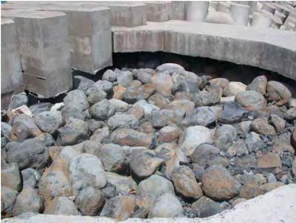
Figure B25. Damage location 31, sta 29+27, harbor side, rib #50, Centerline of first turnaround; settling of armor stone - unsupported rib cap.
