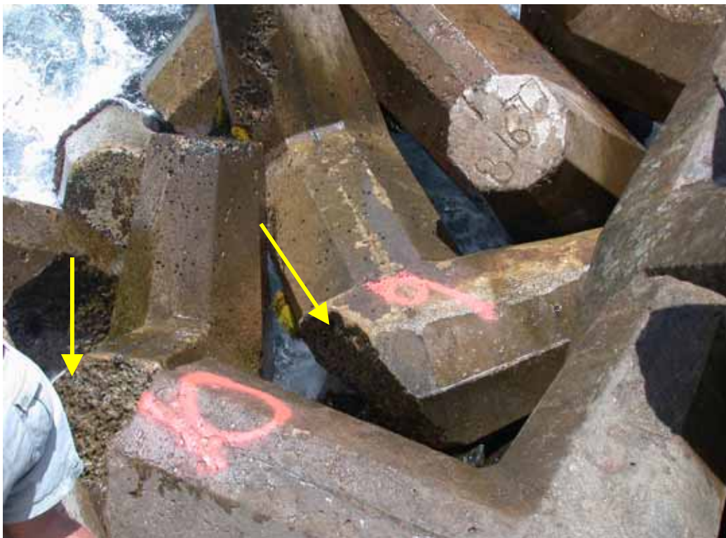
Figure B19. Damage locations 23 & 24, sta 27+69, ocean side, rib #23, dolosse with fluke-shank break and dolosse with shank-fluke break.
