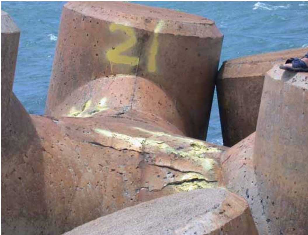
Figure B34. Damage location 45, sta 32+74, ocean side, rib #108, tribar with spalling.
