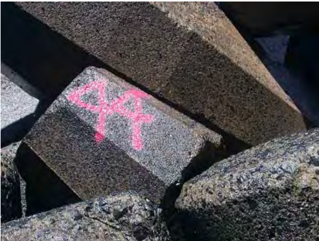
Figure D58. Damage location 76, sta 18+24, ocean side, rib #105, dolosse with fluke tip break.
