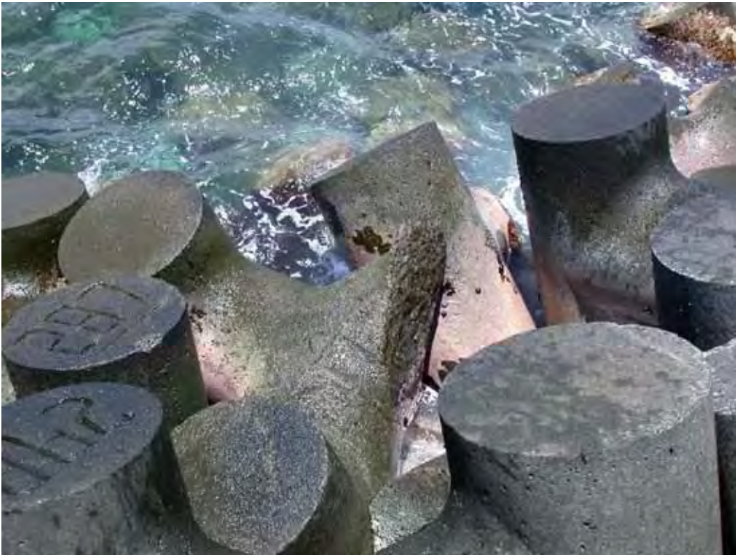
Figure A15. Damage location 16, sta 17+40, ocean side, broken tribar at waterline.
