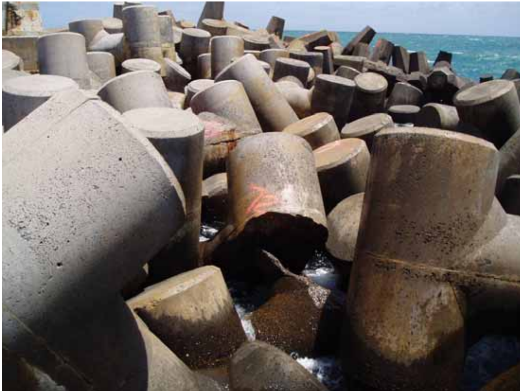
Figure B79. Damage location 48, sta 22+90, harbor side, tribar with broken can.
