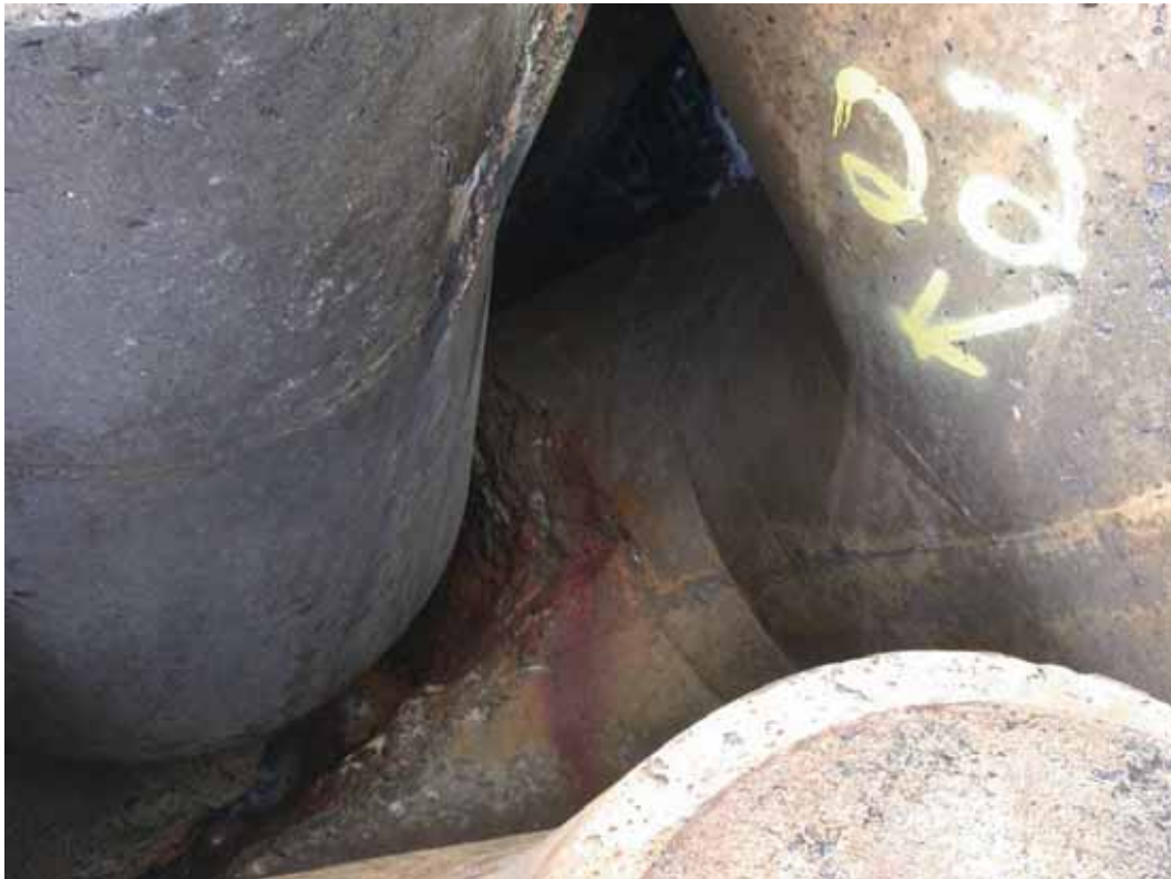
Figure B37. Damage location 50, sta 33+52, ocean side, rib #121, tribar with top of leg broken.
