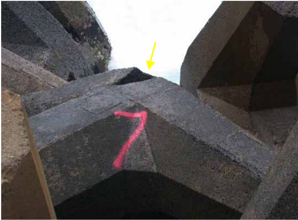
Figure D32. Damage location 37, sta 13+38 – 13+44, ocean side, rib #24 & 25, dolosse with fluke-shank break.
