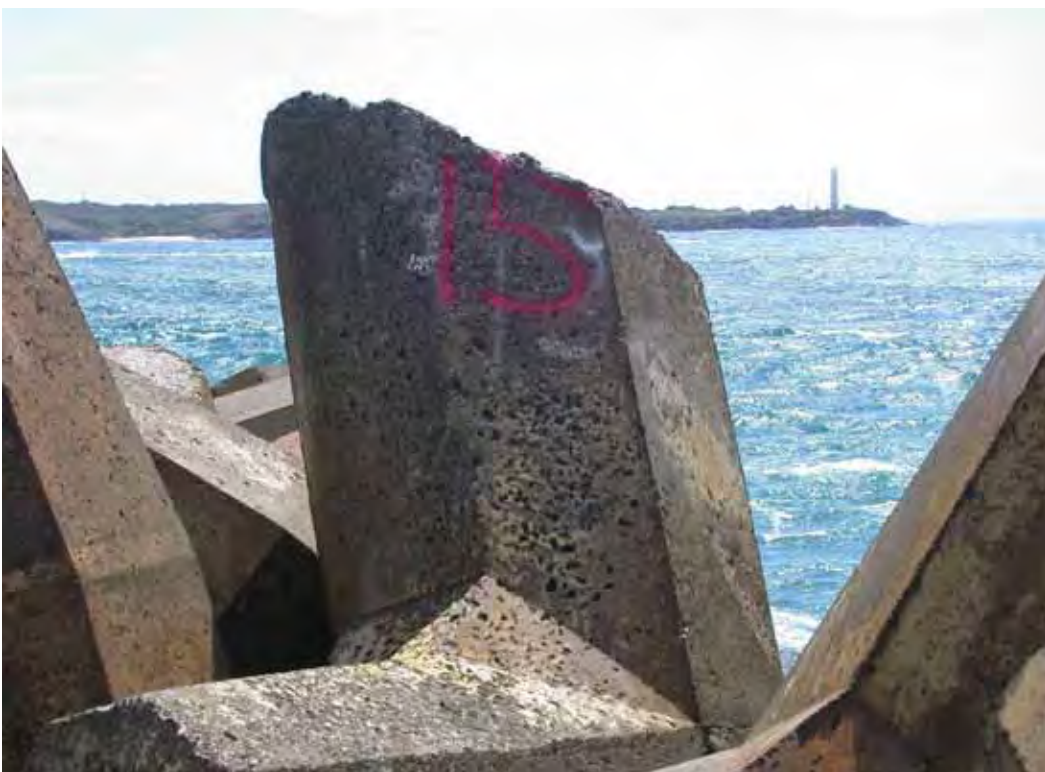
Figure D39. Damage location 45, sta 14+52, ocean side, rib #43, dolosse with shank-fluke break.
