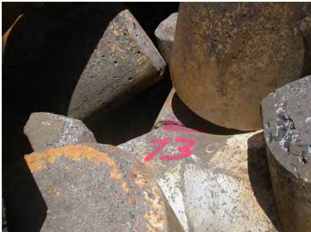
Figure D75. Damage location 106, sta 20+26, ocean side, rib #137, tribar with broken leg.
