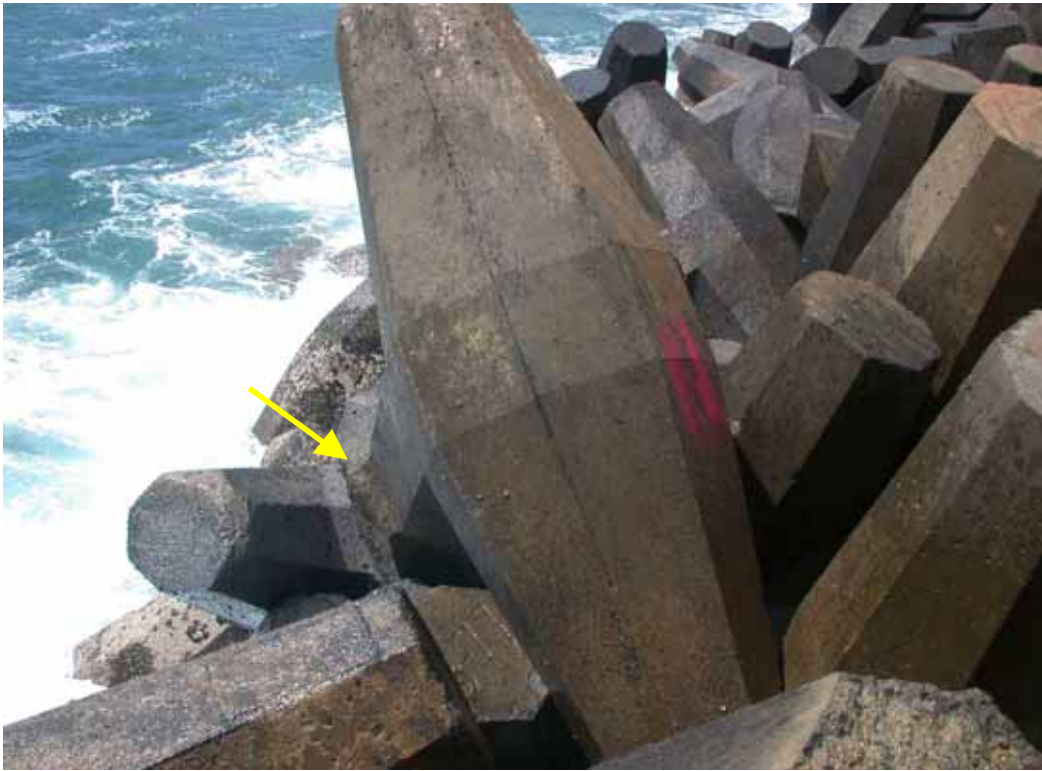
Figure D36. Damage location 41, sta 13+92 – 13+98, ocean side, rib #33 & 34, dolosse with fluke-shank break.
