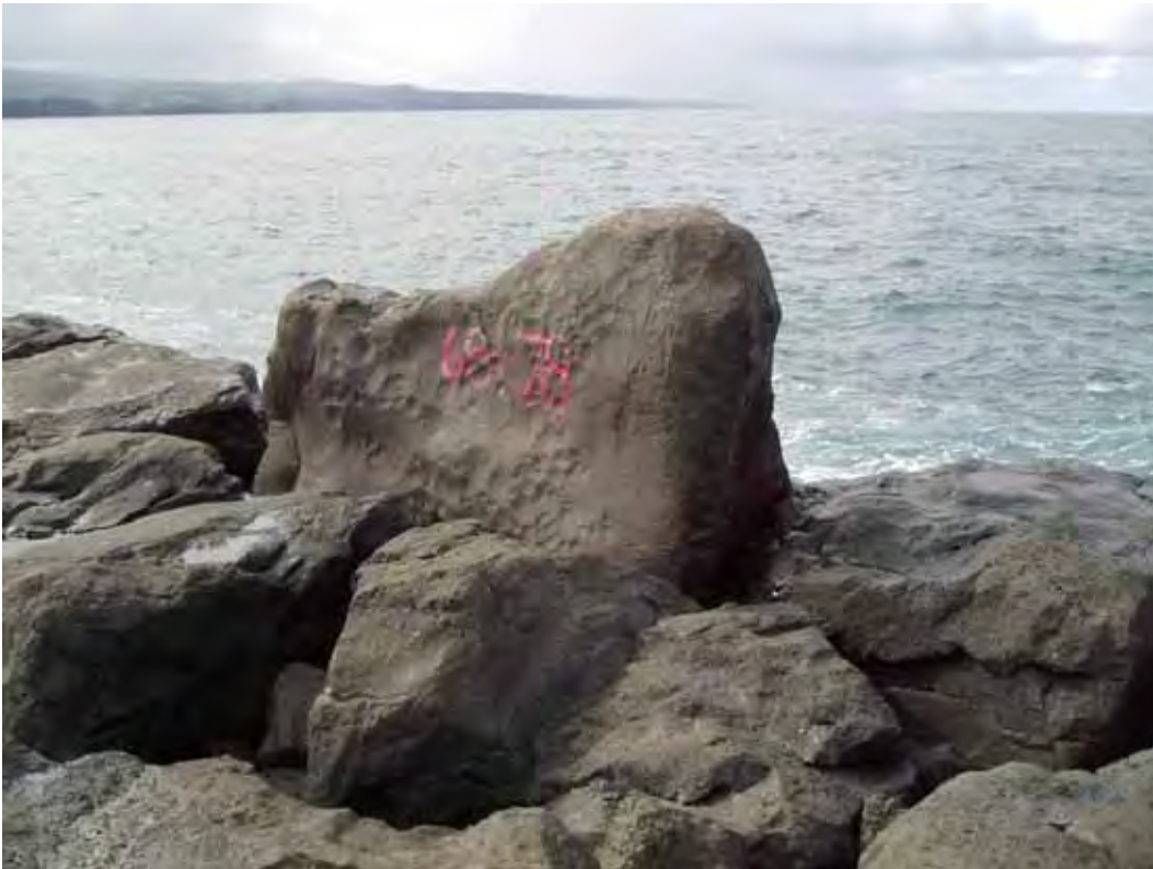
Figure A59. Damage location 67, sta 68+78, ocean side, perched armor stone "Tombstone."
