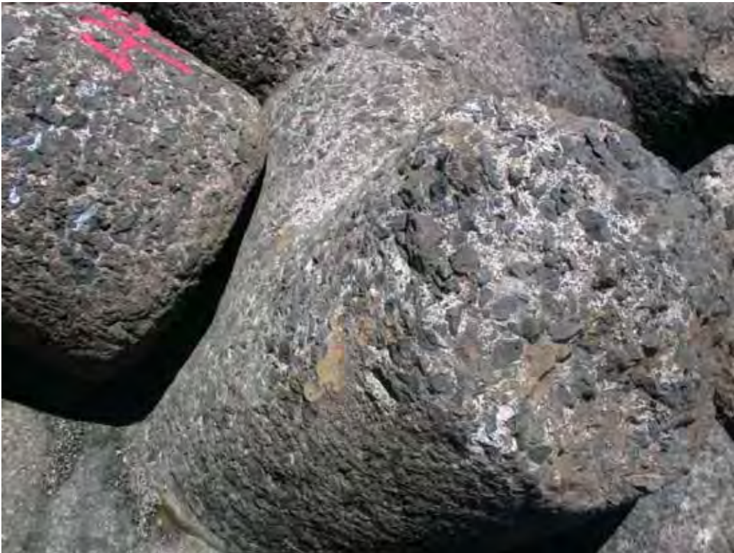
Figure D60. Damage location 81, sta 18+72, ocean side, rib #113, tribar with broken can.
