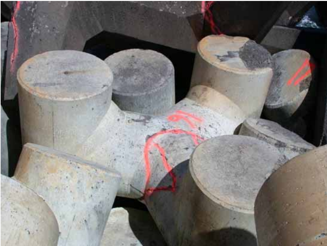
Figure B59. Damage location 21, sta 21+81, ocean side, tribar with cracks through center.
