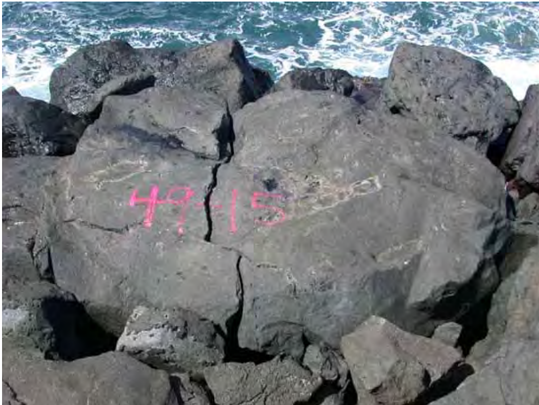
Figure A46. Damage location 49, sta 49+15, ocean side, broken stone on crest.
