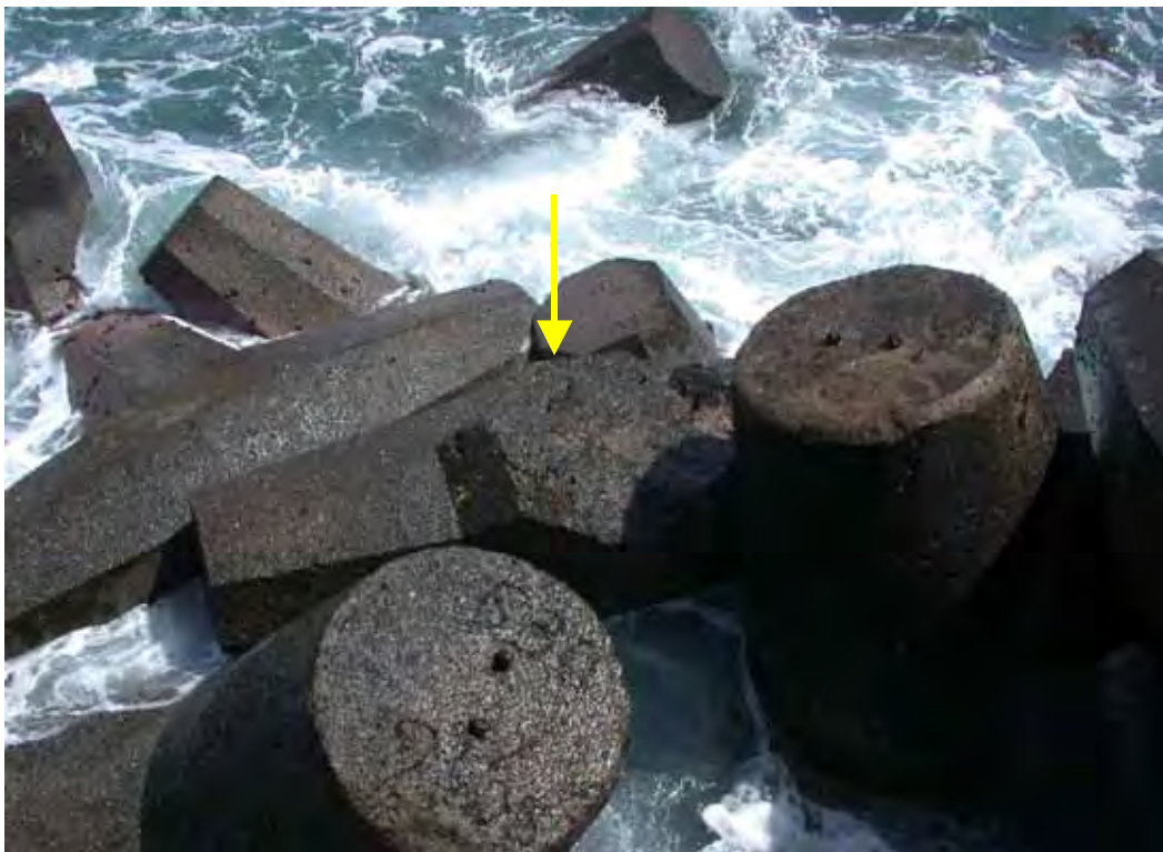
Figure B68. Damage location 31, sta 22+20, ocean side, dolosse with shank-fluke break at waterline.
