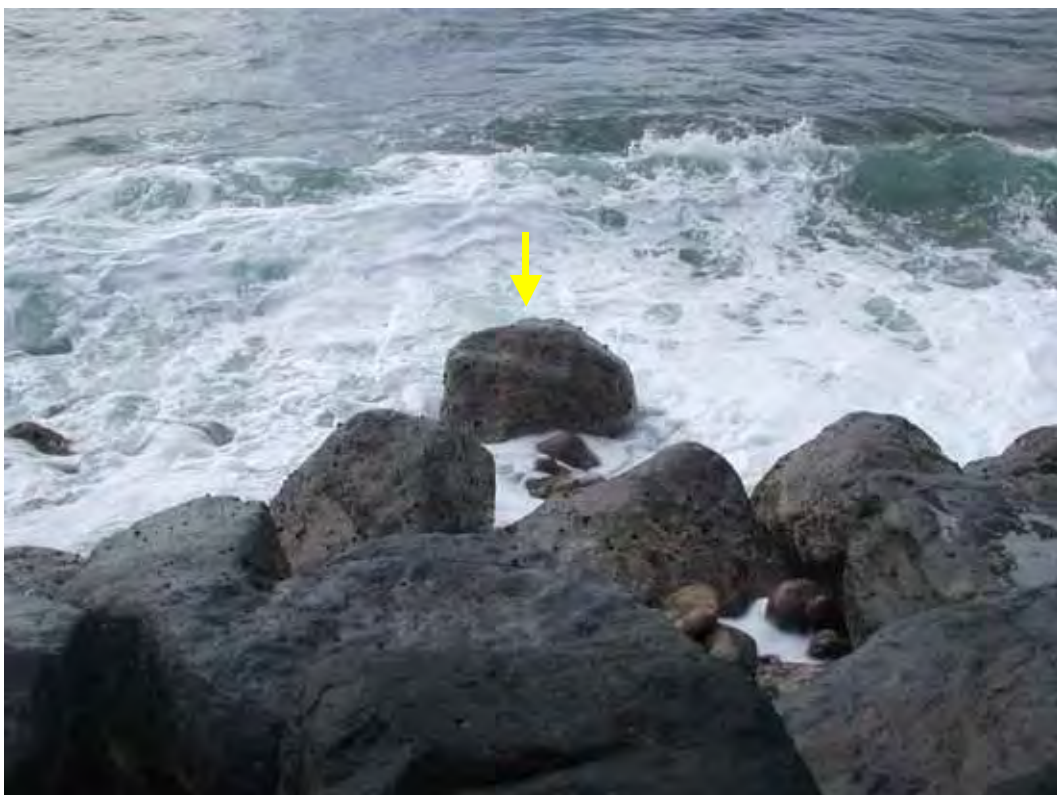
Figure D2. Damage location 1, sta 5+50, ocean side, dislodged armor stone at toe.
