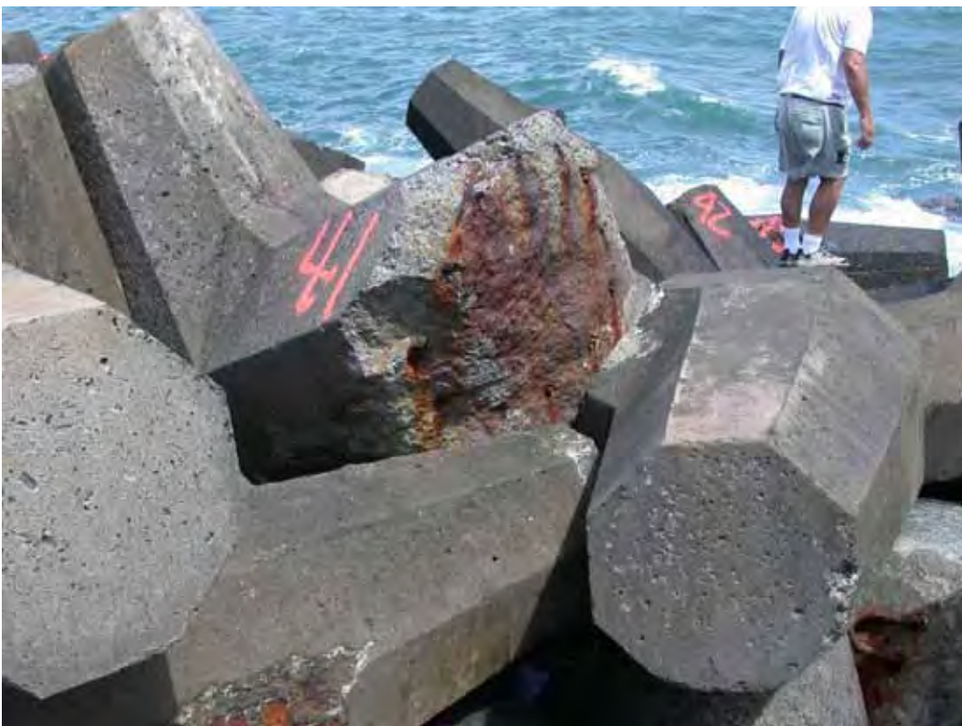
Figure B86. Damage location 55, sta 23+19, ocean side, dolosse with shank-fluke break.
