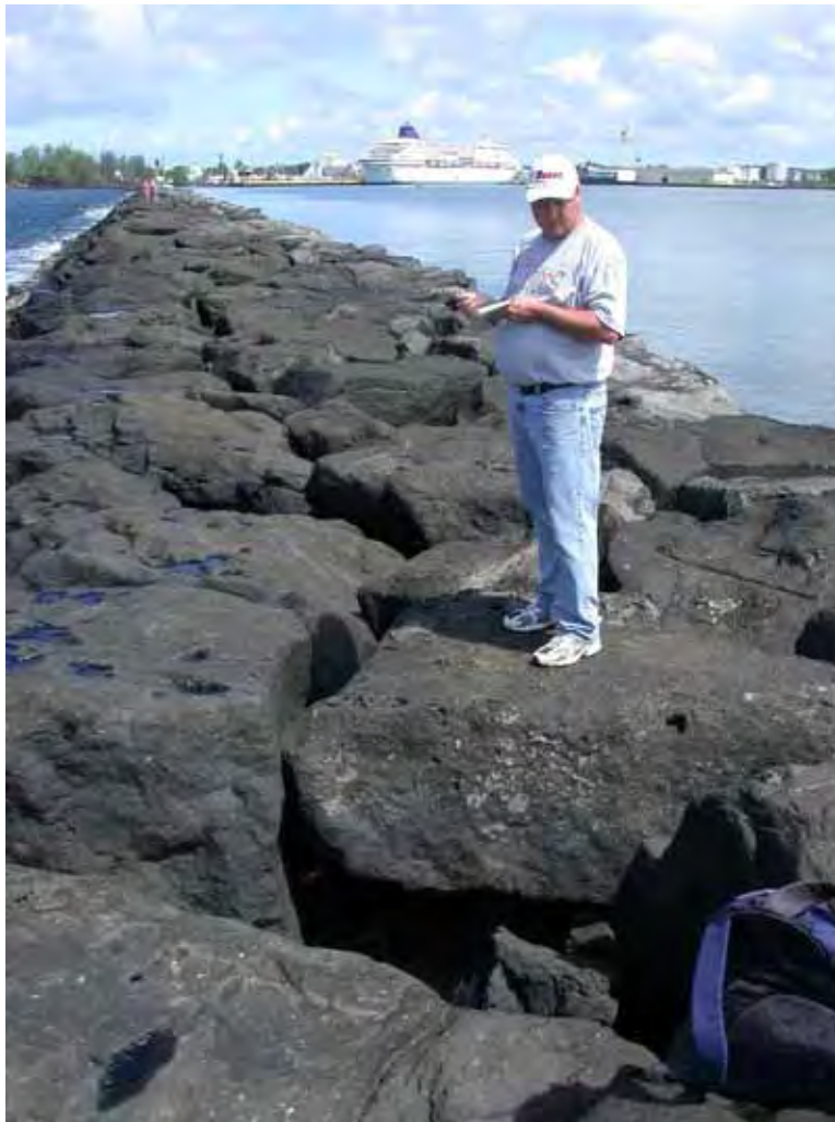
Figure A43. Damage location 45, sta 40+55, major settling and bridging from centerline to waterline; void extends to waterline but structure is not completely breached.
