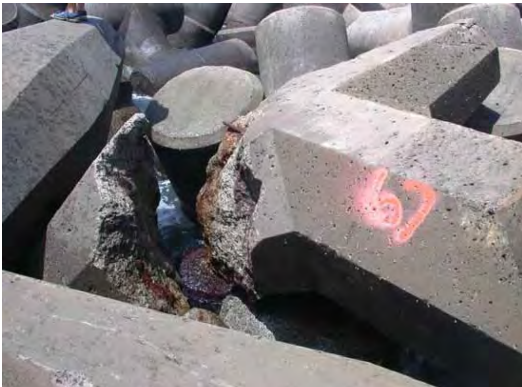
Figure B98. Damage location 81, 15 deg harbor side of head, dolosse with fluke-shank break.
