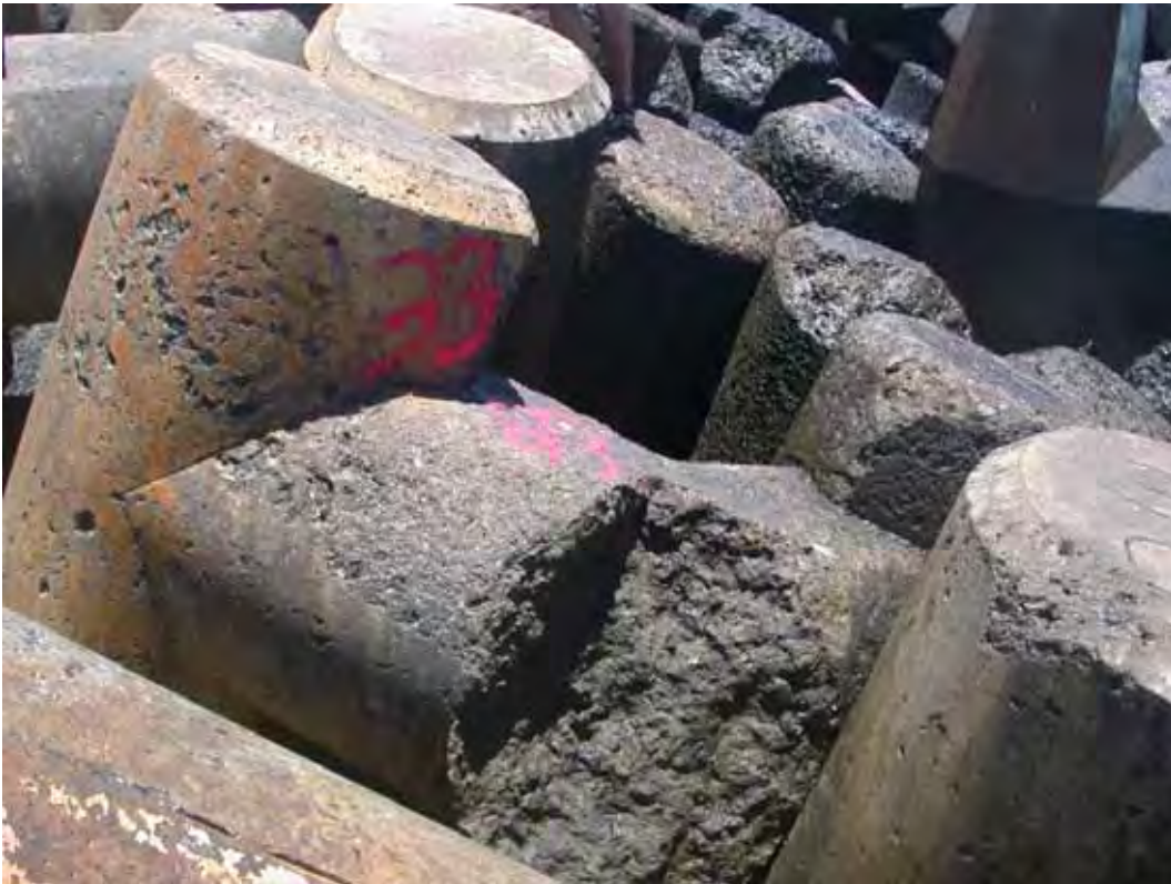
Figure D49. Damage location 65, sta 16+50, ocean side, rib #76, tribar with broken leg.
