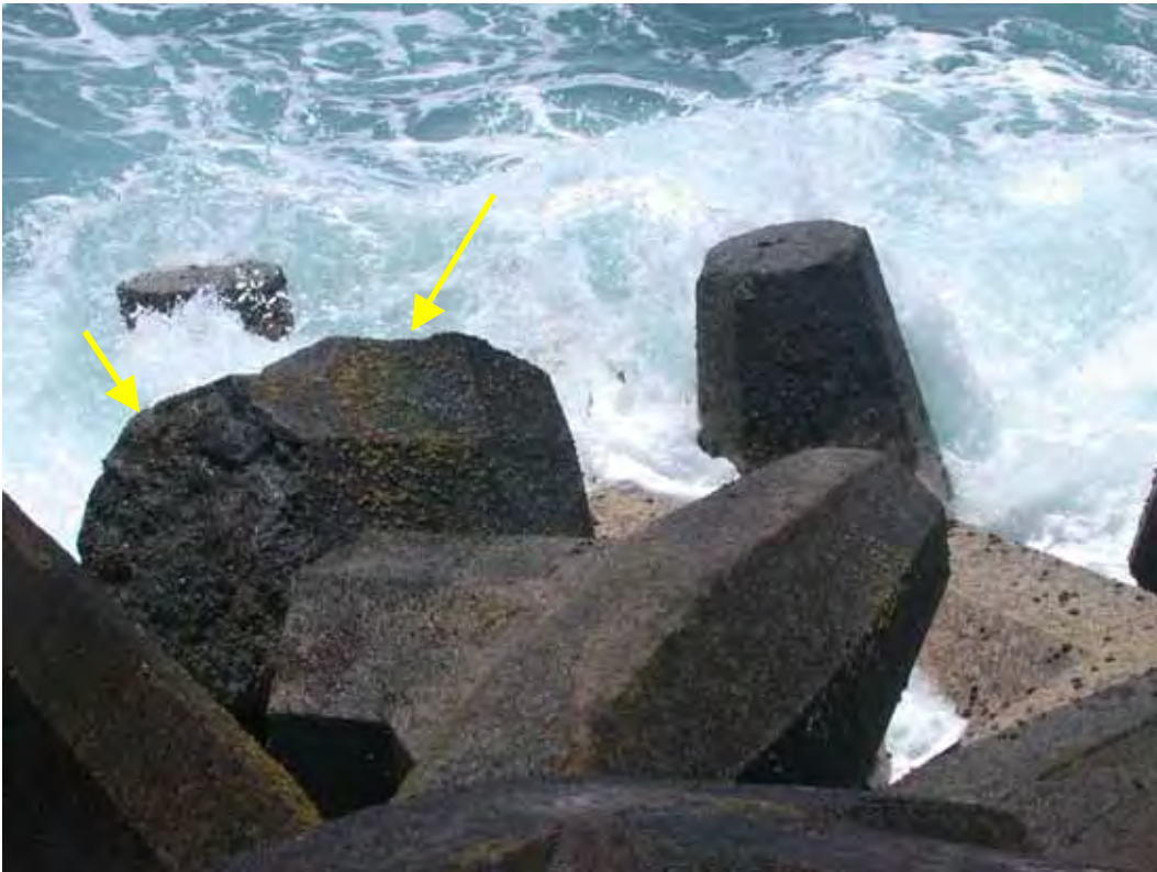
Figure D59. Damage location 79, sta 18+54, ocean side, rib #110, dolosse with multiple breaks.
