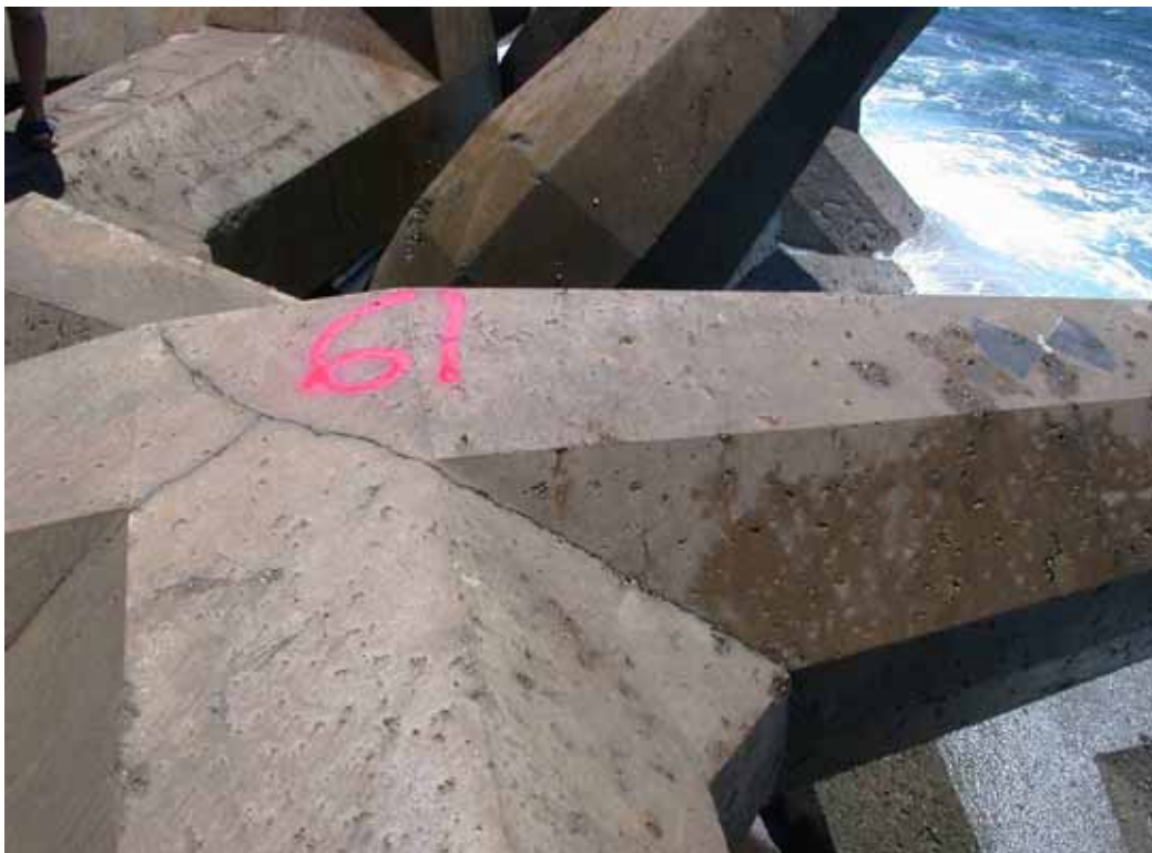
Figure D69. Damage location 93, sta 19+78, ocean side, rib #129, target dolosse cracked through fluke.
