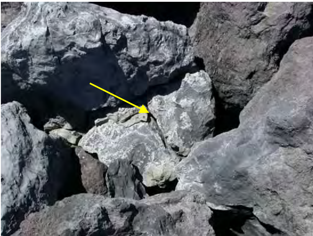
Figure C2. Sta 0+40, cracked armor stone.
