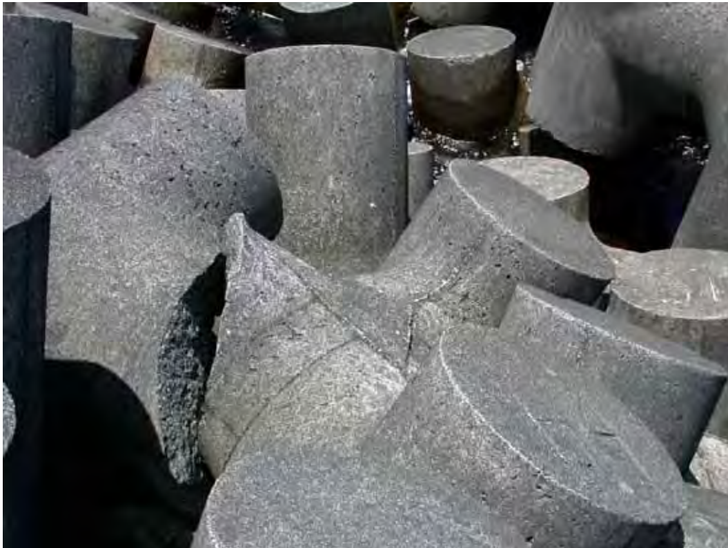
Figure A17. Damage location 17, sta 19+52, rib #143, tribar #64, broken leg.
