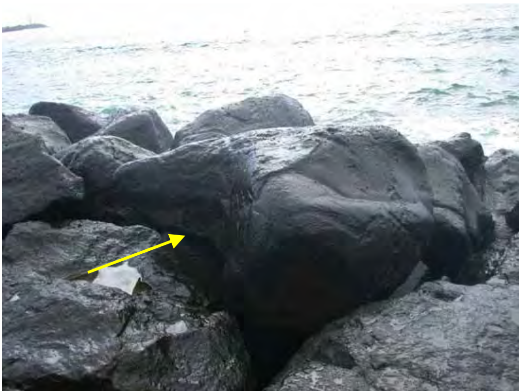
Figure D18. Damage location 17, sta 9+87, ocean side, perched armor stone.
