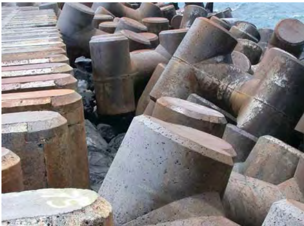
Figure B28. Damage location 37, sta 30+88 - sta 31+48, ocean side, rib #77 - #87, 10 ft separation of tribar from ribcap.
