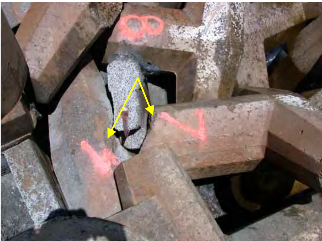
Figure B17. Damage location 20, sta 27+09, ocean side, rib #15, dolosse with shank-fluke break.
