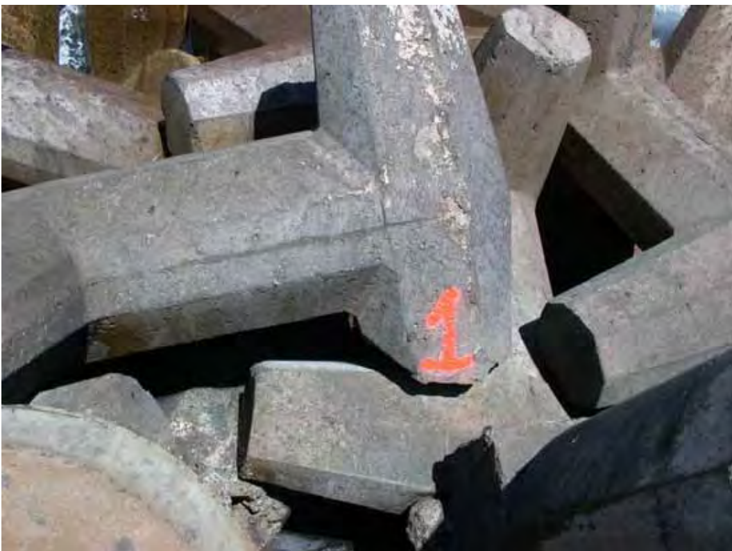
Figure B11. Damage location 14, sta 26+70, ocean side, rib #8, dolosse with fluke tip break.
