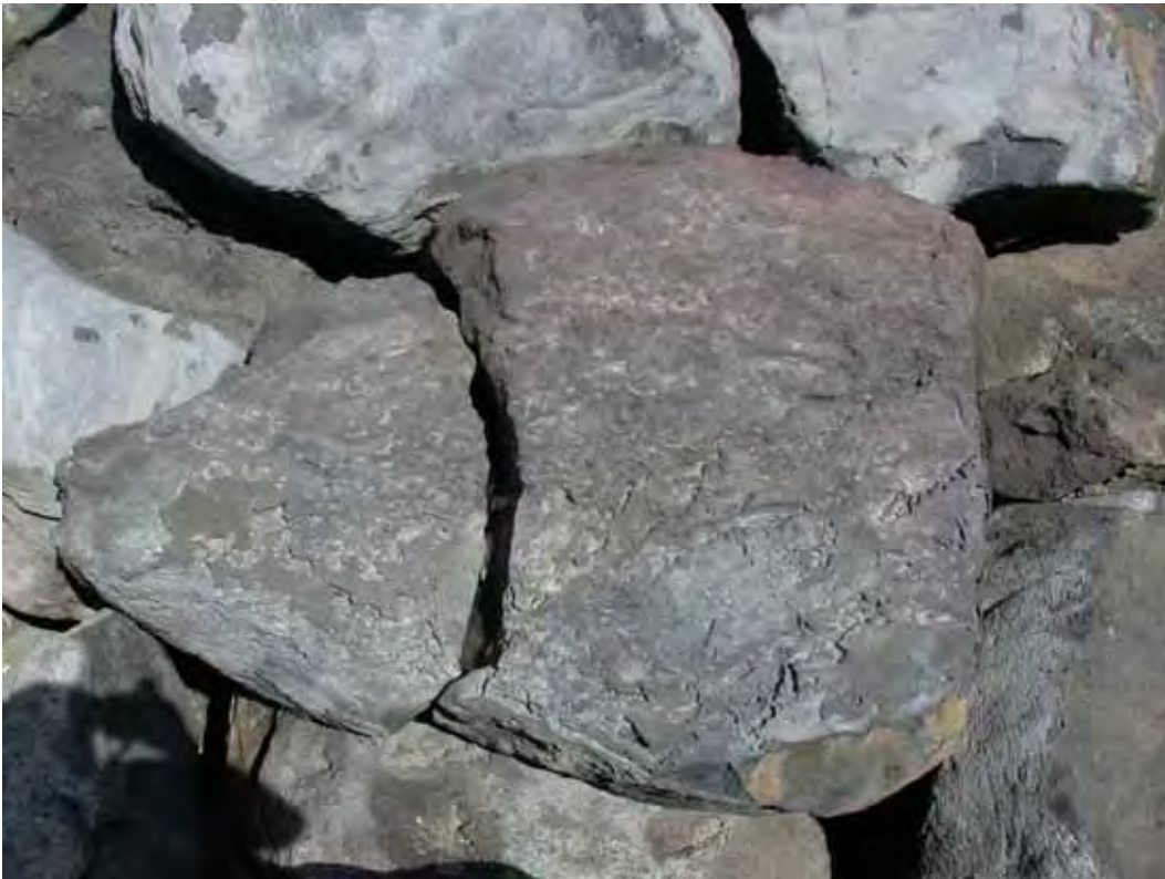
Figure B4. Damage location 9, sta 21+60, crest, broken armor stone.
