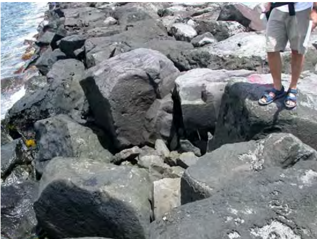
Figure A31. Damage location 31, sta 28+78, missing crest stone.
