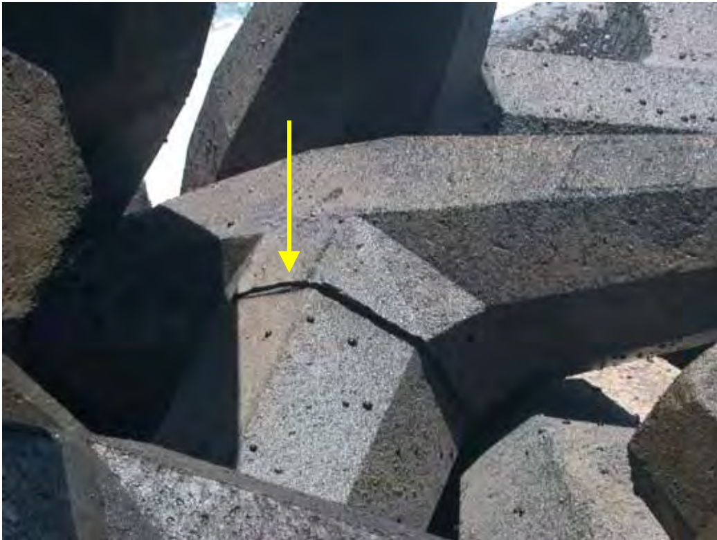
Figure D57. Damage location 75, sta 18+18, ocean side, rib #104, dolosse with shank break.
