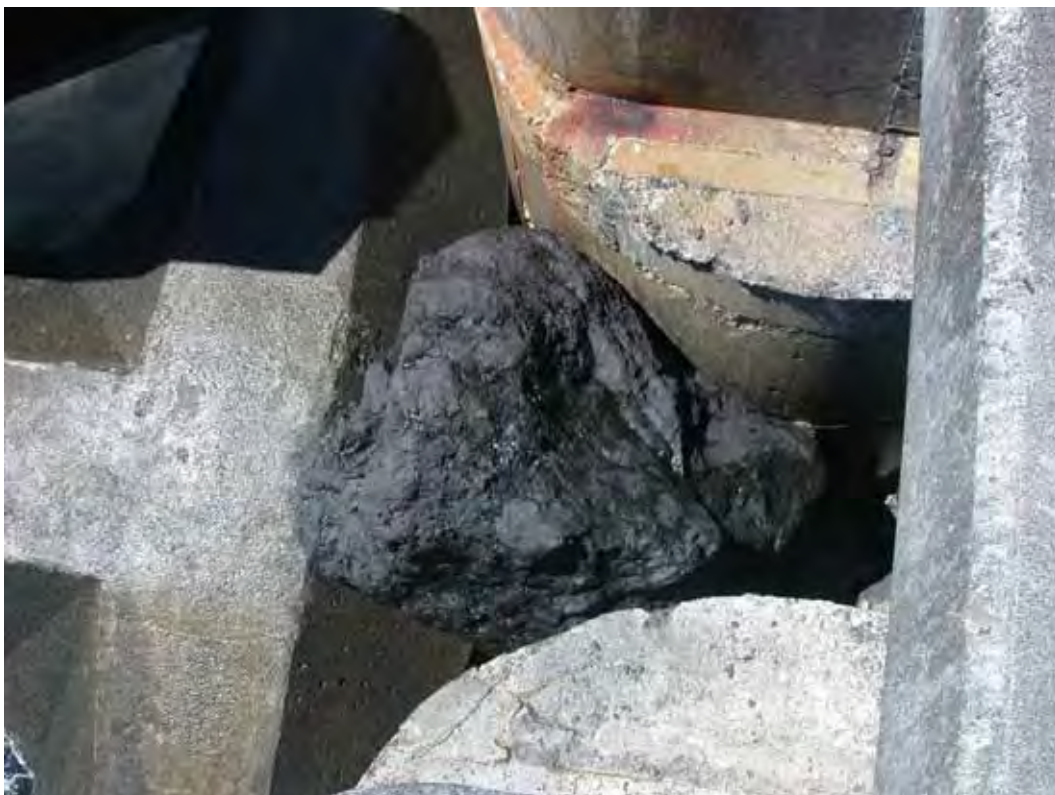
Figure C14. Displaced armor stone, tossed onto dolos.
