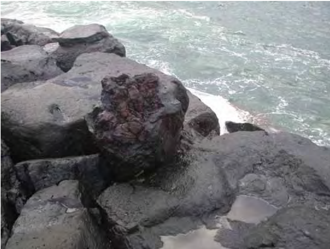
Figure A72. Damage location 86, sta 95+70, ocean side, flipped stone at hinge.
