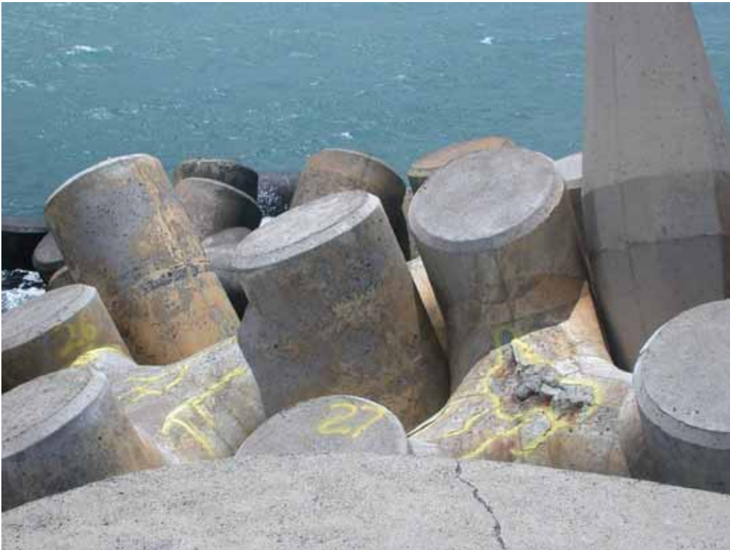
Figure B43. Damage location 58, harbor side of head, tribar with cracking and spalling.
