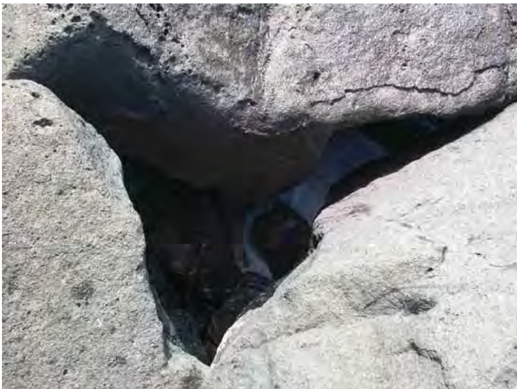
Figure A47. Damage location 51, sta 52+60, bridging.
