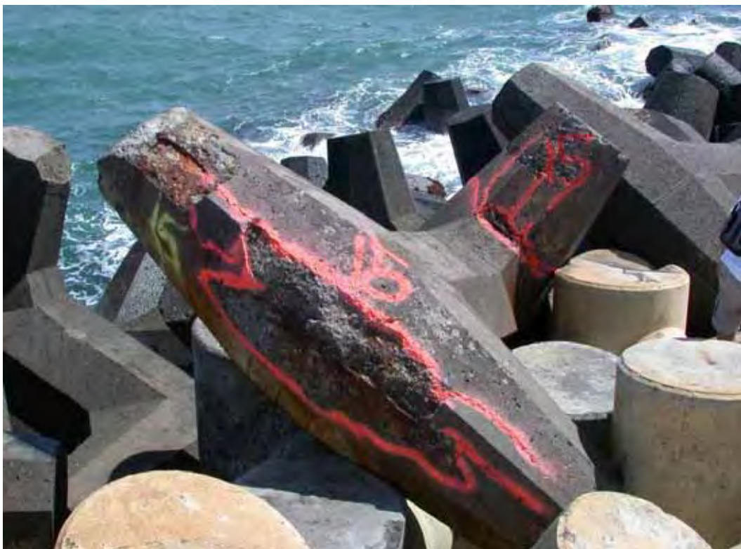
Figure B60. Damage location 23, sta 21+83, ocean side, spalling of dolosse and concrete rib cap.
