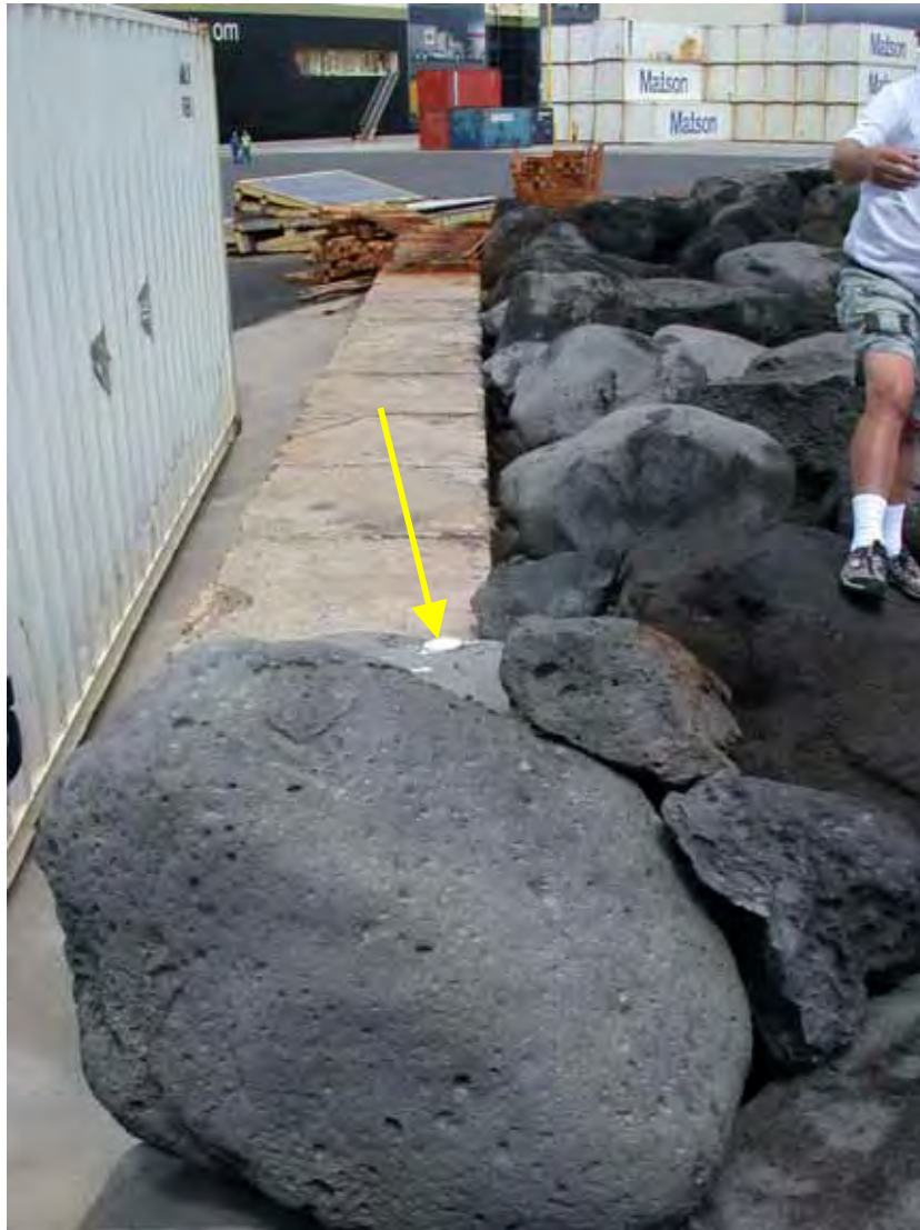
Figure B2. Sta 18+86, beginning of concrete wall adjacent to structure (marker shows 18+25).
