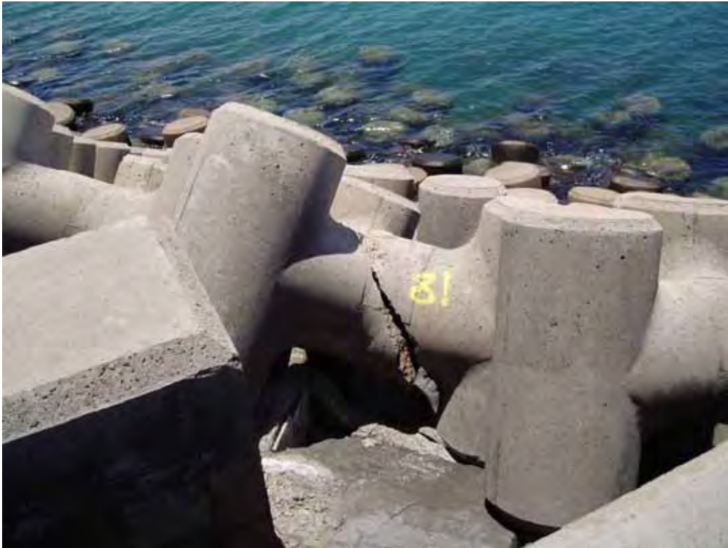
Figure B47. Damage location 4, sta 18+82, harbor side, rib #14, tribar with crack through center.
