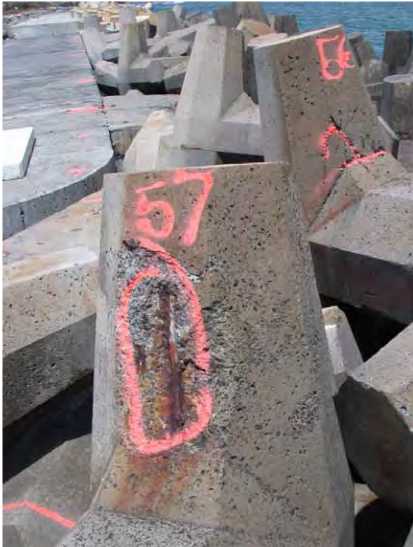
Figure B93. Damage location 71, 30 deg ocean side of head, dolosse with spalling and exposed rebar.
