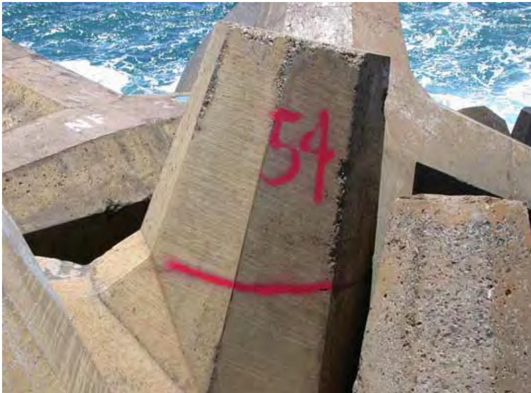
Figure D65. Damage location 87, sta 19+42, ocean side, rib #123, dolosse with crack through fluke, still intact.
