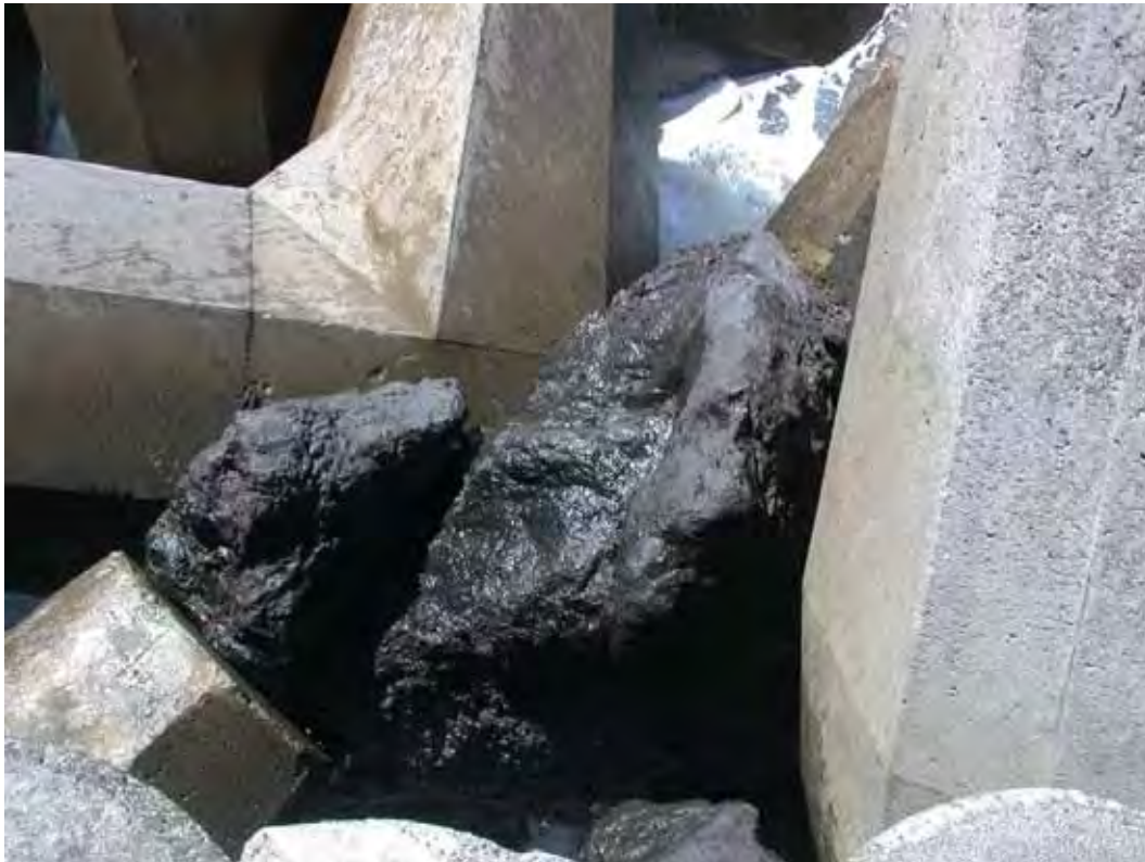
Figure C13. Displaced armor stone, tossed onto dolos.
