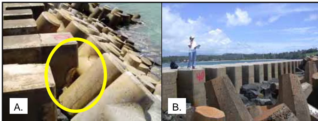
Figure 38. Evidence of armor stone subsidence.
