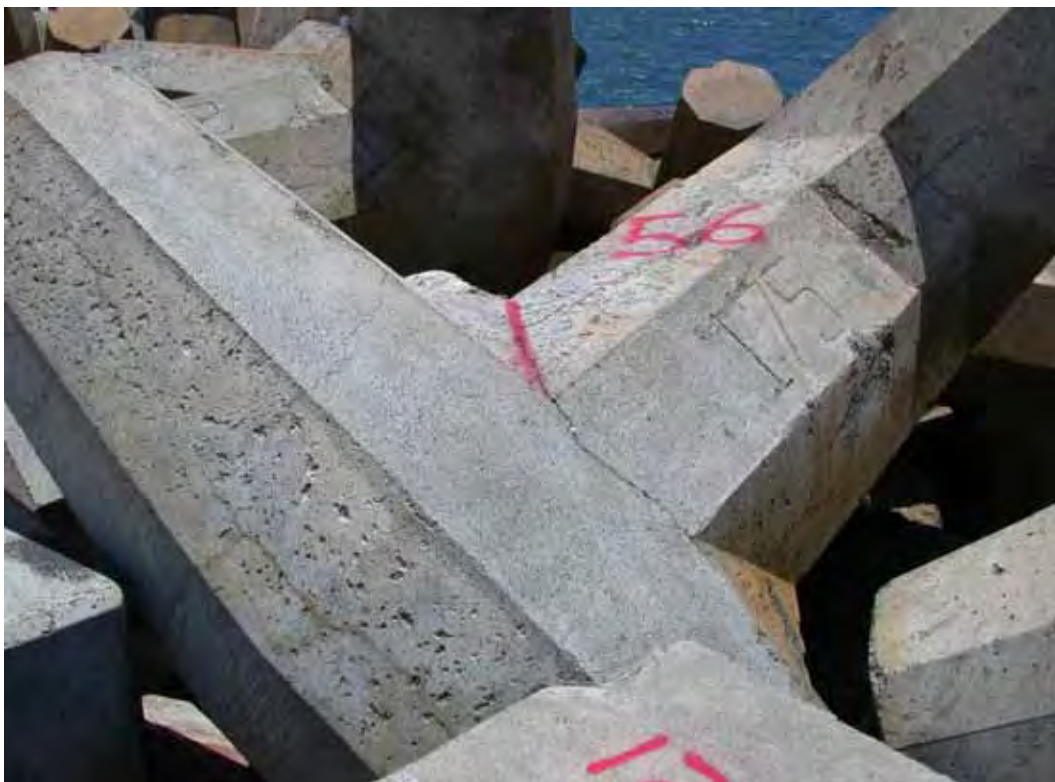
Figure D67. Damage location 89, sta 19+60, ocean side, rib #126, dolosse with shank-fluke crack, still intact.
