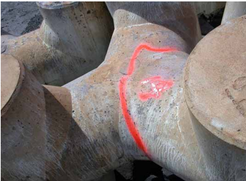
Figure B58. Damage location 20, sta 21+54 - 21+60, ocean side, rib #48-49, tribar with cracks through center.
