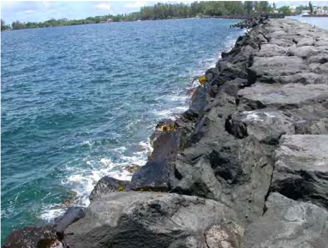
Figure A23. Damage location 22, sta 23 +40, ocean side, sharp drop.
