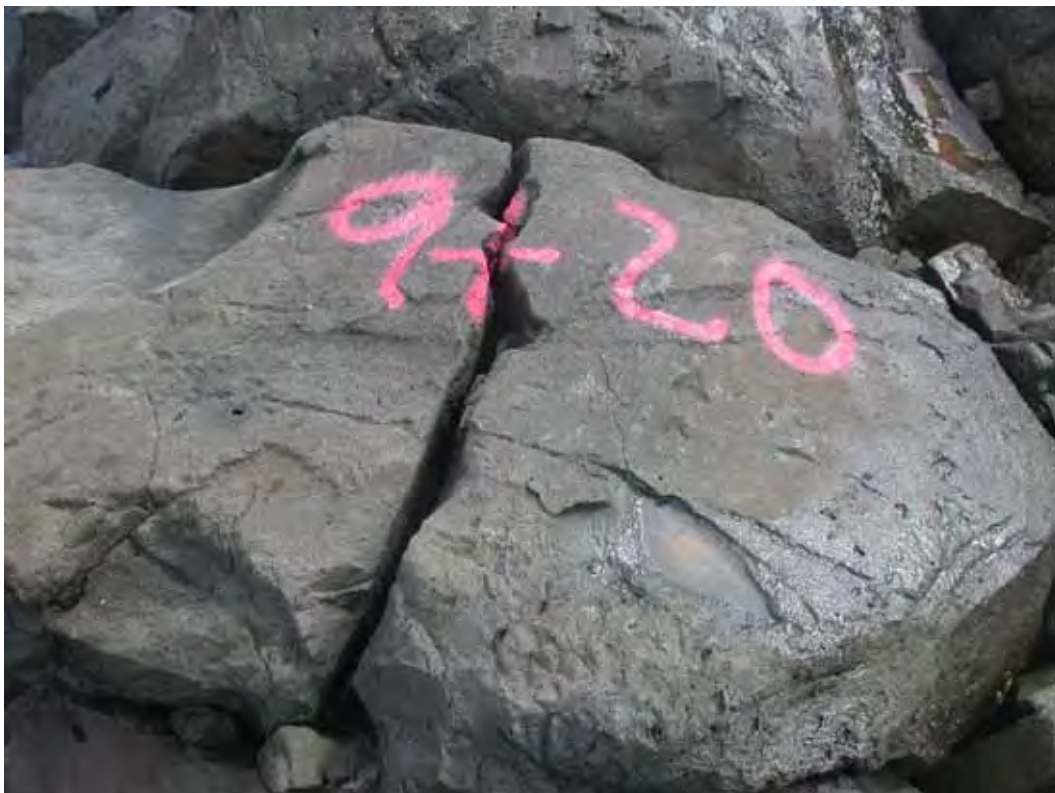
Figure D14. Damage location 13, sta 9+20, harbor side, cracked armor stone at hinge.
