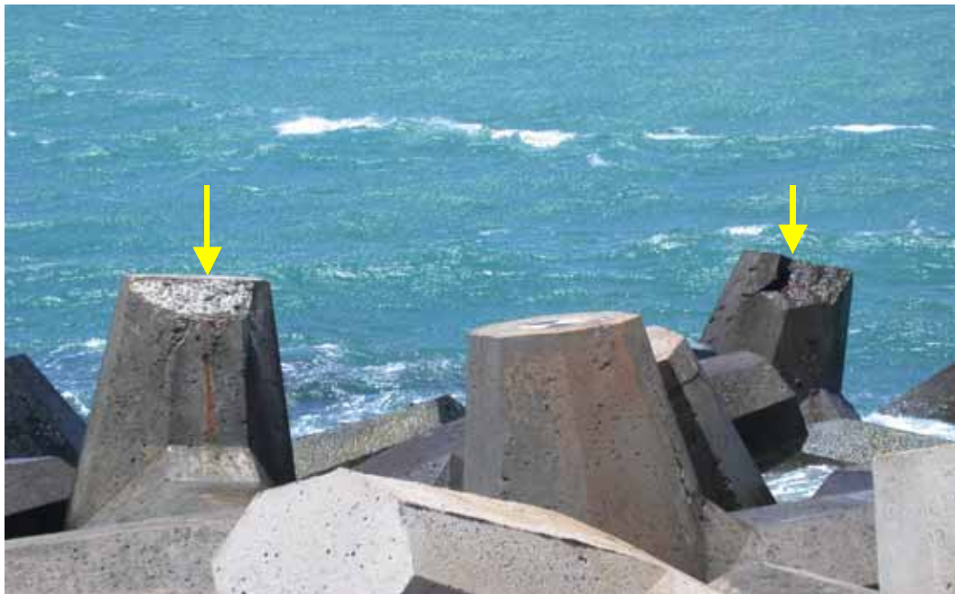
Figure B38. Damage locations 52 & 53, sta 33+82 and sta 34+09, ocean side, rib #126 and 129, dolosse with fluke tip breaks.
