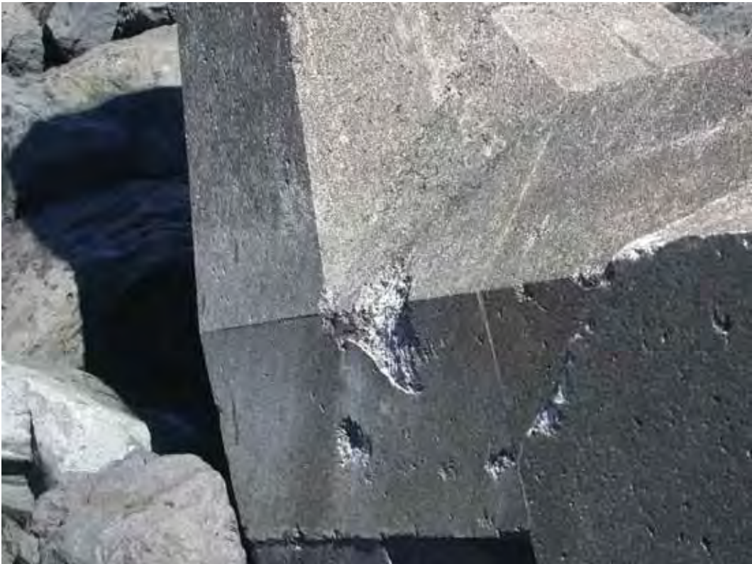
Figure C18. dolosse damage possibly caused by displaced armor stones.
