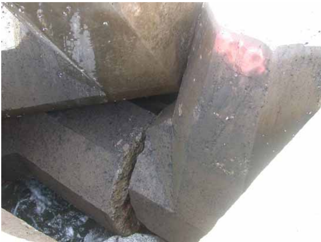
Figure B80. Damage location 49, sta 22+92, ocean side, dolosse with shank-fluke break.
