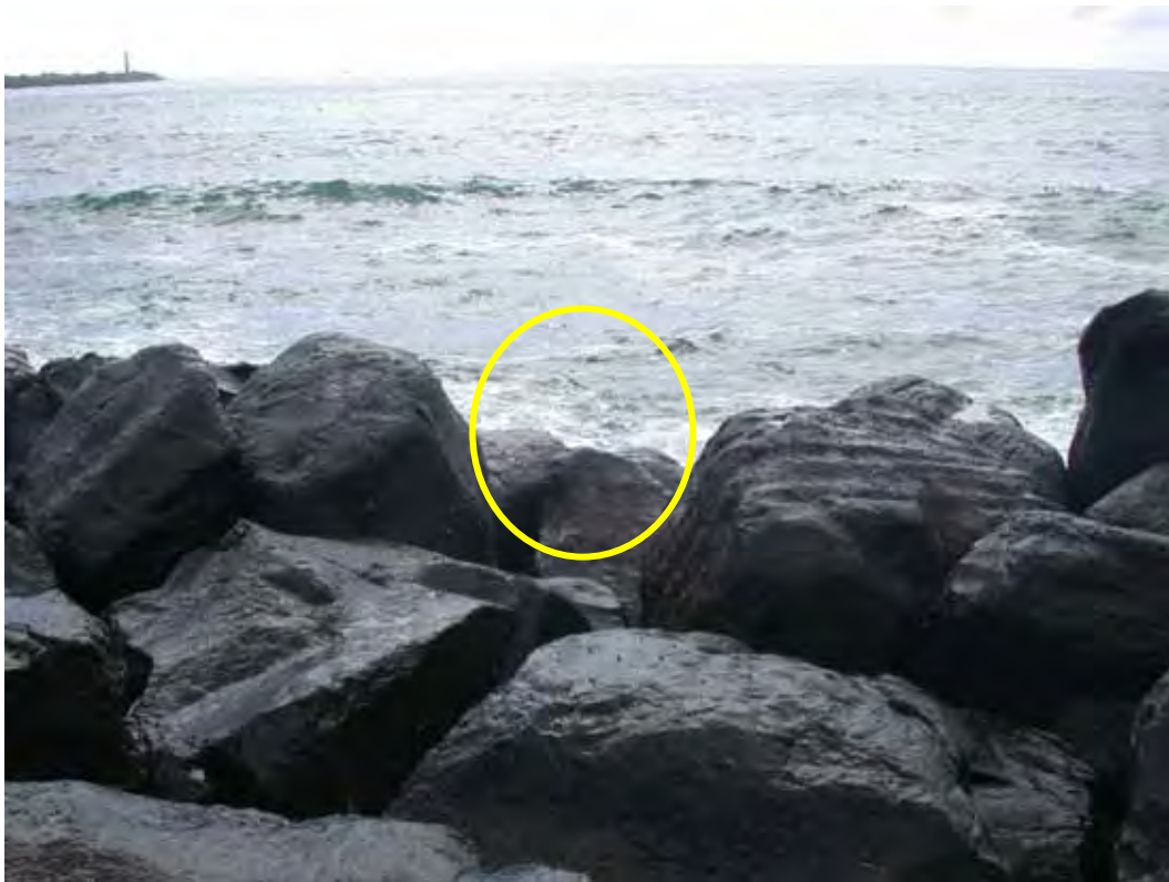
Figure D17. Damage location 16, sta 9+67, ocean side, void at hinge.
