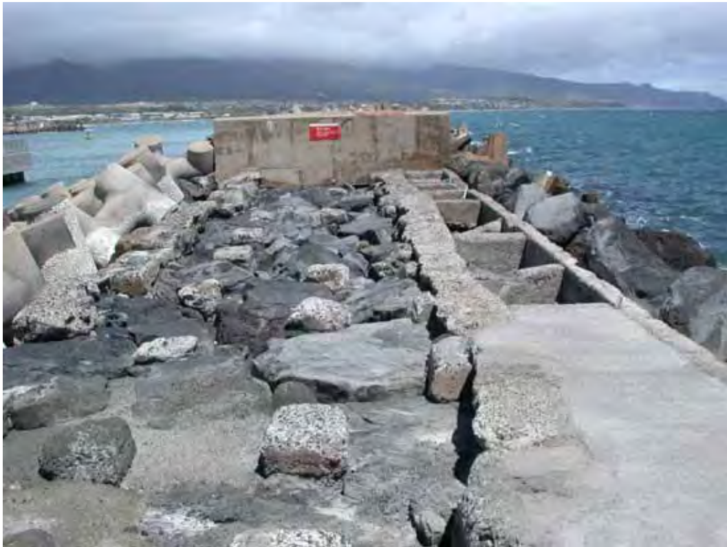
Figure B8. Sta 26+26, begin rib cap; extension of Pier 1 harbor side of breakwater.
