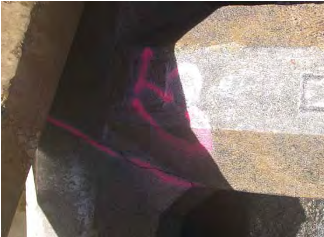
Figure D72. Damage location 97, sta 19+96, ocean side, rib #132, dolosse with fluke-shank crack.
