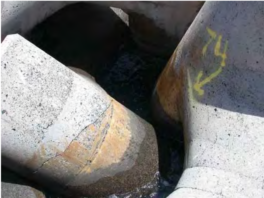
Figure B83. Damage location 52, sta 22+98, harbor side, cracked tribar.
