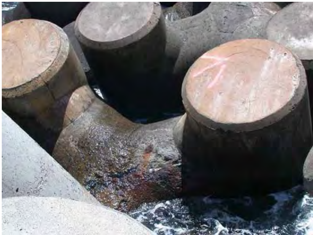
Figure B100. Damage location 85, 90 deg harbor side of head, tribar with spalling at center.
