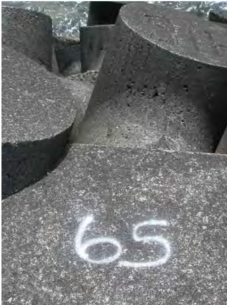
Figure A12. Damage location 14, sta 14+80, rib #65, tribar with broken leg.
