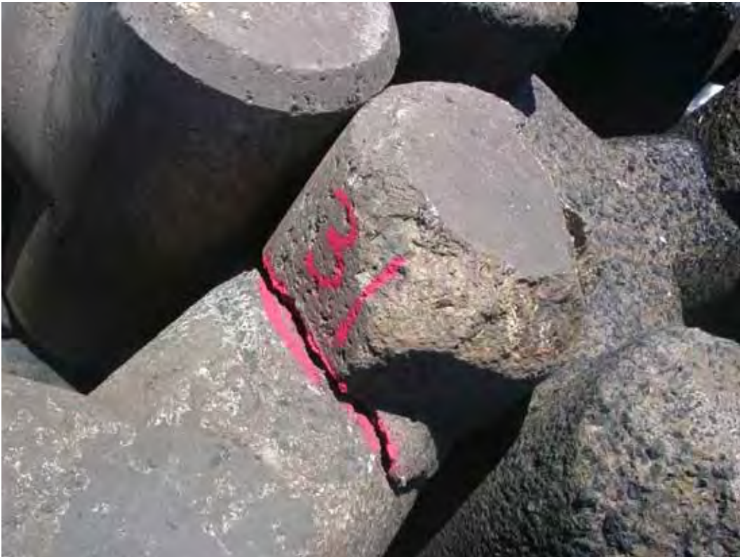
Figure D47. Damage location 64, sta 16+14, ocean side, rib #70, tribar with broken can.
