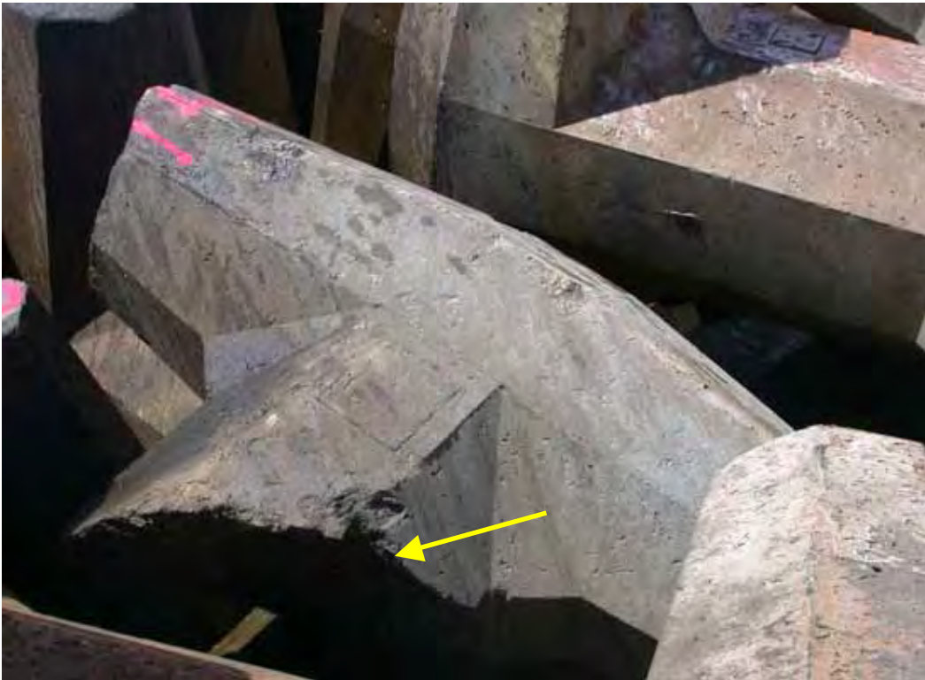
Figure D38. Damage location 44, sta 14+04, ocean side, rib #35, dolosse with mid-shank break.
