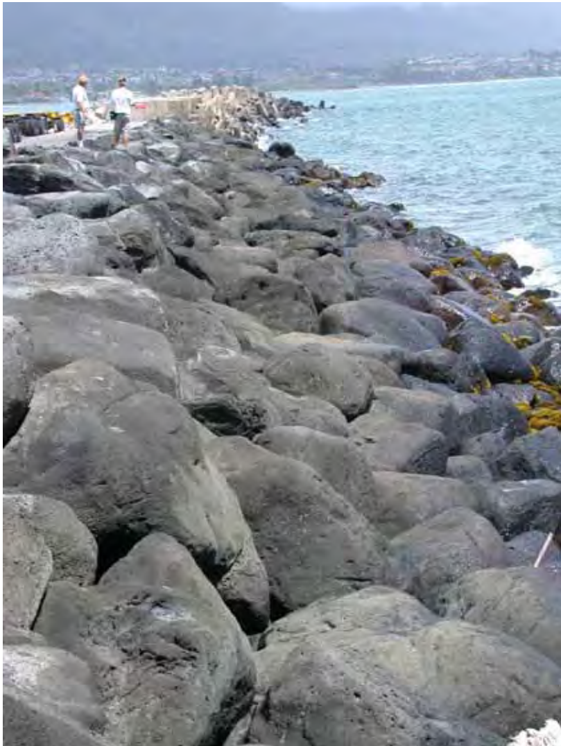
Figure B3. Damage location 8, sta 19+00-21+00, ocean side, side slope flattening.
