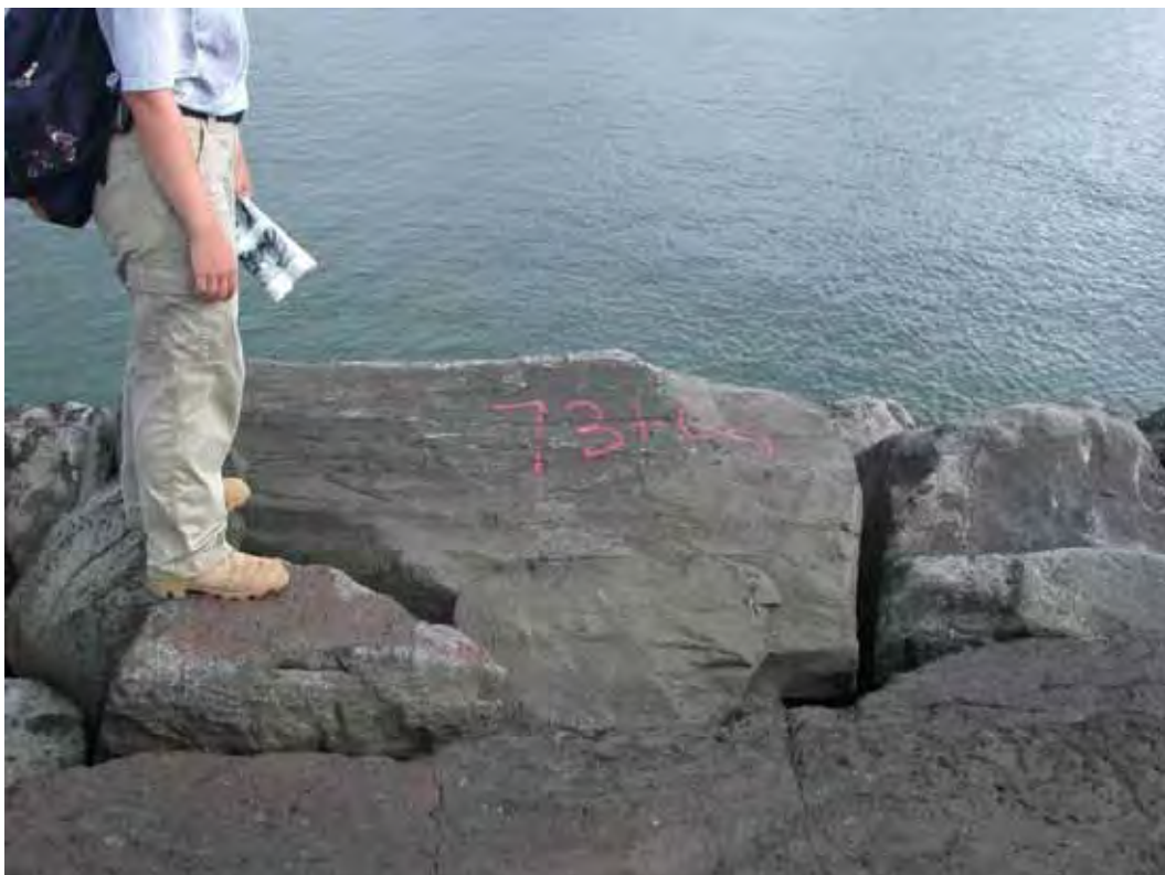
Figure A62. Damage location 71, sta 73+00, harbor side, slight settling of crest.
