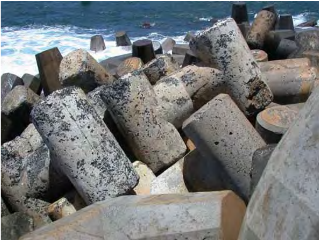
Figure D80. 90 deg harbor side of head, four tribars that are extremely abraded and have coral growth, appear to have been moved from below waterline to harbor side slope.
