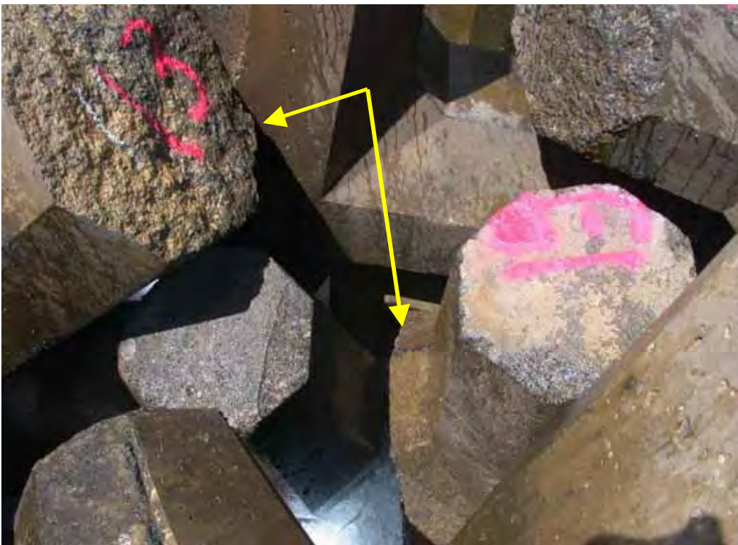
Figure D37. Damage location 43, sta 14+04, ocean side, rib #35, dolosse with mid-shank break.
