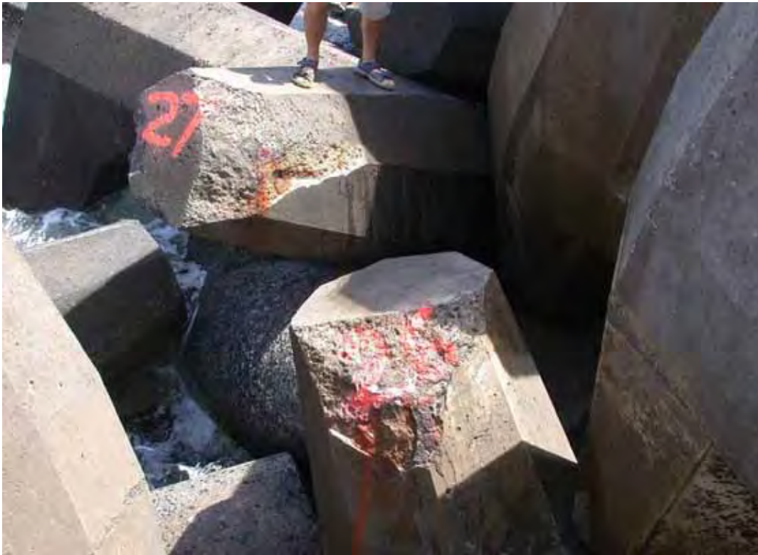
Figure B69. Damage locations 33 & 34, sta 22+35, ocean side, two dolosse with fluke tip breaks.
