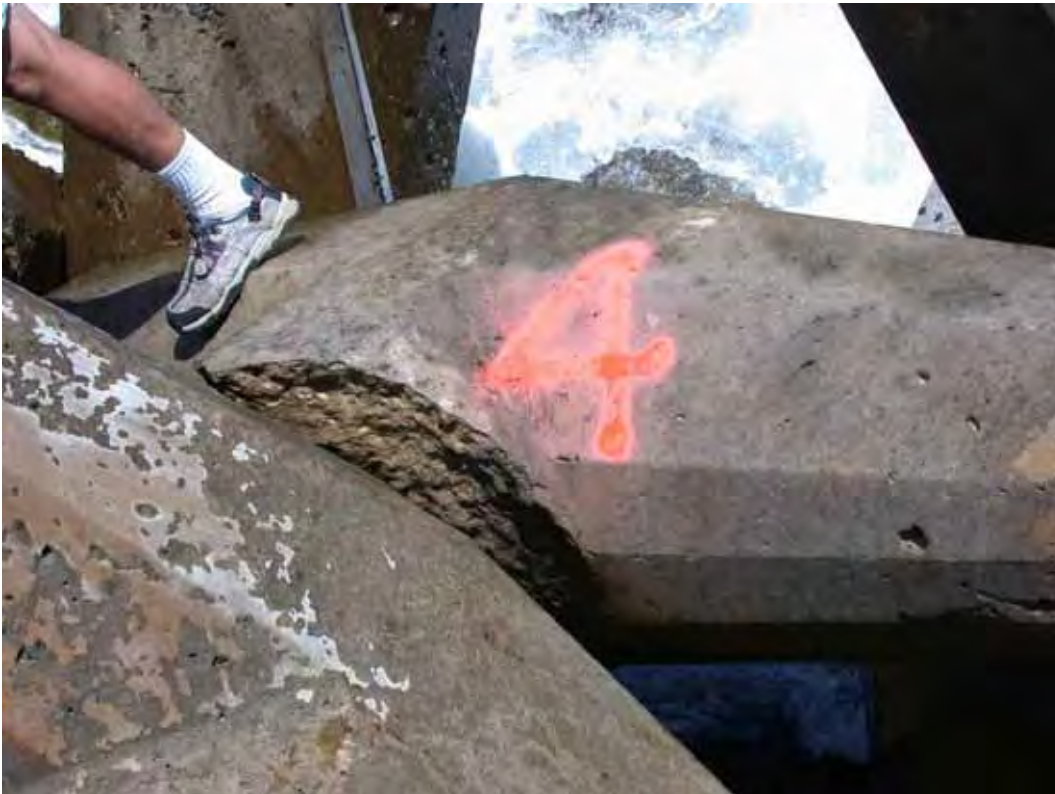
Figure B14. Damage location 17, sta 26+97, ocean side, dolosse with shank-fluke break.
