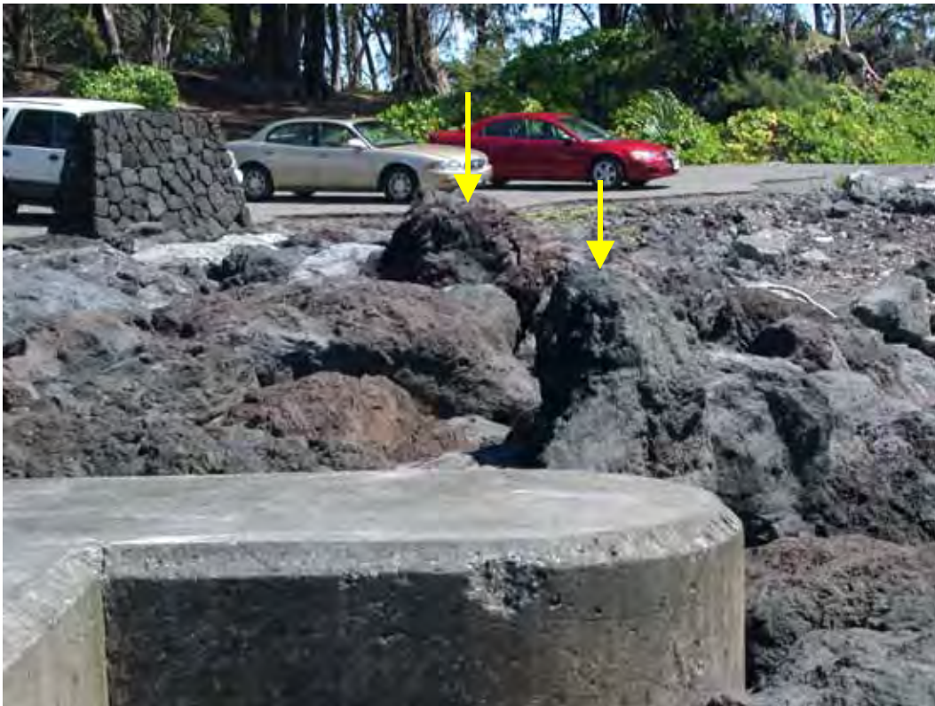
Figure C6. Oceanside, flipped armor stones.
