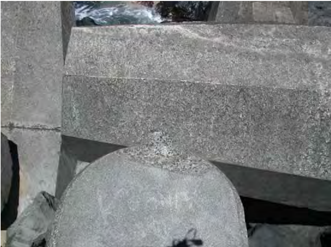
Figure C17. Rib damage possibly caused by displaced armor stones.
