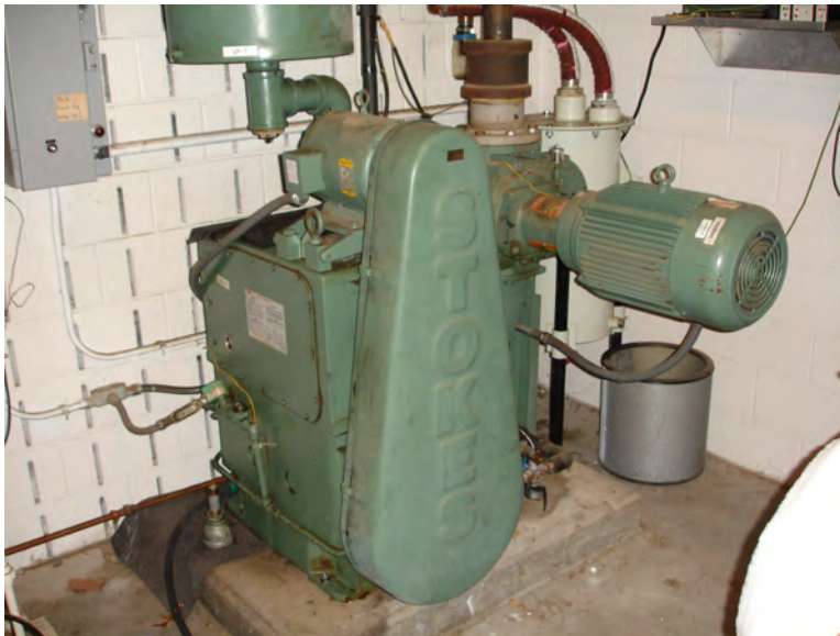
Figure F.19: Stokes Microvac vacuum pump
