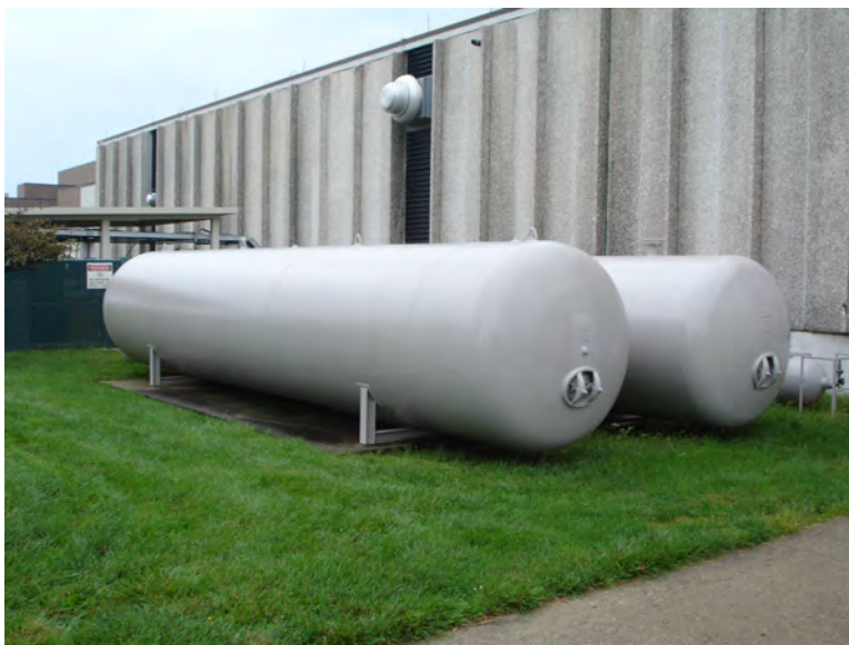
Figure F.5: High pressure and vacuum chambers
