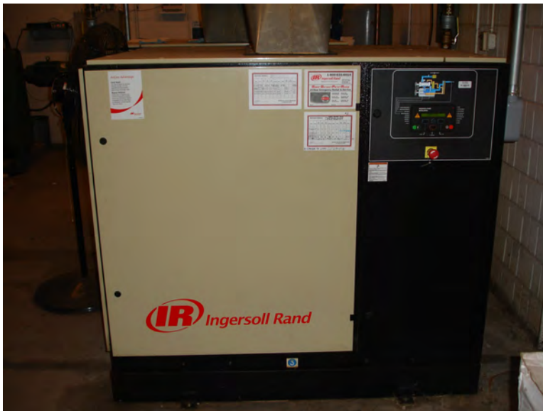
Figure F.3: Ingersoll Rand rotary screw compressor
