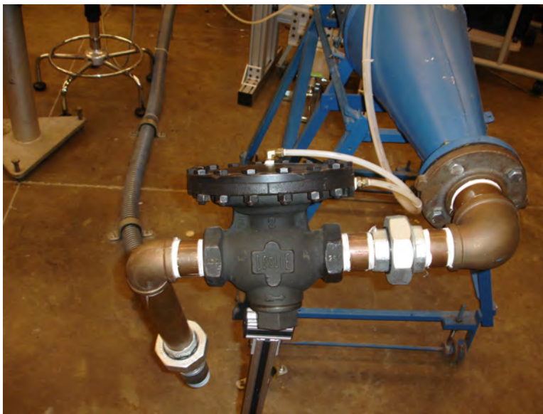
Figure F.10: Leslie air-loaded pressure reducing valve
