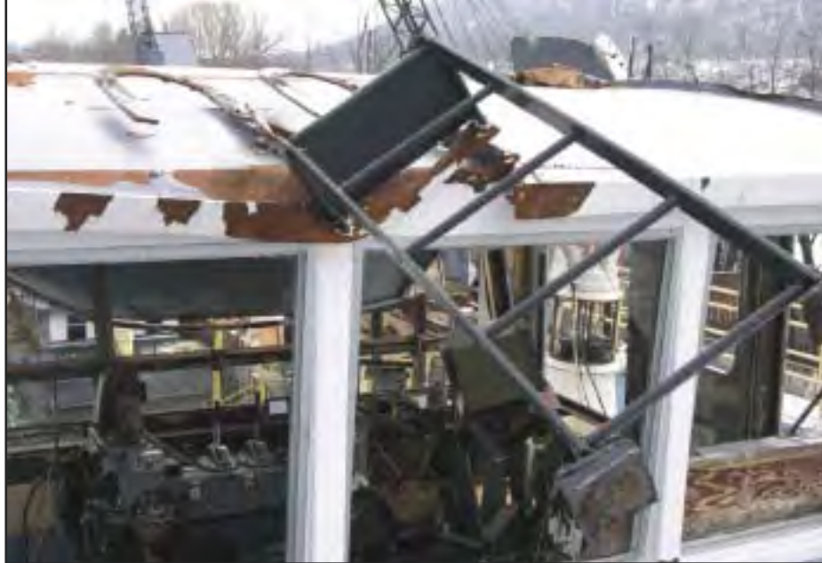
Post-casualty photograph of the ladder leading to the top of the pilothouse used by the deckhand to secure himself and the captain until they were rescued.
