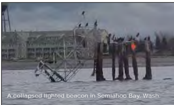
A temporary lighted buoy marks the wreckage of a lighted beacon, which was damaged after a vessel collision.
