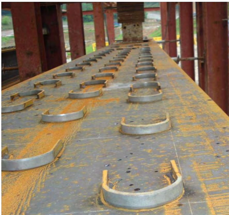
Figure 22. Horseshoe shear connectors installed on the top flange of the pre-flex beam.
