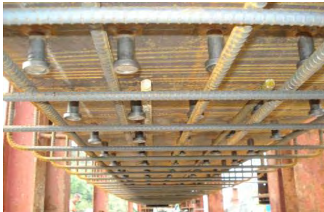
Figure 2. Bottom flange encasement of pre-flex beam under construction.
