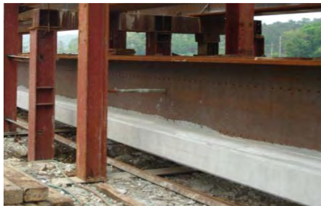
Figure 3. Pre-flex beam with cast concrete at bottom flange ready for release stage.
