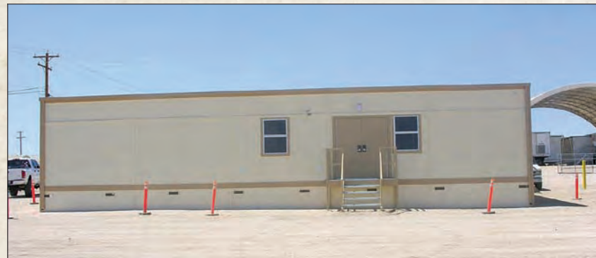
An exterior view of MCOTEA's facility at Camp Wilson
