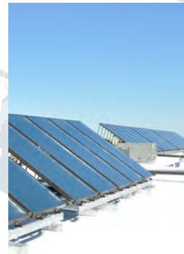
Rooftop Solar Array for Pool Heating
