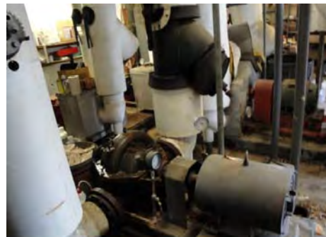
Two-pipe HVAC system in building SC-1 of the Joint Forces Staff College, Naval Support Activity, Norfolk, Virginia. Photo taken by DoD Office of Inspector General
