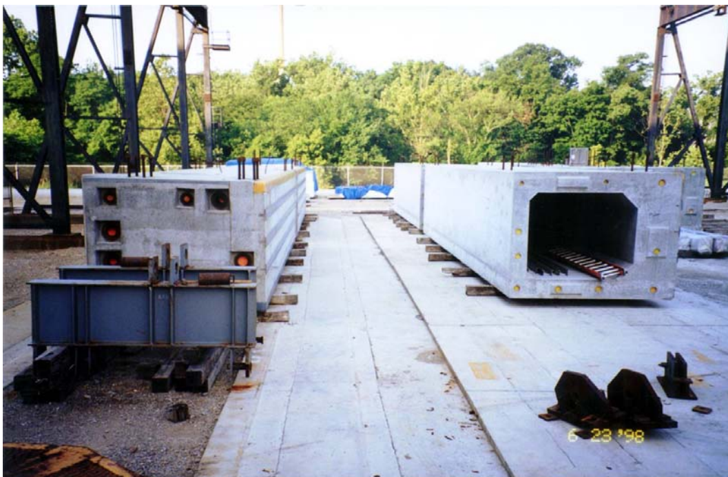
Figure 1.8 End view of the match-cast guide wall box beams at the fabrication yard (courtesy of Huntington District)
