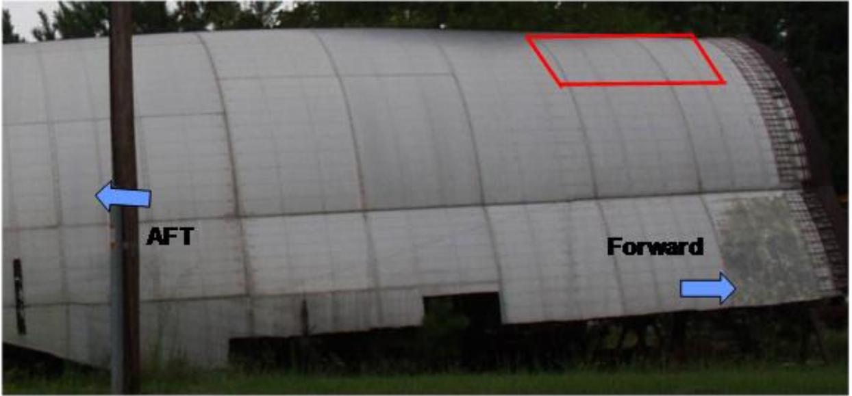
Figure 27. Side View of X997 with section to be removed in red
