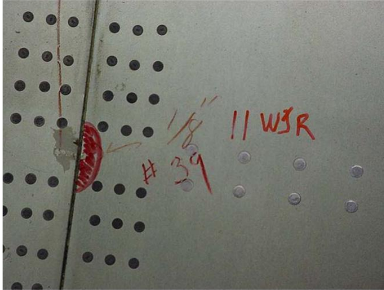
Figure 24. Cracking Found on A/C 70-0453
