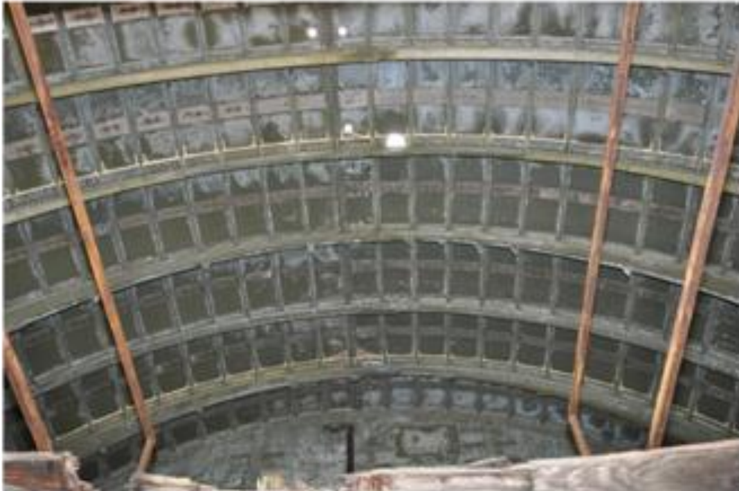
Figure 29. Interior View of X997
