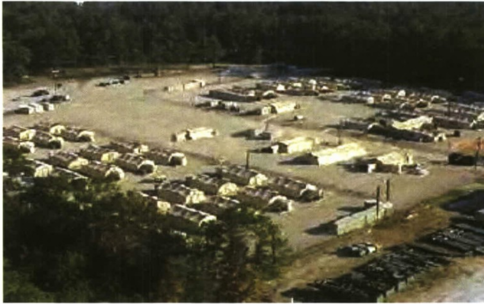
Figure 7. Example of a Base Camp
