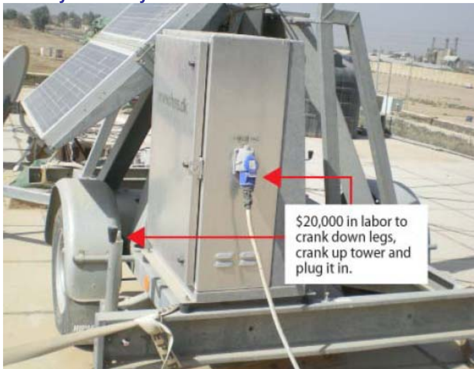
Figure 4—Anham, through Knowlogy, Billed $20,000 for Installation of a “Plug and Play” Voice System
