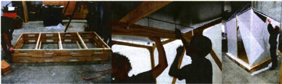
Figures 12a-c. Refinements in prototype 4 included a more functional base (a, left), interlocking, friction-held joints (b, center), and semi-rigid cladding of corrugated polypropylene (c, right).
