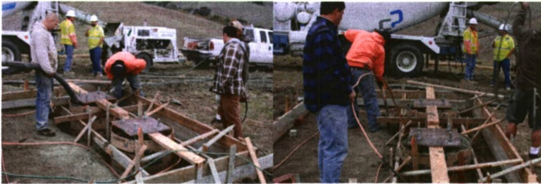
FIGURE 10: POURING OPERATION FOR THE TURBINE FOUNDATION.
