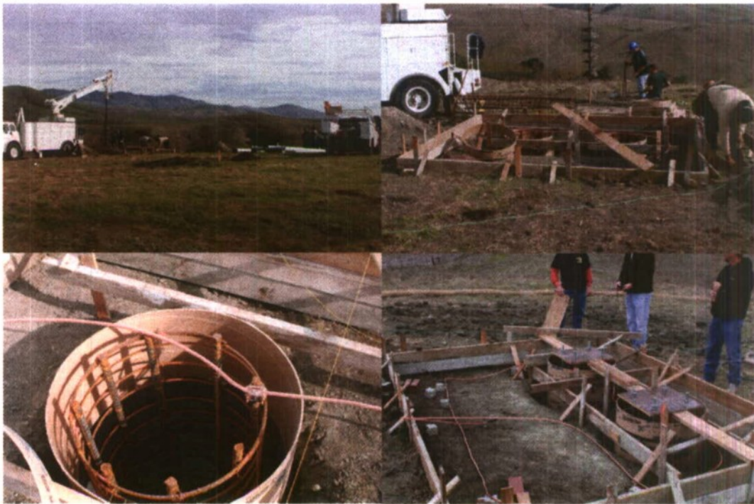
FIGURE 9: FROM TOP LEFT, CLOCKWISE: CAL POLY FACILITIES SERVICES EXCAVATING GROUND FOR THE TURBINE FOUNDATION; CONSTRUCTING FORMS; WORKING ON THE MAIN PAD (NOTE THE COPPER WIRE SURROUNDING THE PAD AND CAISSONS, PROVIDING LIGHTNING PROTECTION TO THE TURBINE); CAISSON CAGE
