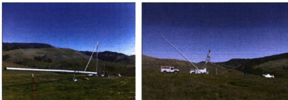
FIGURE 14: FINAL TOWER ASSEMBLY AND TILT-UP TEST. NOTE THE TRUCK AT THE RIGHT OF THE LOWER PICTURES, WHICH PROVIDES THE SOLE MOTOR FORCE FOR TILTING UP THE TOWER.
