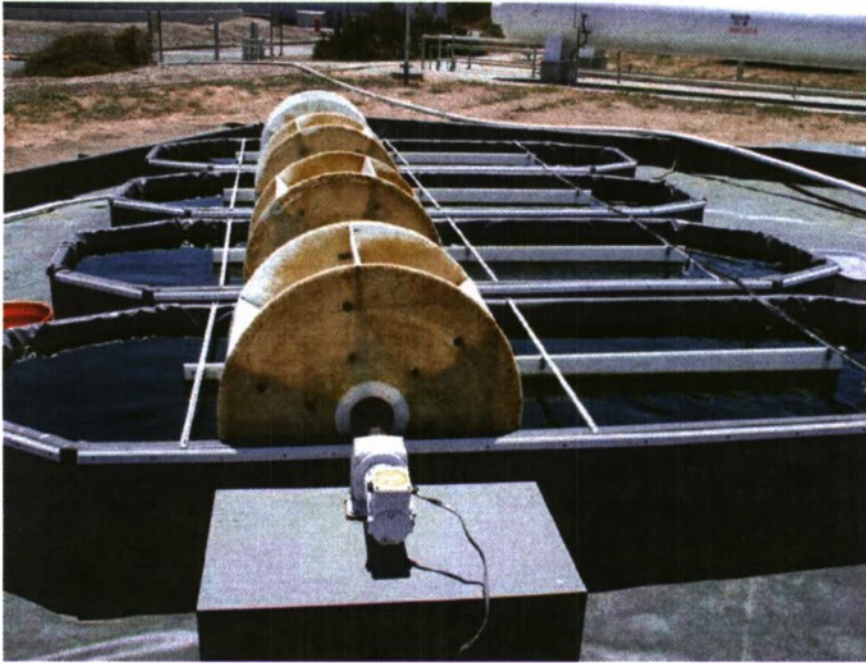
Figure 6: Post-construction photograph of ponds and paddle wheel motor assembly.
