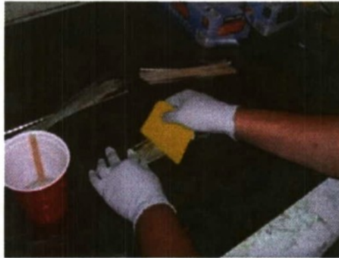
Figure 5 - "Wet Layup" Technique
