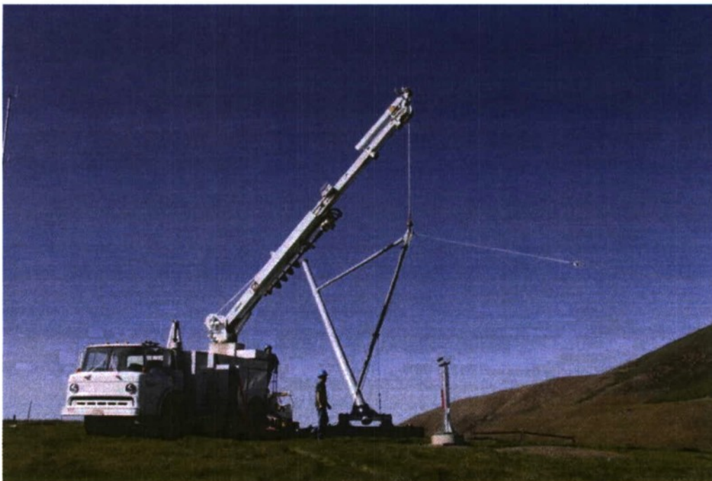
FIGURE 13: TEST OF TOWER TILT-UP OPERATION, PRIOR TO FINISHING TO THE ASSEMBLY OF THE UPPER TOWER SECTION.
