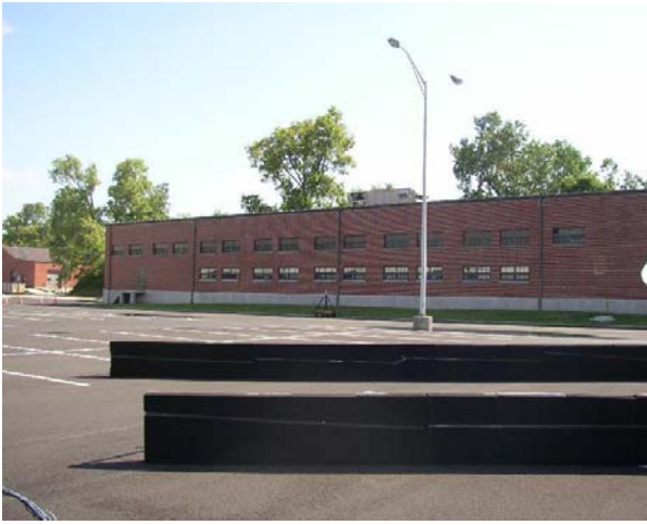
Fig. 2. The reflecting wall as seen from the transmitter. Absorber fences are positioned to mitigate ground bounce interference. The light pole intercepts some energy on the right side on the transmit beam.
