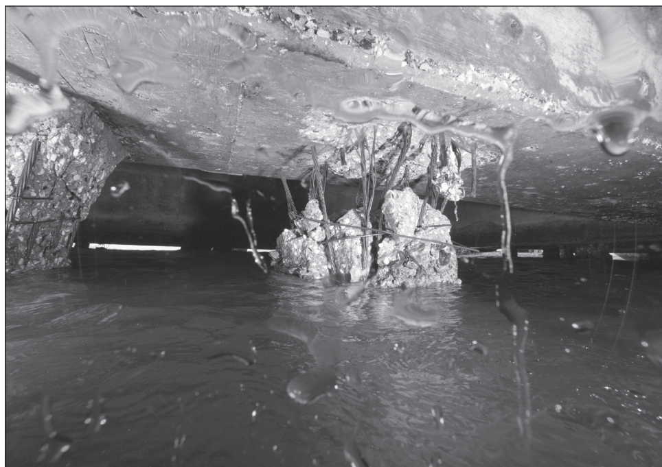
Divers found many severely damaged piles like this one.
