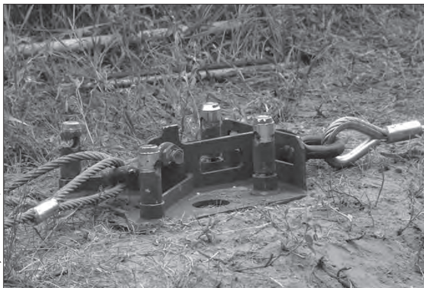
This close-up shows the main component of the new "thrust and shore guy" cable system used to anchor the IRB installed on the Missouri River.
