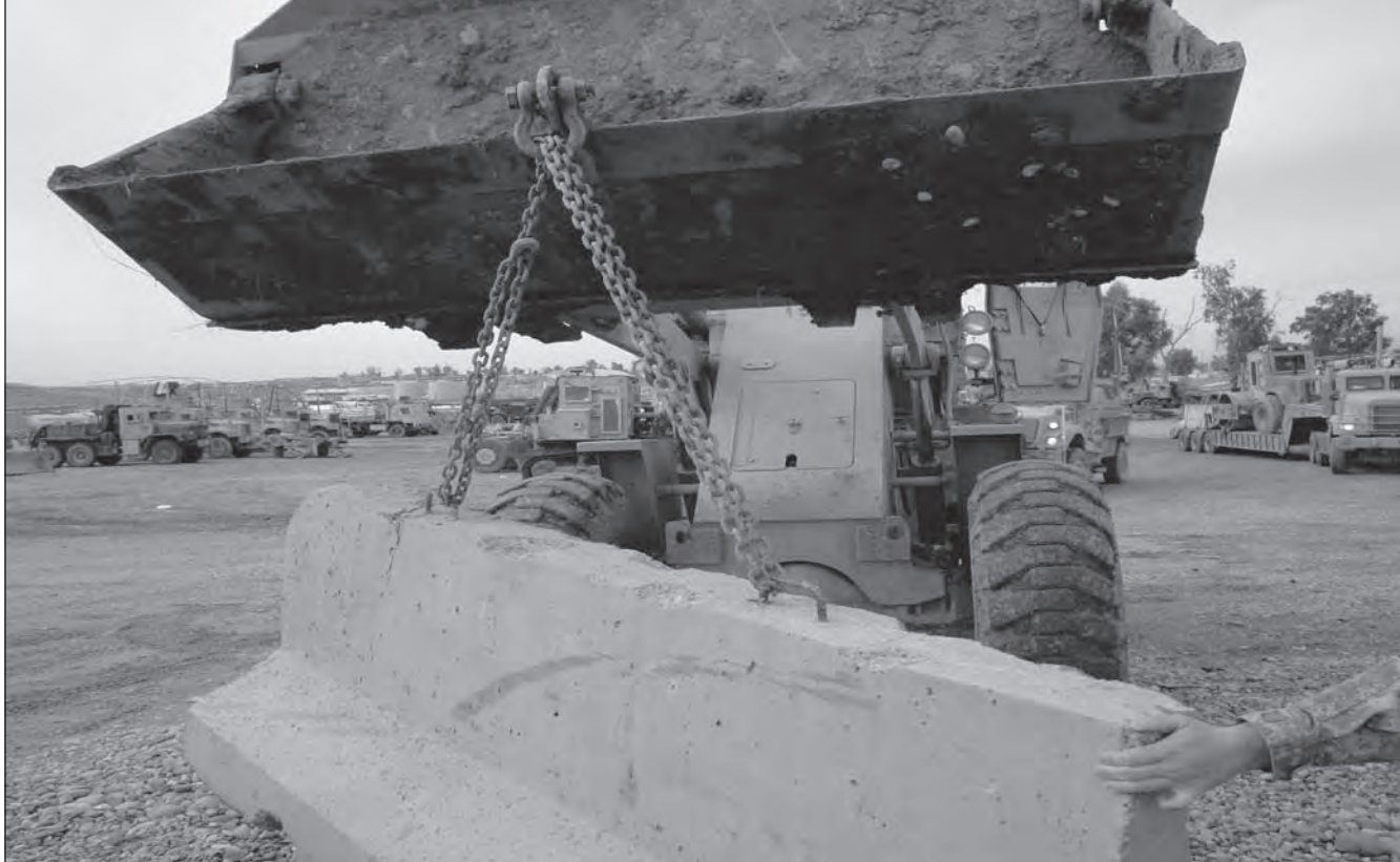
This is one of the many ways to use a chain to lift a Jersey barrier, as demonstrated by the 1313th Engineer Company in Mosul, Iraq.
