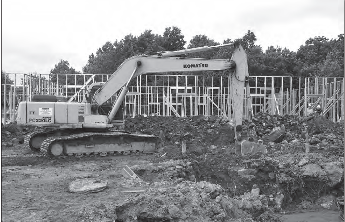
Crews work on trenches for geothermal wells, part of the heating and cooling system at the Fort Drum, New York, child development center.
