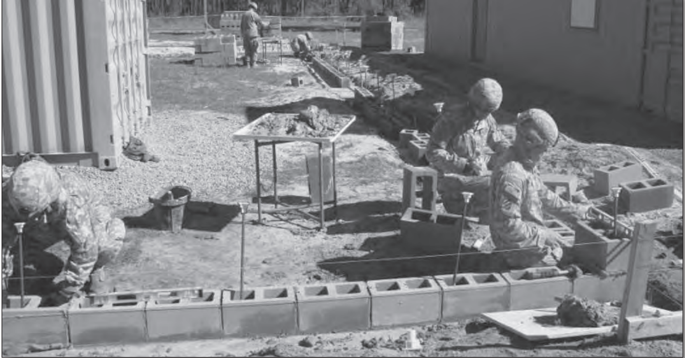
Soldiers from the 92d Engineer Battalion lay the first course of a concrete masonry unit wall.
