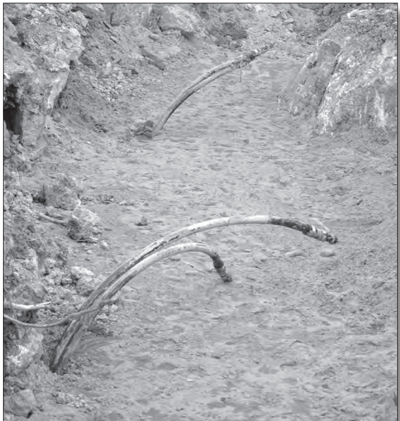
Pipes are installed as part of geothermal wells during construction of the Fort Drum child development center.
