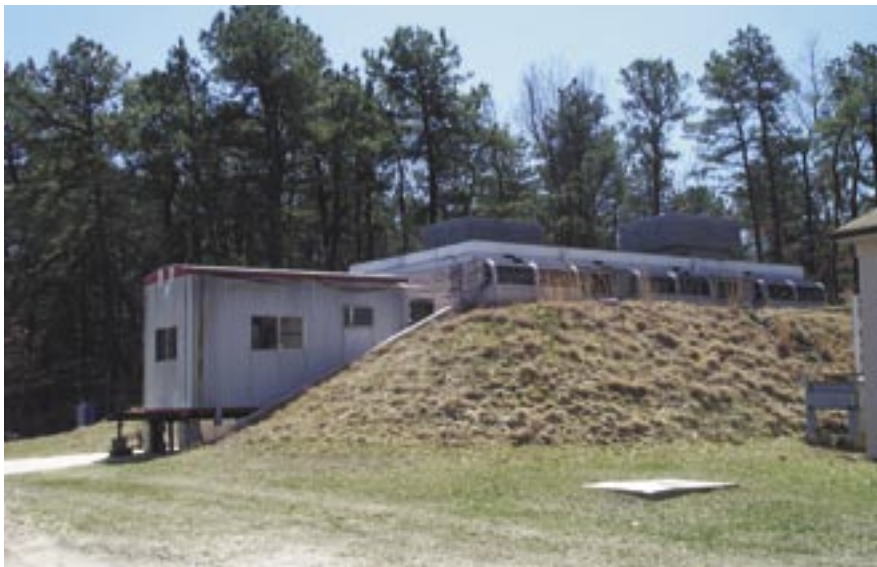
Figure 3. Pressure Fire Modeling Facility: the surrounding building and data acquisition trailer
