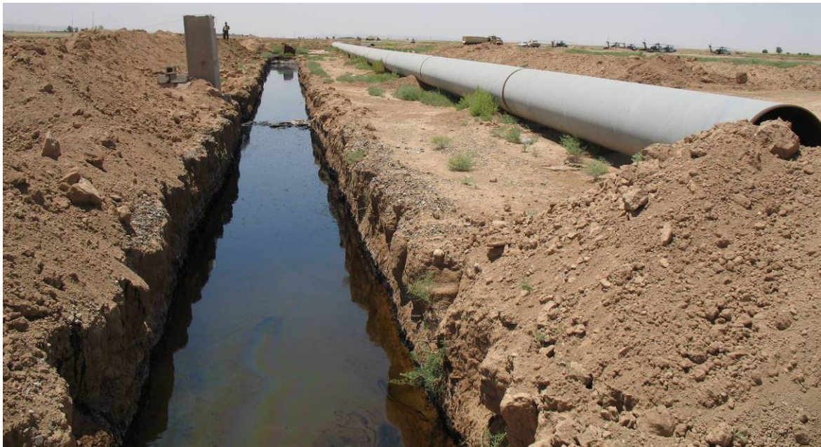
Site Photo 14. Welded pipe string and excavation at Zegeton Canal (Courtesy of IRMO - May 06)
