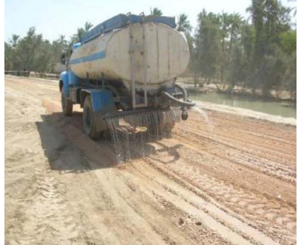
Site Photo 5. Watering the sub-base. (Photo provided by USACE)
