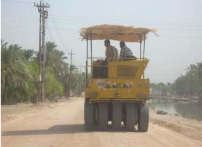
Site Photo 4. Rolling operations to compact sub-base. (Photo provided by USACE)
