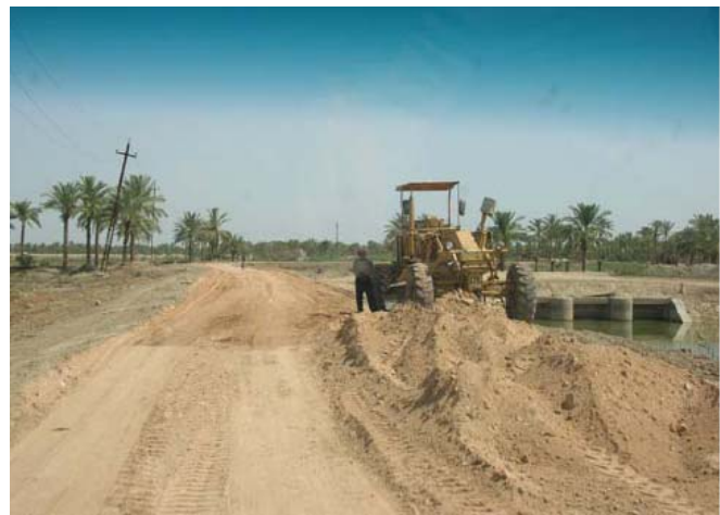
Site Photo 2. Fill material being leveled. (Photo provided by USACE)
