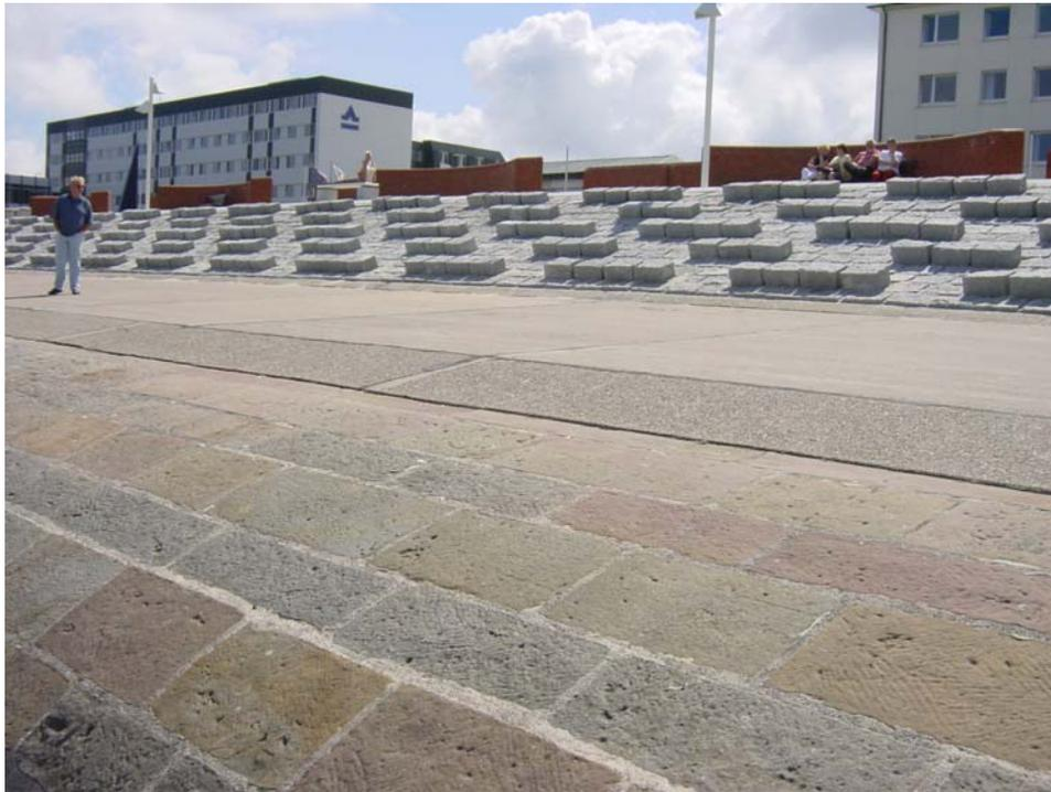
Figure 32. Illustrative photograph showing the use of discontinuous roughness elements (Photo Courtesy of Prof. Holger Schüttrumpf).
